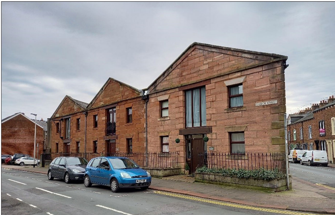
Figure 19: The Bonded Warehouse on Lower Church Street, the original warehouse of 1842 is on the right, the two bays to the left had been added by 1900 (© Historic England, photograph: Fiona Wooler, 2021)
