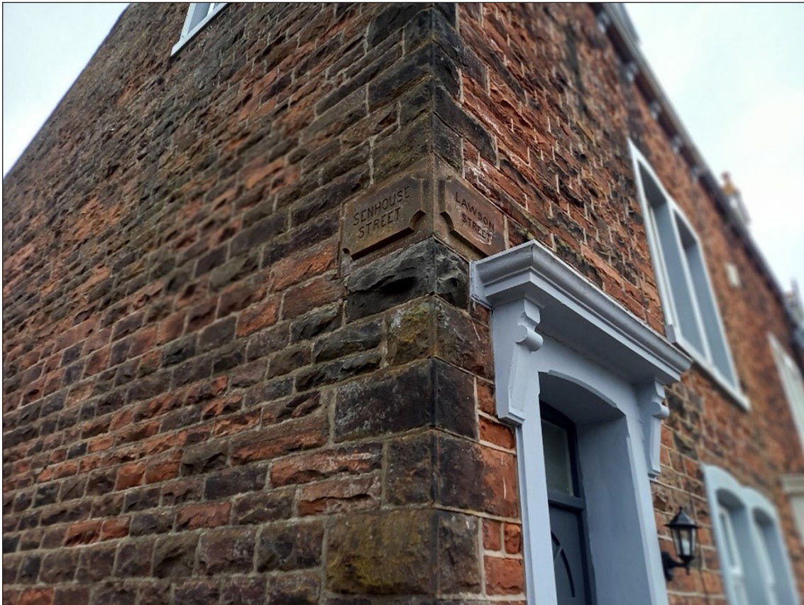
Figure 31: Examples of engraved street name stones, corner of Senhouse Street and Lawson Street (© Historic England, photograph: Fiona Wooler, 2021)
