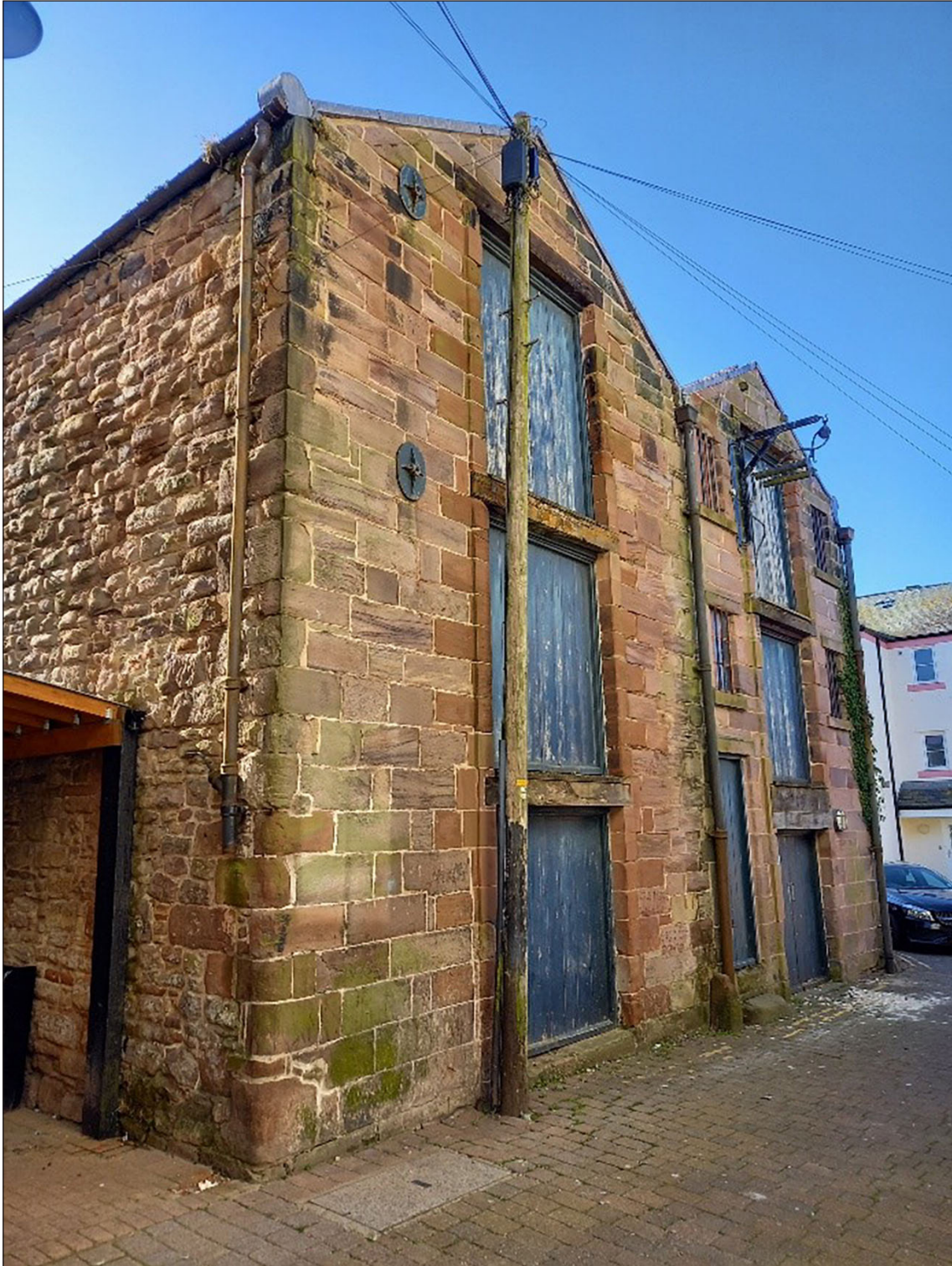
Figure 20: Warehouses on Chapel Street, Whitehaven (© Historic England, photograph: Fiona Wooler, 2021)
