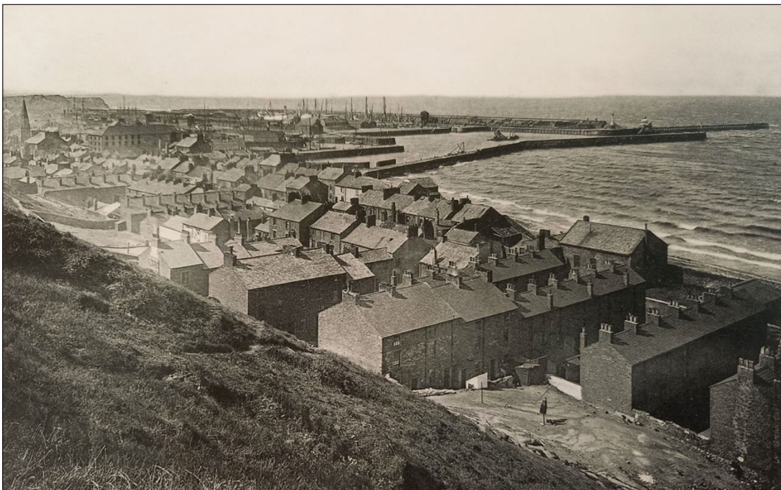
Figure 35: View from Camp Hill showing the Down Street area of Maryport c 1900 (CASC Ref. DX366/1, reproduced by kind permission of Cumbria Archive Service)
