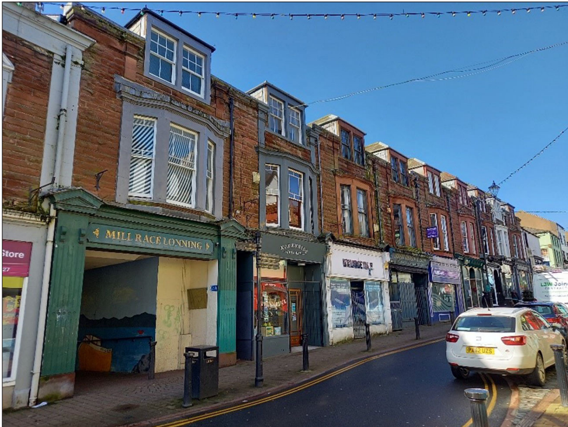
Figure 66: South side of Senhouse St (Nos. 69 to 85) (© Historic England, photograph: Fiona Wooler, 2021)
