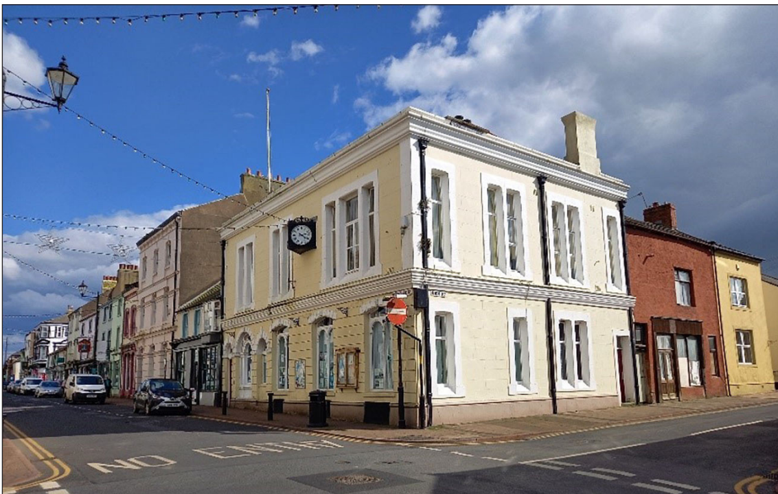
Figures 57: The Town Hall on the south-east corner of Senhouse Street and High Street (© Historic England, photograph: Fiona Wooler, 2021)
