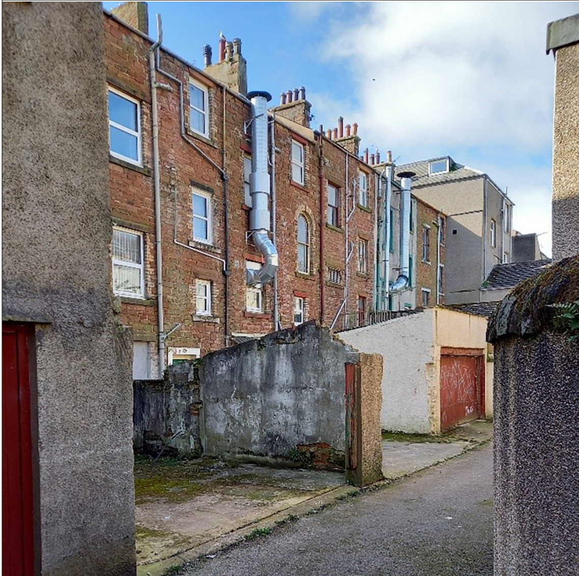
Figure 65: Rear of Nos. 90 to 104 Senhouse Street as seen from back lane (© Historic England, photograph: Fiona Wooler, 2021)
