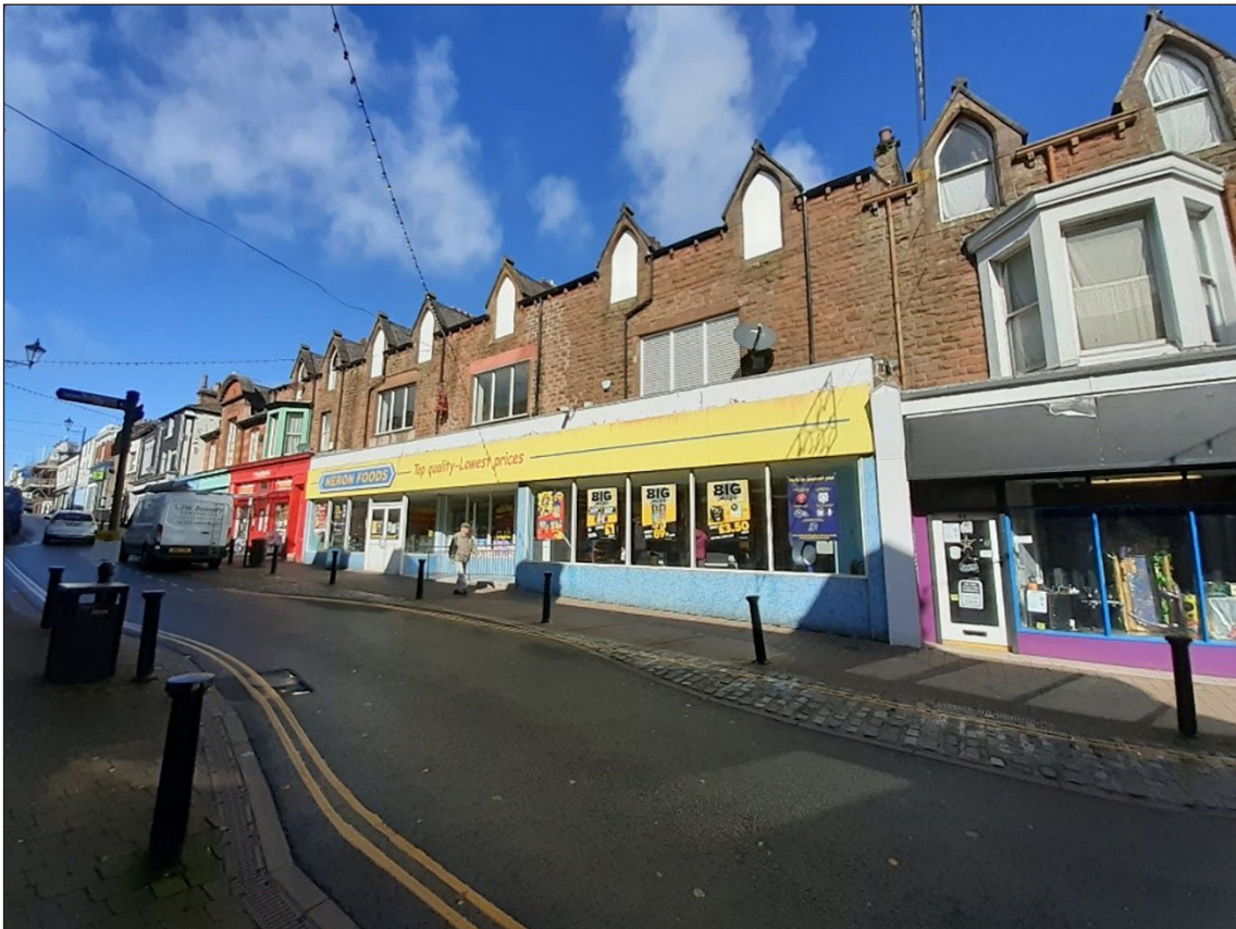
Figure 63: North side of Senhouse Street, part of Nos. 74 to 86 (© Historic England, photograph: Fiona Wooler, 2021)
