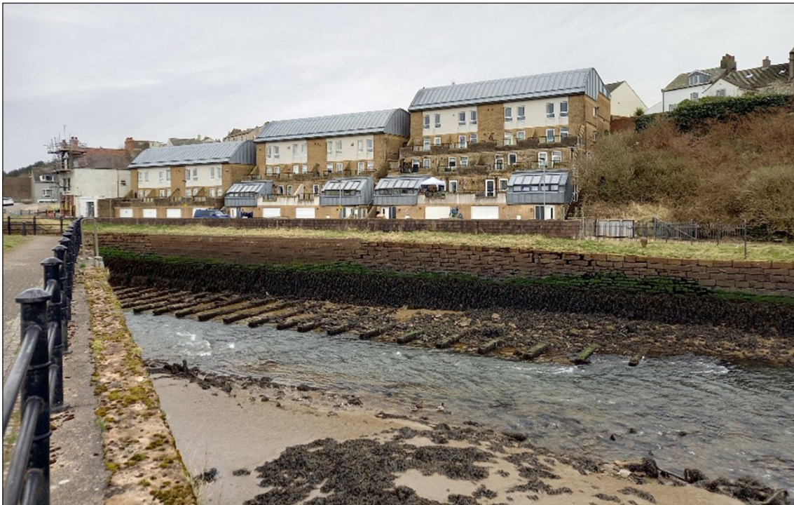
Figure 49: The Well Lane development as seen from the opposite side of the River Ellen (© Historic England, photograph: Fiona Wooler, 2021)
