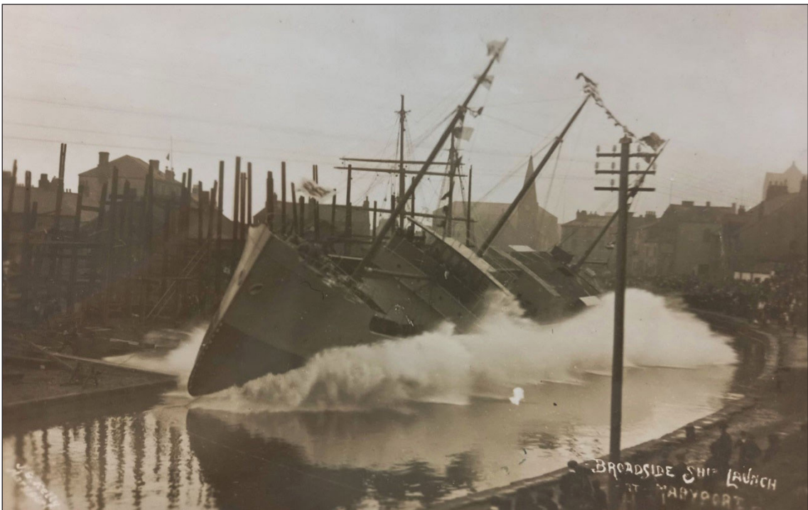
Figure 18: Undated (c 1900) broadside launch from the Irish Street shipyard (CASC Ref. DCR 76G, reproduced by kind permission of Cumbria Archive Service)
