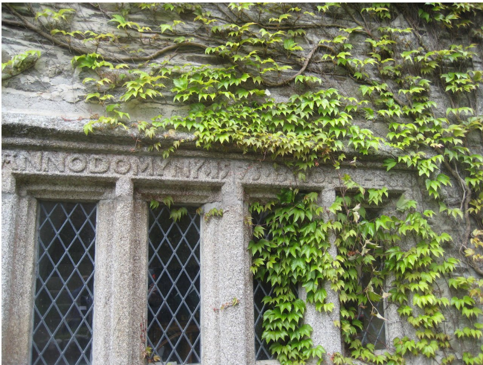
Figure 3: The carved inscription on the lintel of the reset four-light mullion window in the front range (photograph Cathy Tyers)
