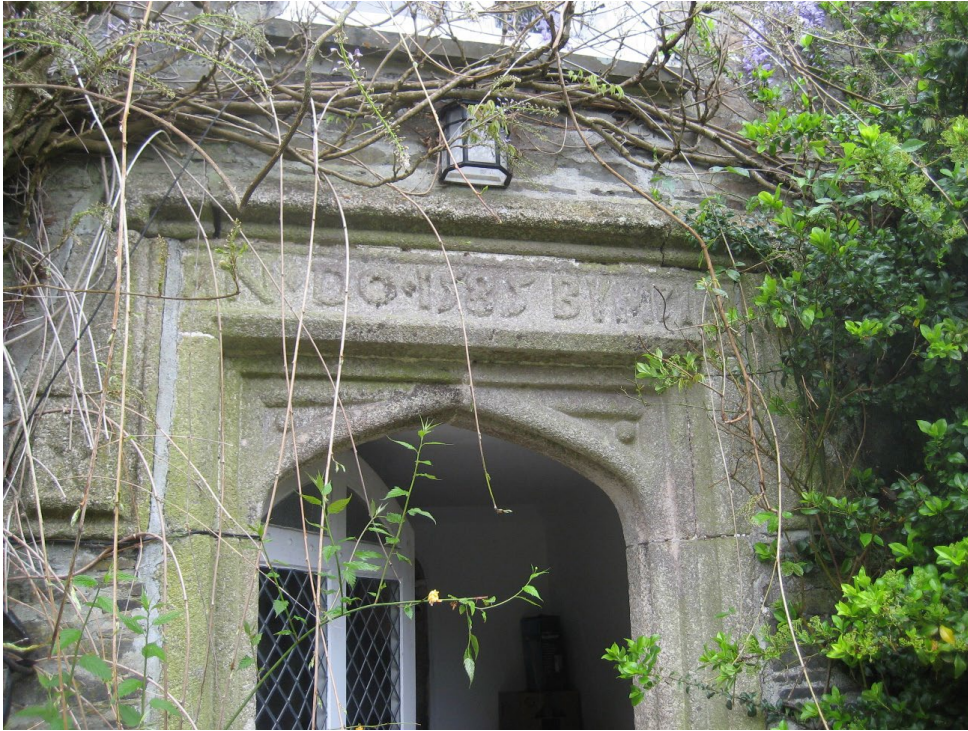
Figure 2: The carved inscription on the lintel of the two storey porch to the front of the main range (photograph Cathy Tyers)
