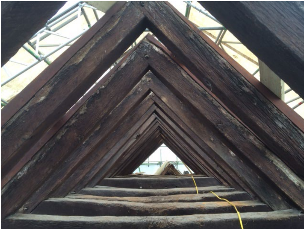
Figure 4: Extant nave roof, upper, from the west (photograph Robert Howard)
