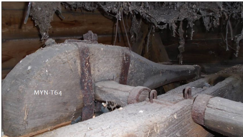
Figure 9: Bell-levers for bell 1 (above; photograph George Dawson) and bell 2 (bottom; photograph Robert Howard)
