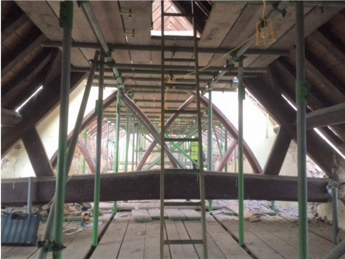
Figure 7: Extant chancel roof, truss 2, from the east (photograph Alison Arnold)
