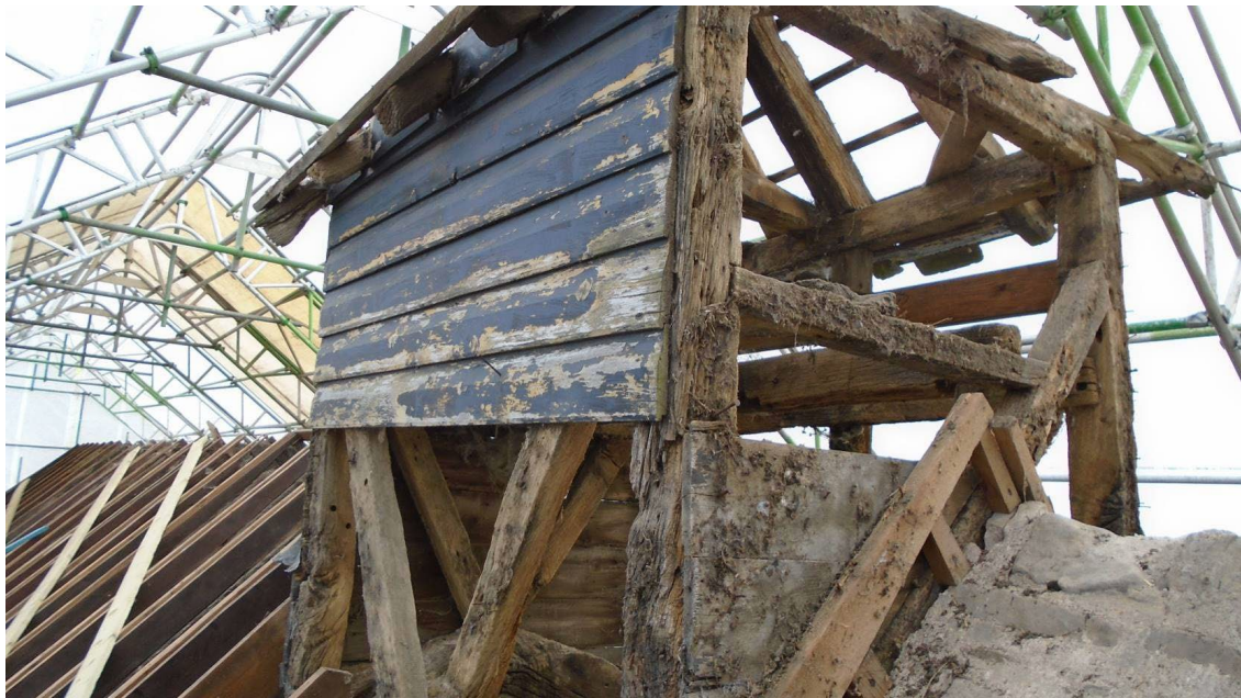
Figure 8: Bell-cote, from the north-west (photograph Robert Howard)
