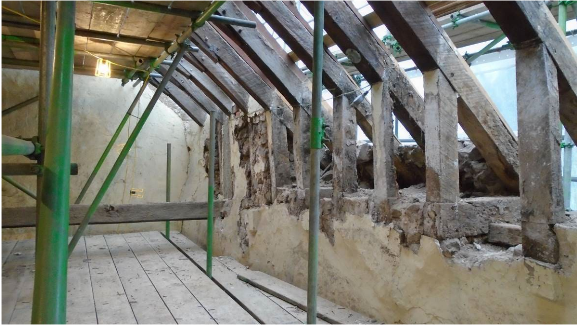
Figure 5: Extant nave roof, lower, from the east (photograph Robert Howard)
