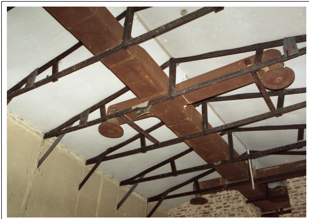
Plate 31: Rednal Operations Block, Interior View showing Laing trusses and ventilation trunking
