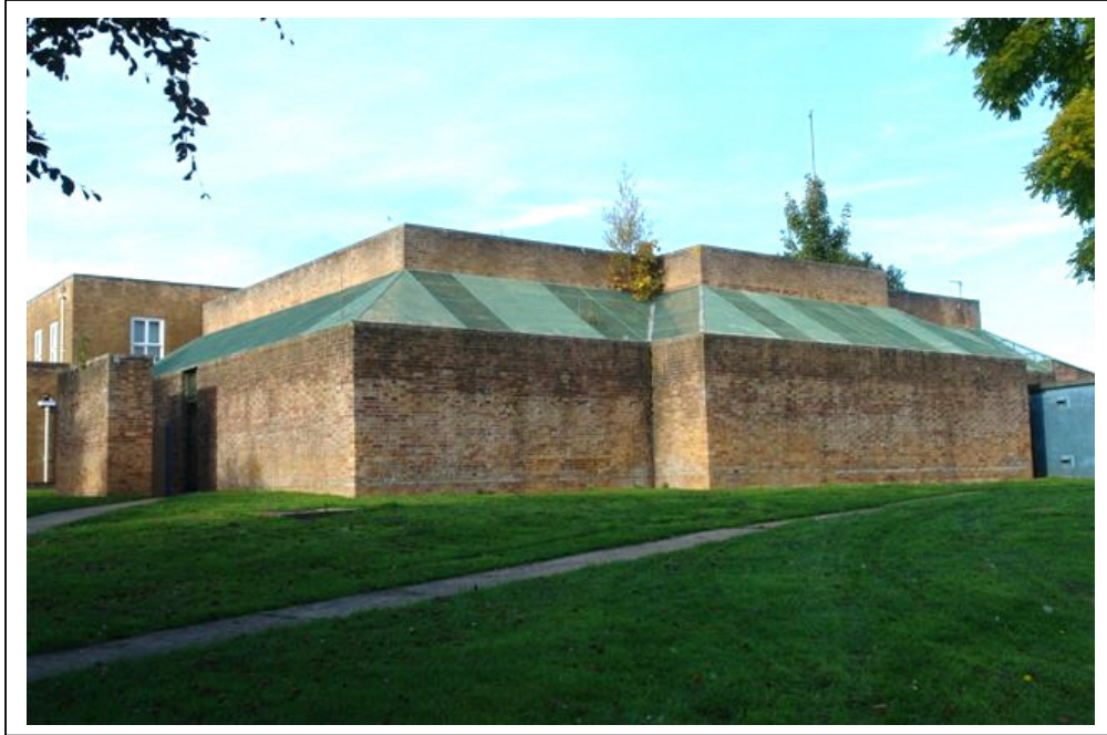
Plate 18: Coltishall (Norfolk) Operations Block Type 1723/36 with blast wall extant
