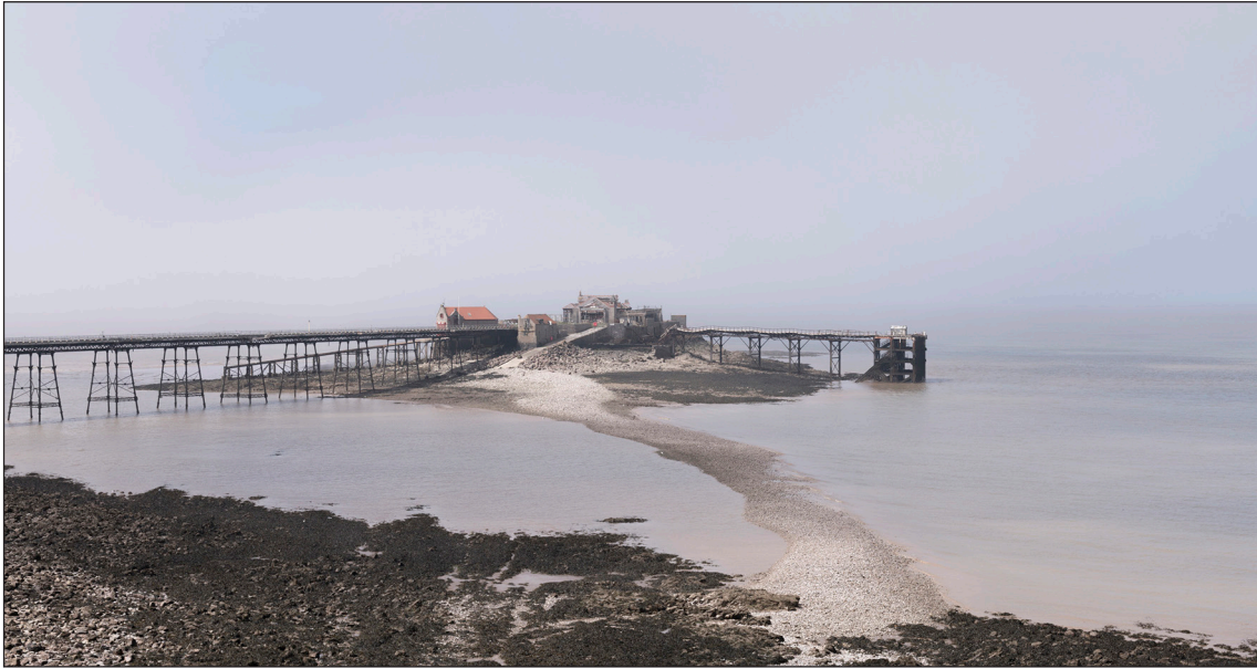
Figure 2: Birnbeck Pier and the causeway from the mainland in 2018. [Steven Baker © Historic England Archive, DP218653]
