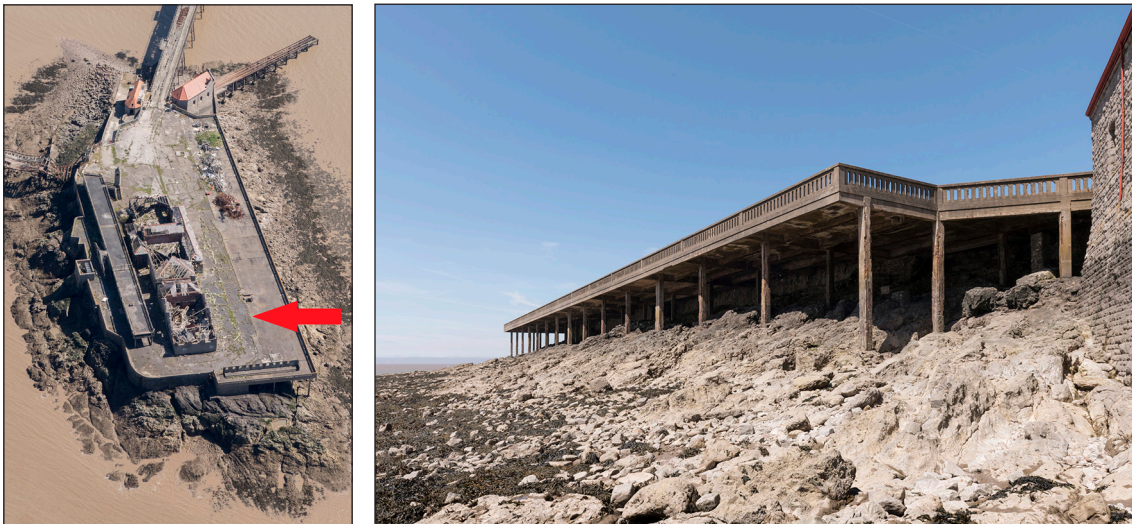
Figure 42: Left: the pier head in an aerial photograph of 2018, looking east, with an arrow indicating the junction between the old platform and the 1932 extension. [Damian Grady © Historic England Archive, 33488_048] Right: the concrete extension of 1932 in 2018. [Steven Baker © Historic England Archive, DP218672]
