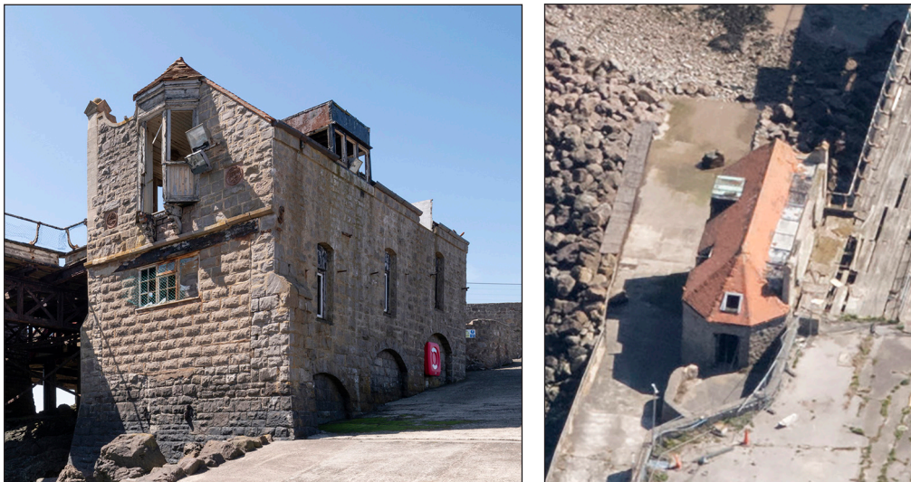
Figure 45: Left: the lifeboat house and slipway in 2018, from the east. [Steven Baker © Historic England Archive, DP218681] Right: in a detail of an aerial photograph of 2018, from the west. [Damian Grady © Historic England Archive, 33488_048]
