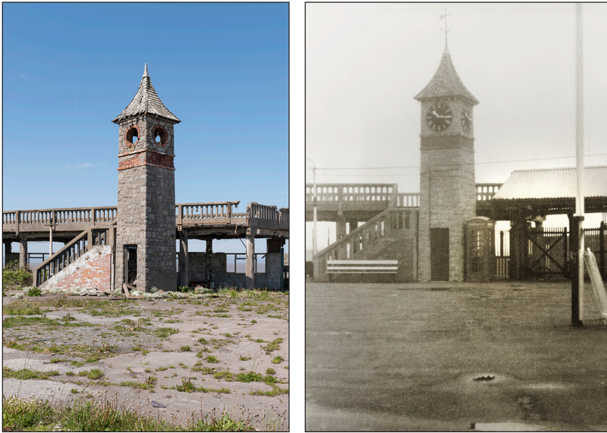
Figure 50: Left: the clocktower in 2018. [Steven Baker © Historic England Archive, DP218718] Right: in a photograph of 1960 [Copyright: Richard John Collins. Source: Historic England Archive, RBO01_01_OP15691]
