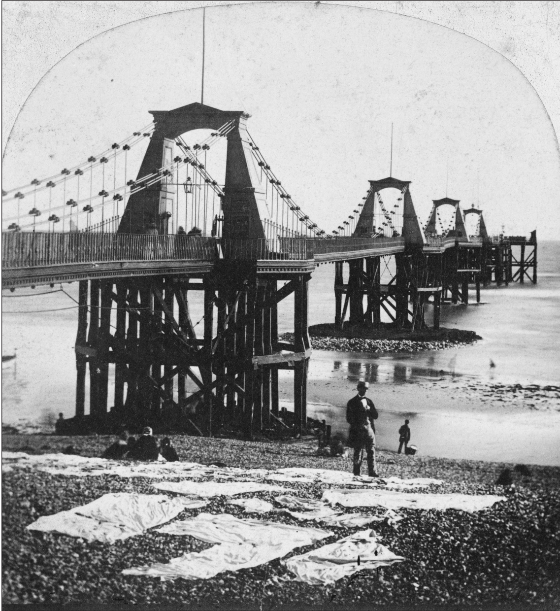
Figure 3: The Chain Pier at Brighton in a 19th-century photograph by William Henry Goodburn Mason. [Source: Historic England Archive, BB85/01743b]
