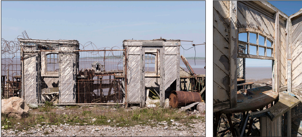
Figure 66: Left: the entrance to the north jetty in 2018, from the south; right: the inside of the right-hand (east) booth, 2018. [Steven Baker © Historic England Archive, DP218723, DP218724]
