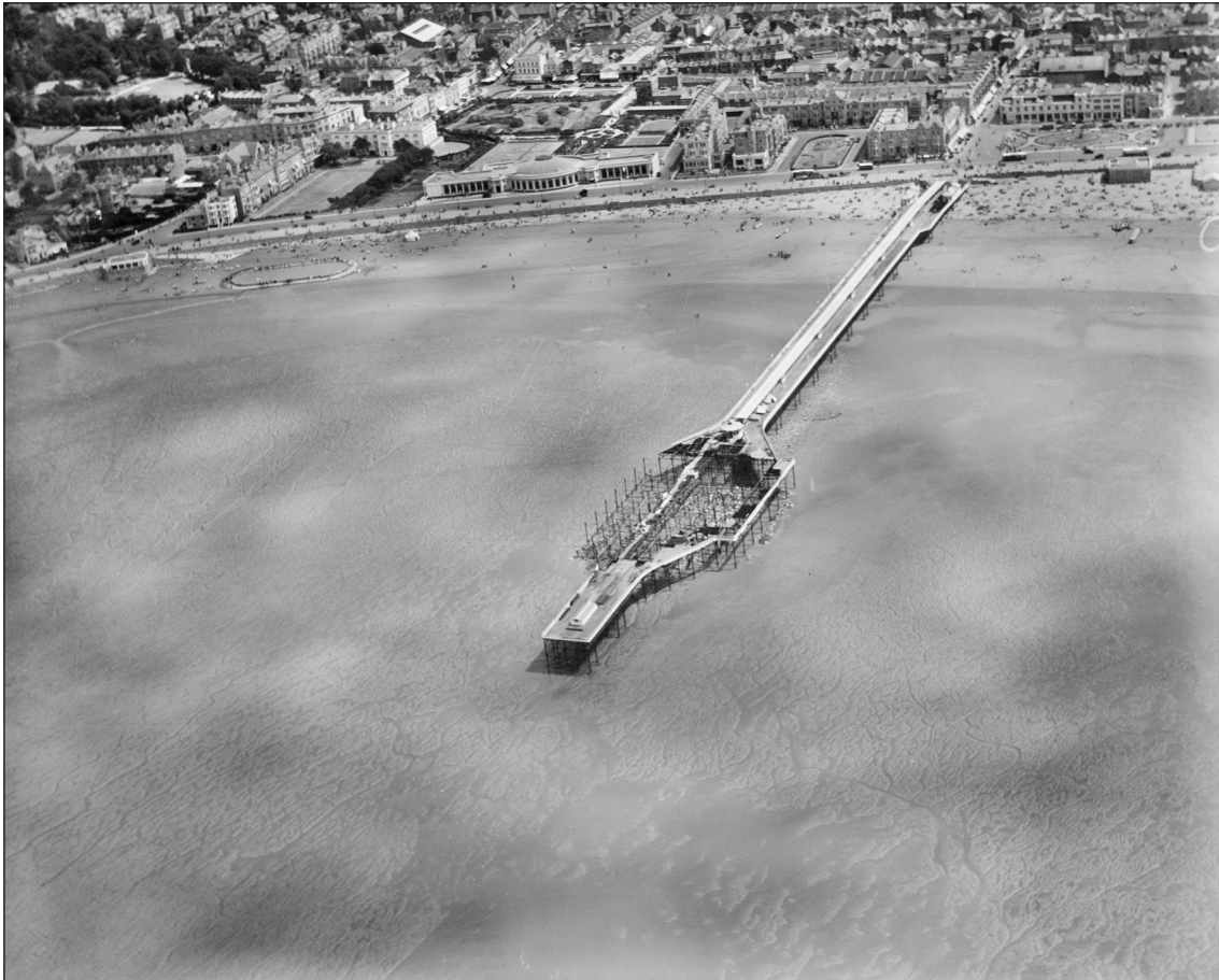
Figure 13: An aerial photograph of 1930 showing the fire-damaged Grand Pier. [© Historic England Archive. Aerofilms Collection, EPW033286]
