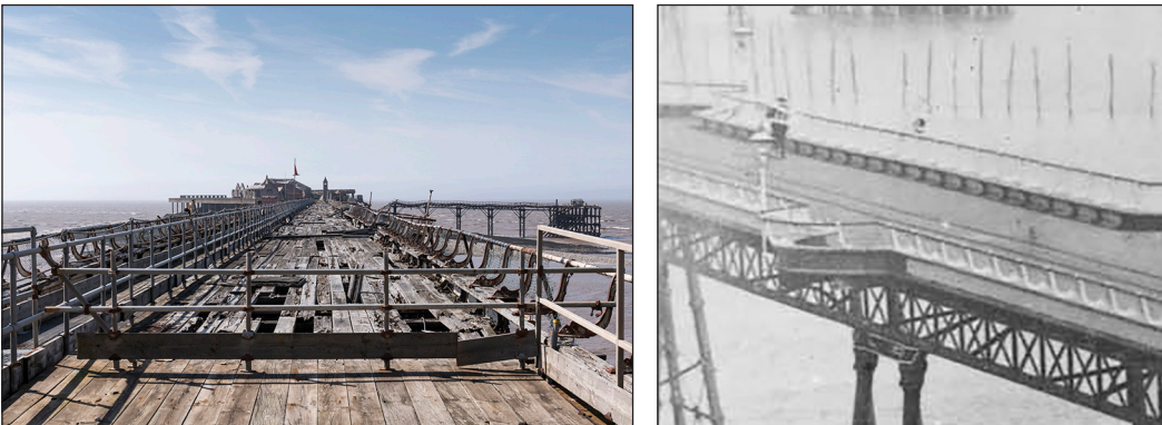
Figure 40: Left: the pier deck in 2018. [Steven Baker © Historic England Archive, DP218733] Right: detail of a postcard of about 1901 showing the original semi-circular recesses with lampposts. [Source: Historic England Archive, PC48006]
