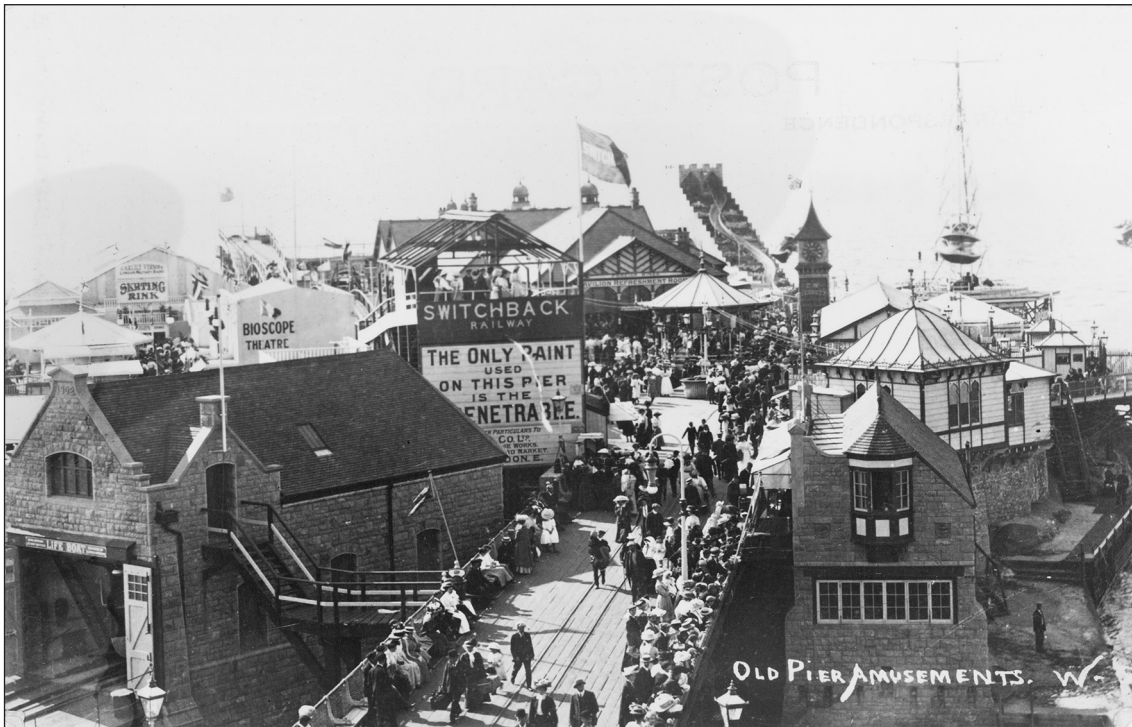
Figure 18: A postcard dating from between 1905 and 1915, showing Birnbeck Pier and the various rides and entertainments. [Source: Historic England Archive, PC48002]
