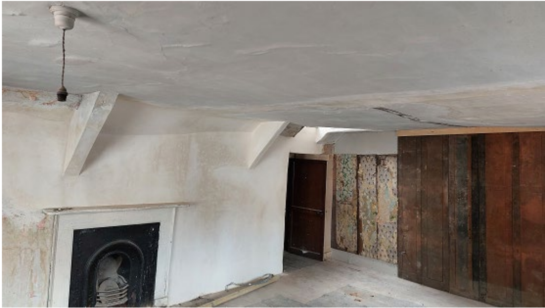
Figure 2c/d: General views of the middle cellar (top) and the south cellar (bottom), both viewed looking north (photographs Robert Howard)
