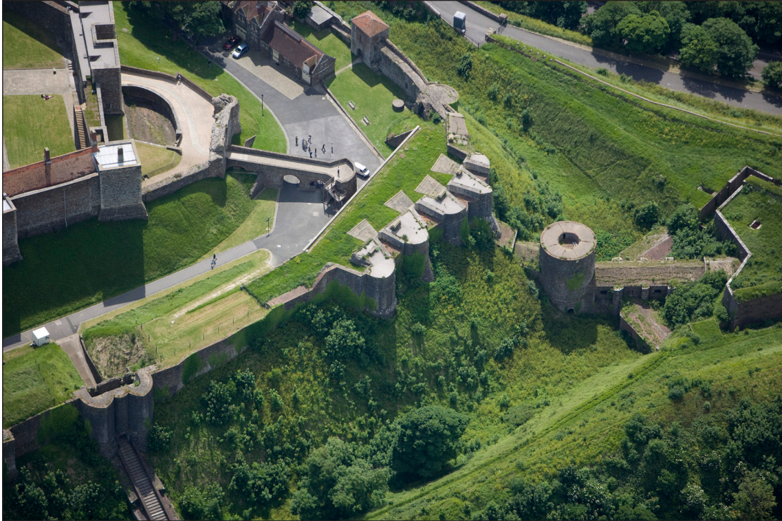
Figure 27 St John's Tower in centre with caponier, former bridge, to right and tunnels from Norfolk Towers to the left. [HE Archive 26028/010]
