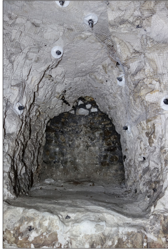
Figure 25 Possible countermine tunnel – eastern section. [Geraint Franklin © Historic England HE0129/P5]
