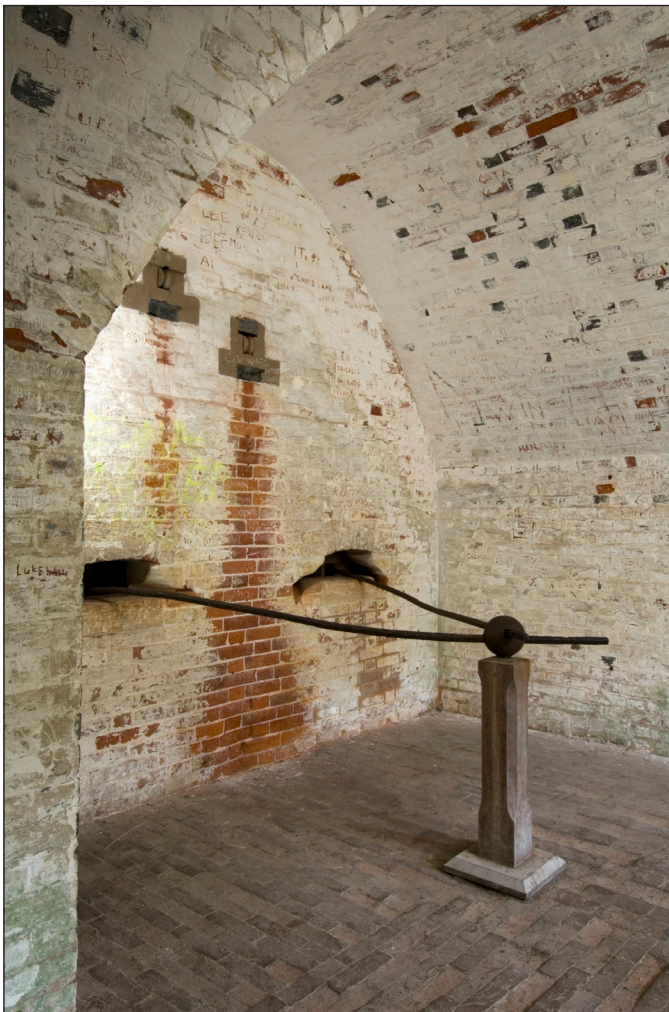
Figure 53 (top) Guard room within the Redan. The near doorway leads to the sally port complex, while the opening beyond gives access to a chamber from where the sally port doors were remotely operated. [DP047941; photographer Nigel Corrie]
