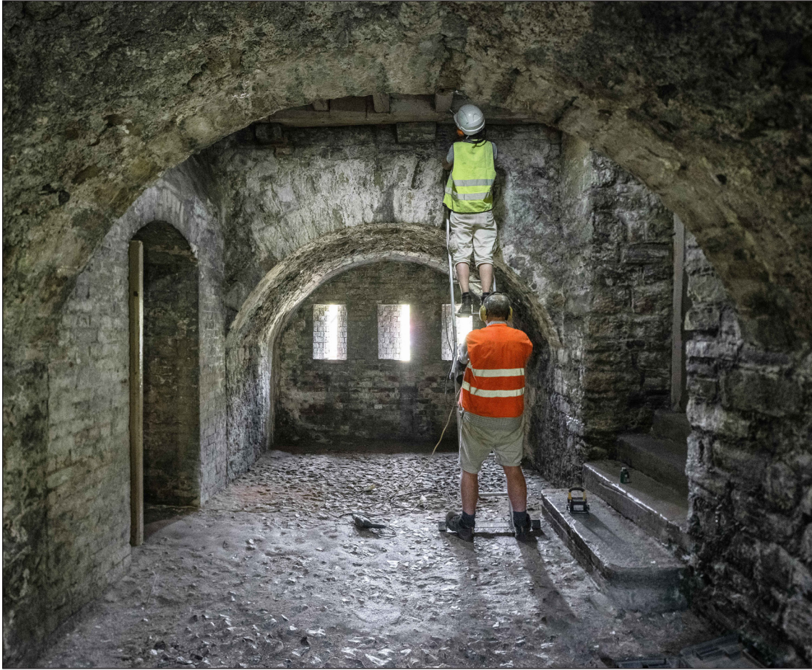
Figure 41 Dendrochronologists taking core samples from the timber ceiling occupying the position of the former drawbridge. To the left (south) is the inserted entrance to St John's Tower; to the right (north) is a set of steps ascending to the lower passage of the caponier, excavated c.1800. In the background is a brick blocking of c.1800 incorporating angled musket loops [DP289568]
