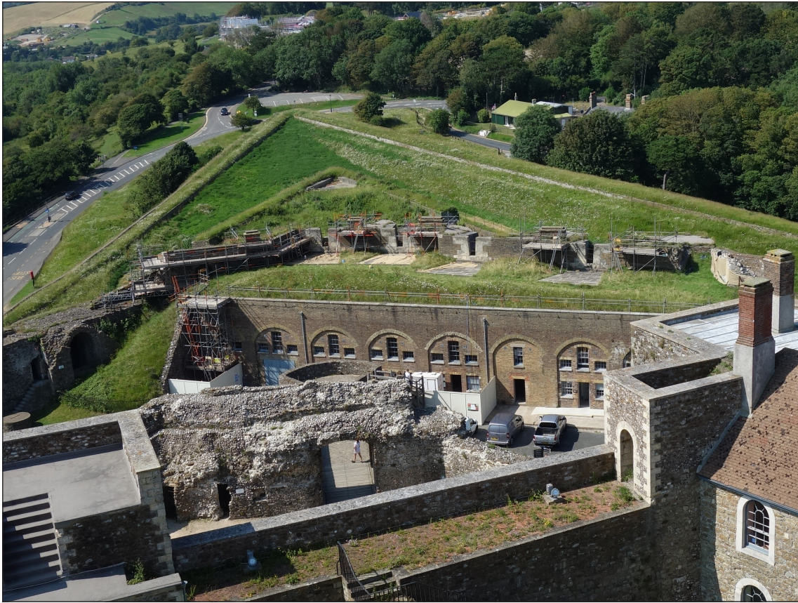
Figure 20 The Spur Casemates, with gun emplacements above. Above, note the different alignments of the redan and the Spur on which it is constructed [Geraint Franklin © Historic England HE 0129/P2]
