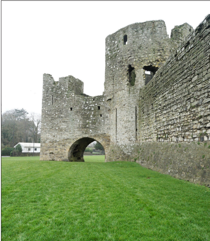
Figure 43: The early 13th-century south gate at Trim Castle, County Meath, Ireland. A drawbridge is enclosed within the forework to the tower which incorporates round arches on either side of the drawbridge pit. The forework may originally have been roofed. This provides a possible parallel to the relationship between the medieval bridge, drawbridge and St John's Tower at Dover. [Photograph by William Murphy, Wikimedia Commons, Creative Commons Attribution-Share Alike 2.0 Generic]
