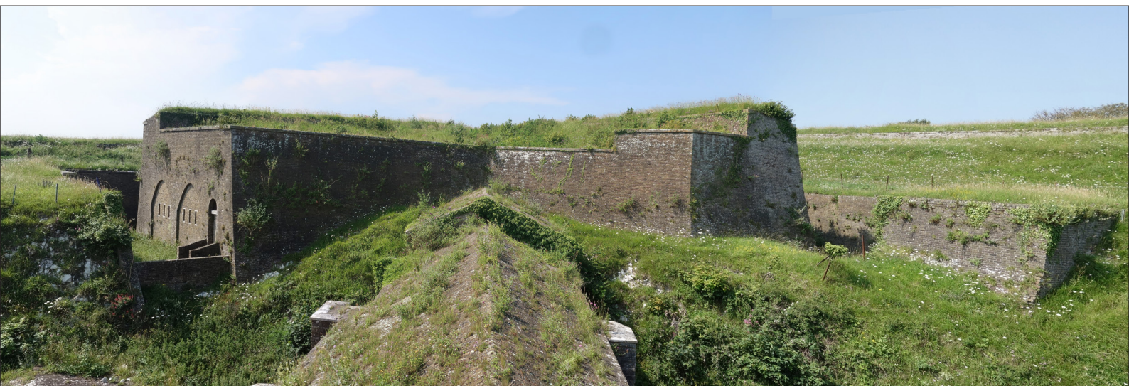
Figure 48: A view of the gorge of the redan, looking north from St John's Tower and showing the brick roof of the caponier. To the left is the sally port. [Geraint Franklin © Historic England HE0129/P7]
