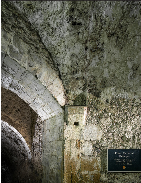
Figure 50 Remains of rib vault on south side of crossing. [DP289573]
