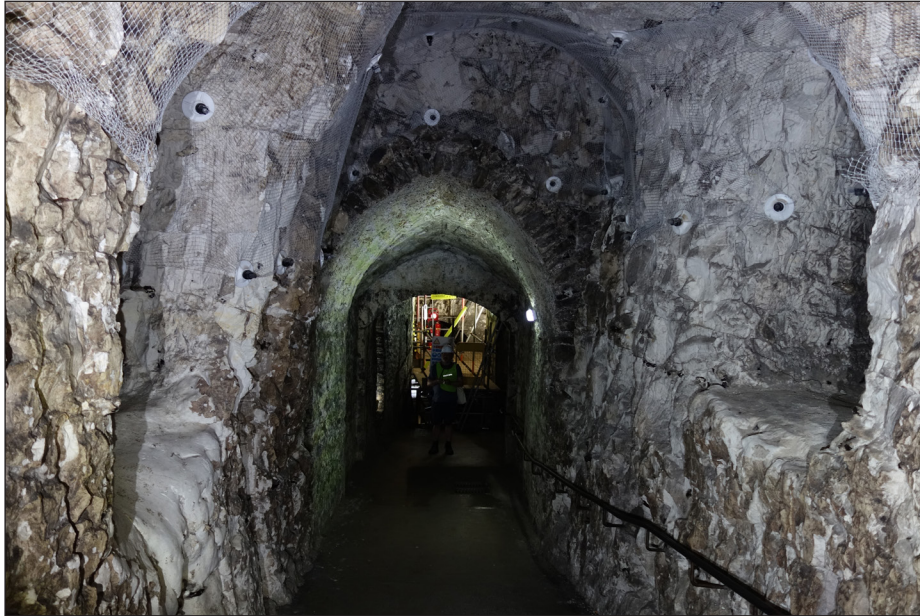
Figure 4 Possible countermine to left and right of main tunnel. At the end of the tunnel is the entrance to St John's Tower . [Geraint Franklin © Historic England HE0129/P1]
