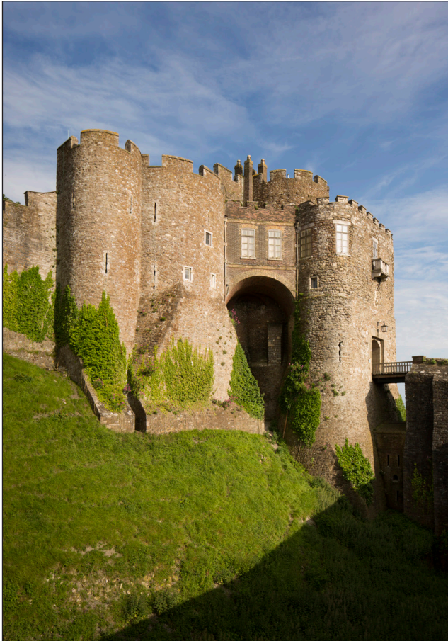
Figure 5 Constable's Gate, inserted into the earlier Outer Bailey wall. [DP187450, photographer Patricia Payne]
