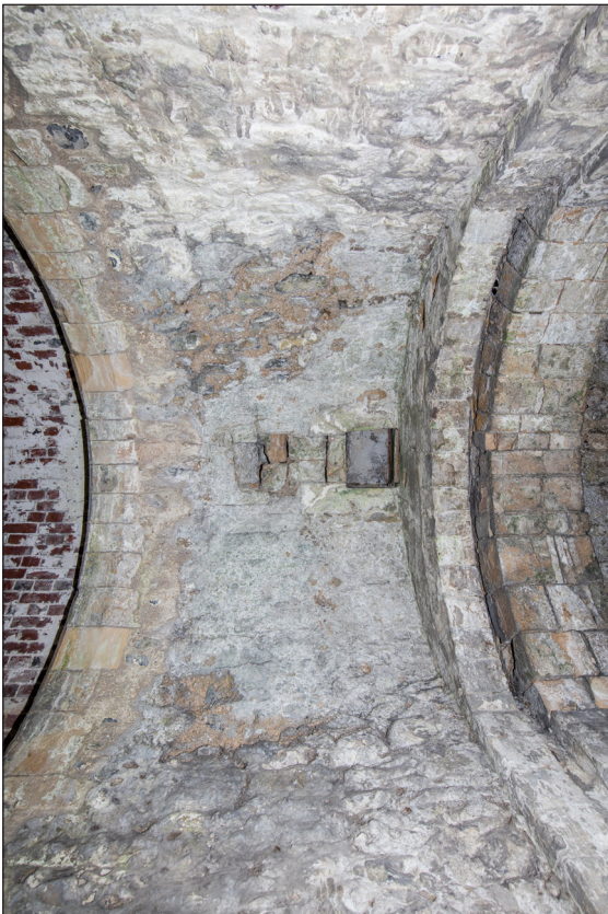
Figure 38 Spiral stair entrance at second-floor level and opening at third-floor level above where spur of five steps is located. [Courtesy of English Heritage]
