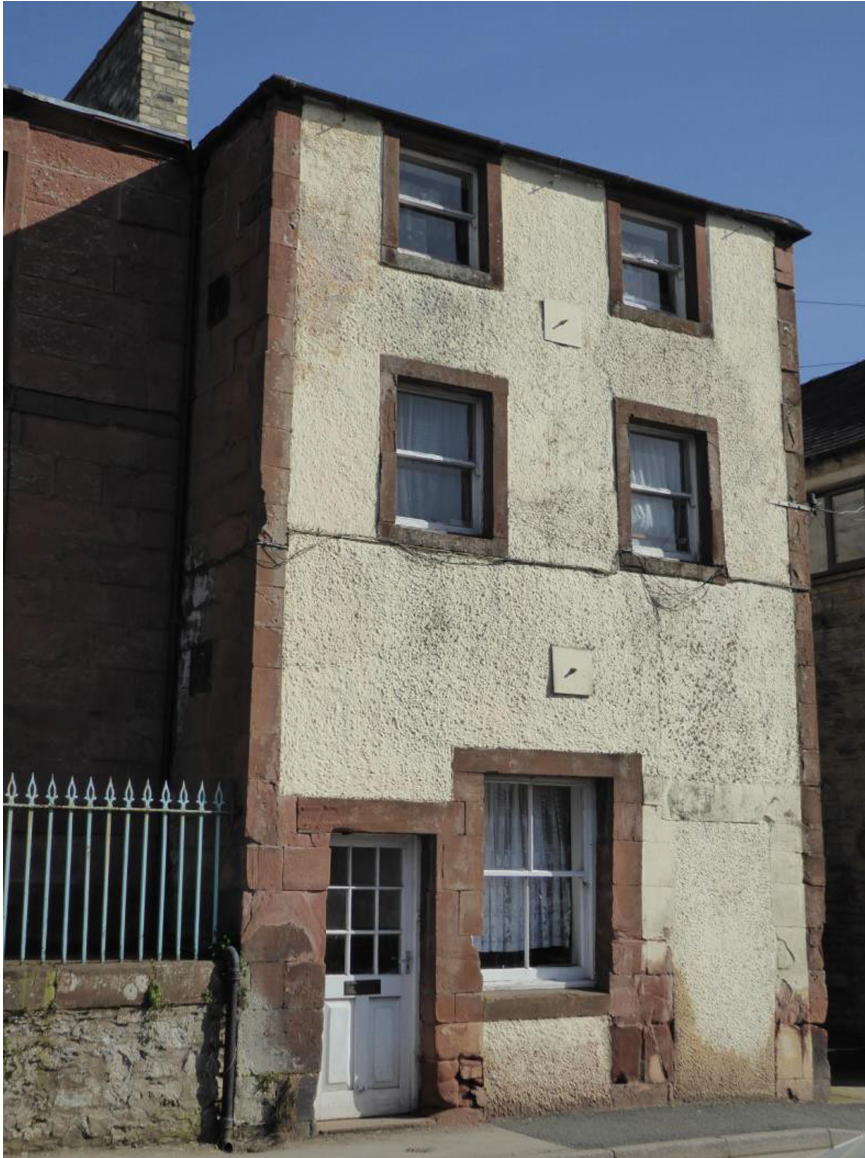
Figure 2 – Building 2: Appleby before fabric improvements. (Historic England © Rebecca Pullen)
