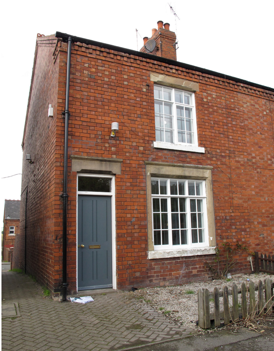
Figure 1 – Building 1: New Bolsover after fabric improvements. (Historic England © Iain McCaig)
