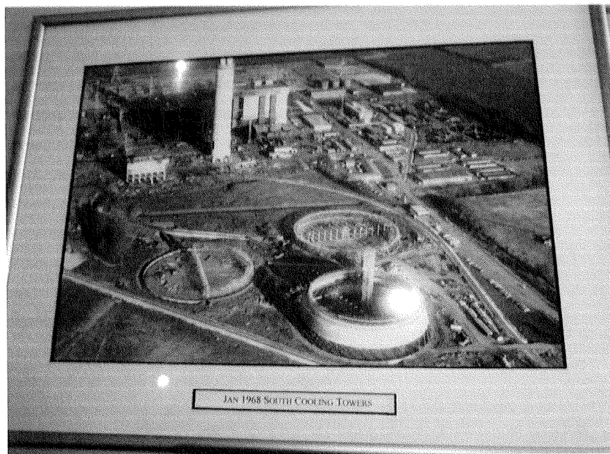
Figure3 .Southern cooling towers in 1968.Note the different stages of the build, the free-standing 650 ft .chimney, turbine hall and ancillary buildings ( RWE npower photograph).
