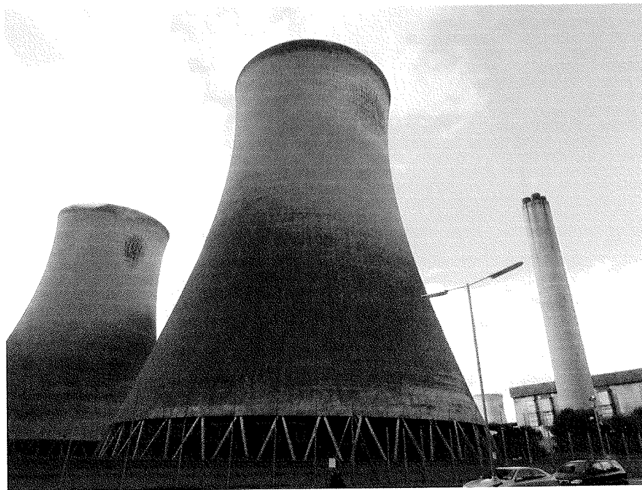
Figure 10. Grey reinforced concrete hyperbolic shell of cooling tower on reinforced concrete piloti and four-flue chimney for expulsion of combustion gases
