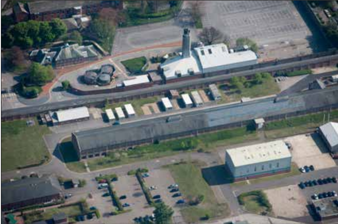
Figure 26: Aerial view of the eastern end of No. 2 Ship Tank showing the exposed arches of the arcade which carries the tank building (HEA 26/26941/016)
