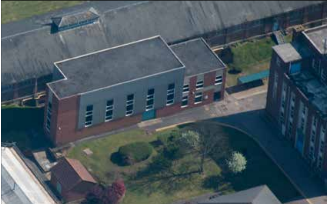
Figure 34: The circulating water channel building from the north in 2011. The adjacent building is Building 47 which houses No 2 Cavitation Tunnel (HEA 26941/15)
