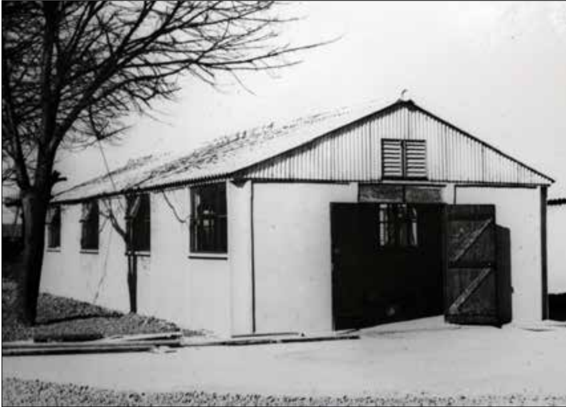
Figure 38: The newly completed anchor tank building in 1948 (TNA ADM 226/59)
