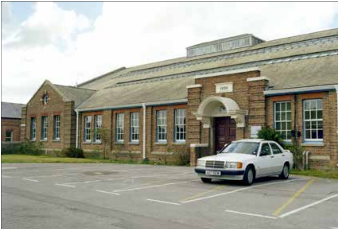
Figure 28: The neo-Georgian south-east elevation of the workshop of No 2 Ship tank bearing a date stone of 1930 to commemorate its completion (IWM 2005-02-20 2052/98)
