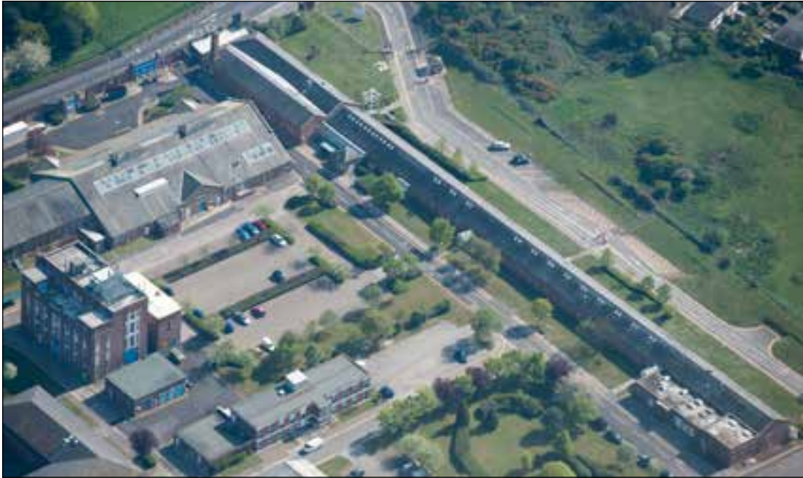
Figure 22: AEW Haslar from the north in 2011. No 1 Ship Tank (right) was converted for use as offices in 1993 however the former workshop (top), waterway and later drawing office (bottom right) remain discernible elements of the building. Also pictured are the Administration Building (bottom), No. 2 Cavitation Tunnel (left) and the workshop of No. 2 Ship Tank (top left). (HEA 26941/14).
