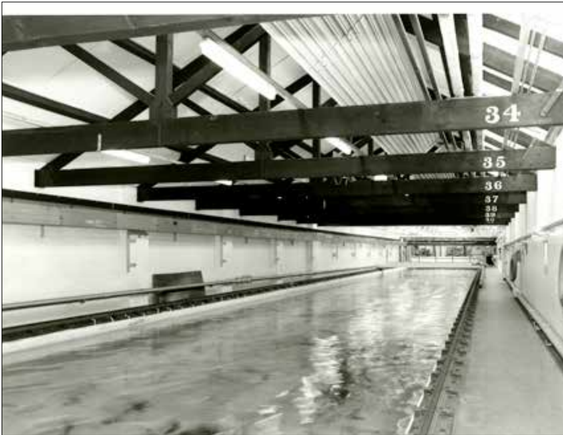
Figure 24: View from the south along the waterway of No 1 Ship Tank in 1993 (HEA BB94/5069)
