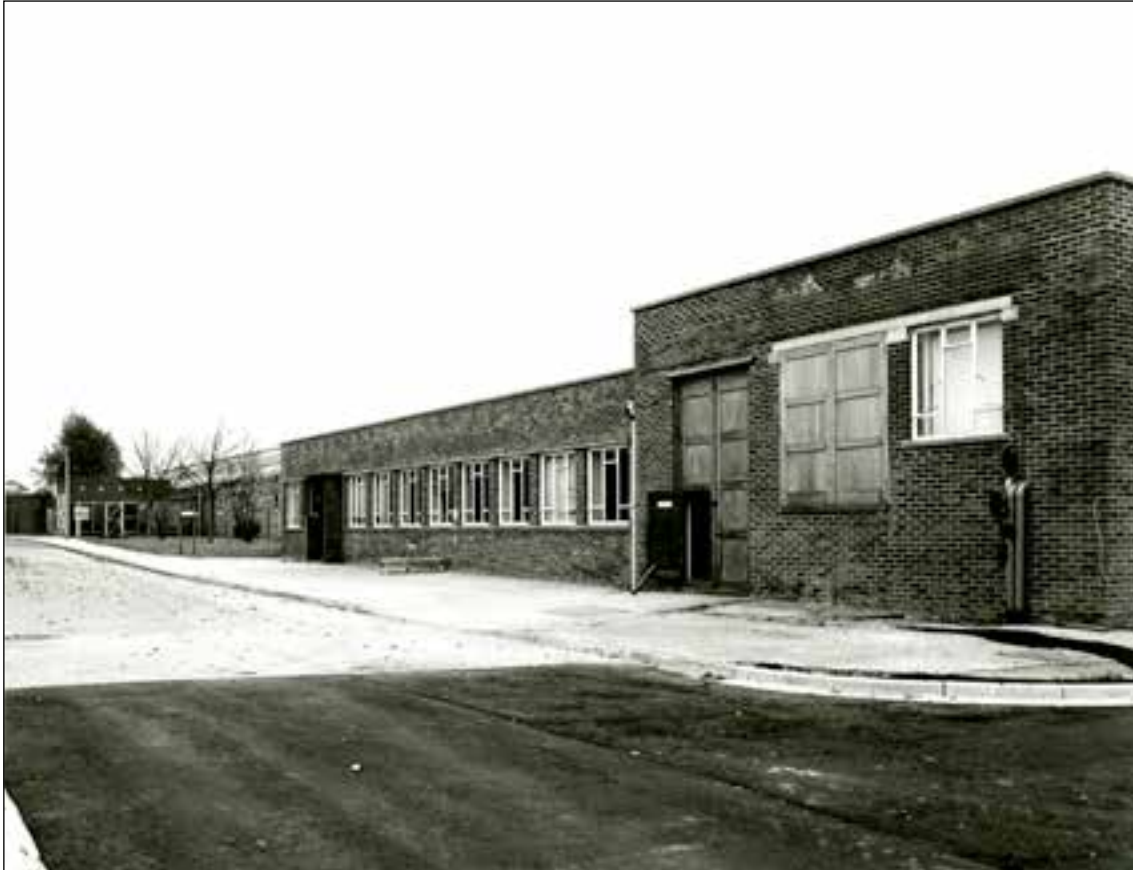
Figure 25: North-eastern elevation of the 1957 extension of No 1 Ship Tank and the new drawing office indicating the height of the raised dock area within (HEA BB94/5075)
