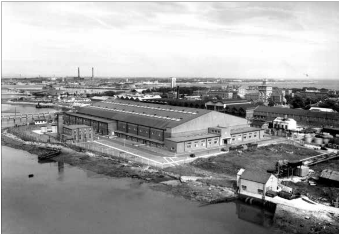
Figure 32: Oblique aerial photograph of the manoeuvring tank from the east showing the workshop range and adjacent boiler house. In the foreground and right of picture, the inlet pipes of the pumping house are clearly visible as are the initials of the Admiralty Fuel Experimental Station. © IWM 2005-02-20 19426
