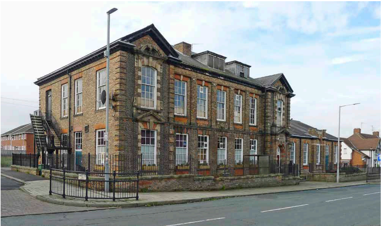
Figure 70: The North East Railway Institute on Redworth Road. [Lucy Jessop © Historic England]
