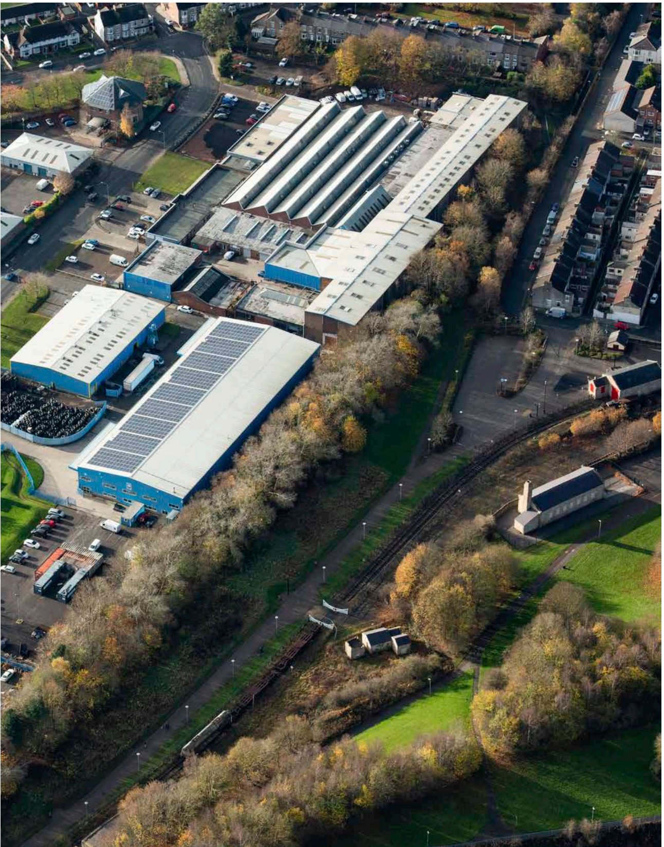
Figure 38: An aerial view of part of Character Area 1, showing the lineside cabins, the Soho Shed and part of the original S&DR trackbed. [Detail of HEA_34133_043 23-NOV-2021 © Historic England Archive]
