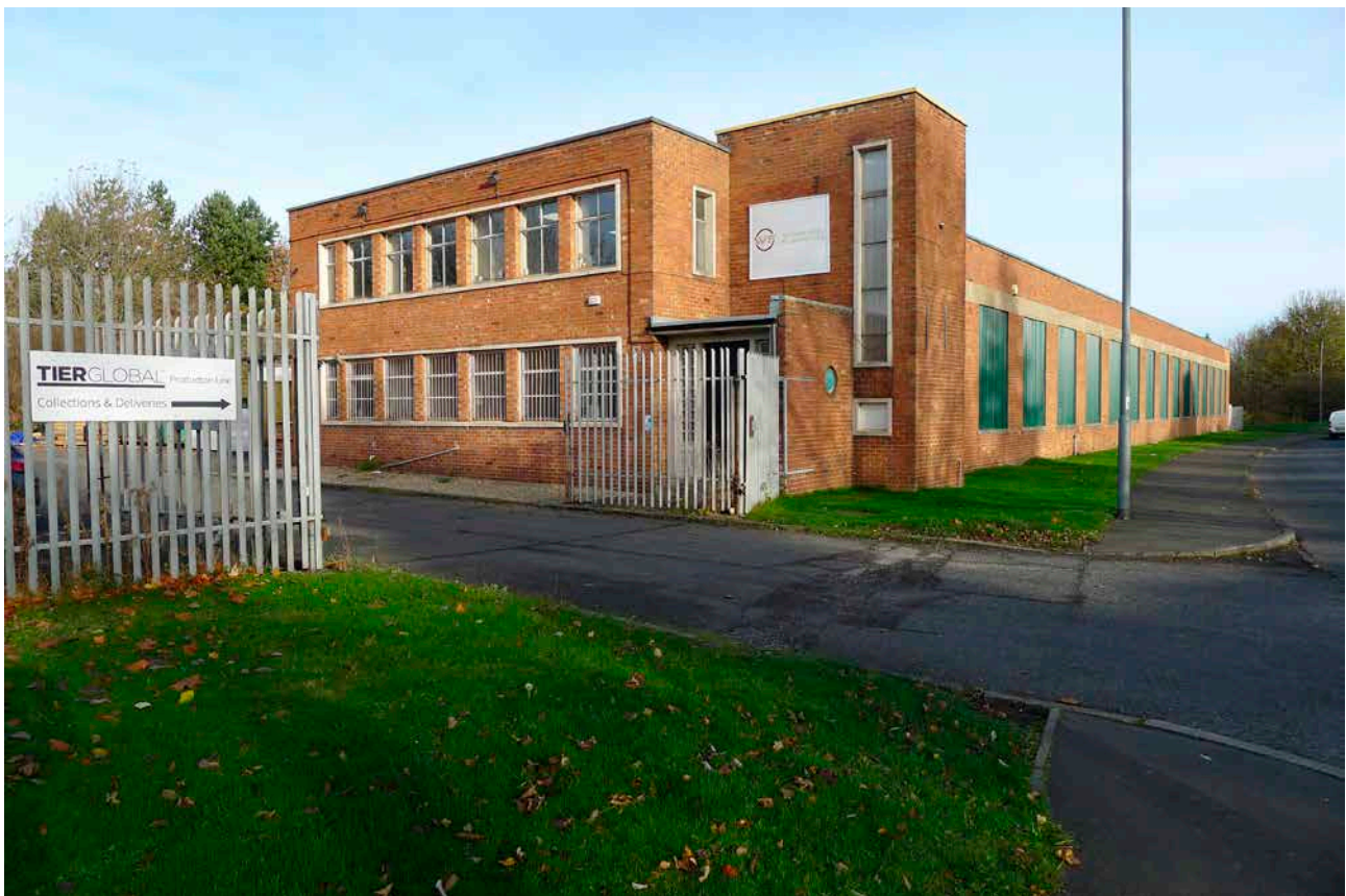
Figure 68: A factory built in the 1940s, with concrete window surrounds and a projecting stair tower. [Lucy Jessop © Historic England]
