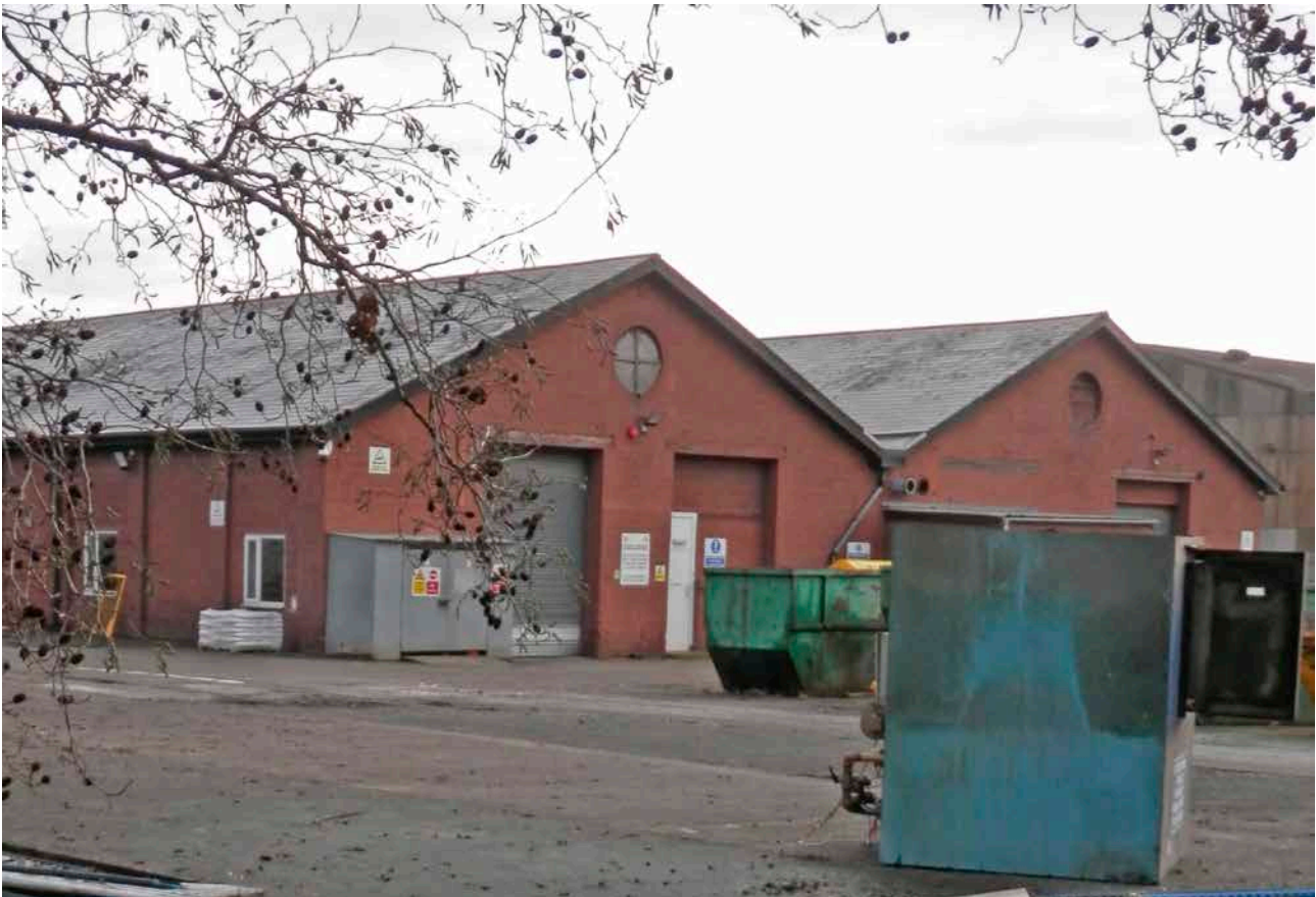
Figure 61: The former wheel lathe and iron machinery shop, now occupied by AMETEK Solartron ISA. [Lucy Jessop © Historic England]
