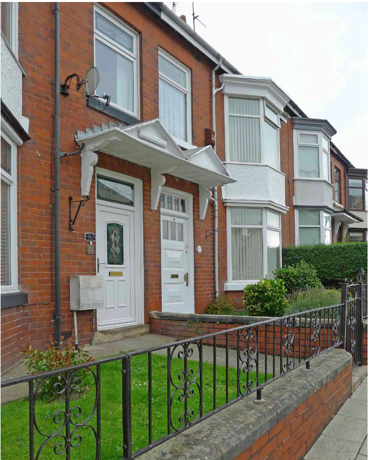
Figure 74: Nos 163-167 (odd) Redworth Road, with original door canopies and one original front door. [Lucy Jessop © Historic England]
