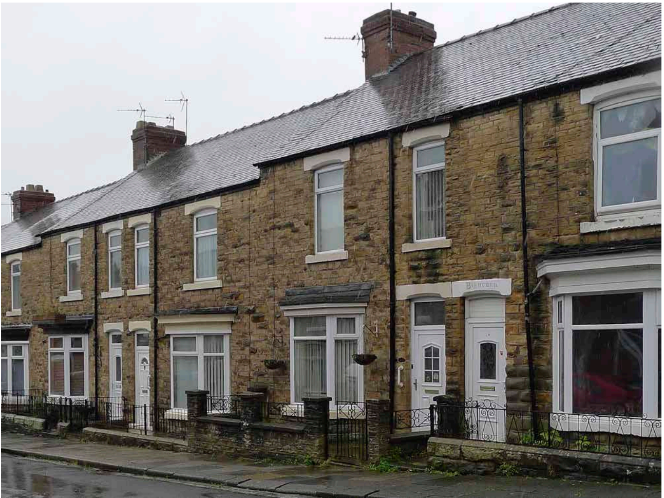
Figure 73: Stone-faced brick row in All Saints Road, showing the stone forecourt walls. [Lucy Jessop © Historic England]
