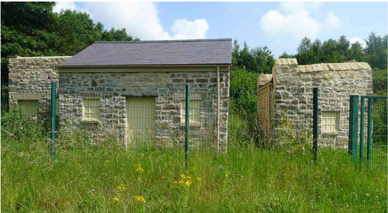
Figure 40: The lineside cabins, seen from the south. [Lucy Jessop © Historic England]
