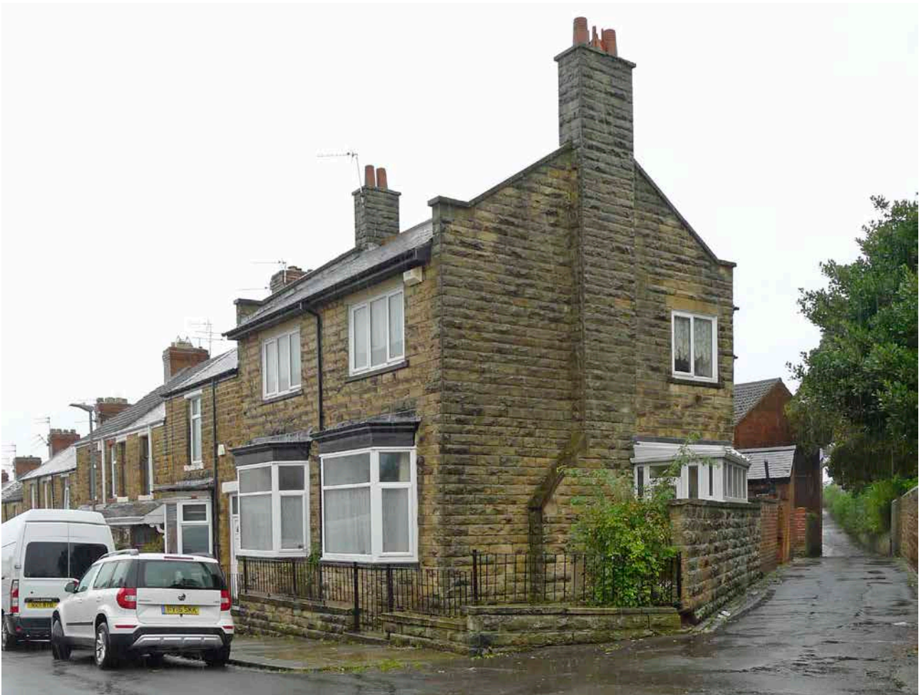
Figure 31: The curate's house, All Saints' Road, built in 1912. [Lucy Jessop © Historic England]
