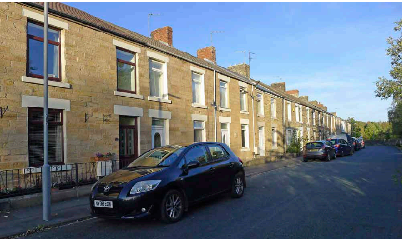
Figure 57: Station Street, with some of the stone kneelers in the eaves. [Lucy Jessop © Historic England]
