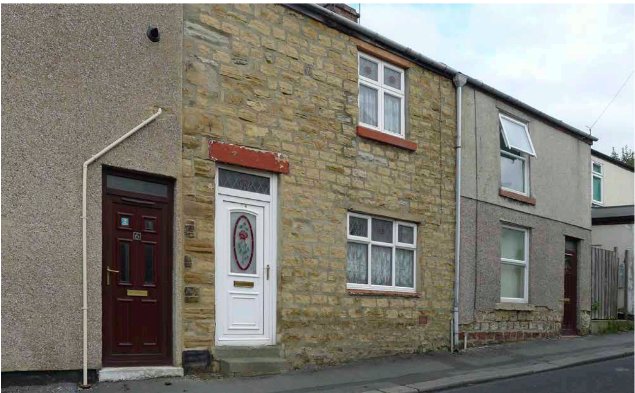
Figure 48: Nos. 2-6 Mill Street, with a variety of renders mostly hiding the sandstone elevations. [Lucy Jessop © Historic England]
