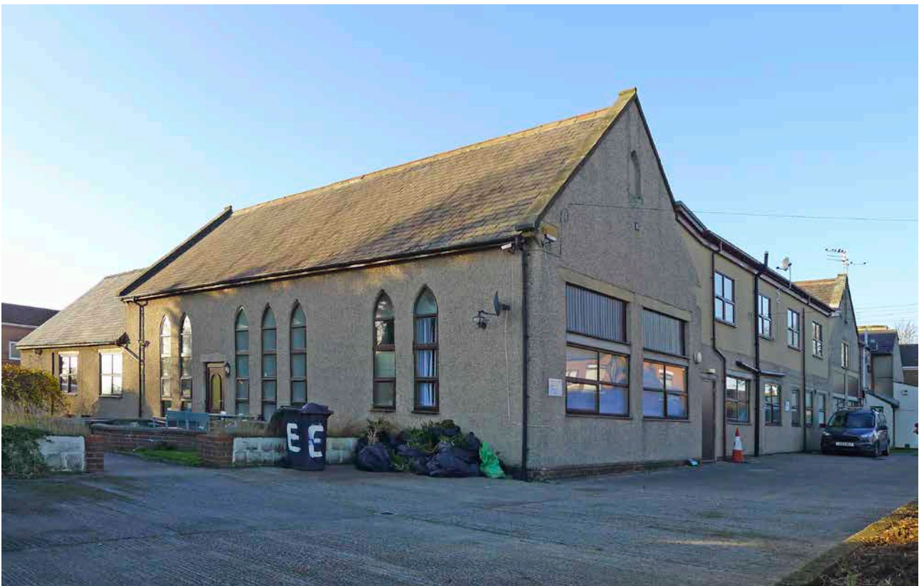
Figure 81: The former All Saints School, now the Grange. [Lucy Jessop © Historic England]
