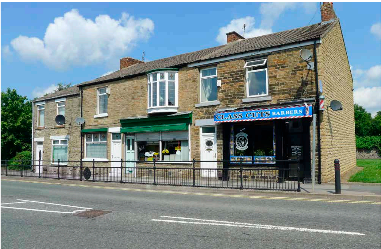
Figure 50: Nos. 7 to 11a Redworth Road, a group of early to mid-19th-century houses with their front rooms used as shops. [Lucy Jessop © Historic England]
