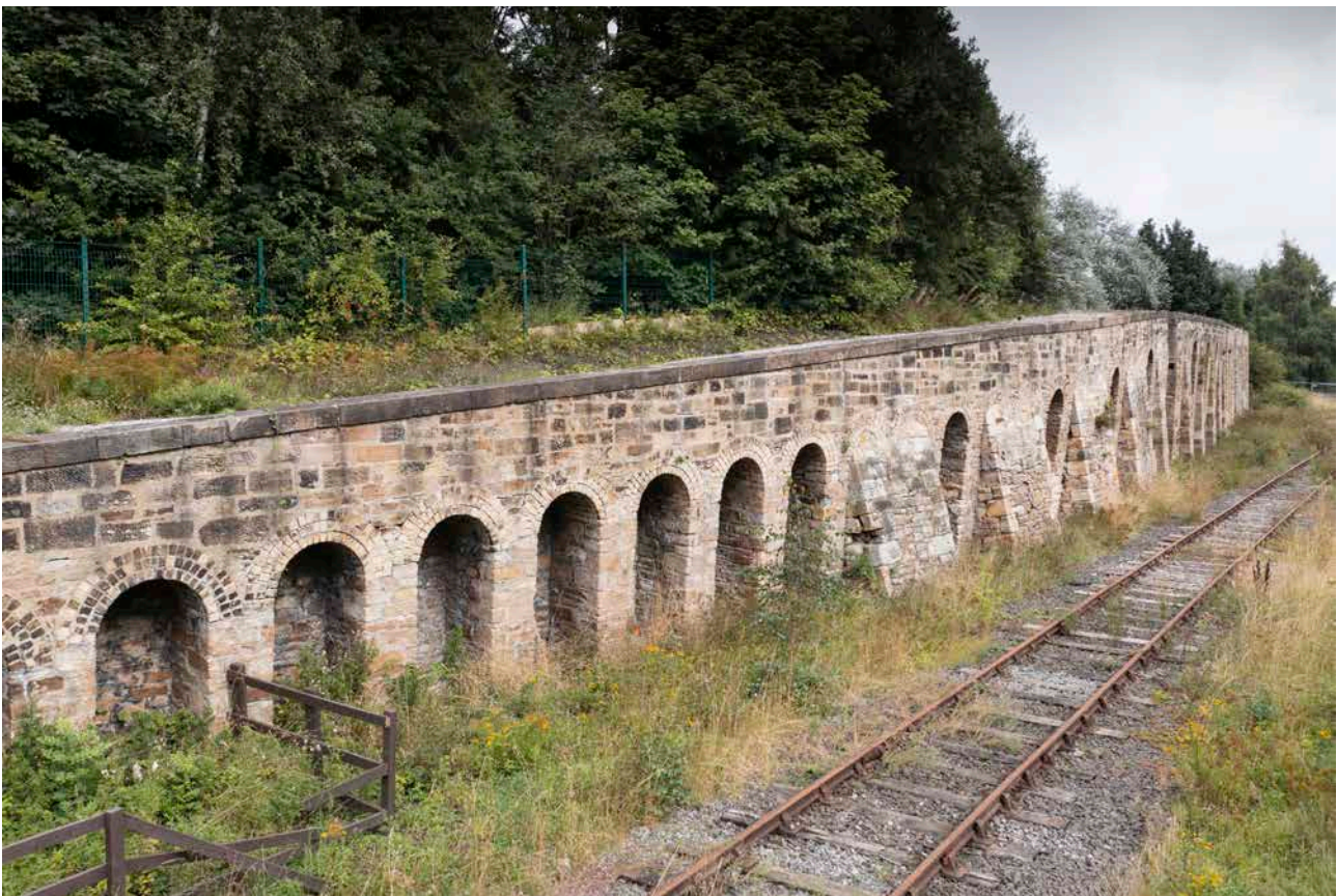
Figure 42: View of the Coal Drops. [Alun Bull © Historic England Archive, DP289852]
