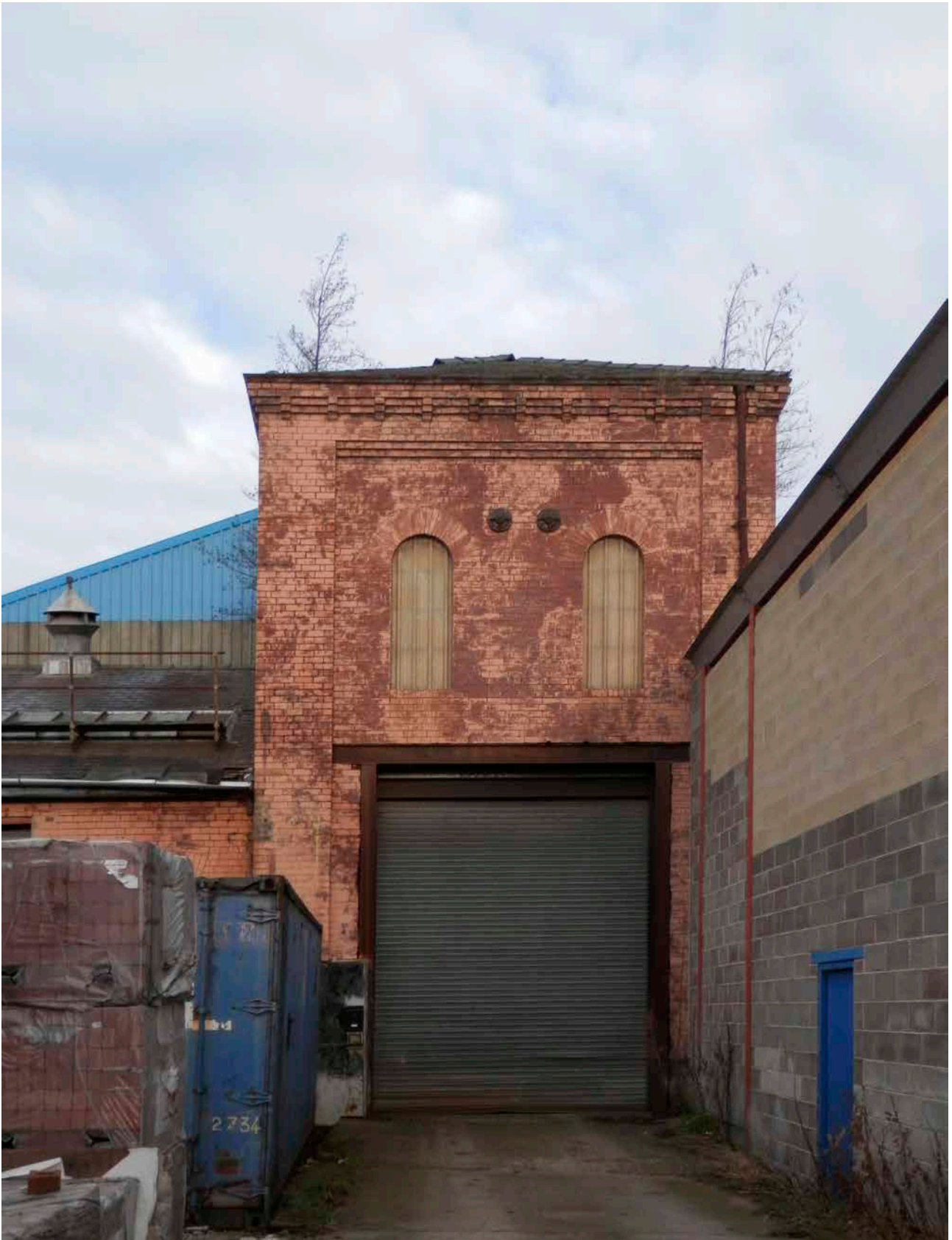
Figure 62: The former Hydraulic Power House. [Lucy Jessop © Historic England]
