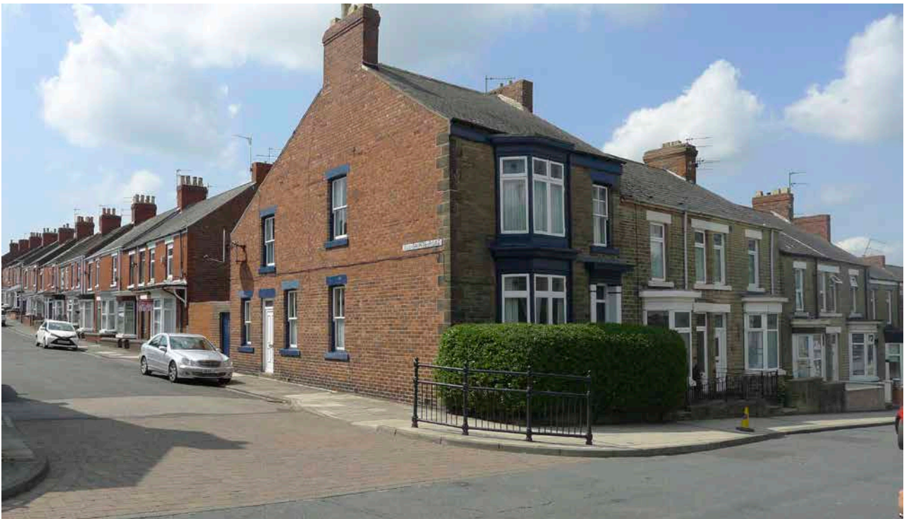
Figure 71: The corner of Redworth Road with All Saints Road, showing the large rear outshots of Redworth Road's houses. [Lucy Jessop © Historic England]
