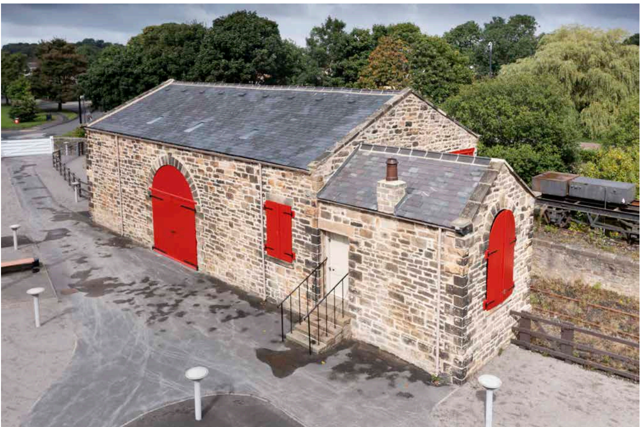
Figure 41: The Goods Shed. [Alun Bull © Historic England Archive, DP289841]
