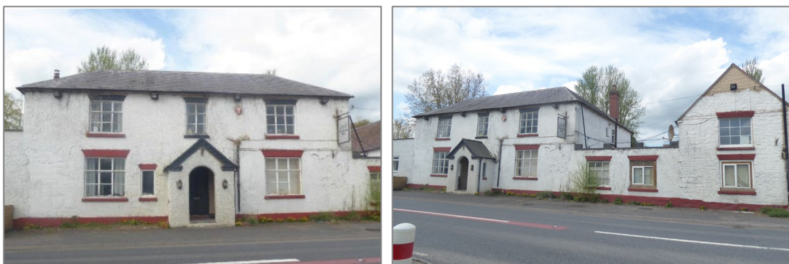
Figure 4: Affcot Lodge, near Church Stretton is an example of a pub that had undergone significant change between 2014 and 2021, notable when comparing photographs from the site visit against earlier images on streetview. In this instance a series of original windows in the ancillary building, which had originally replicated those in the main pub, had been replaced in uPVC. [Images © TDR Heritage, September 2021].
