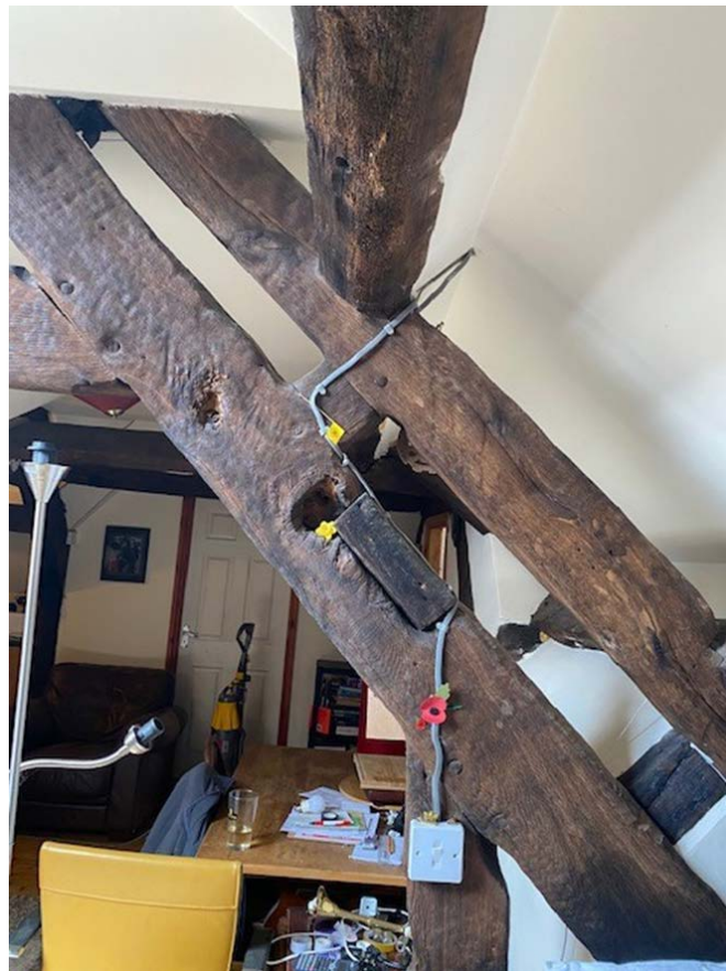
Figure 5: Potentially 'secondary' rafters behind timbers of the primary range roof, truss 1 / 1A, photograph taken from the south. [Alison Arnold]
