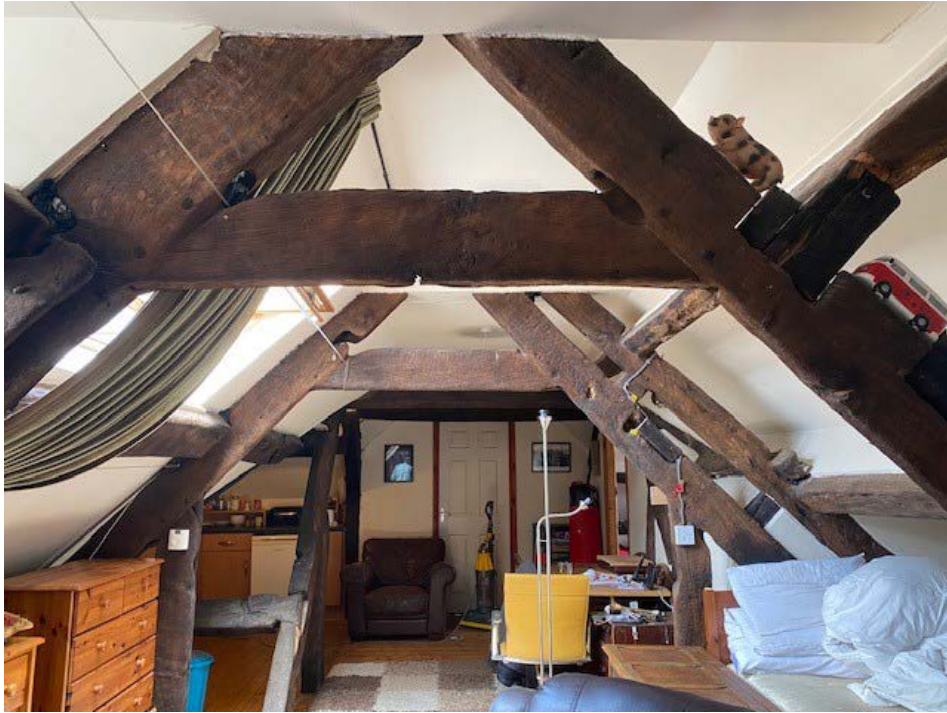
Figure 4: Main range roof, photograph taken from the south. [Alison Arnold]
