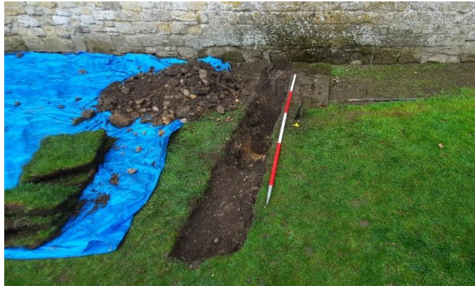
Plate 2: exploratory excavation trench in the vicinity of [gpr67] facing south-west towards the West Range Chamber Block with the grooved paving stone to the immediate right of the ranging rod receiving discharge from water chute S1 above (Source: Historic Property Restoration Ltd 2022).
