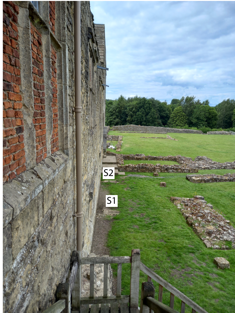
(A) West Range facing north showing location of water chutes
