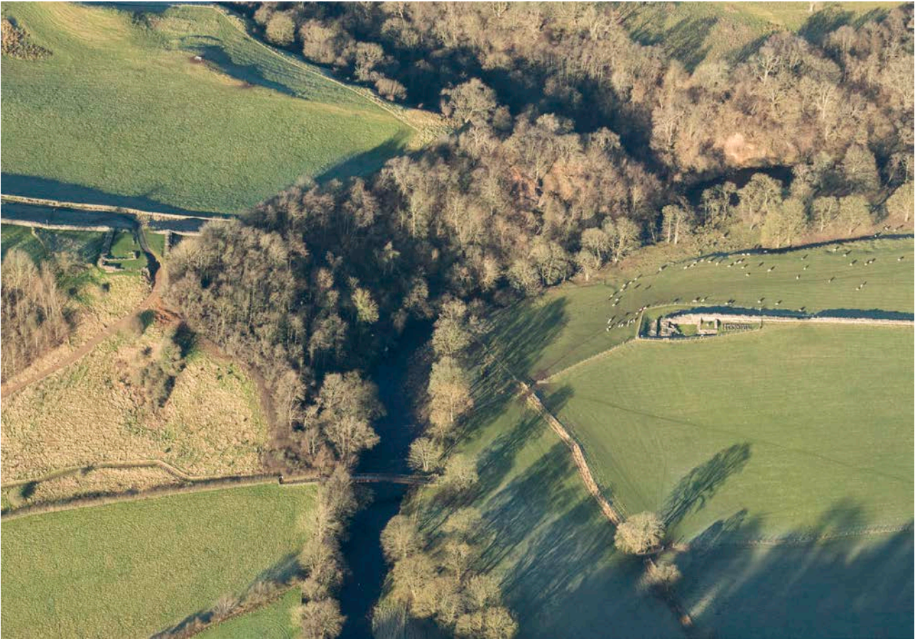
Figure 33: The footings of Willowford Bridge adjoined the Stone Wall east of the River Irthing (centre-right). The bridge carried the Wall across the River Irthing (centre) which has since migrated westward across the valley floor marooning the eastern abutment whilst burying or destroying much of the bridge, its western abutment and adjoining section of Stone Wall. Milecastle 49 (Harrow's Scar) is visible centre left. 33033_521 05-JAN-2017 © Historic England Archive.
