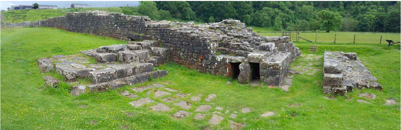
Figure 66: The excavated footings of the east end of Willowford Bridge have been consolidated and can be viewed as part of the Hadrian's Wall walk. Looking south-east. June 2017 © Historic England.
