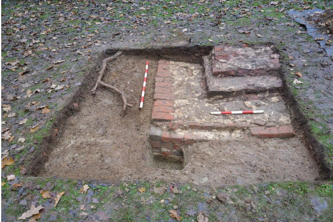
Fig 25: Brick footings in Trench K.
