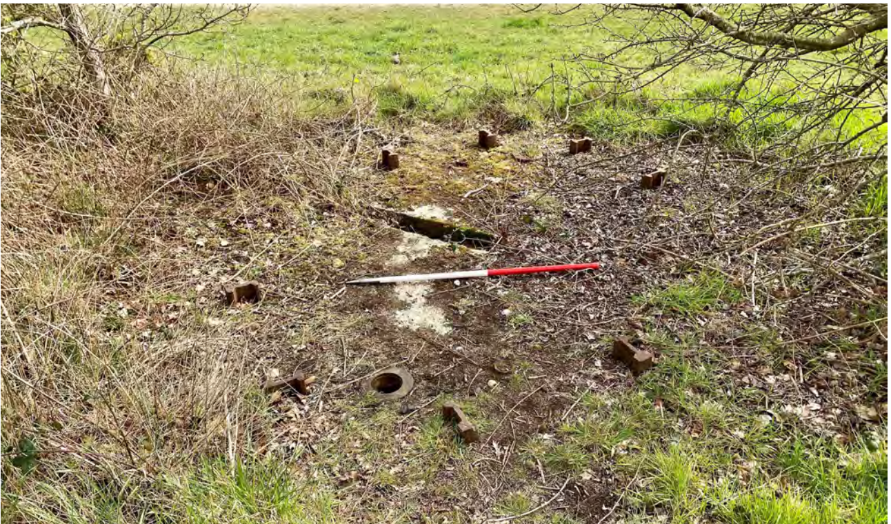
Figure 52: Concrete anti-aircraft gun holdfast, earthwork survey area 2, looking south, 1m scale, 01/04/2021 [Olaf Bayer. © Historic England Archive. AF00452/P010]
