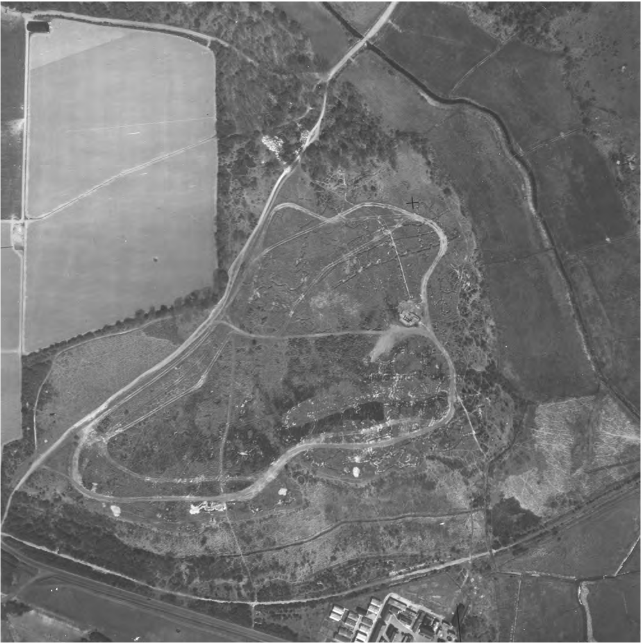
Figure 25: Browndown trenches in April 1953 [Historic England Archive, RAF Photography. Extract of RAF/L82/F766/0349 21-APR-1953]
