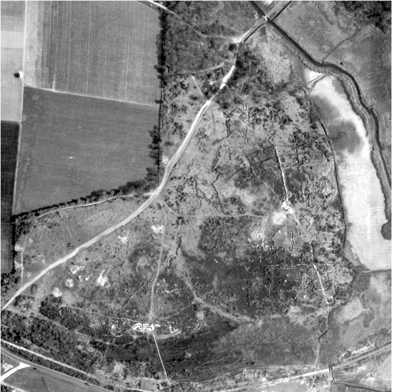
Figure 22: Browndown trenches in April 1946 [Historic England Archive, RAF Photography. Extract of RAF/3GTUD/IK/163 PTIII 5110 2-APR-1946 ]
