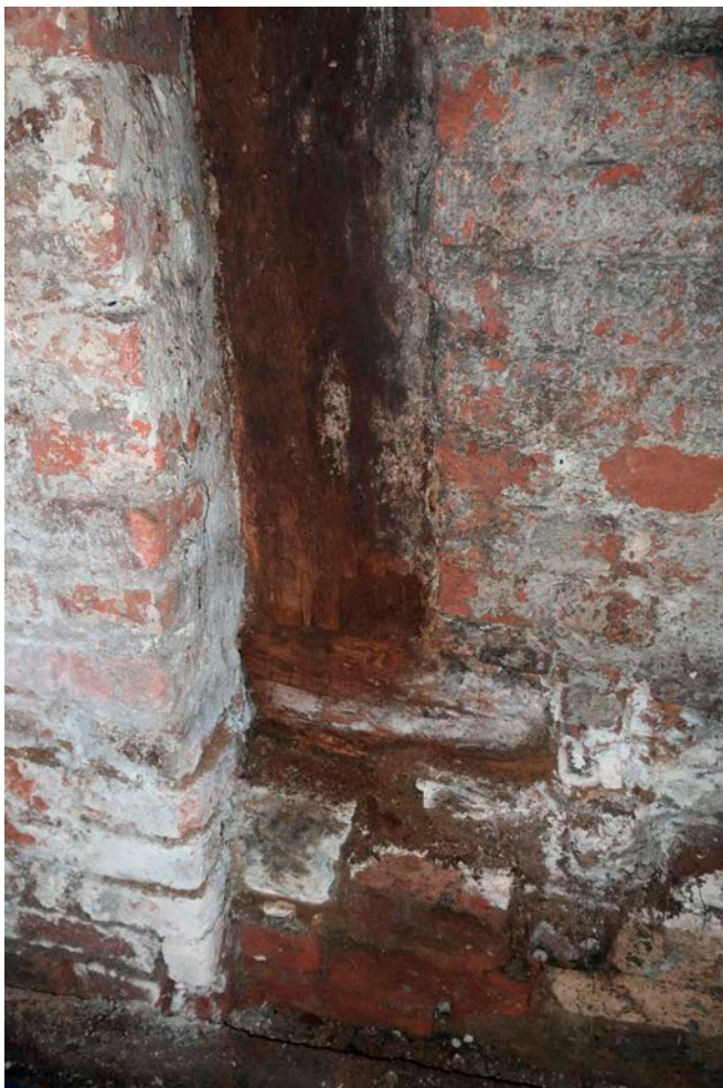
Figure 77: The cellar under No. 21 (bay E), showing timber frame in the east wall (the partition wall between Nos 21 and 19A), looking east, with part of the sill beam and a post in situ. [Rebecca Lane © Historic England]
