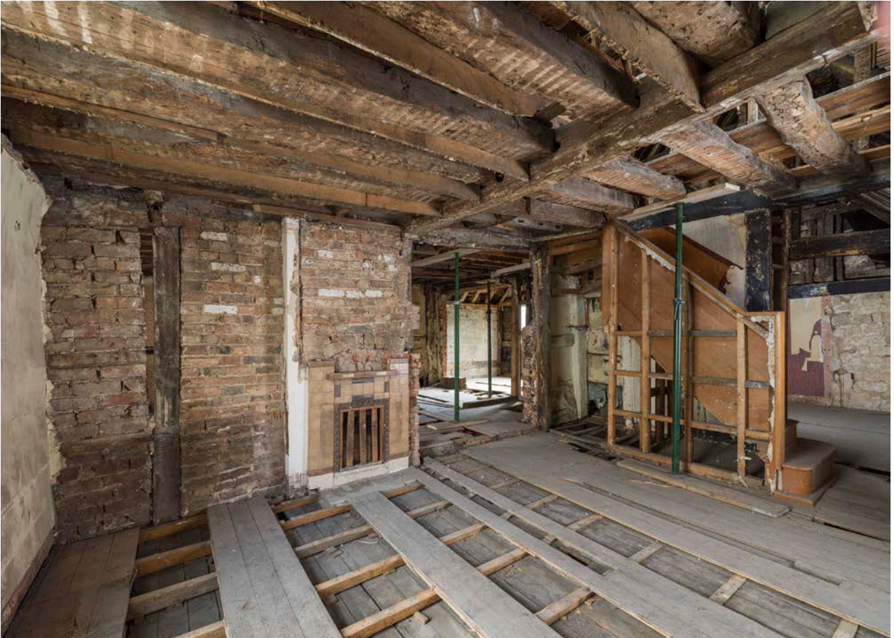
Figure 87: First floor of bay E (No. 21), looking south-east, showing the remaining framing of frame V. [Steve Baker © HEA DP325627]
