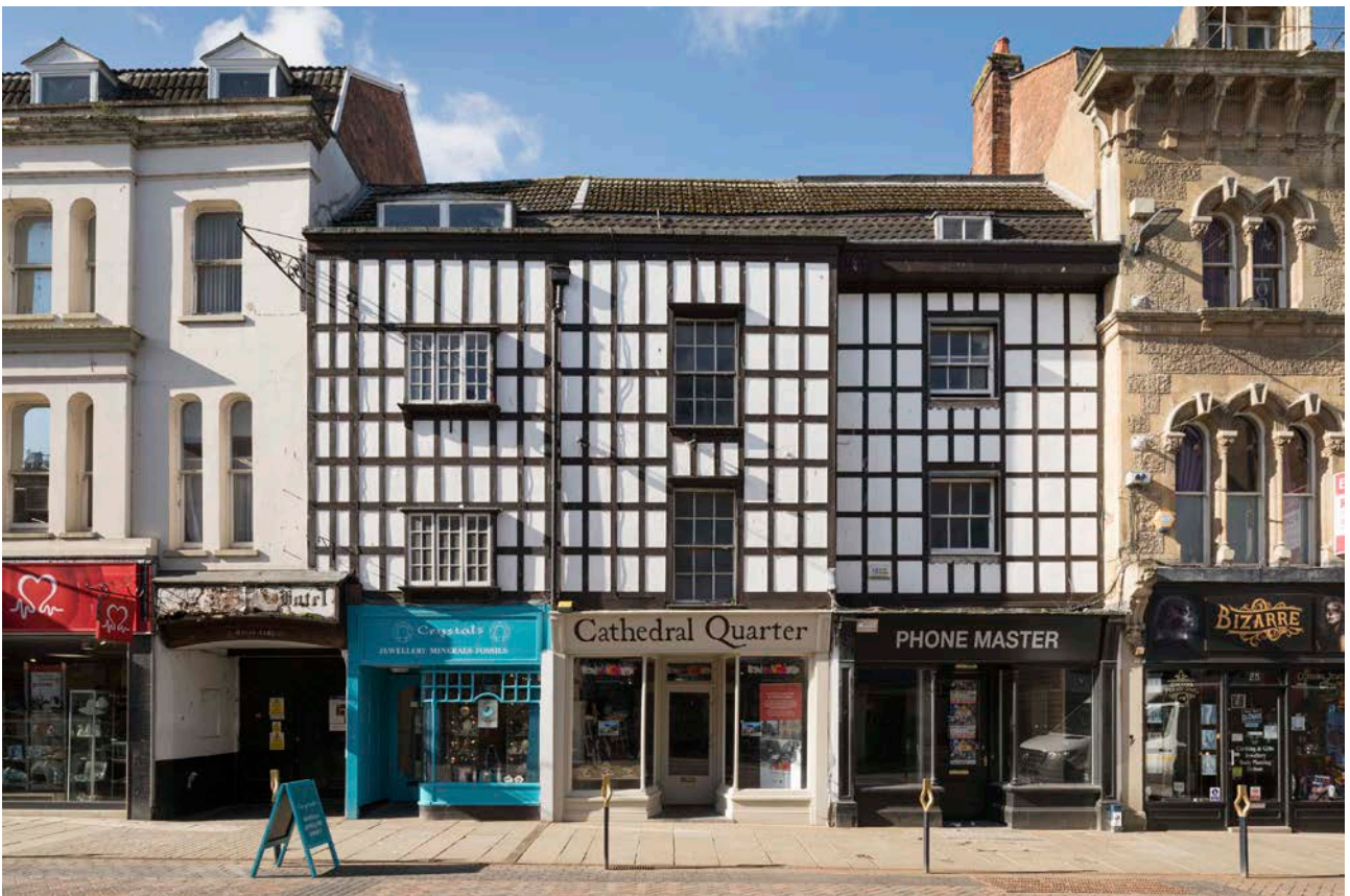
Figure 146: North elevation of the street-front range, fronting onto Westgate Street, showing the fake timber framing applied to no. 19A in the 1920s, and to Nos 21 and 23 probably in the 1970s, looking south. [Steve Baker © HEA DP325614]
