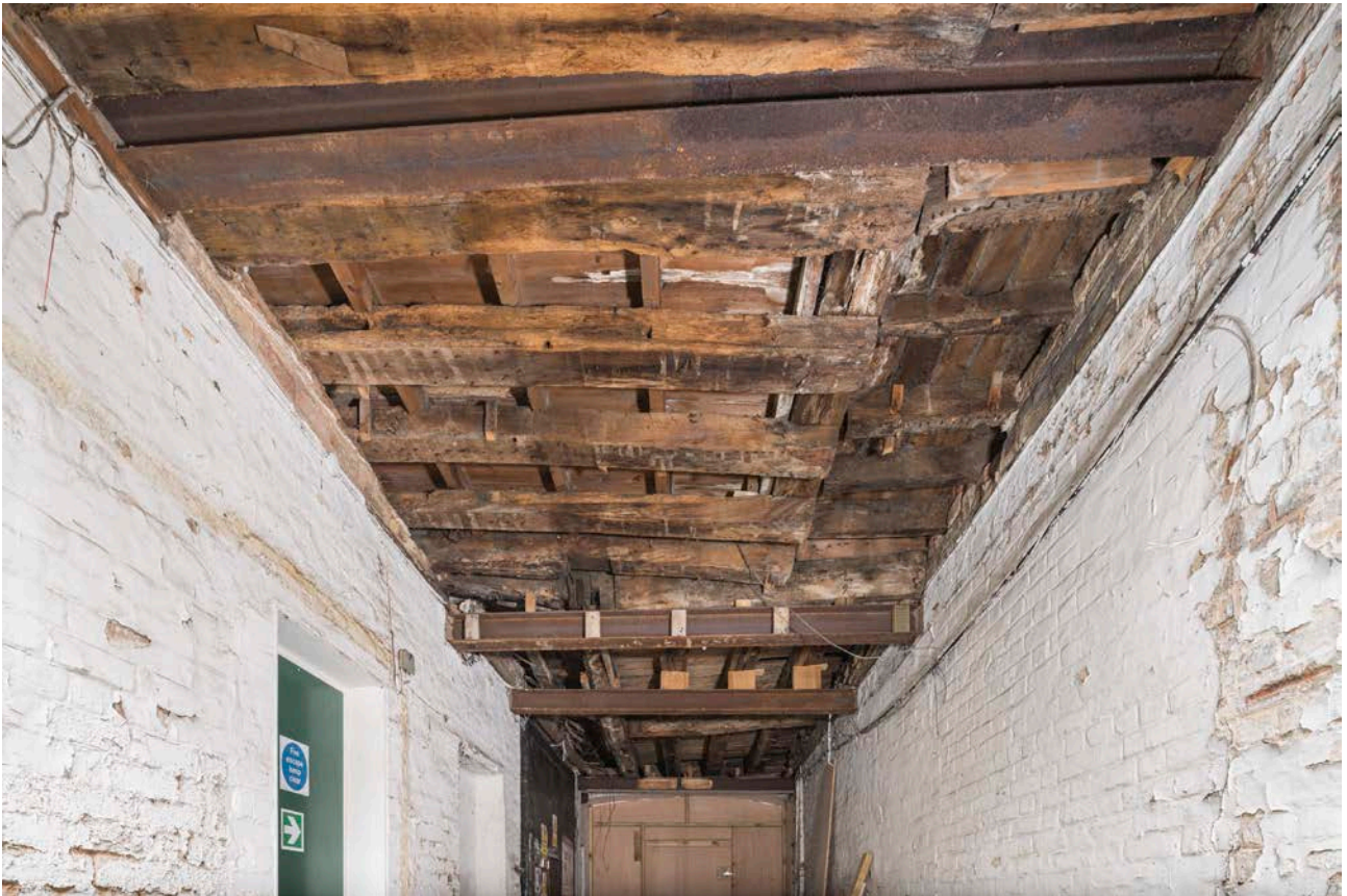
Figure 106: The jetty of the north-east corner bay, as visible from the passageway below, looking north. [Steve Baker © HEA DP325688]
