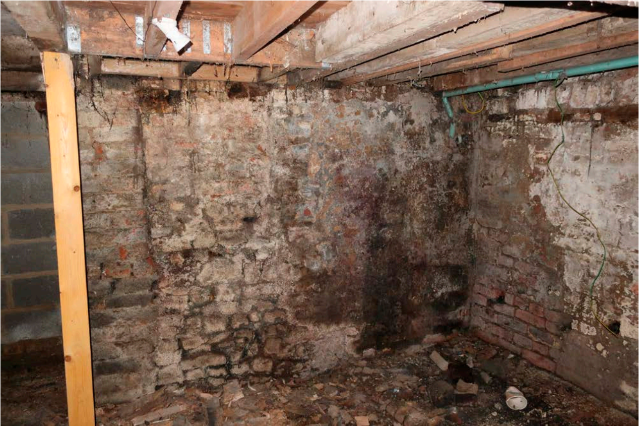
Figure 76: The cellar under No. 21 (bay E), looking north-east, showing the rubble stone walling of the north elevation. [Rebecca Lane © Historic England]
