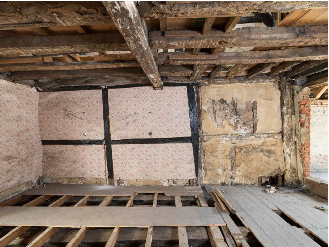
Figure 82: Framing of frame IIII of the street-front range at first-floor level, looking east. [Steve Baker © HEA DP325632]
