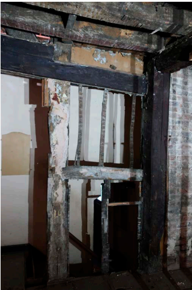
Figure 50: The western elevation of the great inn range in bay F, looking west, showing surviving timber framing of the west wall. [Rebecca Lane © Historic England]
