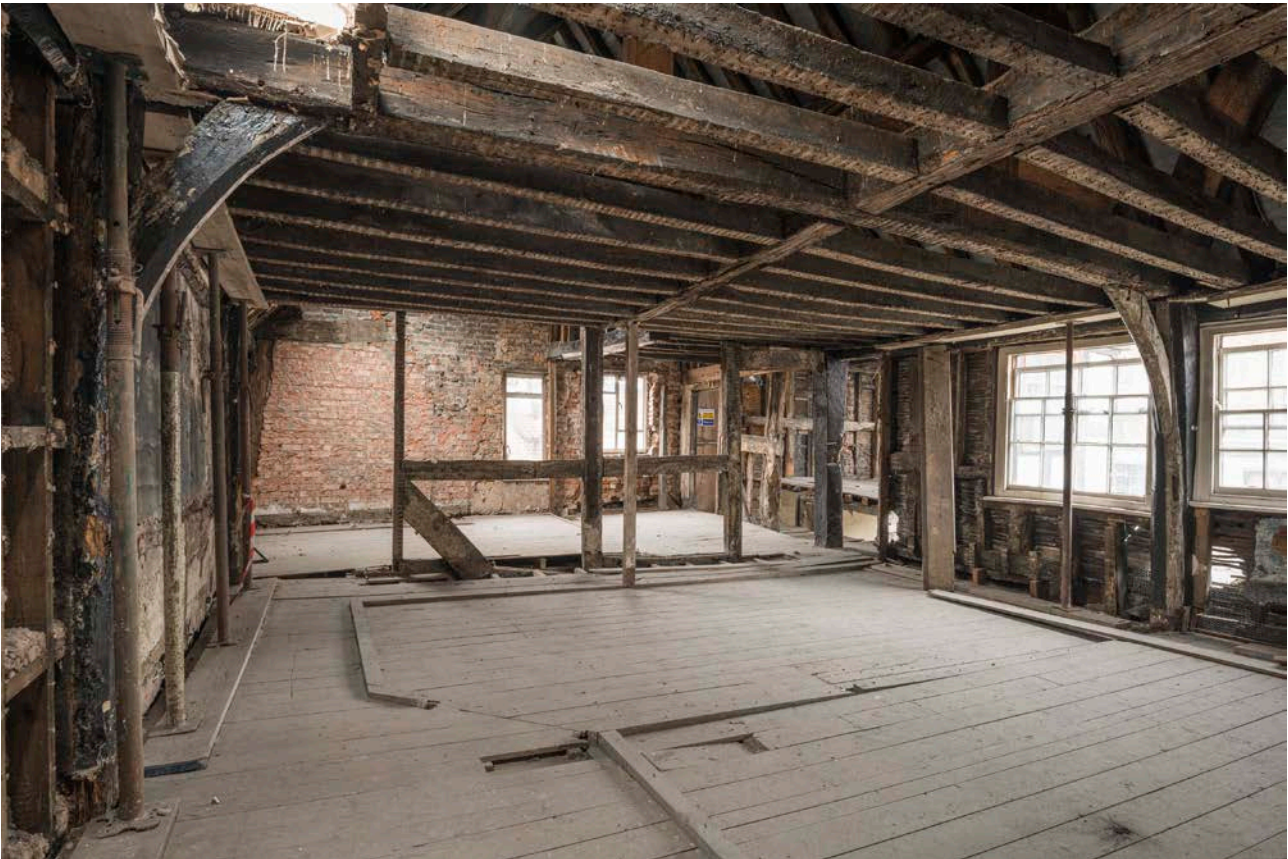
Figure 111: The first-floor central room of the great inn range, looking south-west, showing the ceiling inserted over the room, possibly in the 16th century. [Steve Baker © HEA DP325588]
