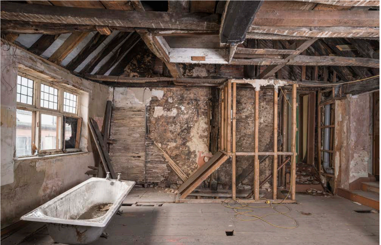
Figure 103: The northern face of frame IIII, looking south, showing smoke blackening on the frame and infill panels at first-floor level and in the roof. [Steve Baker © HEA DP325606]
