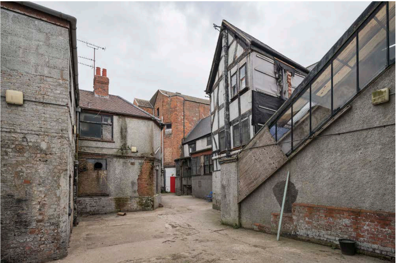
Figure 144: The courtyard of the Fleece, showing the brick building added at the southern end of the west range, added in the early 20th century, looking north-east. [Steve Baker © HEA DP325649]
