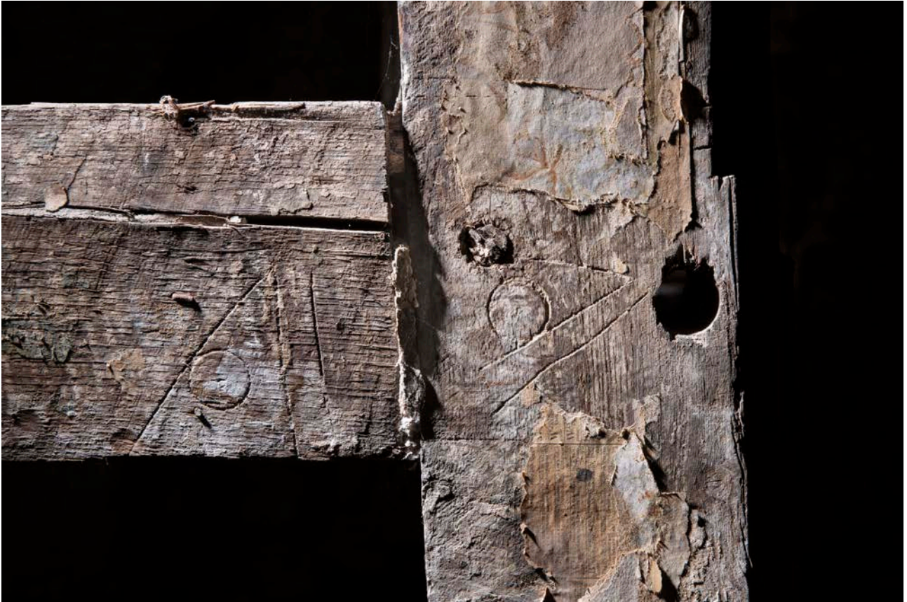
Figure 66: Detail of carpenters' assembly mark on the partition stud of frame VI, looking south. [James O. Davies © HEA DP435647]
