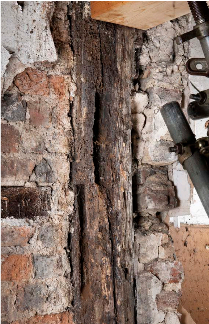
Figure 42: The west post of frame II showing the mortices which indicate the position of an oriel window, looking north-east. [James O. Davies © HEA DP435633]
