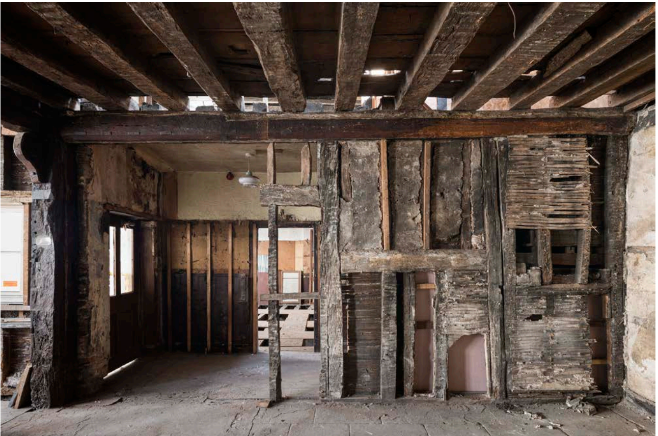
Figure 45: The ground-floor partition forming part of frame IV, looking north. [Steve Baker © HEA DP325620]
