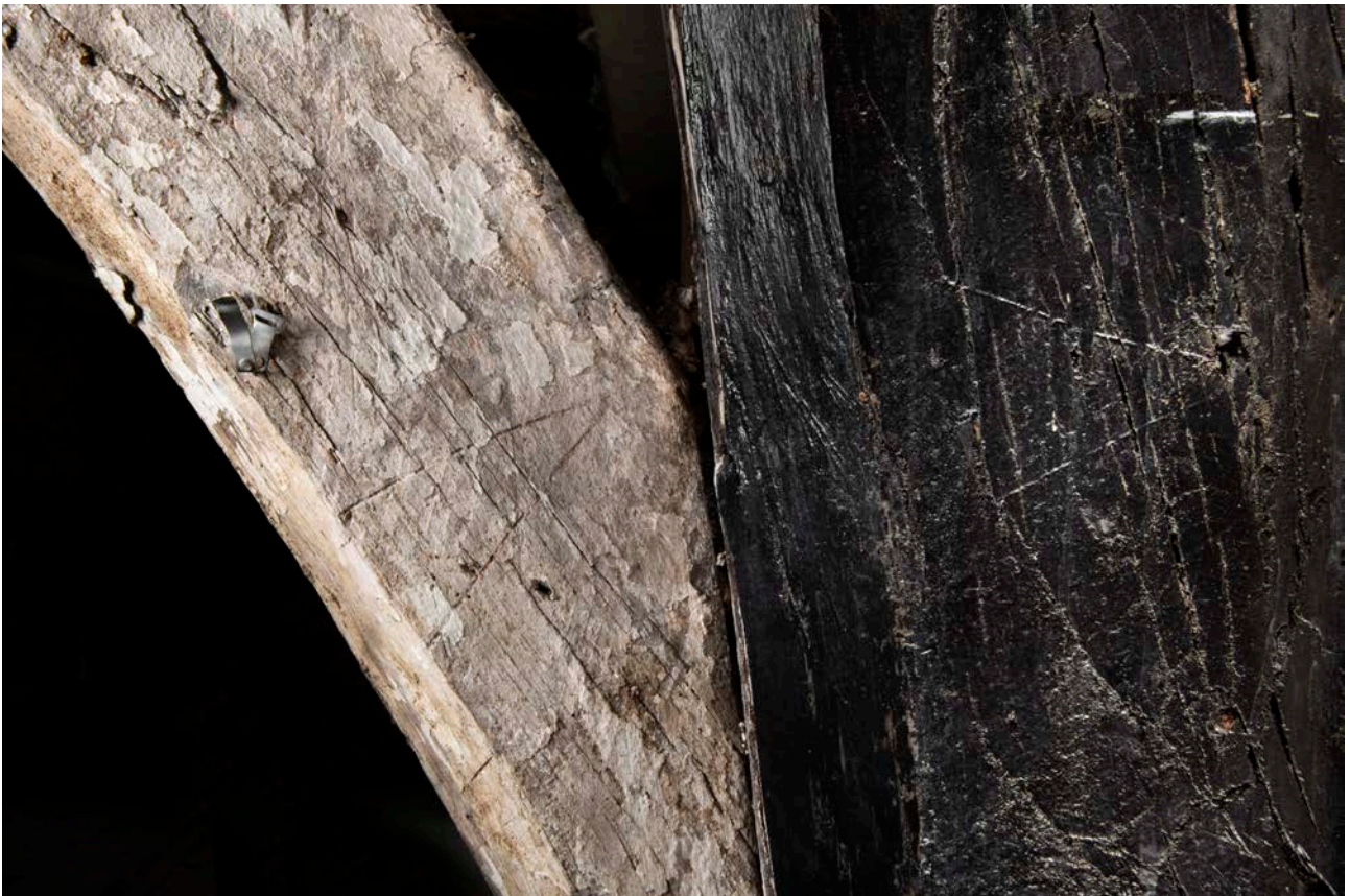
Figure 63: The up-brace of frame V, showing the carpenters' assembly mark on the brace and the adjacent west post, looking south. [James O. Davies © HEA DP435645]
