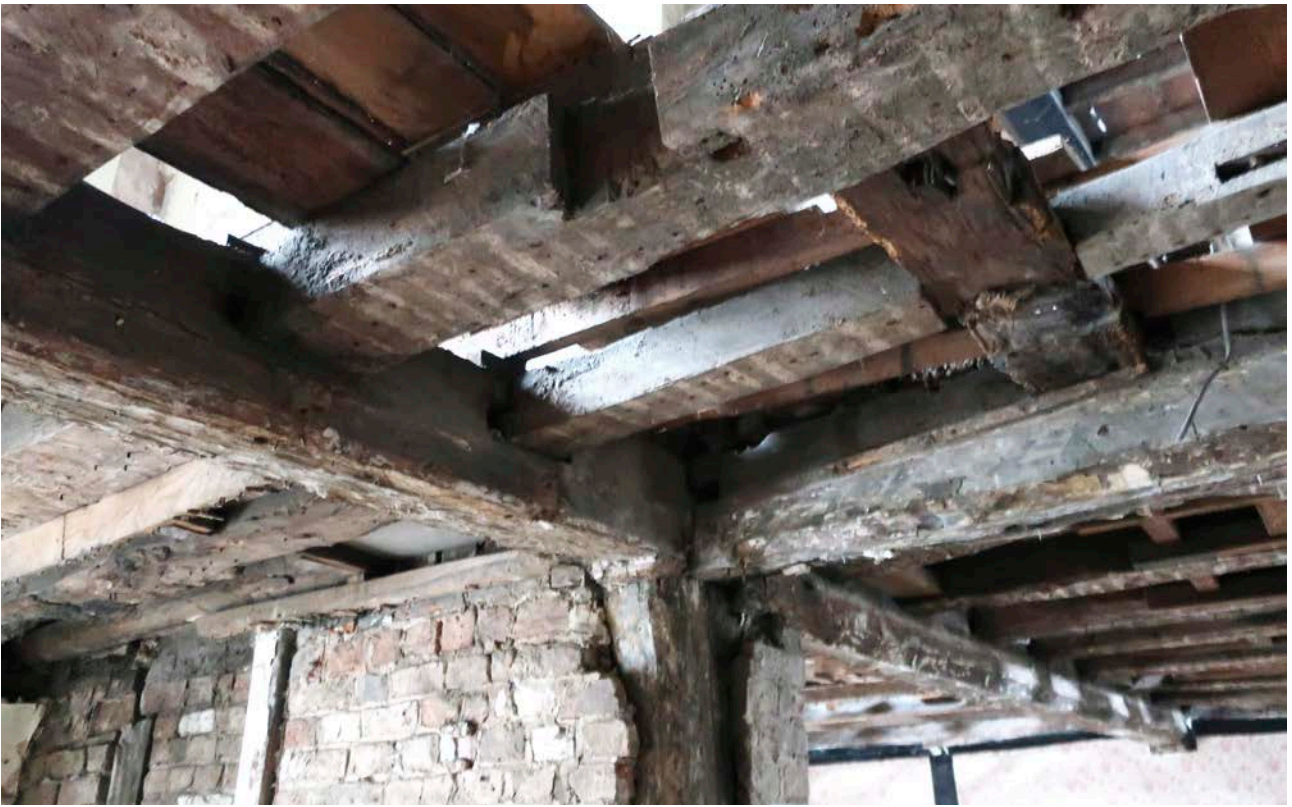
Figure 90: First floor of bay E (No. 21) showing the stair trimmer beam in the ceiling and the possible stair position in the south-east corner, looking north east. [Rebecca Lane © Historic England]
