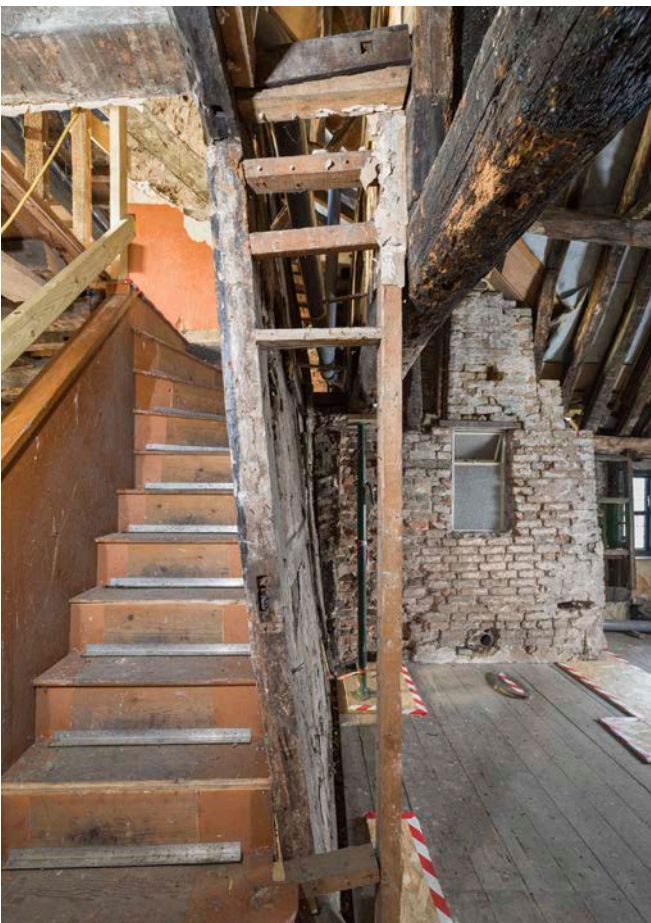
Figure 87: First floor of bay E (No. 21), looking south-east, showing the remaining framing of frame V. [Steve Baker © HEA DP325627]
