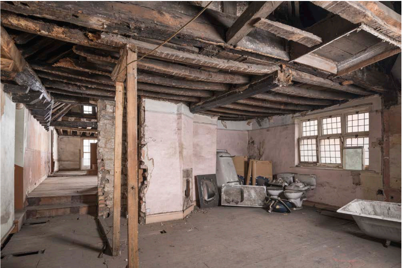
Figure 139: First-floor level in the west range, looking north-west, showing the rebuilt western wall of the range, with the earlier wall plate supported on timber brackets. [Steve Baker © HEA DP325610]
