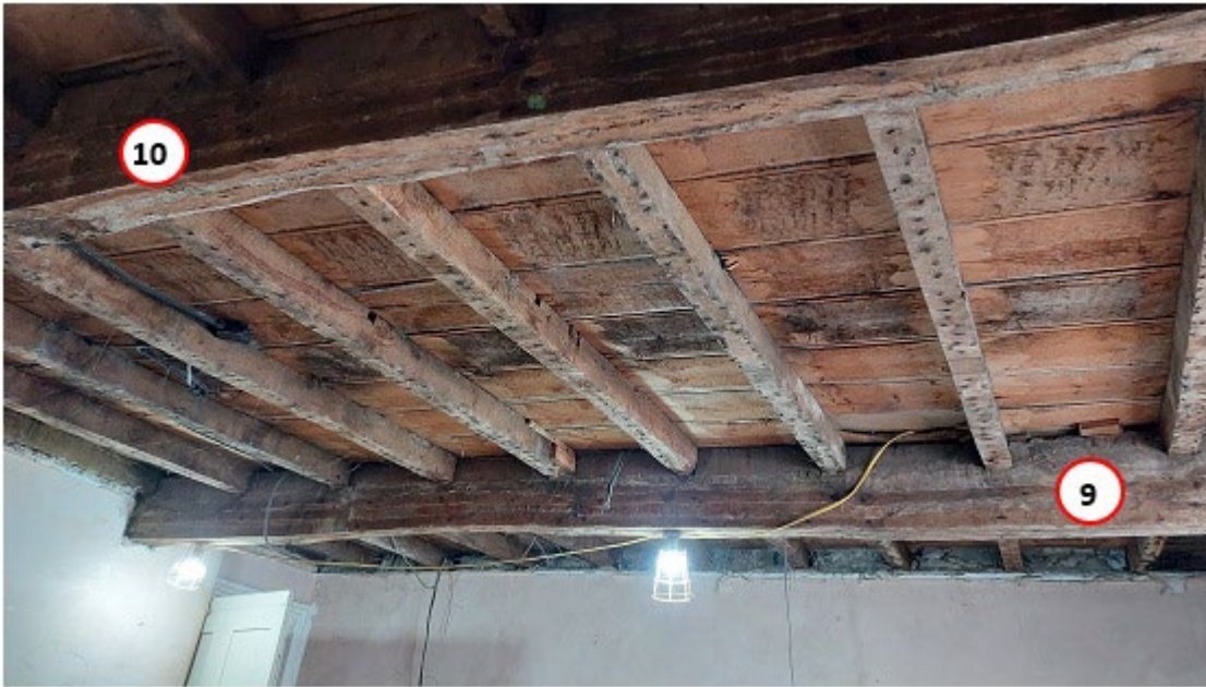
Figure 7: 2nd floor, north-west room, annotated photograph (looking west) to help identify sampled timbers (photograph Robert Howard)
