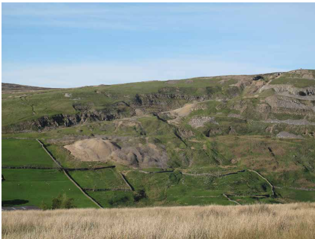
Figure 12.3 Fell End from the Reeth- Arkengarthdale road, showing what Dunham described as Fell End Hush “one of the most spectacular mining excavations in the whole district” (Dunham 1985, 141). The large spoil heaps centre left are from Fell End Level, the orange tones of the unvegetated mineral rich material contrasting with the greyer hues of the driving waste piles, parts of which have been colonised by vegetation
