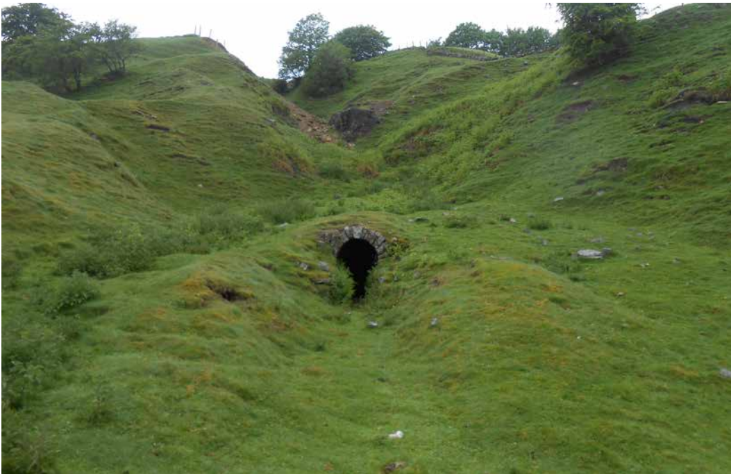
Figure 12.6 An unnamed level, marked as Old Level on the 1 st edition OS 25" map at NZ01680244. The keystone on the intact portal entrance is dated to the 19 th century and is a relatively rare survival of an intact mine portal. The level appears to have been driven along the vein directly underneath the area affected by hushing or opencast working.
