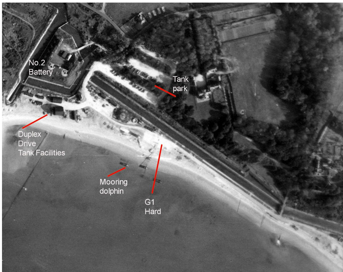
Figure 65: Aerial view of the site of the Duplex Drive Tank saltwater testing facility and G1 embarkation hard adjacent to No. 2 Battery on Stokes Bay. Extract of RAF/3G/TUD/UK/163/PIII 5110 20-APR-1946. Historic England Archive (RAF Photography).
