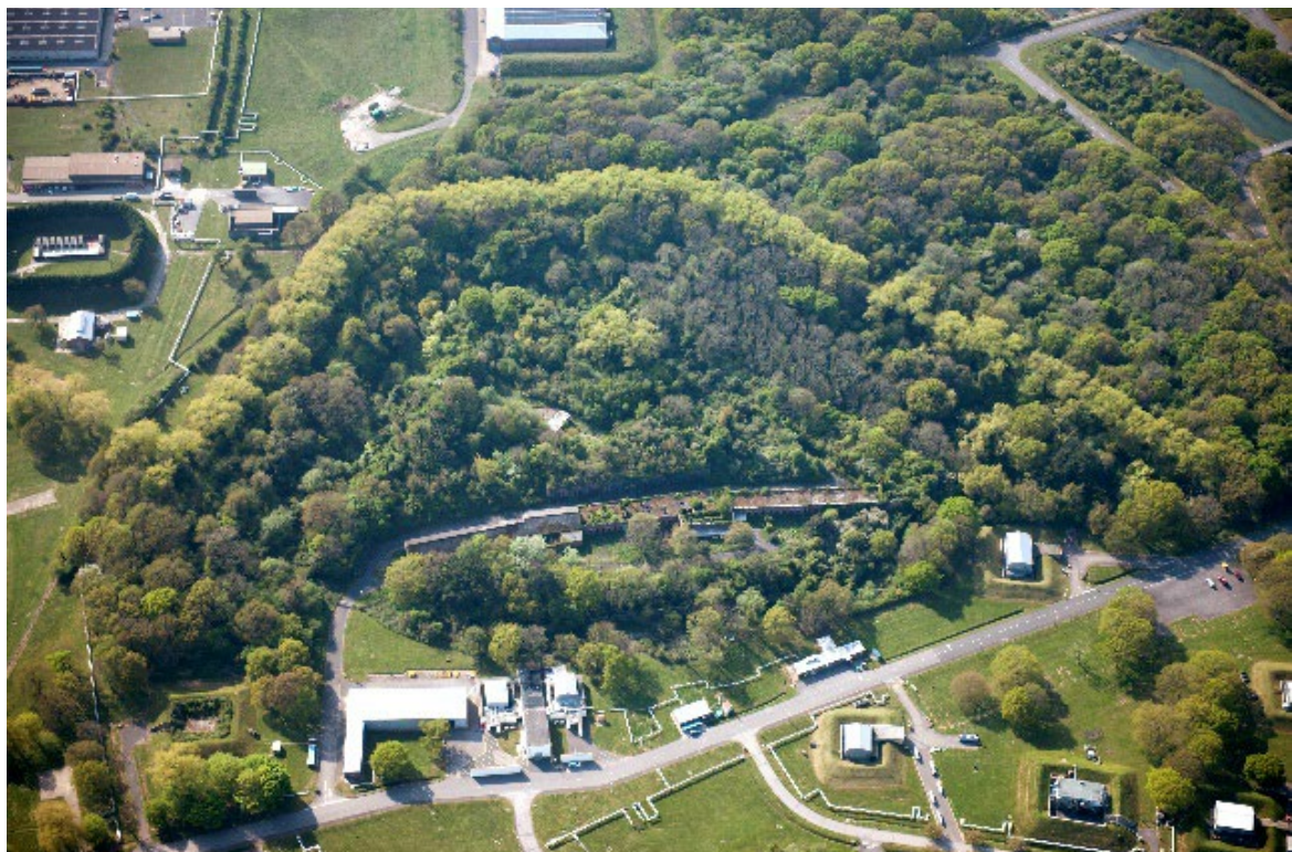
Figure 29: Aerial view of Fort Elson. HEA 26944_033 19-APR-2011 © Historic England Archive.
