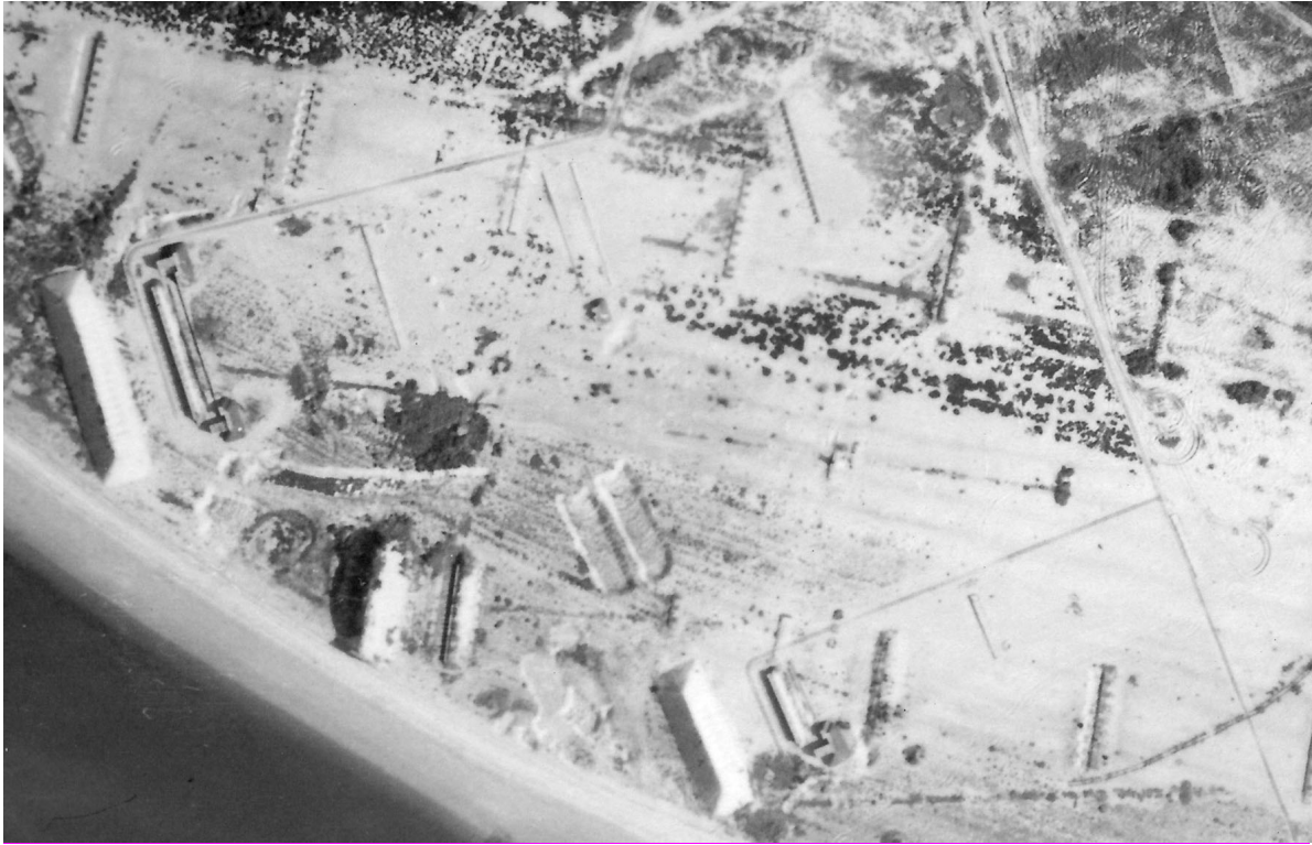
Figure 35: Aerial view of part of the ranges at Browdown (South) showing a number of overlapping ranges from different periods. The largest and most substantial range (in use at the time of the photograph) is served by the tramway. Extract of RAF/3G/TUD/UK/163 VP2 5110 20-APR-1946 Historic England Archive (RAF Photography)
