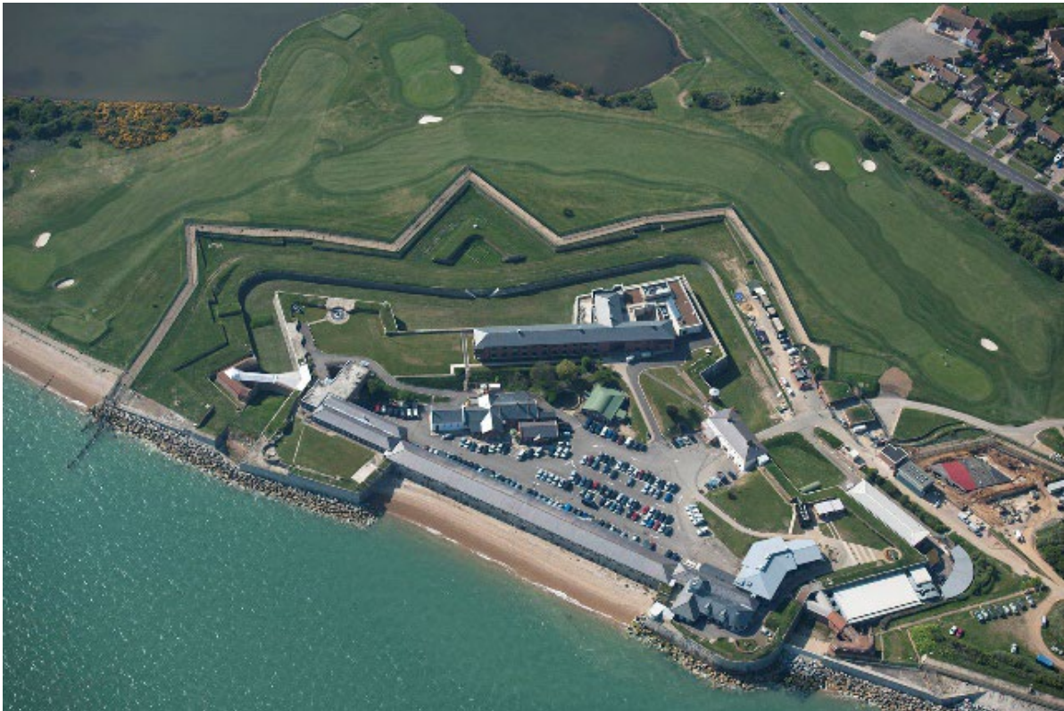
Figure 31: Aerial view of Fort Monckton. HEA 26941_024 19-APR-2011 © Historic England Archive.
