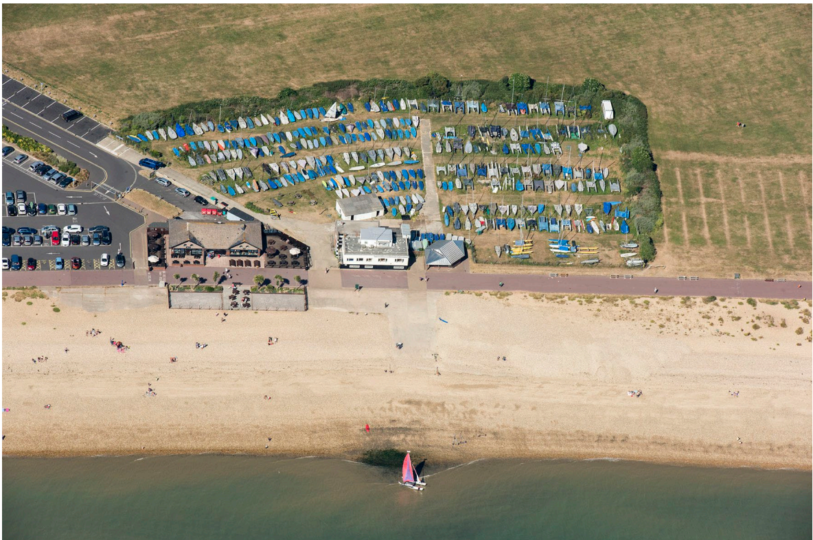
Figure 61 The former location of G3 embarkation hard at Stokes Bay Sailing Club. The concrete areas and slip way are modern. The access road to the hard is fossilised in the north-eastern side of the car park. HEA 33560_034 26-JUN-2018 © Historic England Archive.
