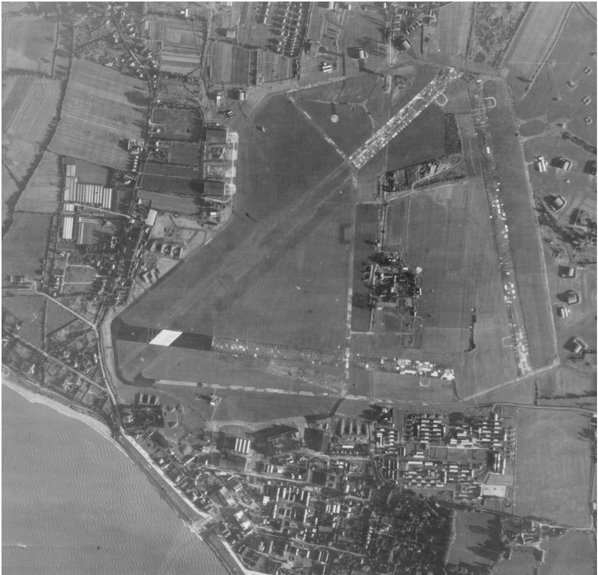
Figure 45: Aerial view of Lee-on-Solent airfield and seaplane base in 1946. Extract of RAF/CPE/UK/1794 4022 21-SEP-1946 Historic England Archive (RAF Photography).
