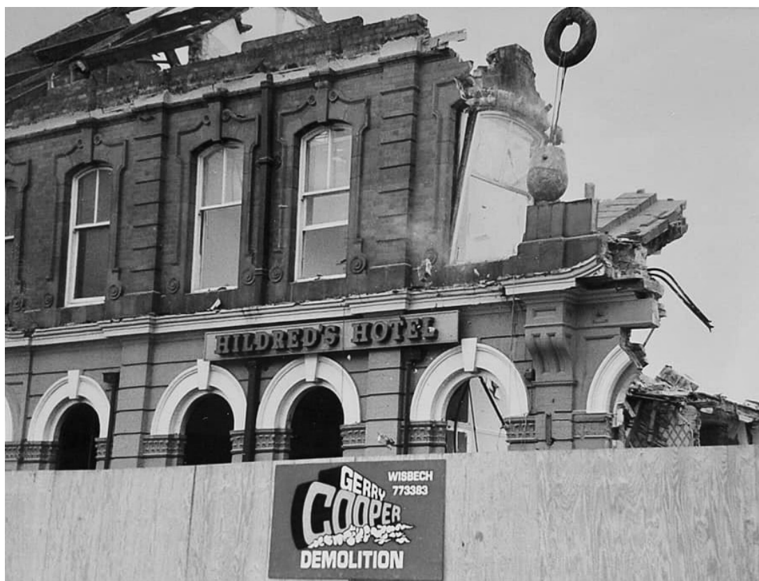
Demolition of Hildred's Hotel, Skegness, c.1987 © Steven Andrews, Hildred's Centre
