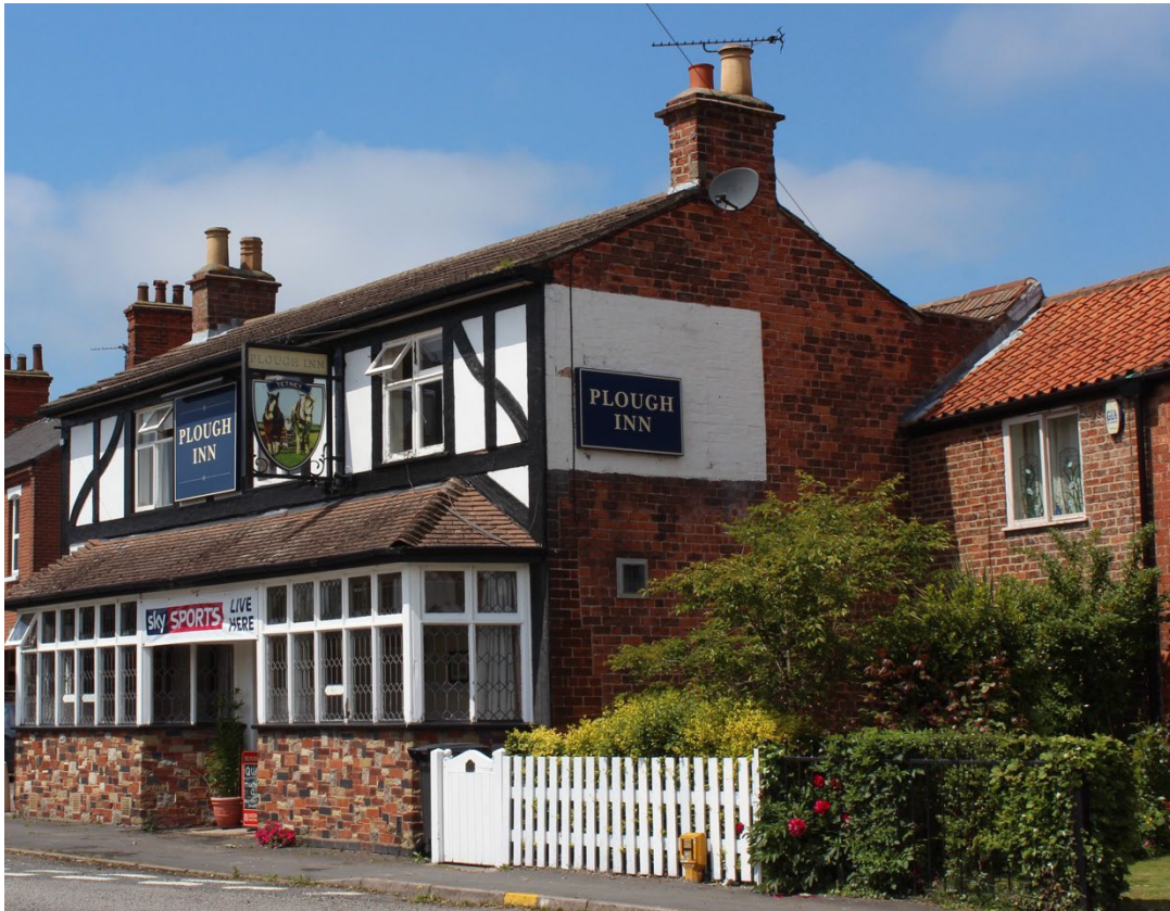
Plough Inn, Tetney, the bay windows and stud work were added later © Historic Place Team, LCC
