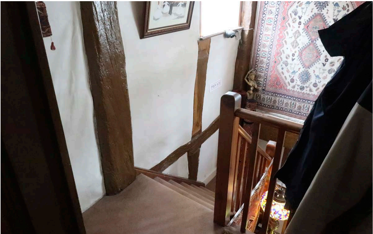
Figure 49: The staircase in the south bay, seen from the first floor. [Johanna Roethe © Historic England]
