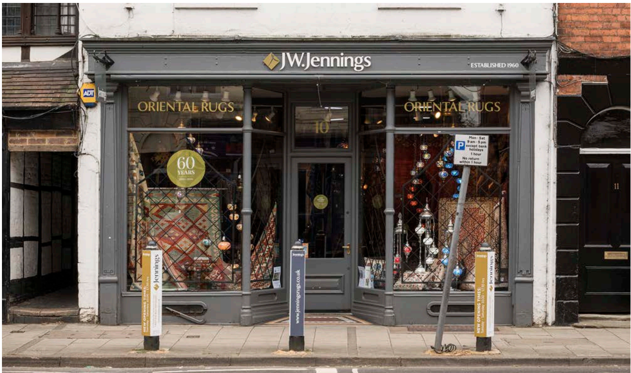
Figure 46: The late 19th-century shopfront in 2023. [Steven Baker © Historic England, DP325768]
