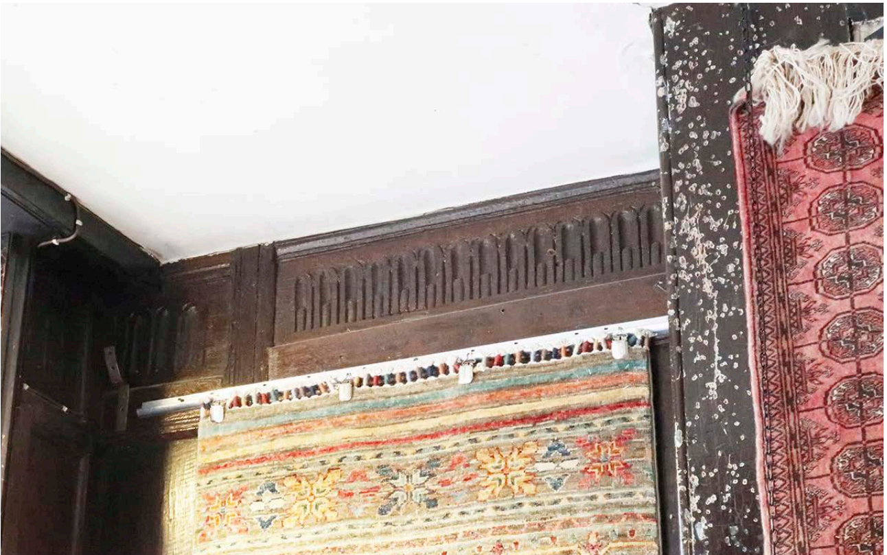
Figure 48: Mismatched arcading patterns in the frieze to the left of the chimneybreast in the north bay at ground-floor level. [Johanna Roethe © Historic England]
