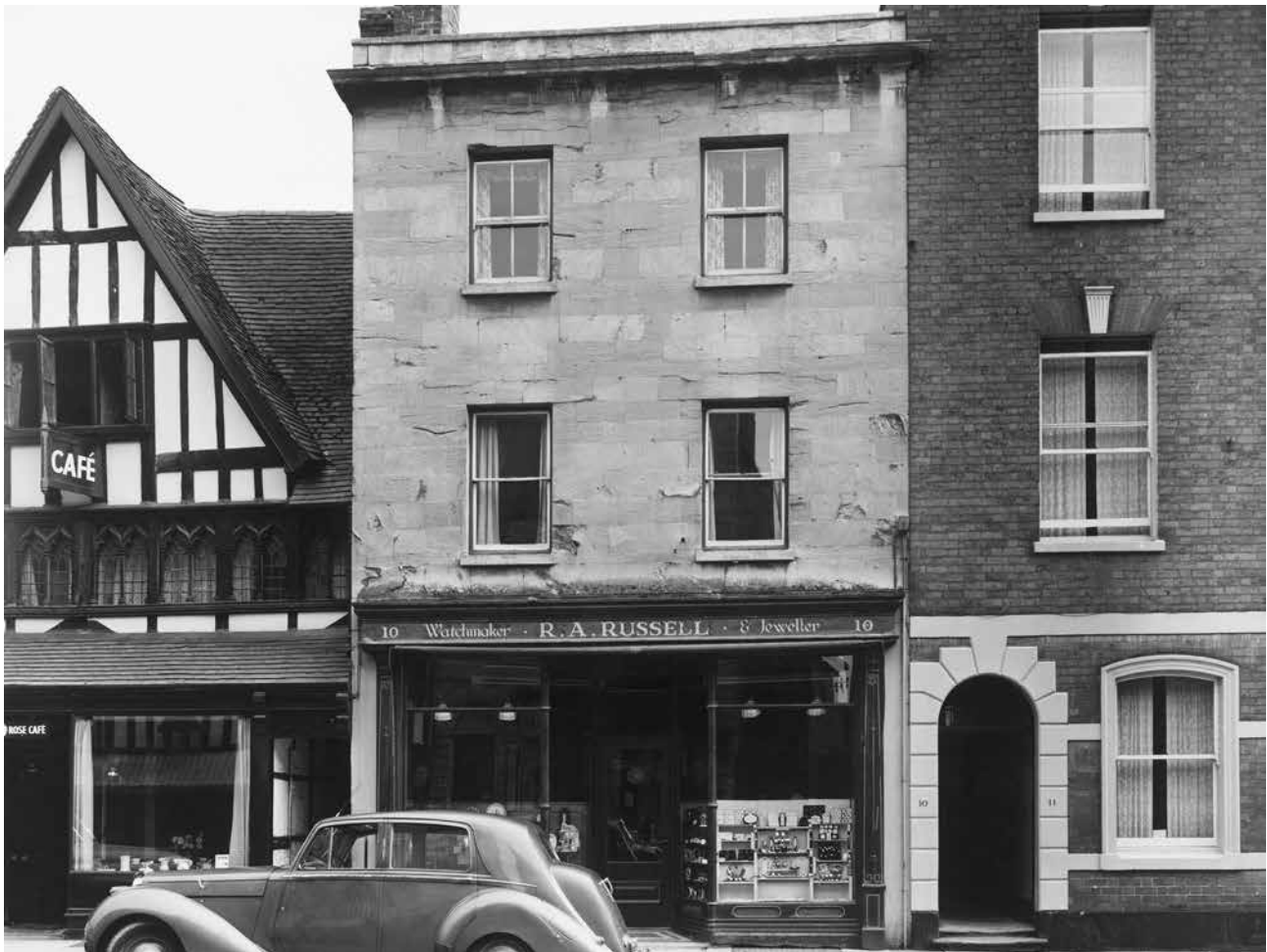
Figure 10: 10 Church Street in 1957. [Source: Historic England Archive, TEW01/01/X74794]
