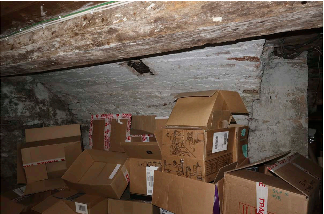
Figure 41: The brick coving on the south side of the chimneystack in the cellar. [Johanna Roethe © Historic England]
