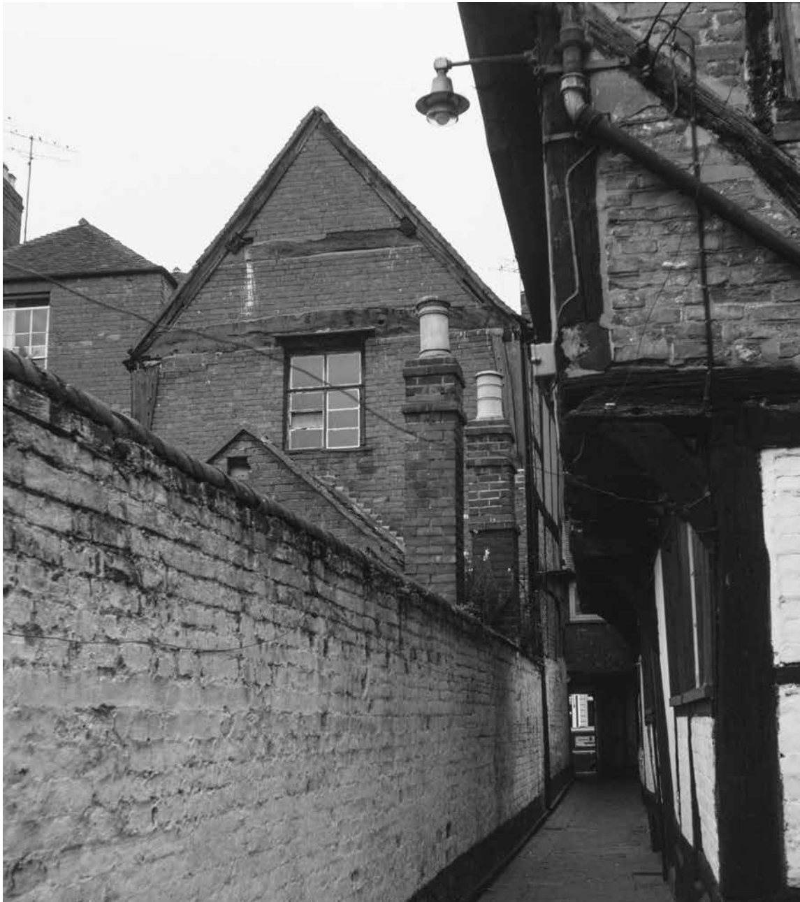
Figure 11: Detail of a photograph taken by Stanley Jones in about 1966-8, showing the rear elevation of 10 Church Street from Lilley's Alley. [© Historic England Archive, SJC01/03/0010]
