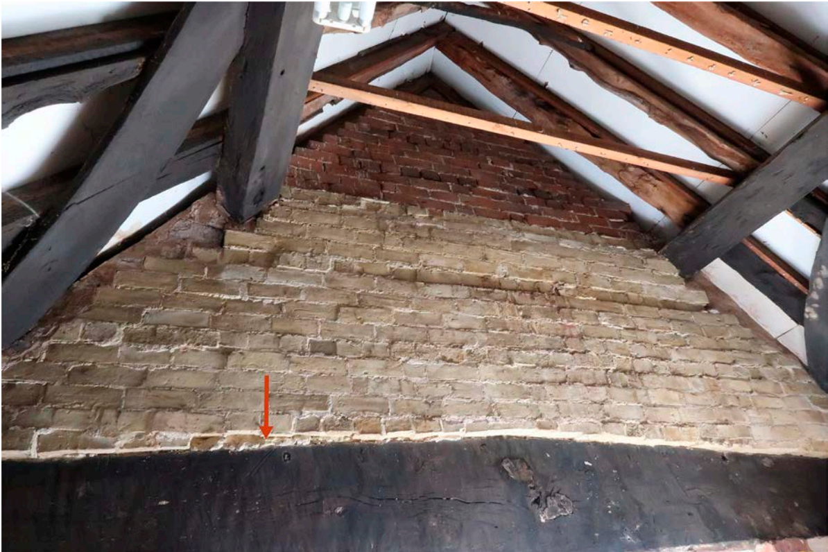
Figure 26: The upper part of the south truss of the south bay. The red arrow indicates the location of the carpenter's mark to the left of a peg hole. [Johanna Roethe © Historic England]
