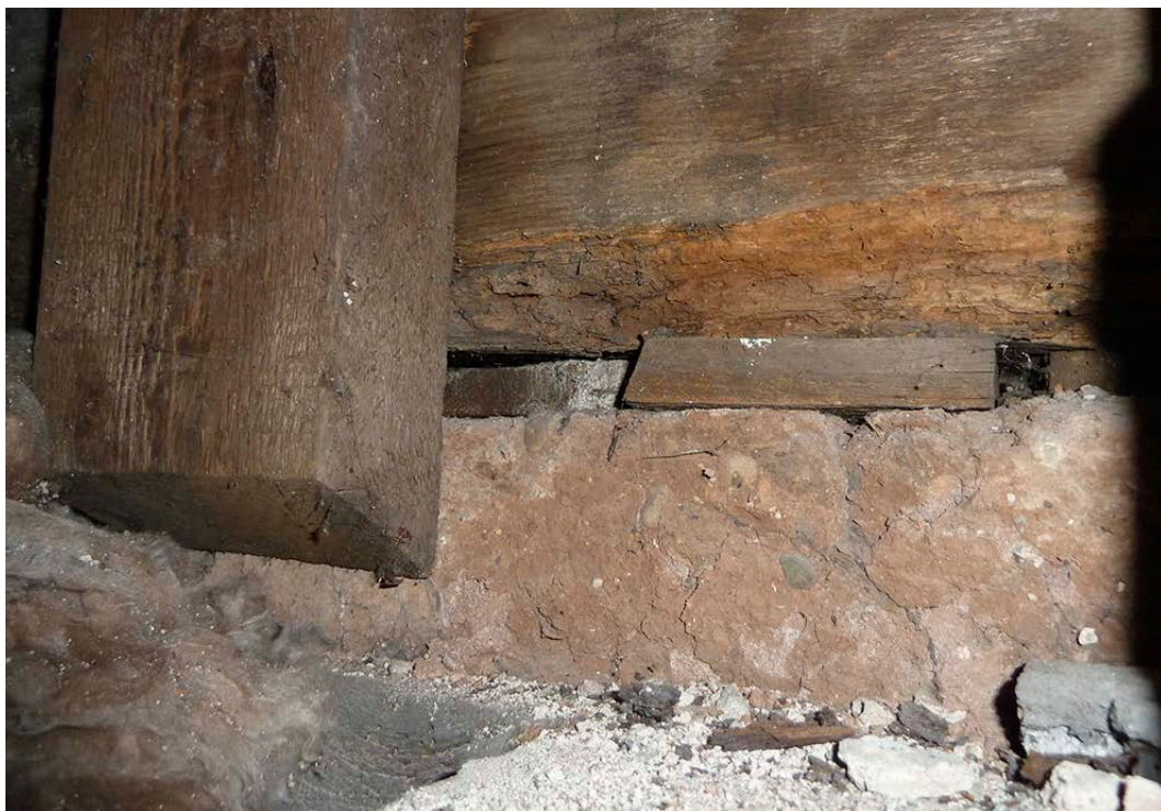
Figure 34: Remnant of daub below the tiebeam of the north truss in the middle bay. [Johanna Roethe © Historic England]
