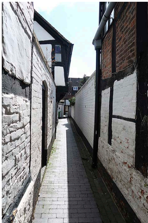
Figure 19: View of Lilley's Alley looking south, with part of the east elevation of 10 Church Street to the right. The east post of the southern pair of posts is just visible behind the downpipe. [Abigail Lloyd © Historic England]
