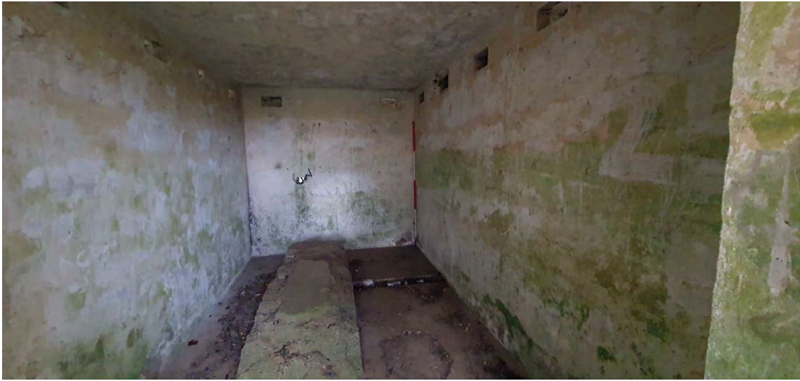
Plate 16: Radar powerhouse interior, looking north.
