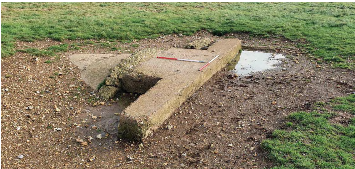
Plate 13: Control bunker (29), looking east.
