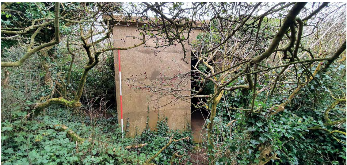
Plate 15: Radar powerhouse, exterior looking north.
