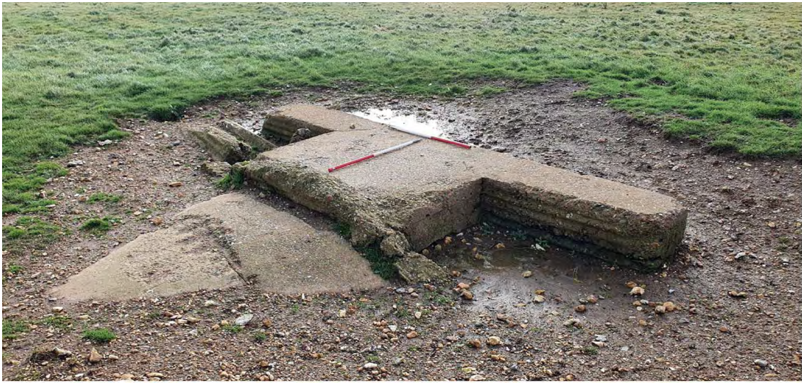
Plate 14: Control bunker (29), looking south-east.
