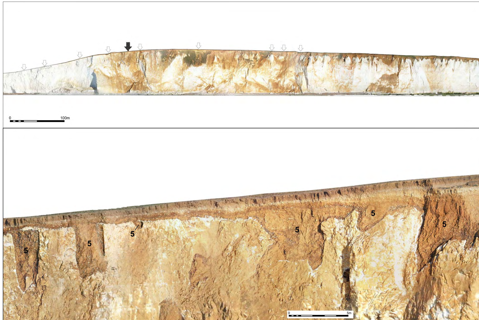
Figure 31: Solution features east of the northern rampart ditch and bank.
