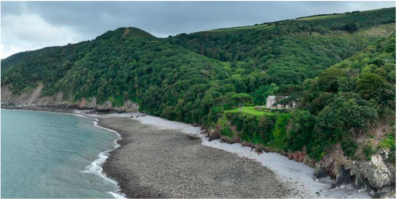
Figure 63: Glenthorne House - a listed building set in a geological SSSI and coastal woodland on Exmoor
