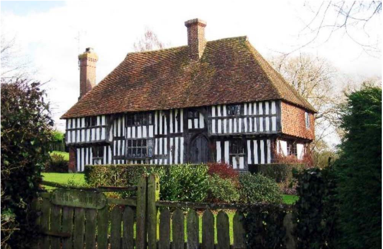
Figure 50: Medieval building in the High Weald NCA
