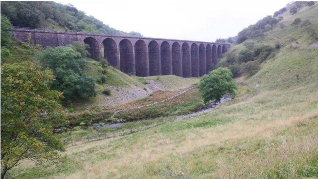
Figure 54: Smardale viaduct in Orton Fells NCA
