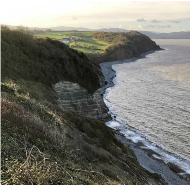
Figure 21: The eroding sea cliff at Daw's Castle, changing from heritage site to coastal cliff habitat (photo: Kate Jeffreys)
