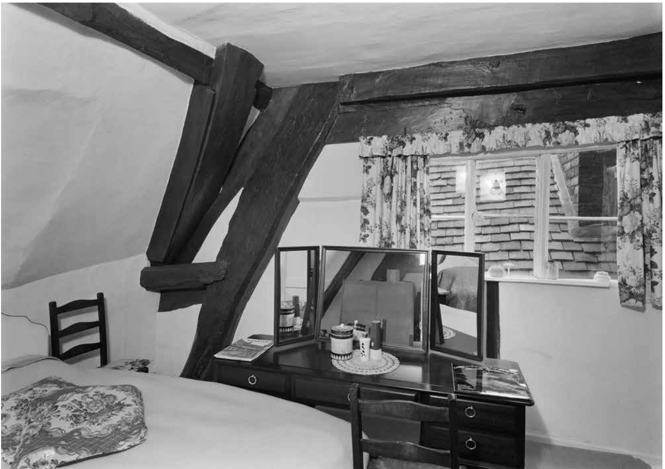
Figure Appendix 3.23: The north side of the east blade of the main range's frame 5, at first-floor level. [© Crown Copyright. Historic England Archive, bb72/00626]
