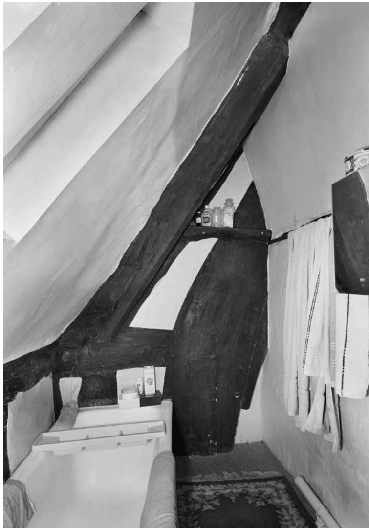
Figure 33: The south side of the west blade of frame 1, at the modern first-floor level, photographed in 1971. [© Crown Copyright. Historic England Archive, bb72/00622]
