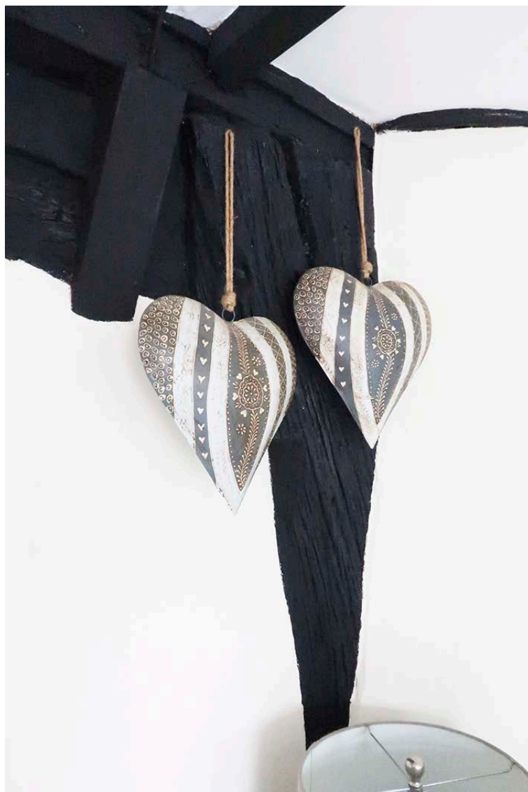
Figure 59: The lower part of the south side of the east blade of frame 5, with later ceiling timbers and bracket. [Johanna Roethe © Historic England]
