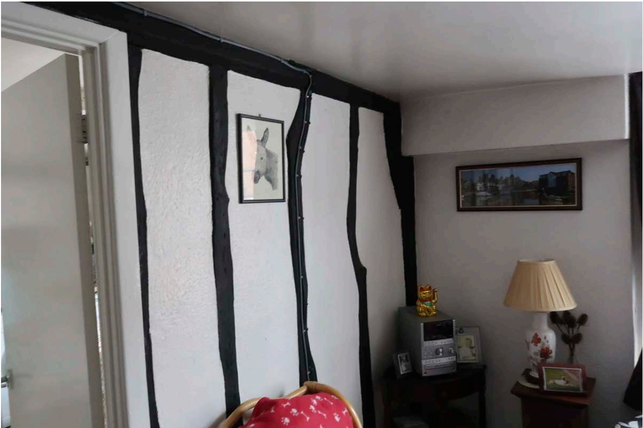
Figure 85: The 17th-century timber stud partition and the original central jowled post in the east room on the first floor of the front range. [Johanna Roethe © Historic England]
