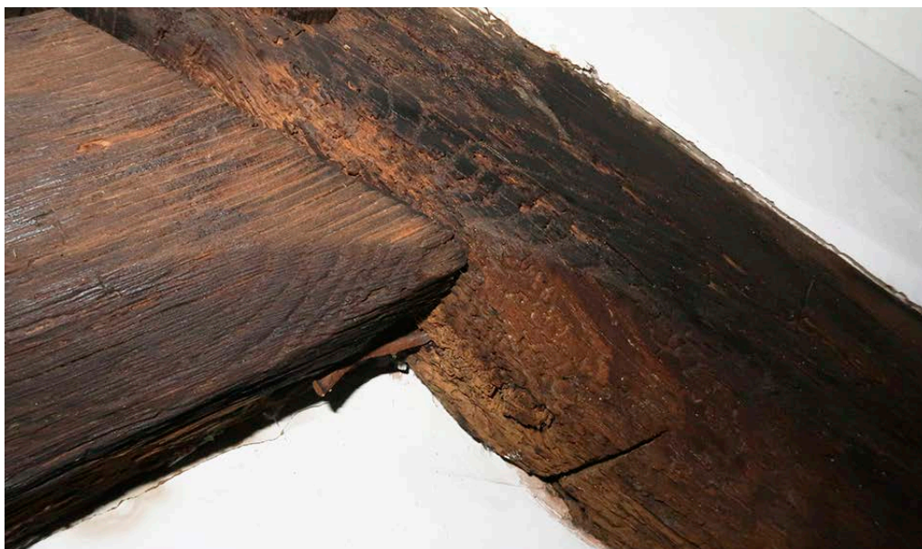
Figure 61: Detail of the north side of frame 5, showing the run-out stops of the upper collar (left) and the cruck blade (right). [Johanna Roethe © Historic England]
