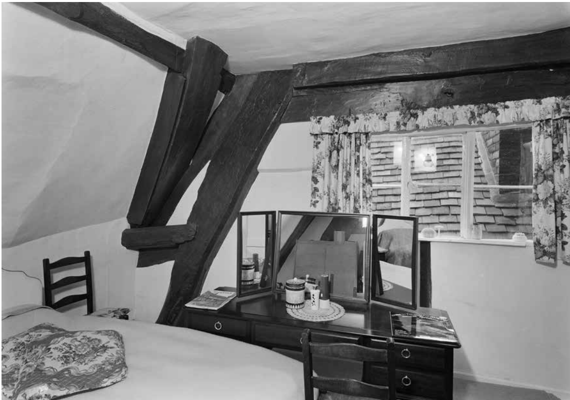
Figure 65: A 1971 photograph showing the north side of the east blade of frame 5 and the lower collar over the window. [© Crown Copyright. Historic England Archive, bb72/00626]
