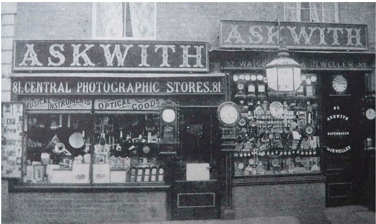
Figure 7: Detail from an advertisement of 1903 showing the shopfronts of 81 (left) and 82 Barton Street. [Gloucestershire Archives, GAL/D5/30357GS]
