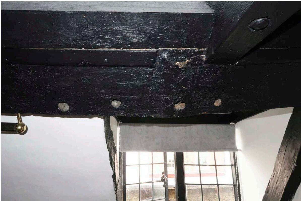
Figure 81: Purlin with peg holes for the former windbraces, north side of west bay in the attic of the front range. [Johanna Roethe]
