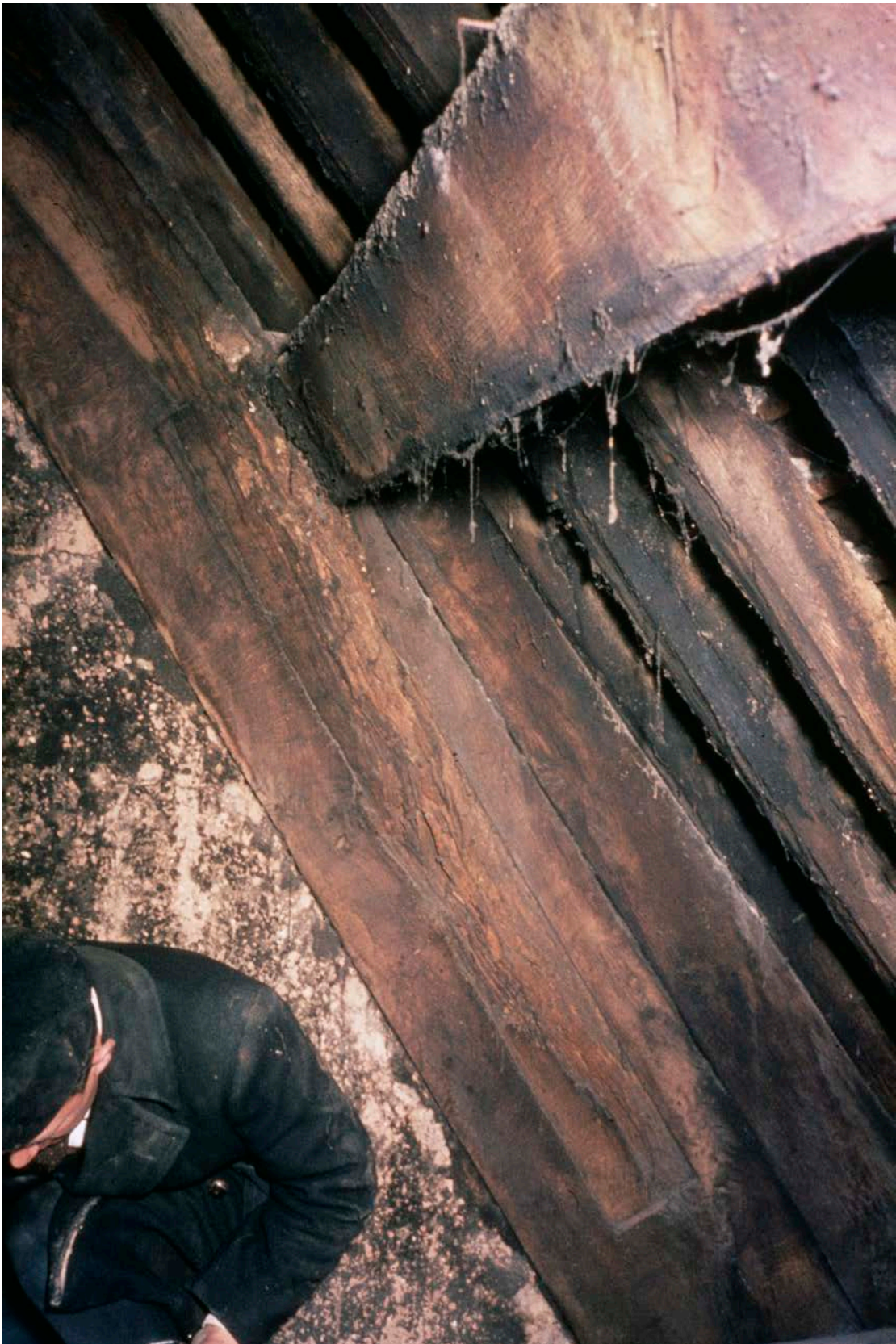
Figure Appendix 1.5: Detail of the east blade of frame 1 in the roof space, with a long, shallow cut out. [© Historic England Archive, SJC01/03/0004]
