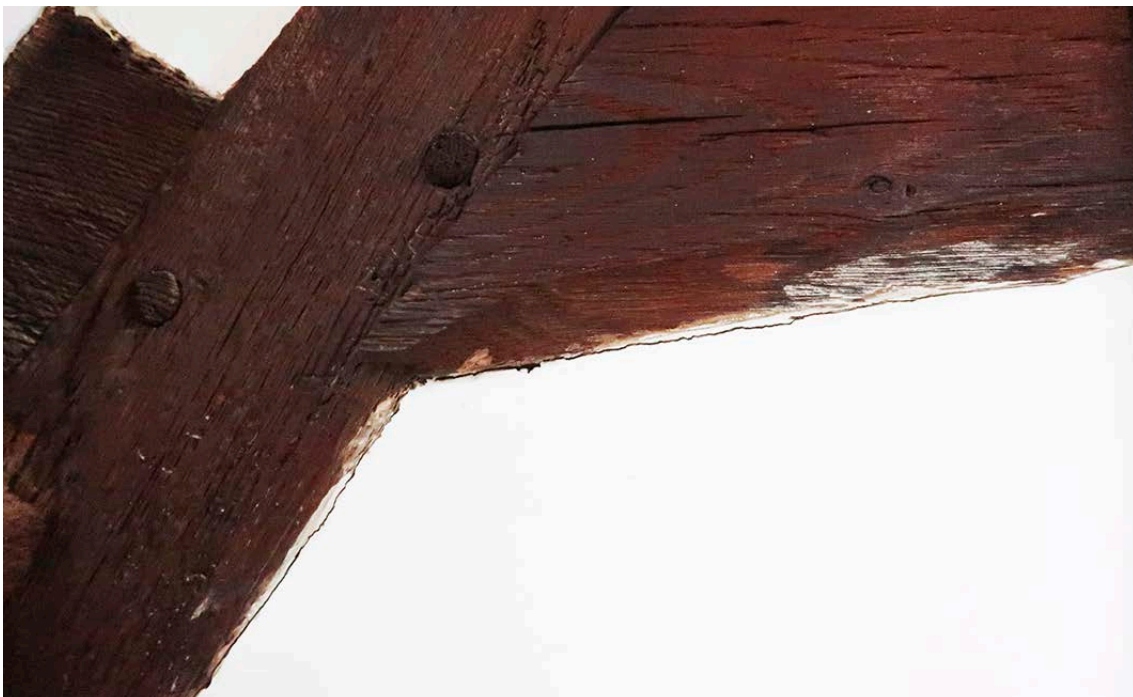
Figure 58: Detail of the collar's run-out stop at the east end of the north side of frame 4. [Johanna Roethe © Historic England]
