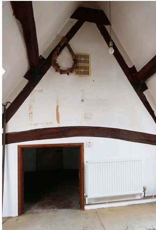
Figure 57: The upper part of the north side of frame 4, at what is now second-floor level. [Johanna Roethe © Historic England]
