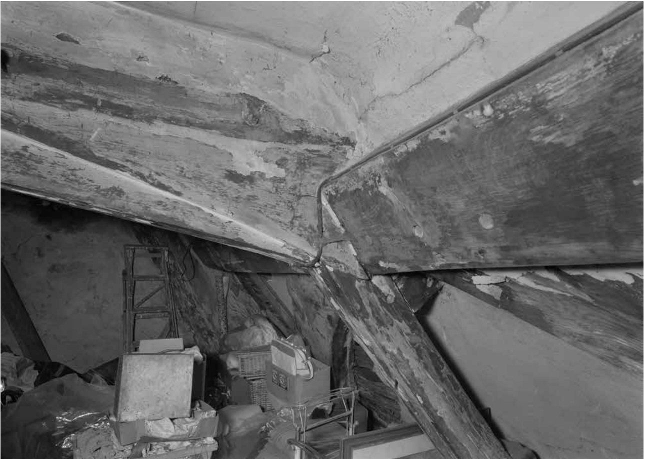
Figure Appendix 3.18: Detail of the birdsmouth joint of the collar and central purlin of frame 2. [© Crown Copyright. Historic England Archive, bb72/00631]
