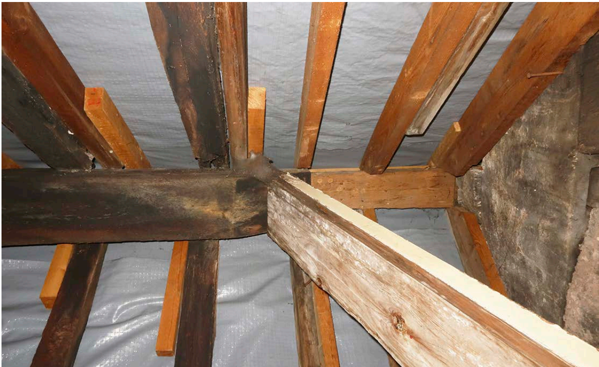
Figure 54: The splayed scarf in the ridge piece, just north of frame 3 (to the right). Part of the ridge piece was removed in the late 20th century and the remaining length propped up. [Johanna Roethe © Historic England]
