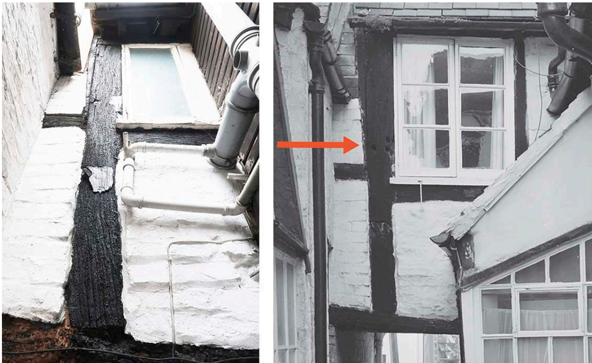
Figure 76: The south-west post, above the passageway [Johanna Roethe © Historic England] and a detail of a photograph of 1971 with an arrow pointing out the empty peg holes in the post. [© Crown Copyright. Historic England Archive, BB72/00611].
