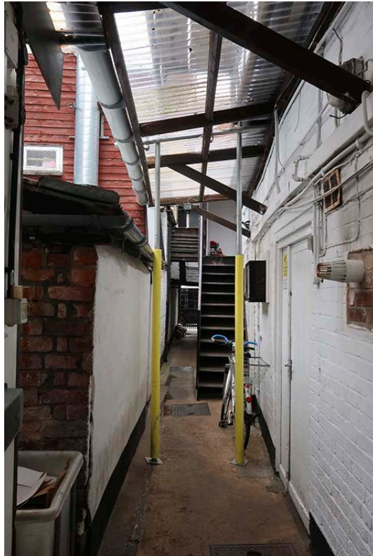
Figure 93: The alleyway, looking north towards the metal staircase installed in the 1970s-80s. The main range is to the right. [Johanna Roethe © Historic England]
