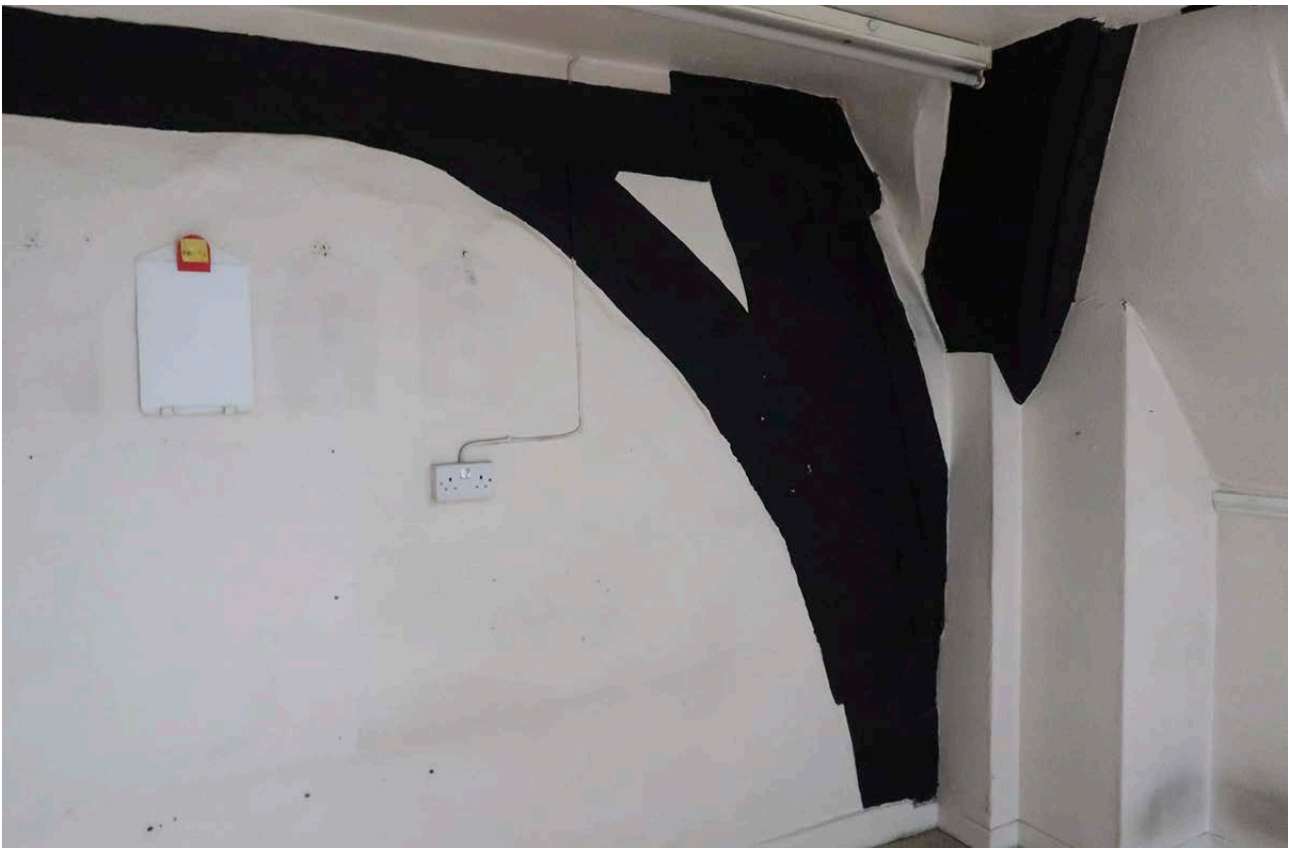
Figure 32: The south side of the east blade of frame 1 at the present first-floor level, showing from left to right the lower collar, arch brace, east cruck blade and windbrace. [Johanna Roethe © Historic England]
