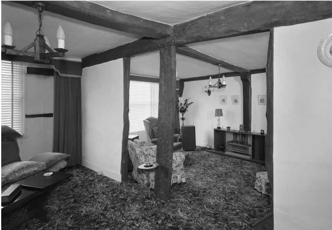
Figure 79: The first floor of the front range photographed in December 1971, looking north-east. The west bay is to the left, the east bay to the right. [© Crown Copyright. Historic England Archive, bb72/00617]
