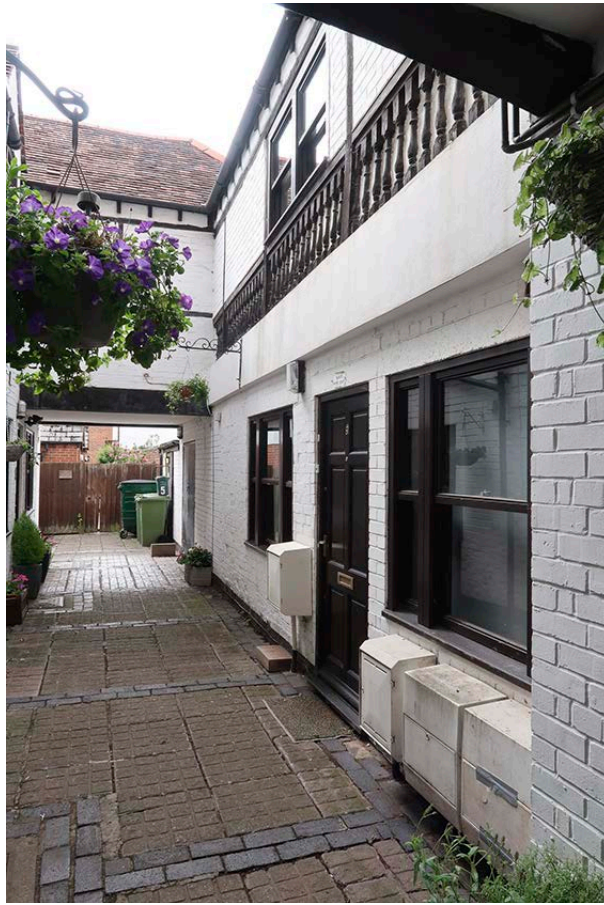
Figure 87: The south (left) and west (right) ranges of the former inn's courtyard. [Johanna Roethe © Historic England]
