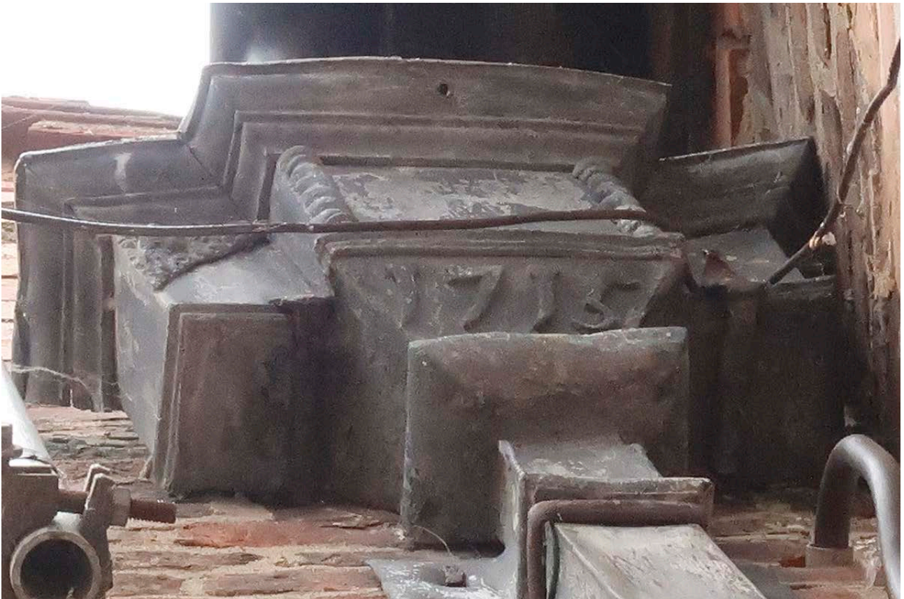
Figure 86: The lead hopper with the date '1715' at the rear of the front range of 78-80 Barton Street. [Johanna Roethe © Historic England]
