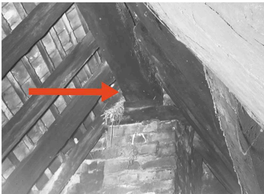
Figure 55: Detail of a photograph taken by Dennis Evans in December 1971, showing the chimneystack just north of frame 3. The arrow indicates the then still intact splayed scarf of the ridge piece. [© Crown Copyright. Historic England Archive, BB72/00632]
