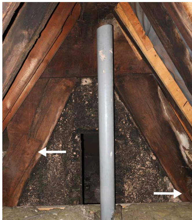
Figure 42: The south side of the apex of frame 1 with white arrows indicating the visible patch infills in the cruck blades. [Rebecca Lane © Historic England]
