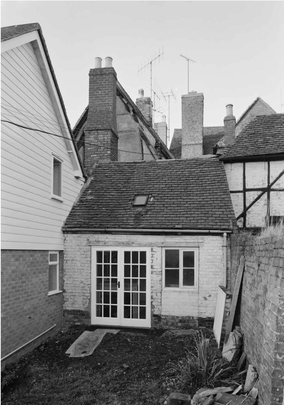
Figure Appendix 3.5: Looking north from the south end of the plot towards the south gable (left of centre) of the main range. In the foreground are a 1970s range (left) and a single-storey 19th-century range (centre). [© Crown Copyright. Historic England Archive, bb72/00613]
