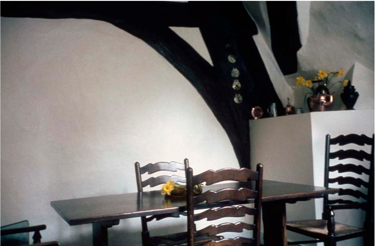
Figure Appendix 1.3: The south side of the east blade of frame 1, at collar level (now first-floor level). [© Historic England Archive, SJC01/03/0001]
