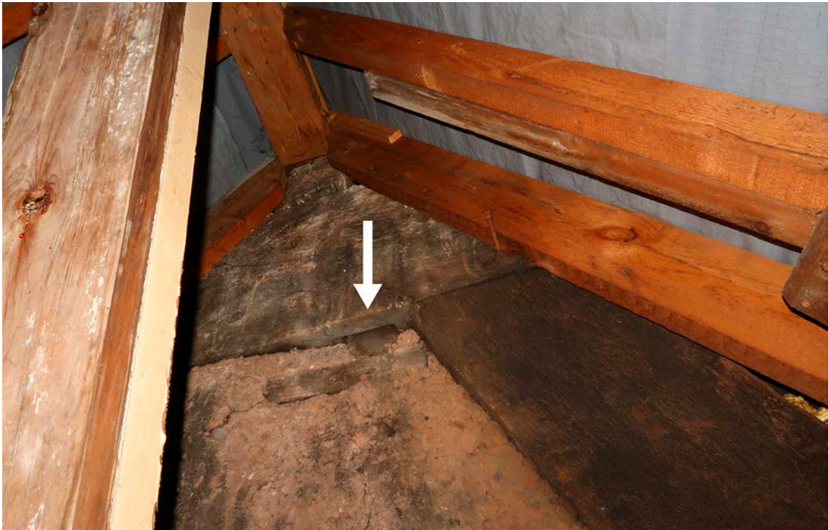
Figure 51: The north side of the apex of frame 3 with an arrow indicating a mortise with stave. [Johanna Roethe © Historic England]
