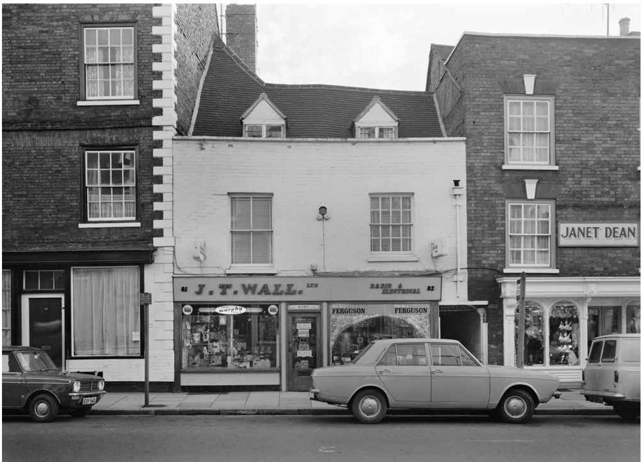
Figure Appendix 3.2: The north elevation of 81-2 Barton Street. [© Crown Copyright. Historic England Archive, bb72/00610]
