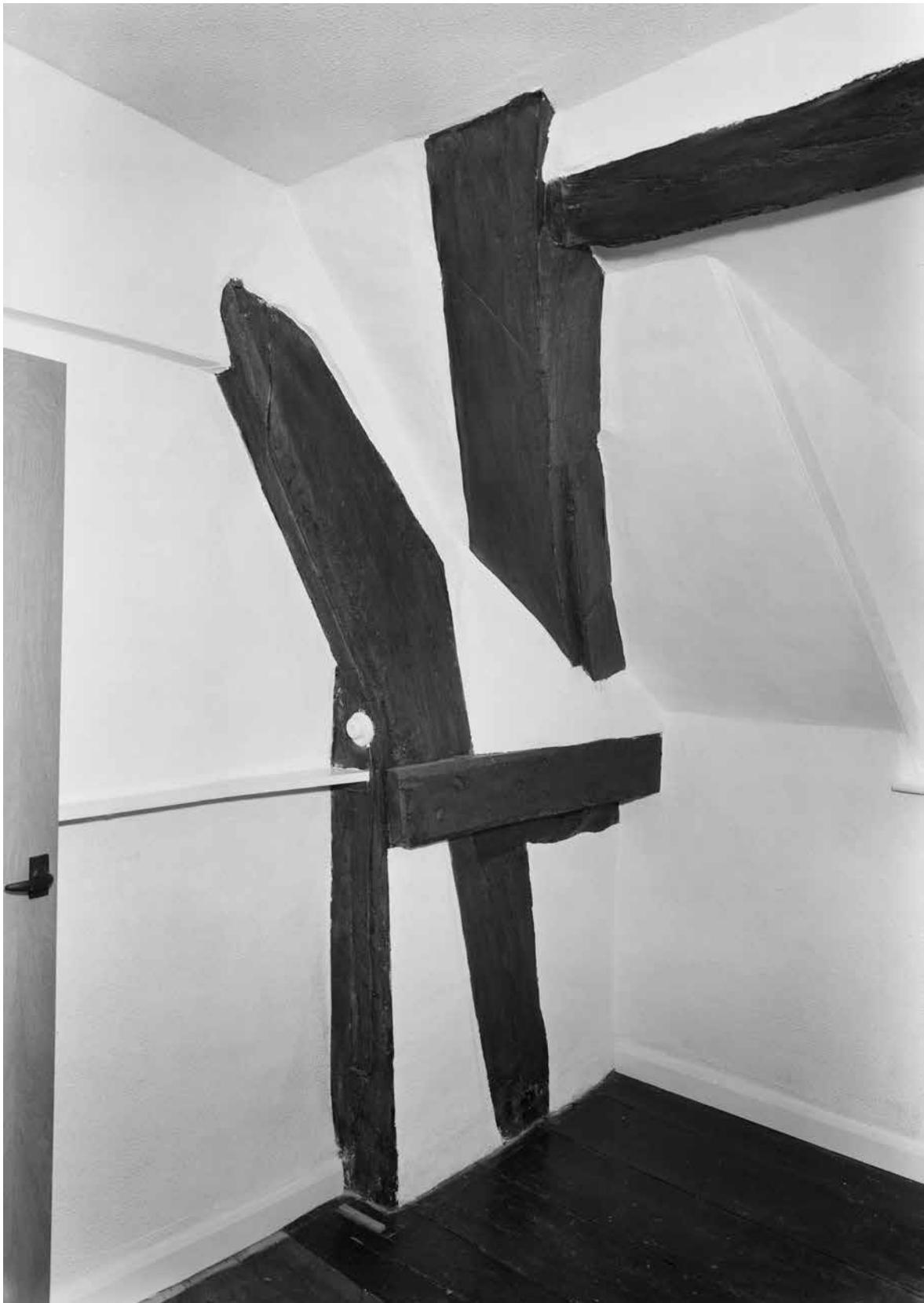
Figure Appendix 3.24: The north side of the west blade of the main range's frame 5, at second-floor level. [© Crown Copyright. Historic England Archive, bb72/00625]
