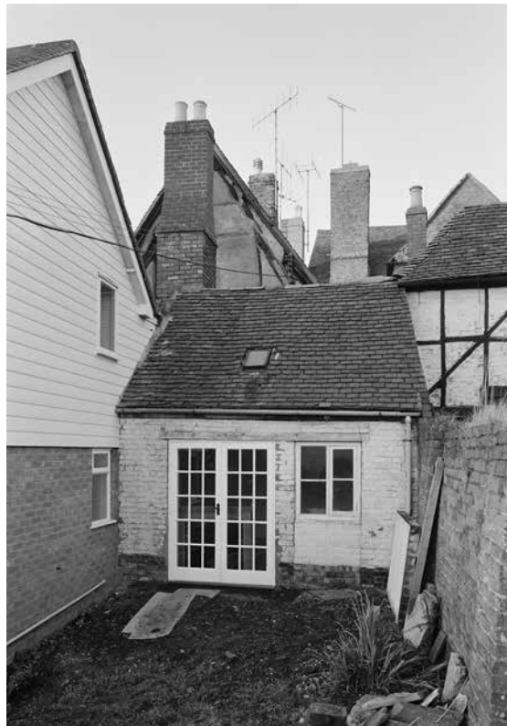
Figure 18: The single-storey range to the rear of the main range and the newly rebuilt south-west range (left) in a photograph by Dennis Evans of December 1971. [© Crown Copyright. Historic England Archive, BB72/00613]
