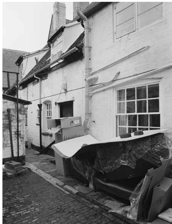
Figure 20: The west elevation of the main range (left) and the rear range (right) in a photograph by Dennis Evans of December 1971. [© Crown Copyright. Historic England Archive, BB72/00612]
