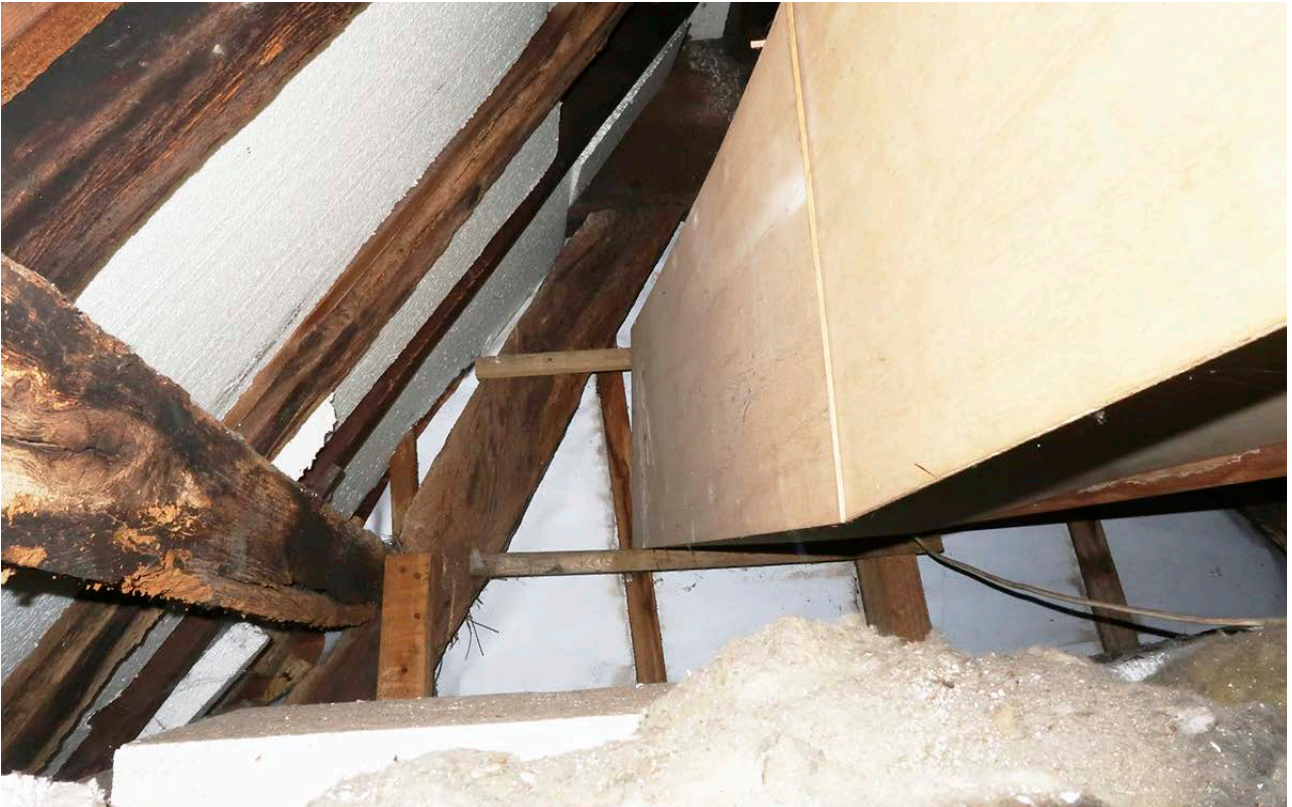
Figure 64: The upper part of the north side of frame 5 with the saddle (top centre) and the upper purlin (left) trenched onto the eastern cruck blade. [Johanna Roethe © Historic England]
