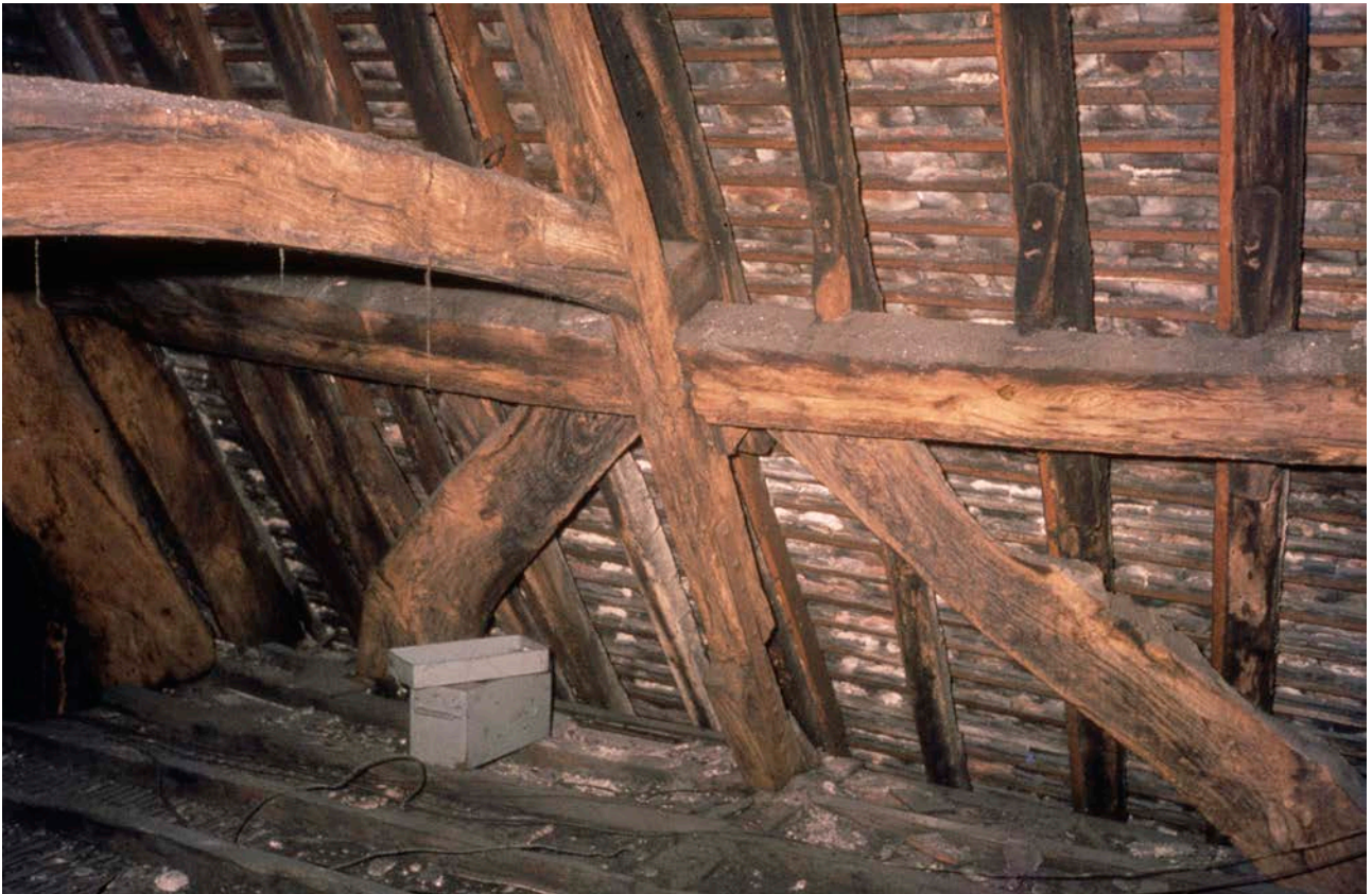
Figure Appendix 1.9: The collar of frame 4 (top left) and the eastern central purlin and windbraces in bays C and D. [© Historic England Archive, SJC01/03/0003]
