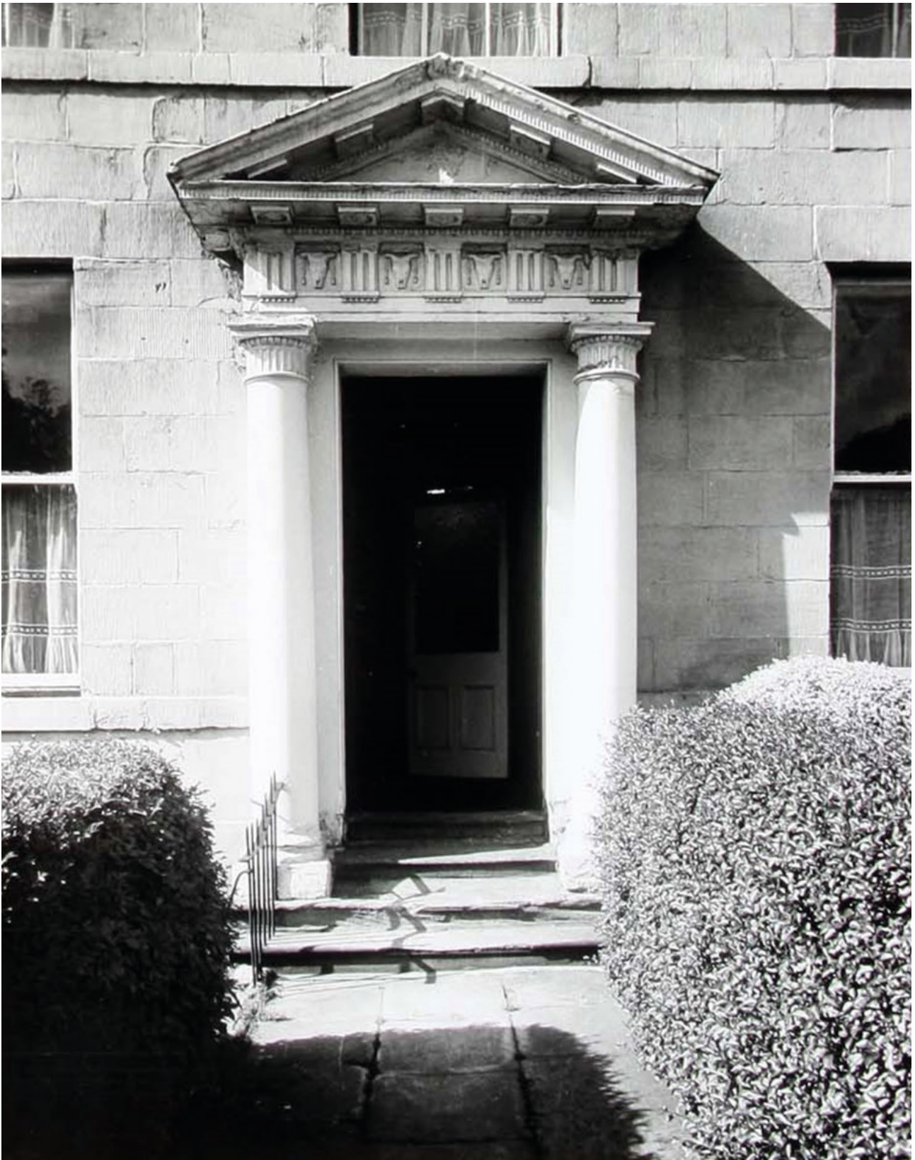
Figure 22: The Doric doorcase of No. 18, photographed in 1969, with its frieze of triglyphs and bucrania. [AA68/1960 © Historic England Archive]
