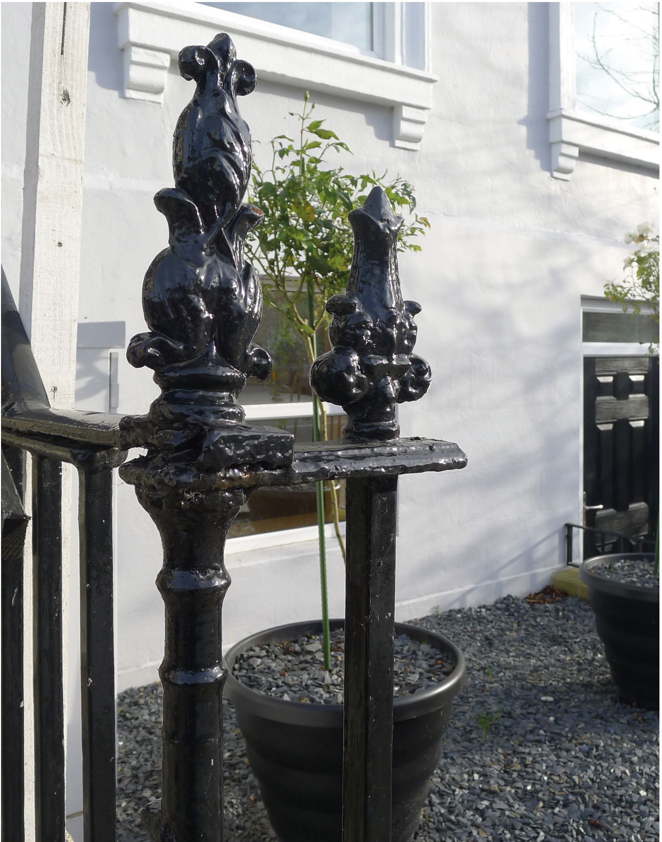
Figure 26: The cast-iron foliate finials of railings outside No. 29. [Lucy Jessop © Historic England]
