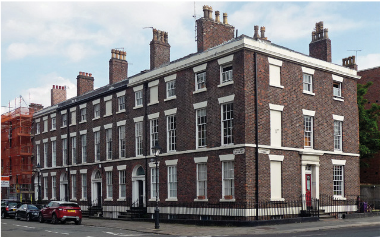
Figure 31: A view of the corner of Falkner Street and Catharine Street, Liverpool, showing their simple cast-iron railings with spear head finials. [© Stephen Richards and licensed for reuse under Creative Commons licence CC BY-SA 2.0 DEED]
