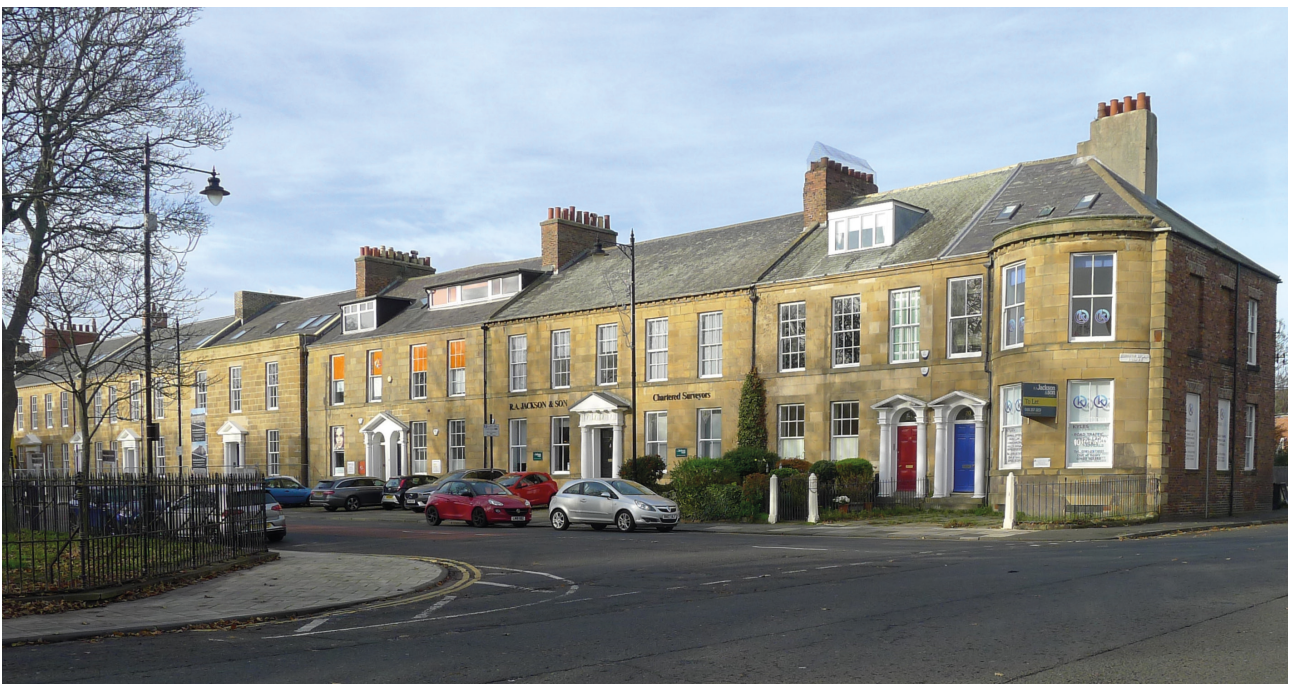
Figure 21: The ashlar-fronted houses on the north side of Northumberland Square. [Lucy Jessop © Historic England]
