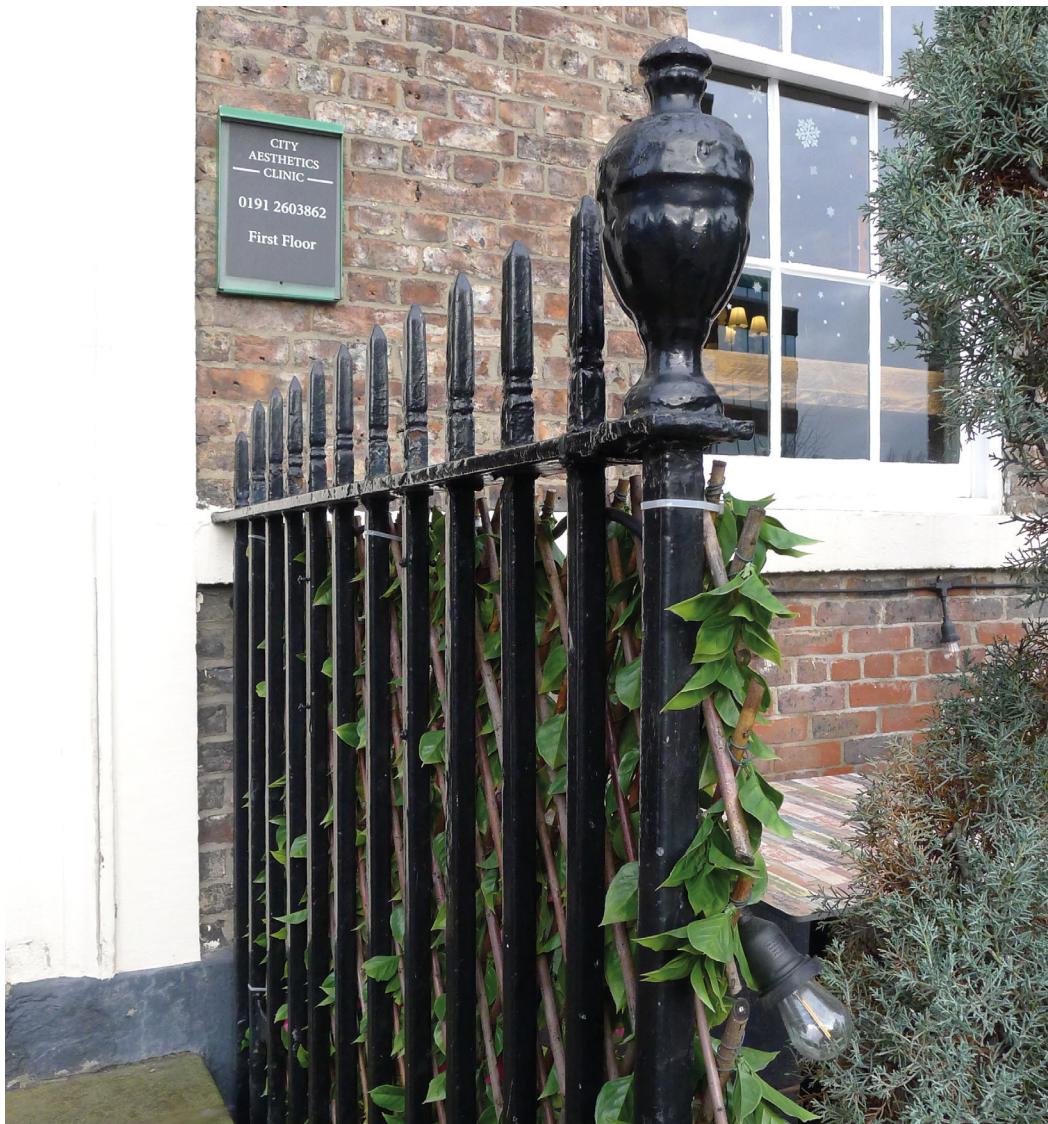
Figure 30: Cast iron railings with simple spear heads and an urn finial for the terminal post outside 5, Savile Place, Newcastle upon Tyne. [Lucy Jessop © Historic England]
