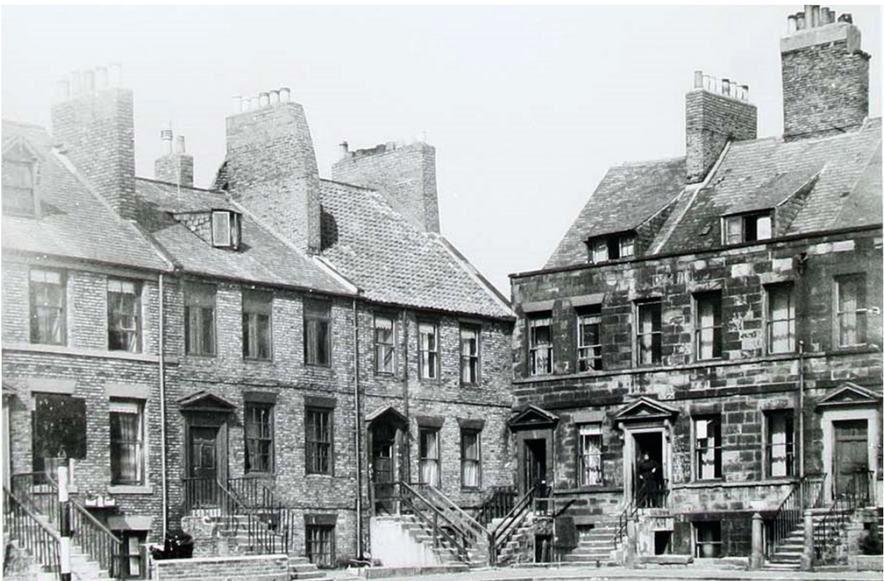
Figure 4: The north-west corner of Dockwray Square, photographed in May 1949. [NBR AR49/7207 © Historic England Archive]
