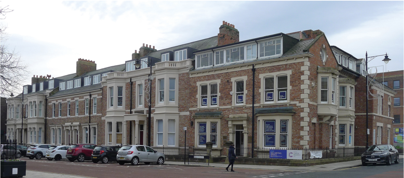
Figure 29: The buildings on the west side of Northumberland Square. The former North Shields Club is on the far left of the photograph. [Lucy Jessop © Historic England]
