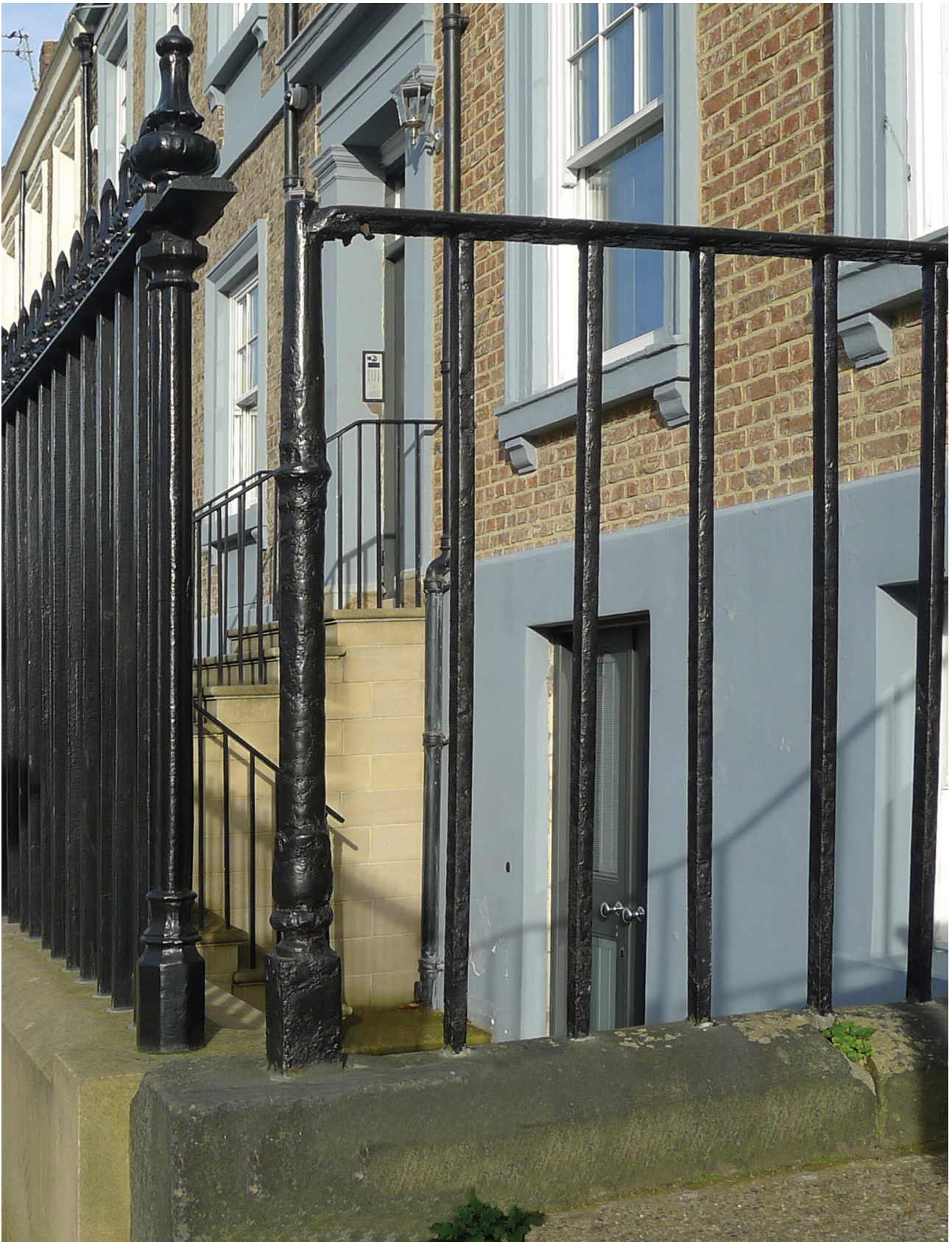
Figure 27: Simple cast-iron railings outside No. 24. [Lucy Jessop © Historic England]
