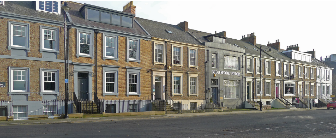
Figure 28: The houses on the east side of Northumberland Square. [Lucy Jessop © Historic England]
