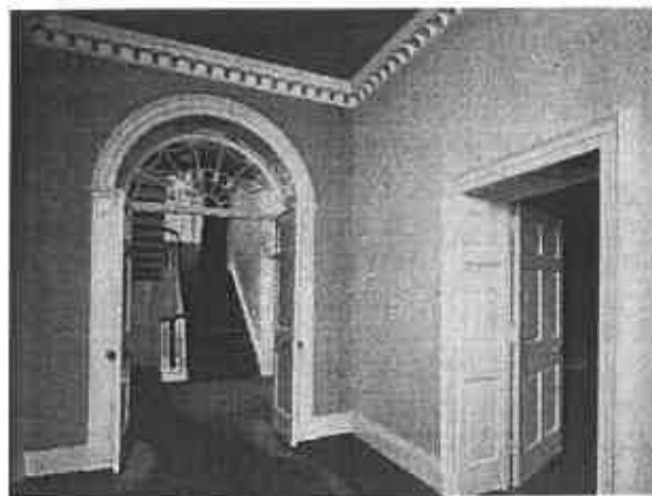
Fig.6 Entrance hall looking through to the main stair hall. (NMR: BB007285)
