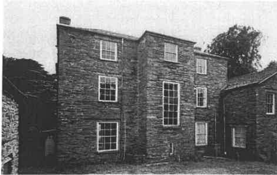
Fig.5 Rear of main block. (NMR: BB007277)
