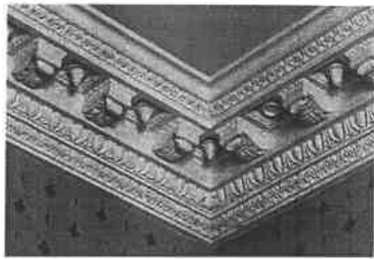
Fig.10 Cornice in west front room on ground floor. (NMR: AA006266)
