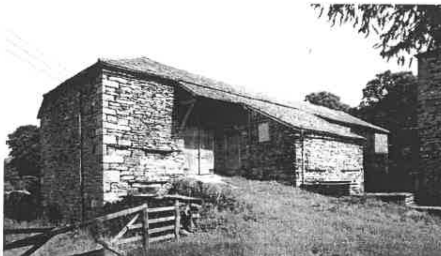
Fig.17 West elevation of east wing showing ramp to first-floor threshing barn. (NMR: BB007282)
