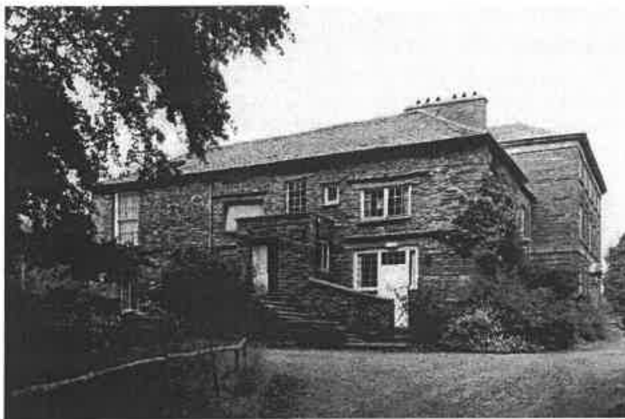
Fig.15 West side elevation of the west wing. (NMR: BB007275)
