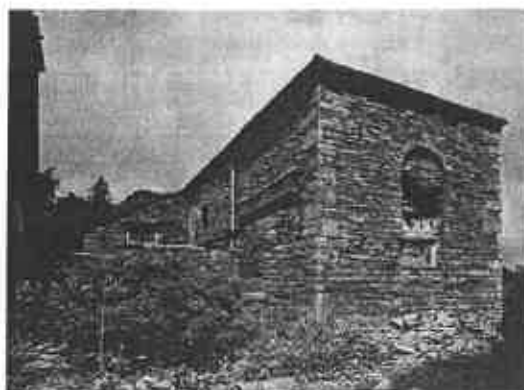
Fig.16 Front elevation of the east wing. (NMR: BB007280)
