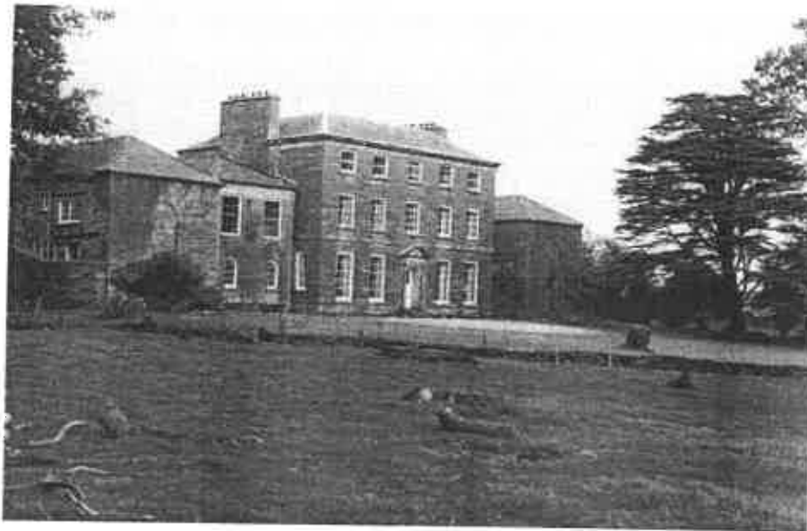
Fig.4 Front elevation of Belmount. (National Trust)
