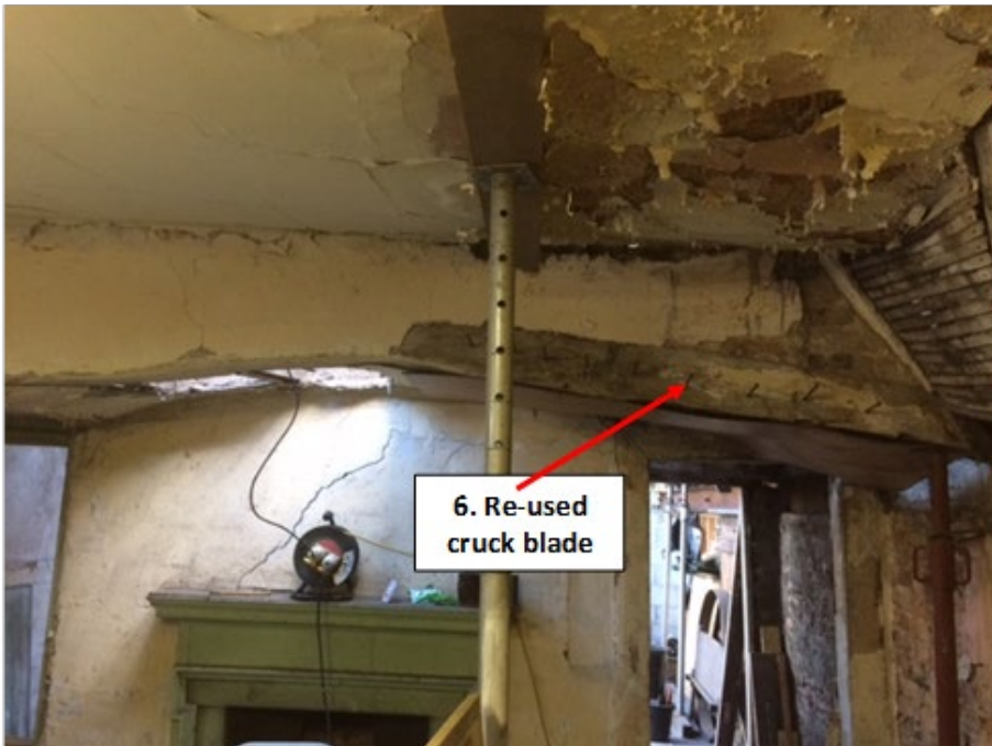
Figure 6: Annotated photograph, facing east, to help locate sampled timber 6 (see Table 1) (photograph Robert Howard)
