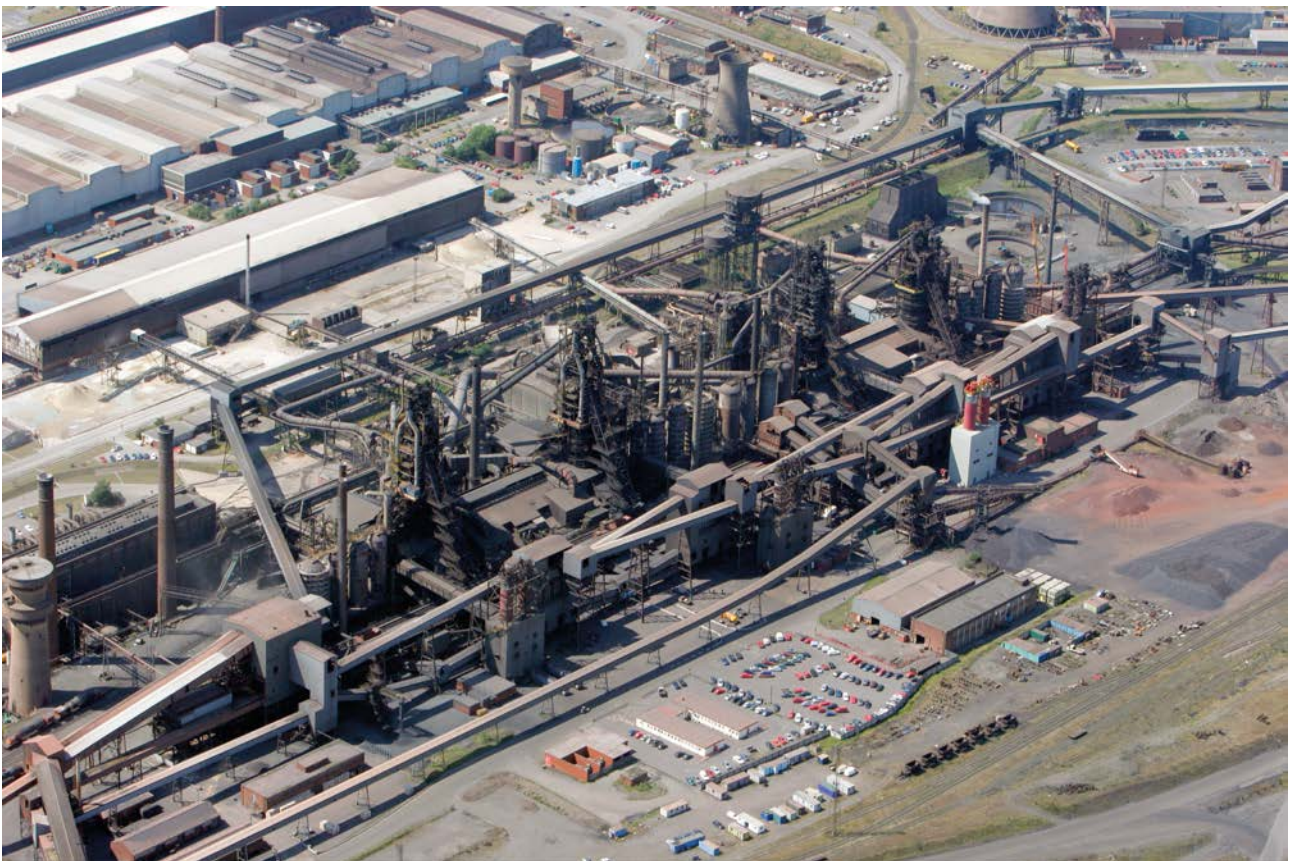
Figure 34: The four blast furnaces at Scunthorpe (NMR 20320_008 28 June 2005 © Historic England Archive).
