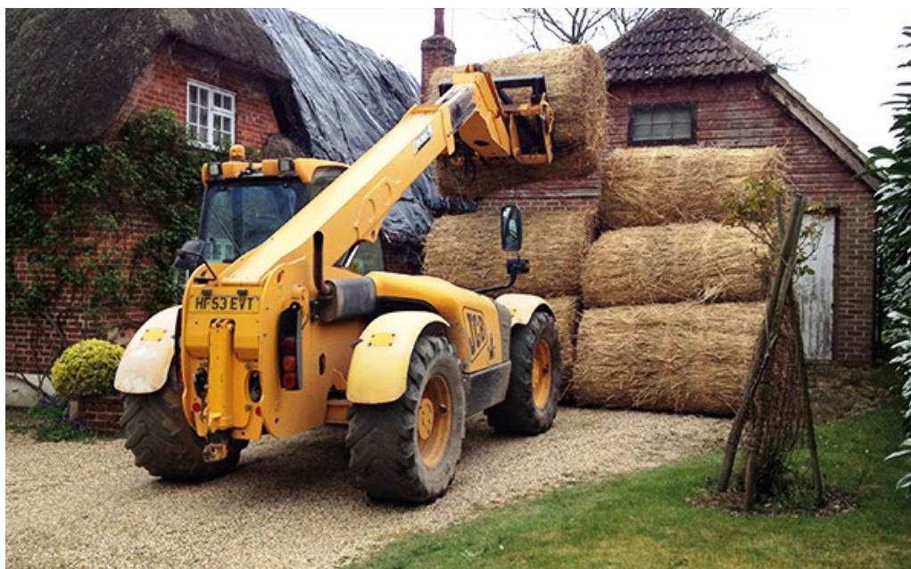
Figure 23: Unloading packs of CWR at a work site.
