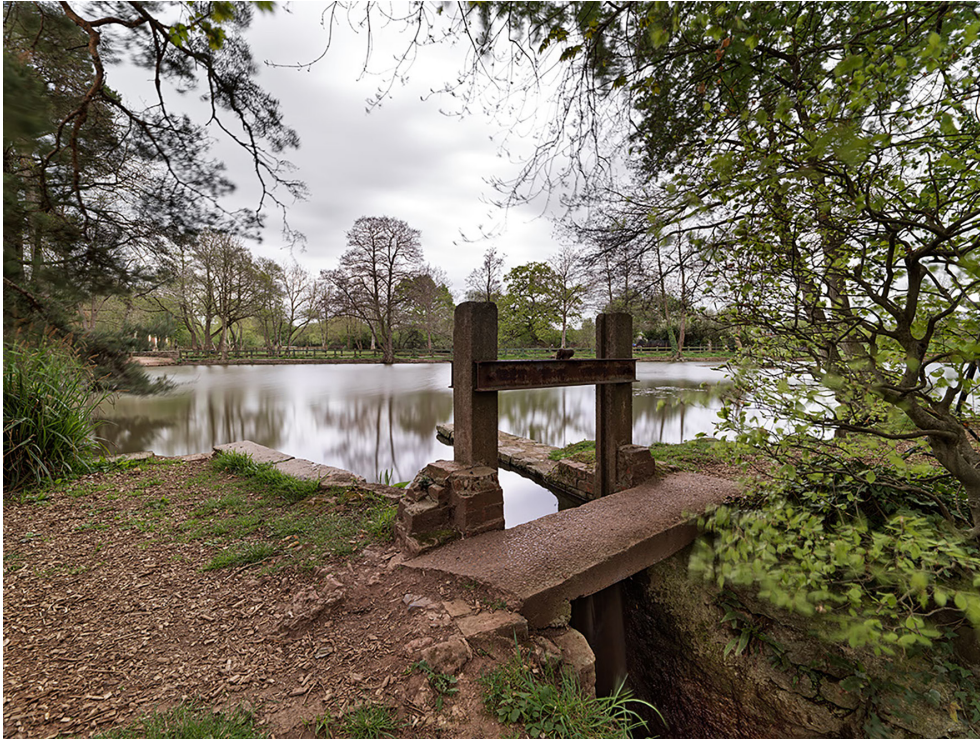
Figure 16: Outflow sluice [36] in the northern water basin, looking south-west, April 2022 [James O. Davies © Historic England Archive, DP347736]
