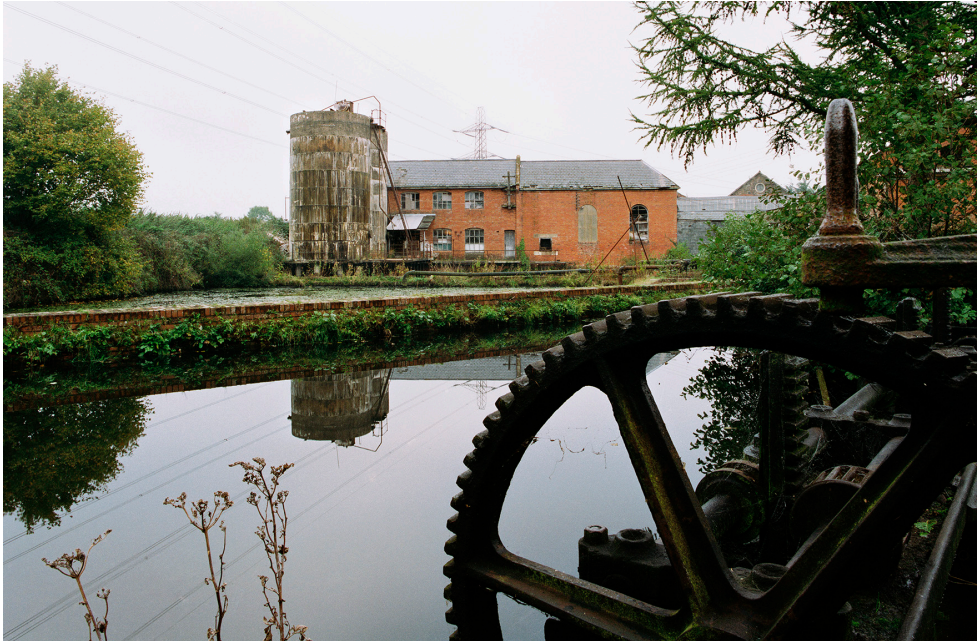
Figure 51: The headrace at Tone Works [73] (foreground), with the soft water reservoir of the early 1890s [71] and the pair of concrete lime soda water softening towers dating from 1914 beyond, looking north-east, October 1995 [Peter Williams © Crown copyright. Historic England, AA96/00645]
