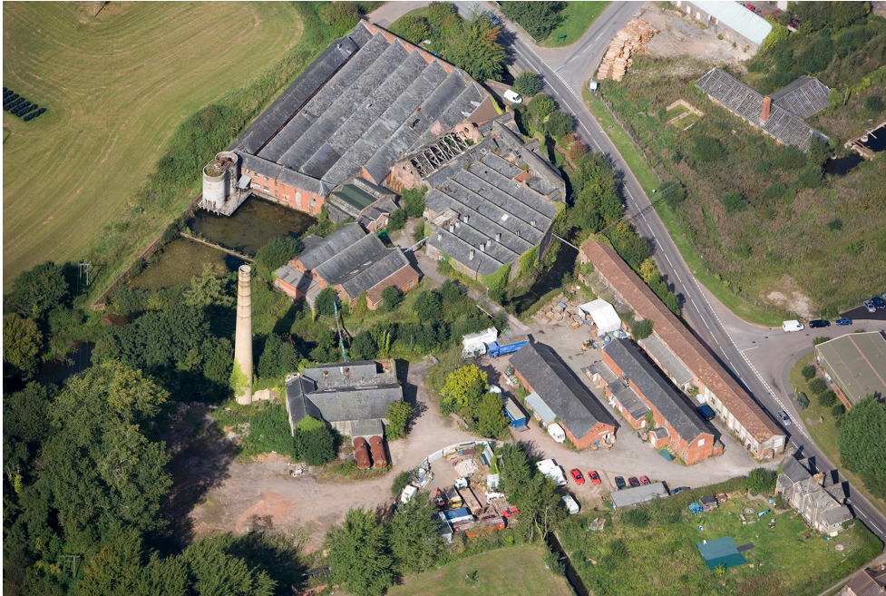
Figure 44: Tone Works in 2007, looking north with the main mill site overgrown and derelict. [HEA 24720_029 18-SEP-2007 © Crown copyright. Historic England Archive]
