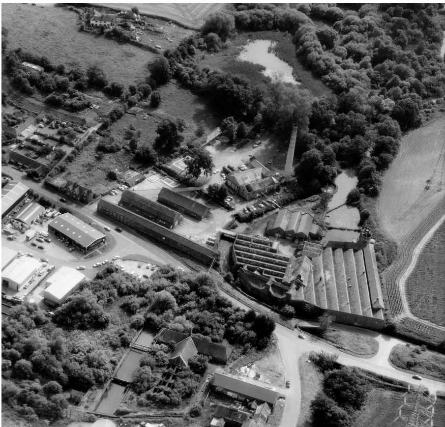
Figure 58: Tone Works in 1993, looking east, with the already overgrown grease works in the foreground. [ST1221/351 22-JUN-1993 © Crown copyright. Historic England Archive]
