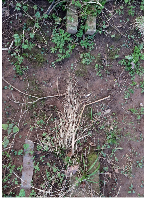
Figure 13: The buried remains of a sluice gate [20] on the Westford Stream at its confluence with the Rockwell Green Stream, January 2022 [Johanna Roethe © Historic England]
