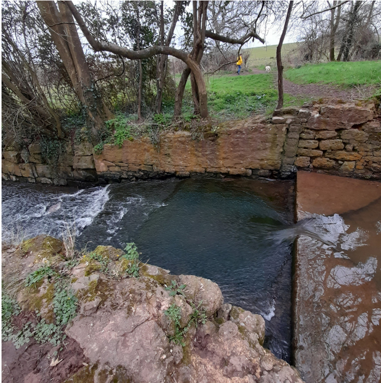
Figure 23: The weir at Oaken Ground [3], looking east, March 2022 [Nicky Smith © Historic England]
