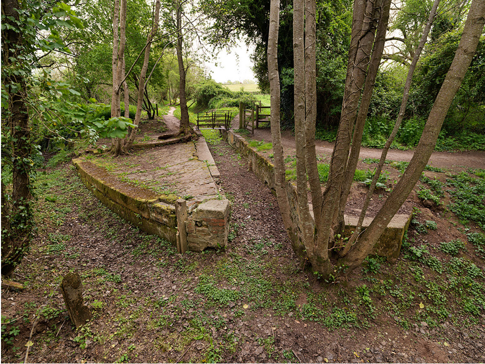
Figure 21: Dry channels [10 (right) and 19 (left)] following the flood alleviation work, looking east, April 2022 [James O. Davies © Historic England Archive, DP347755]
