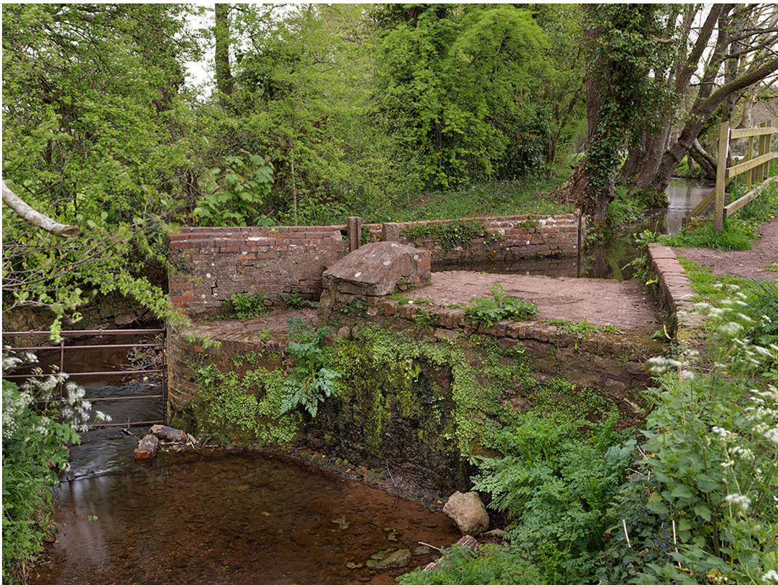
Figure 11: The Waterfall Weir [25], looking east, April 2022 [James O. Davies © Historic England Archive, DP347739]
