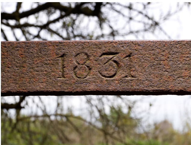
Figure 62: Detail of blacksmith bridge [2] showing the incised date of 1831 on the inner side of the handrail on the north side [James O. Davies © Historic England Archive, DP347760]
