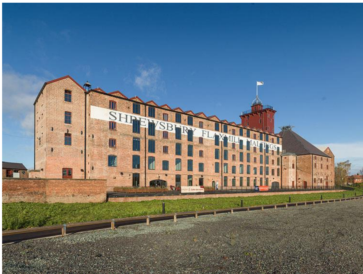
Figure 1. An image of the restored Main Mill and Kiln © Steve Baker, Historic England, November 2022
