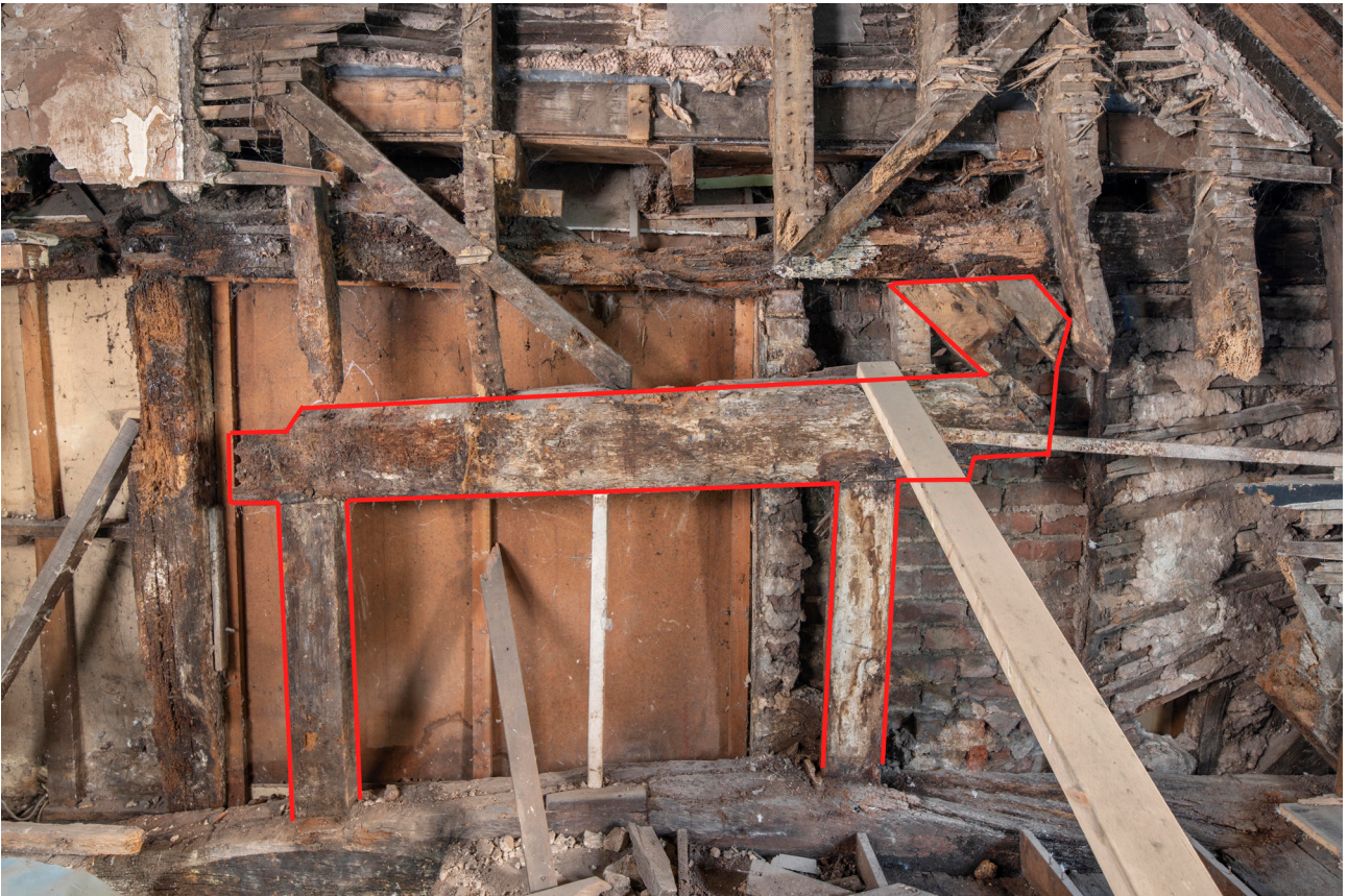
Figure 26: The surviving elements of the roof truss of frame C, with collar, two queen struts and part of the principal rafter outlined in red, looking west. [James O. Davies © HEA DP435502]
