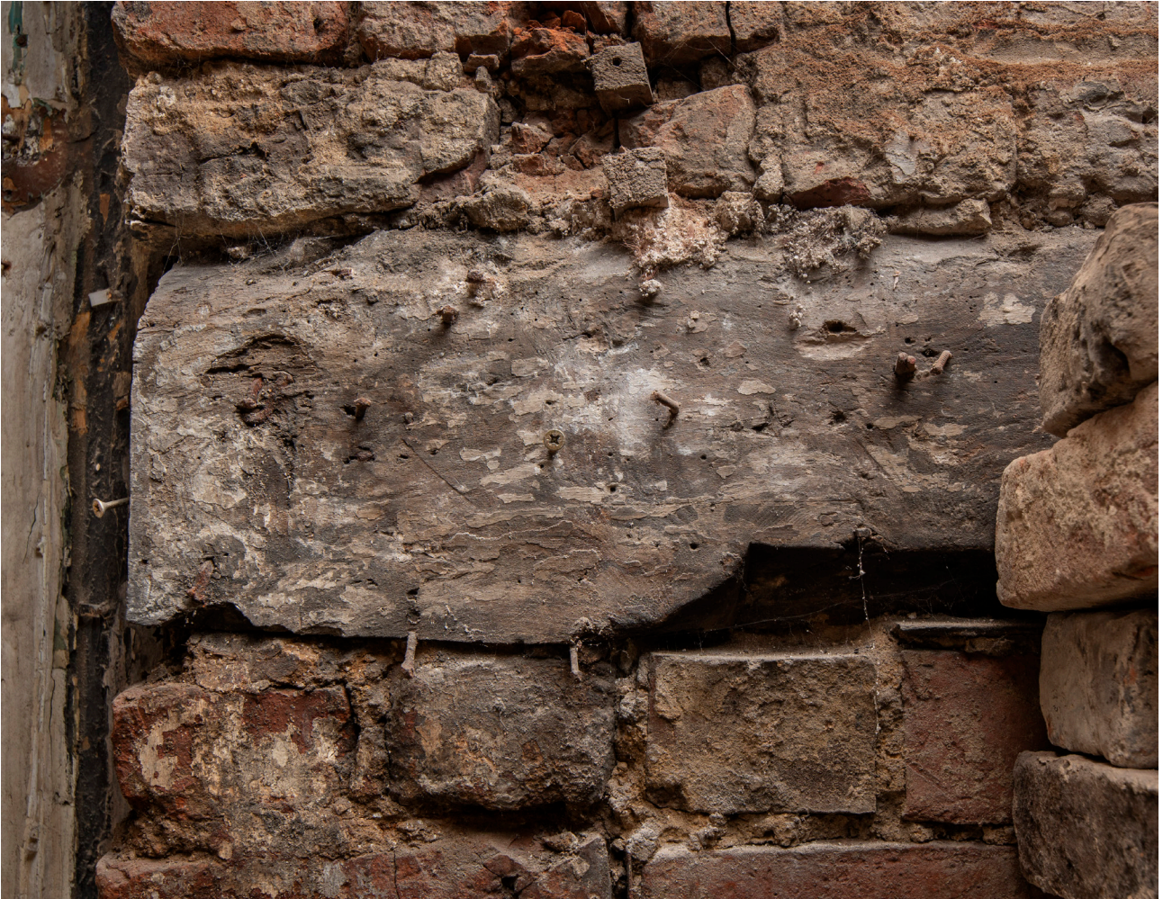
Figure 51: The south end of the cut-down fireplace bressummer, reused in the later fireplace, with an ogee chamfer stop visible at its south end. [James O. Davies © HEA DP435515]
