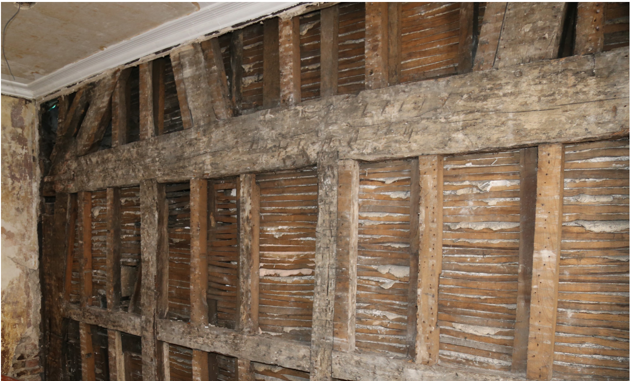
Figure 20: The central frame (frame B) at first-floor level with later timber-framed infill, looking south-west. [© Andrea Kirkham. Reproduced with permission]
