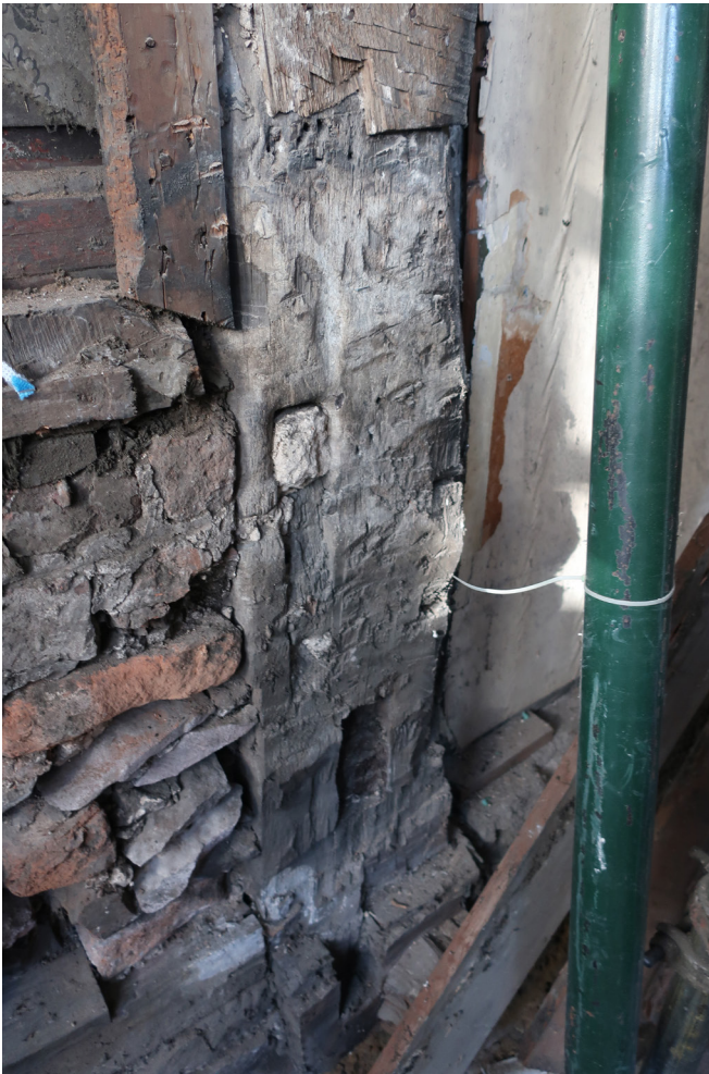
Figure 19: The north post of the central frame (frame B), surviving at ground-floor level in the partition between Nos 39 and 41, looking east. [Rebecca Lane © Historic England]
