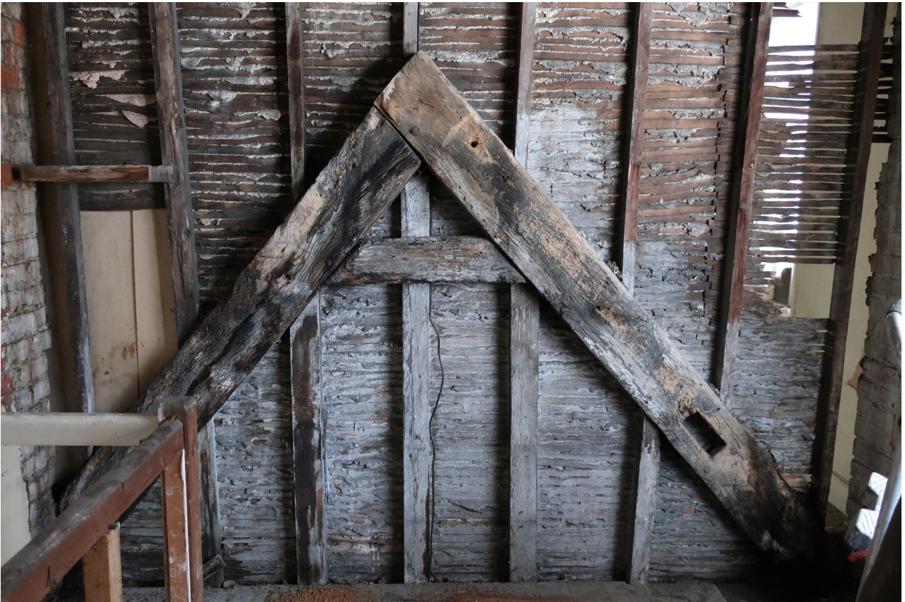
Figure 39: The upper part of the roof truss of the southern frame of the rear range of No. 39, looking north. [Rebecca Lane © Historic England]
