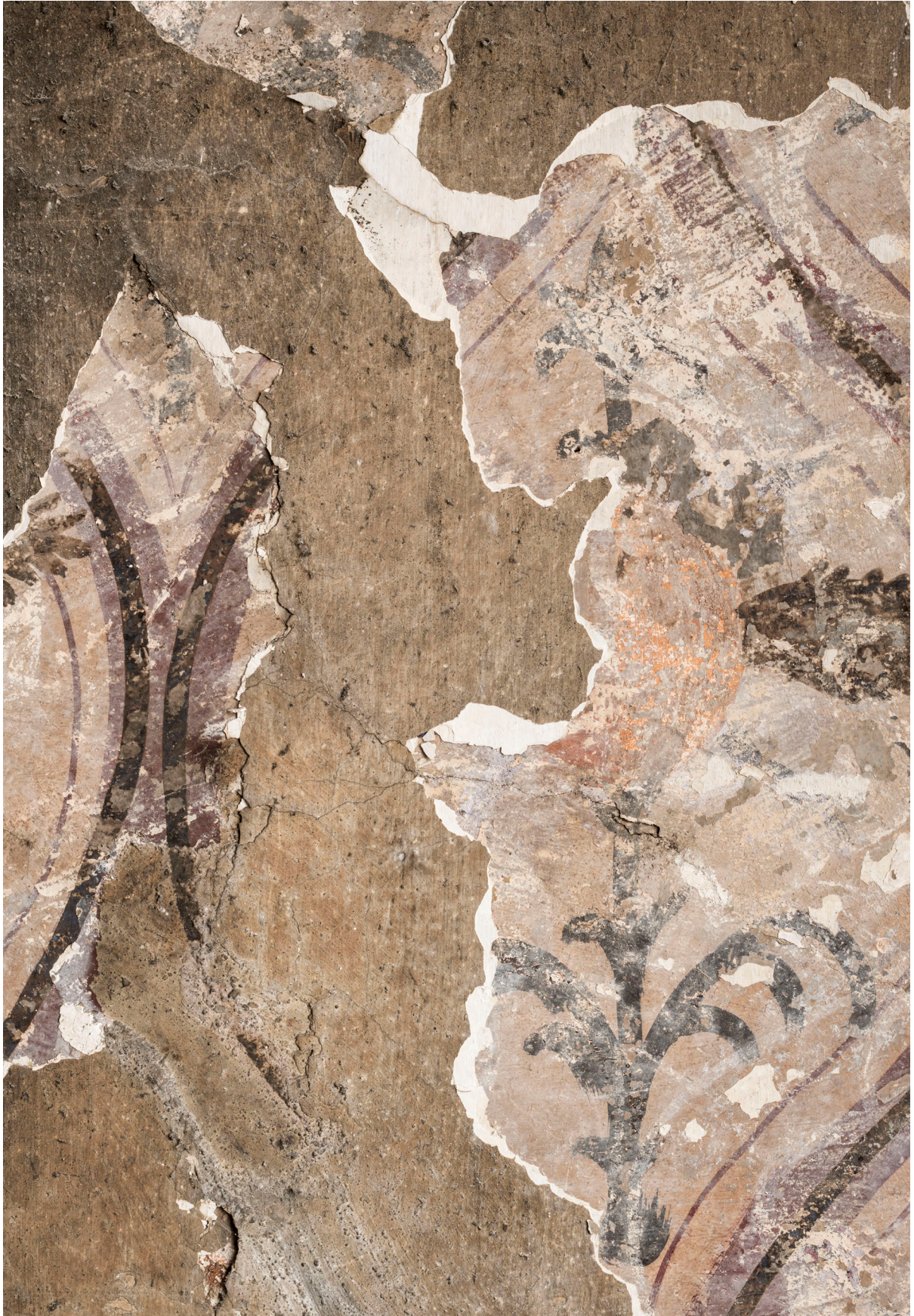
Figure 44: Detail of the scheme of late 16th century wall painting on the east elevation of the rear range of No. 39, showing the red lattice work with floral motif within. [Steve Baker © HEA DP464269]
