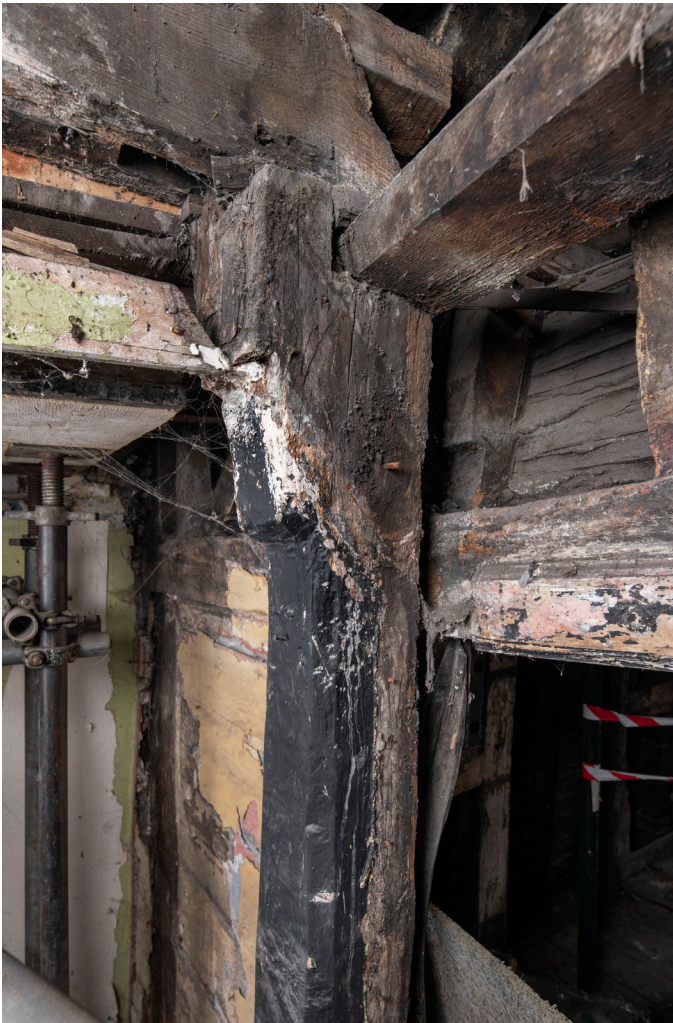
Figure 47: North post of the west elevation of the rear range of No. 41 (Frame G) showing the form of the jowl, which is typical of the 17th century, looking north-west. [James O. Davies © HEA DP435486]
