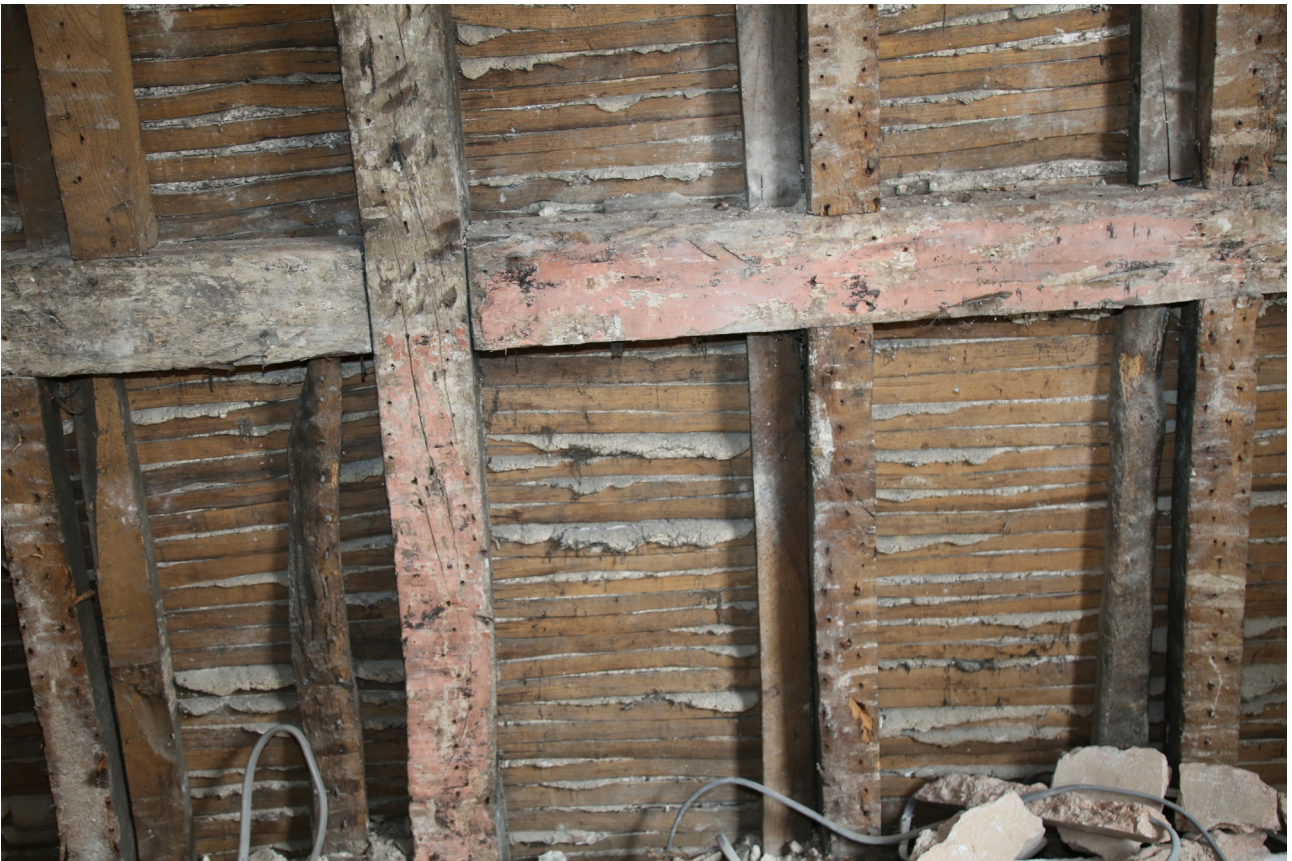
Figure 53: Detail of the later framework inserted into the central frame of the front range (frame B), showing pink paint on the timbers, looking west. [© Andrea Kirkham. Reproduced with permission]
