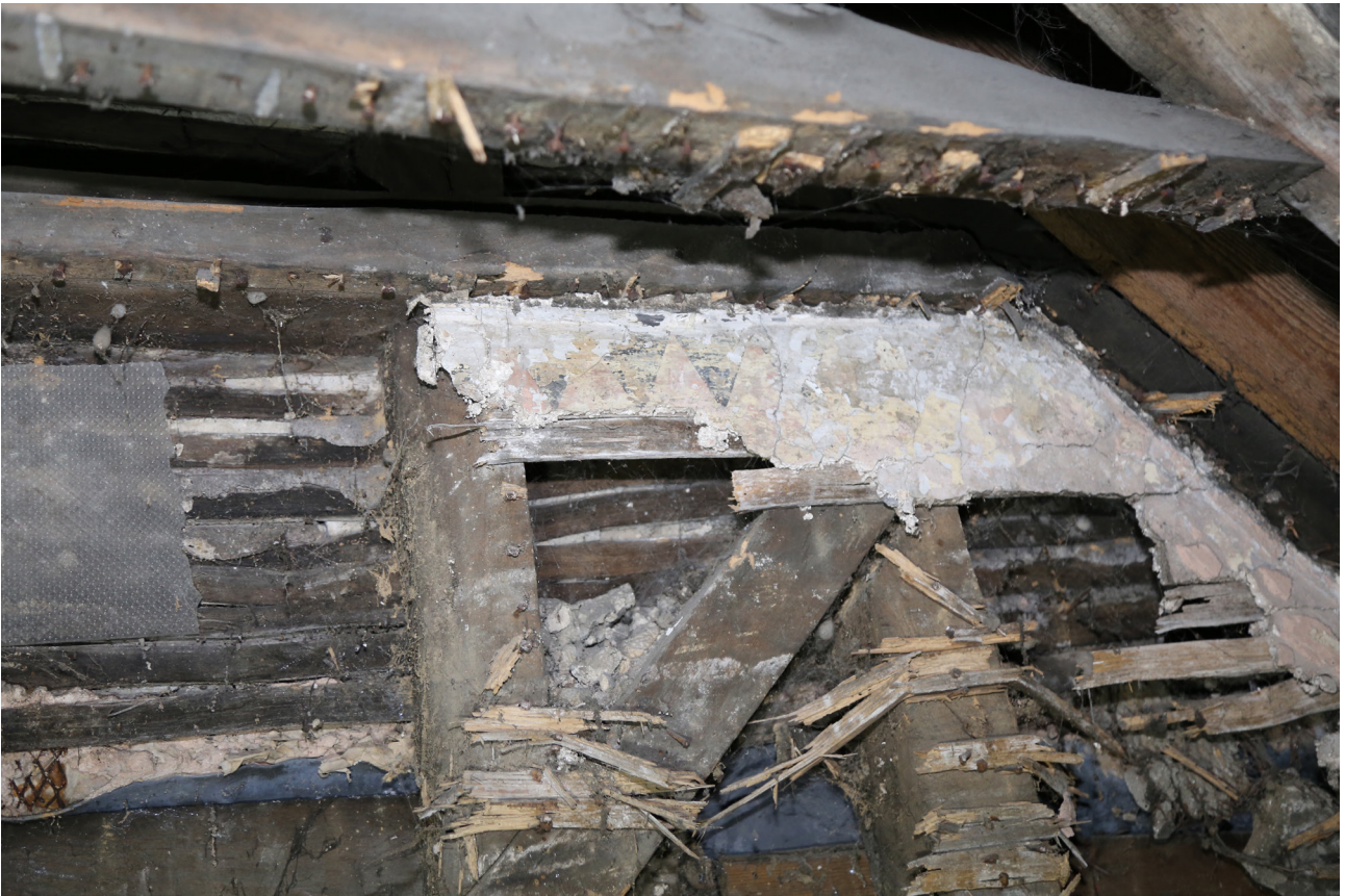
Figure 57: Fragment of wall plaster left in attic room over west bay of the front range (No. 41), showing a painted motif of triangles along the top edge of the plaster, immediately under the ceiling level, looking north-west. [© Andrea Kirkham. Reproduced with permission]
