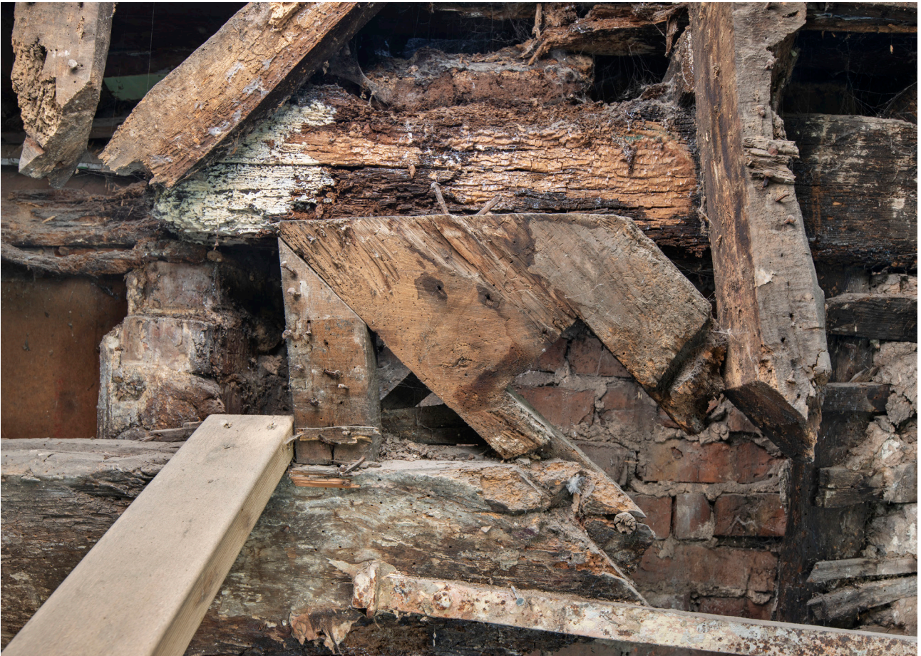
Figure 27: The small section of the surviving north principal rafter where it meets the surviving collar, with a redundant mortice for the purlin, looking west. [James O. Davies © HEA DP435503]
