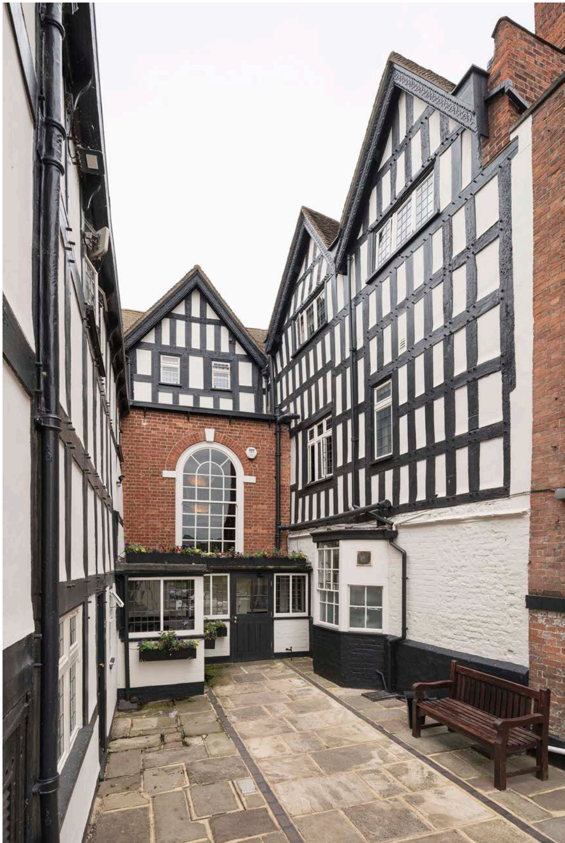
Figure 42: The courtyard to the rear (west) of the front range, with the north elevation of the south wing to the right. [Steven Baker © Historic England Archive, DP325764]
