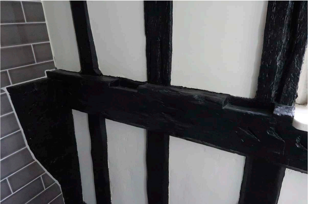
Figure 39: The former wall plate and jowled west post of the north elevation at the modern second-floor level. [Johanna Roethe © Historic England]
