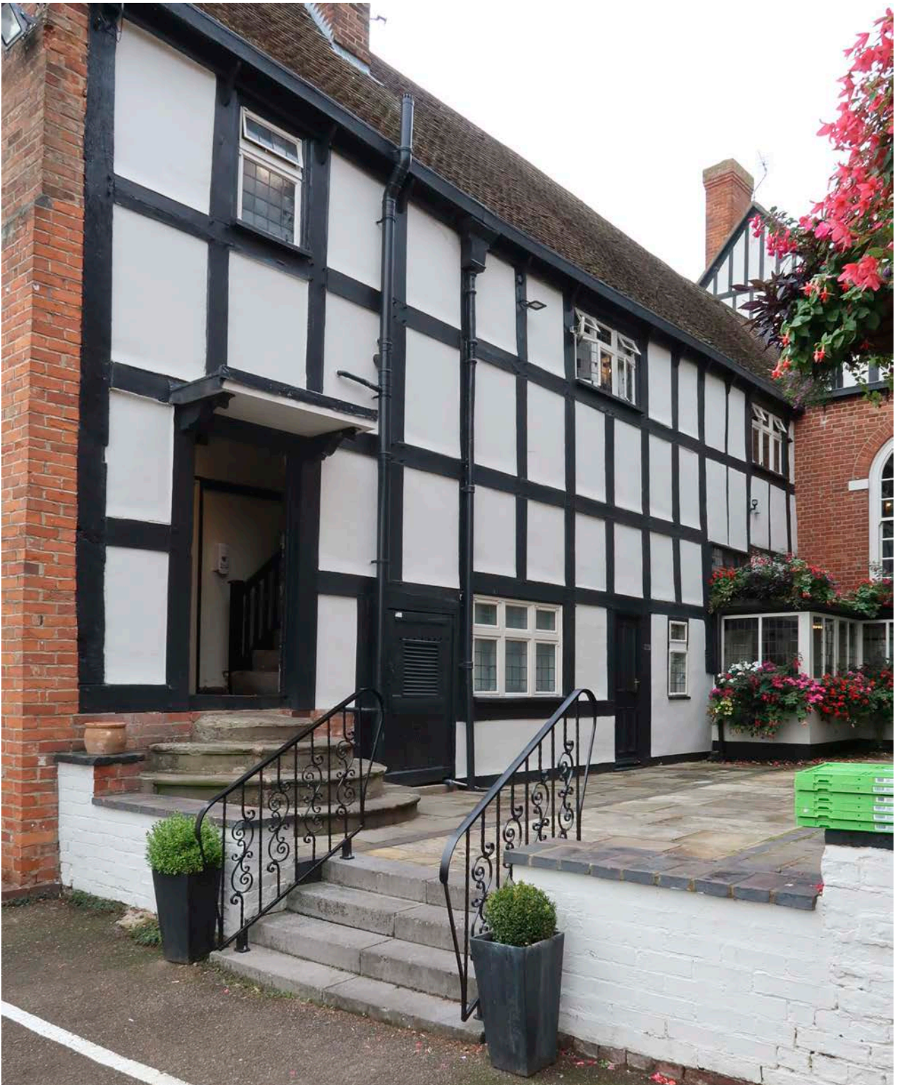
Figure 74: The south elevation of the north wing, from the south-west. [Johanna Roethe © Historic England]
