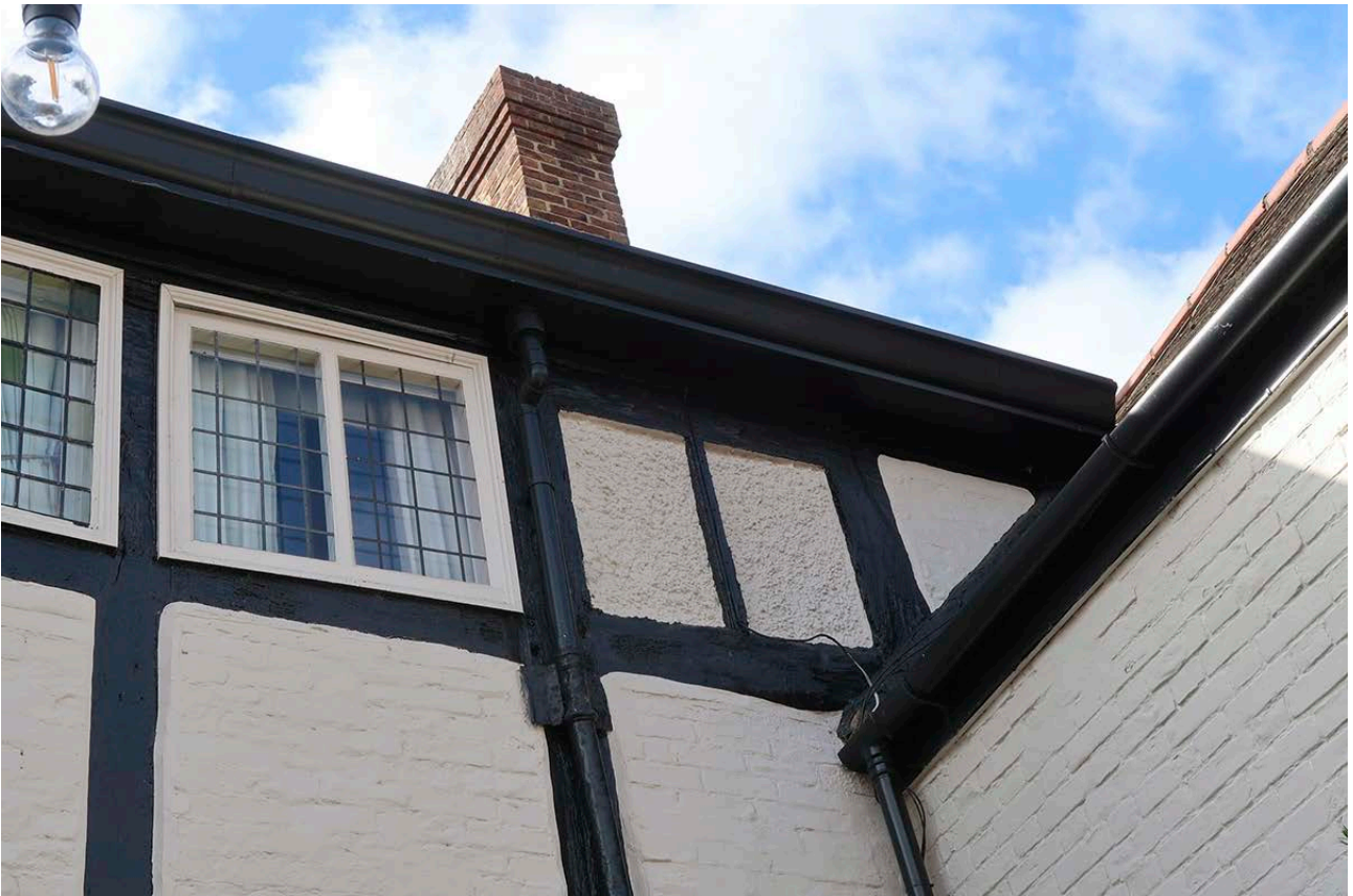
Figure 73: The original window at the west end of the north elevation of the north wing, with a moulded mullion surviving in the centre of the panel. [Johanna Roethe © Historic England]
