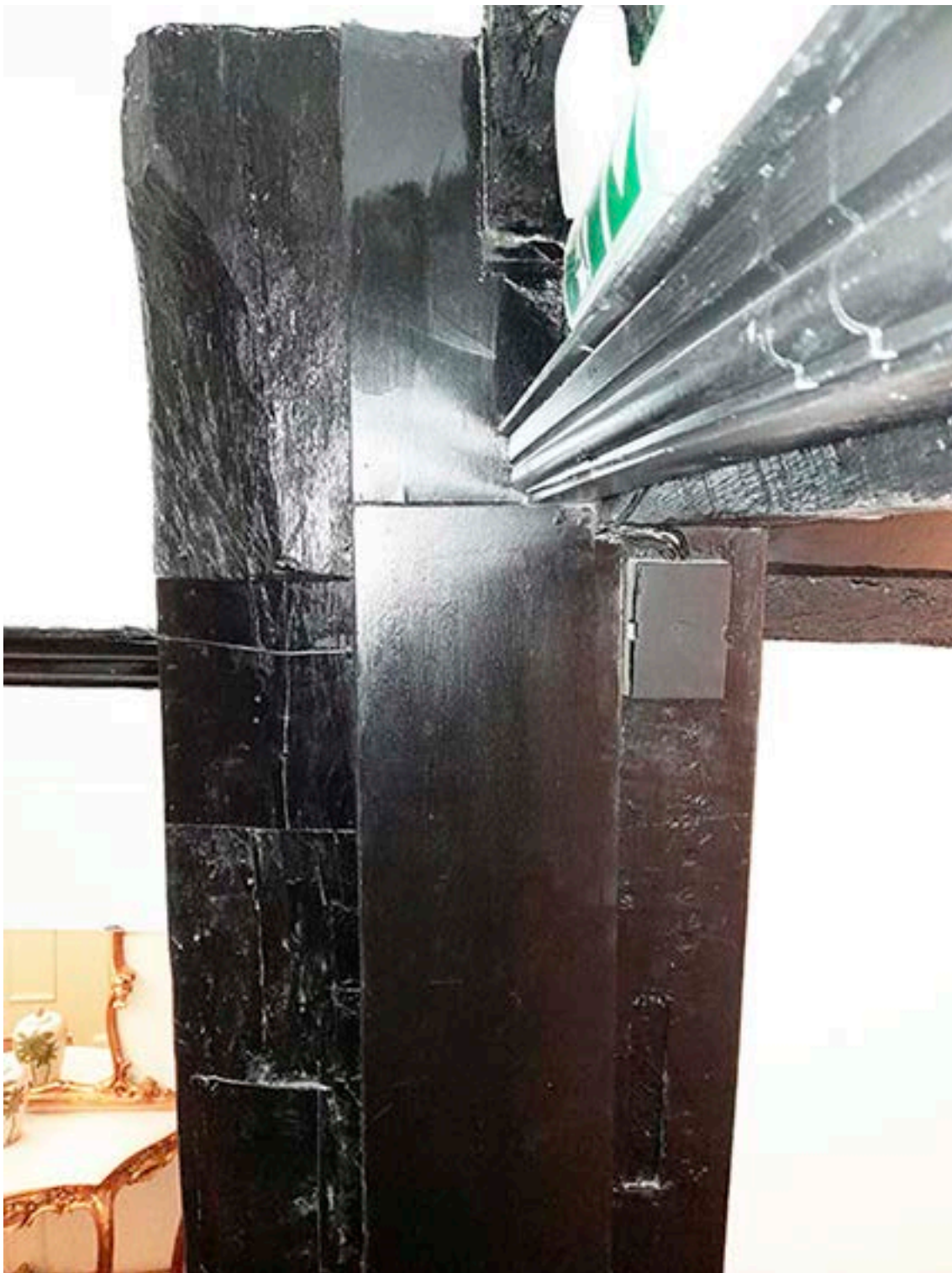
Figure 40: The south corner of the junction of the front range (left) and the north wing, seen at the first floor. The north wing's south-east corner post is to the right and a post belonging to the front range to the left. Their junction is obscured by a modern piece of timber. [Johanna Roethe © Historic England]
