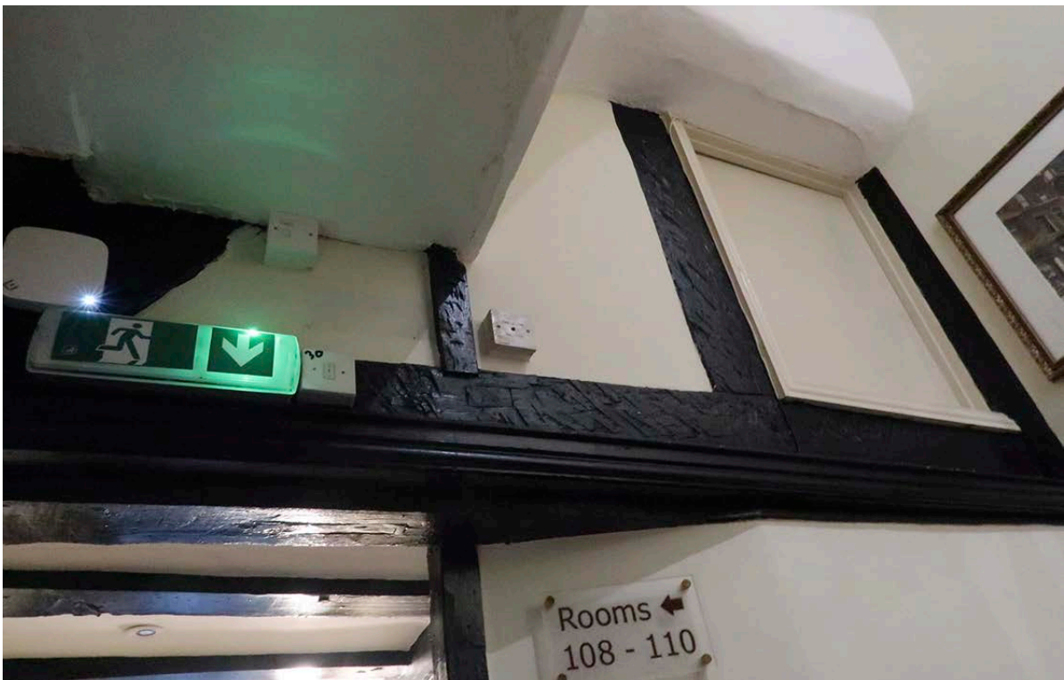
Figure 69: The east gable of the north wing, seen from the front range. [Johanna Roethe © Historic England]
