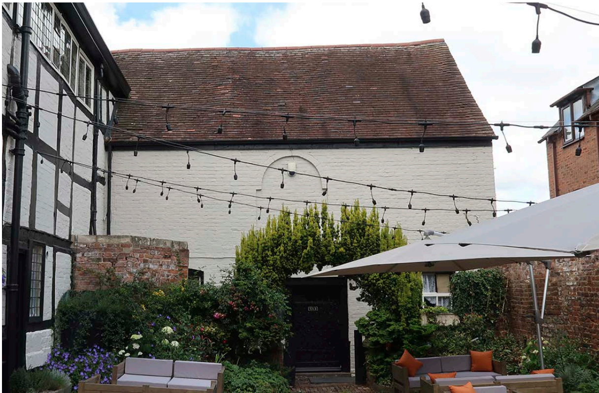
Figure 91: The east elevation of the stable block. [Johanna Roethe © Historic England]
