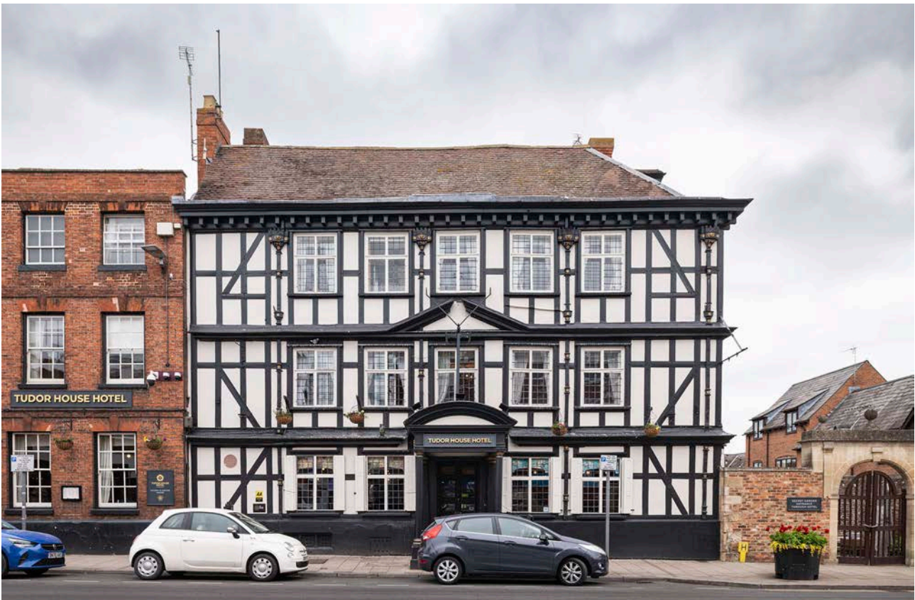
Figure 93: The east elevation in 2023. [Steven Baker © Historic England Archive, DP325757]
