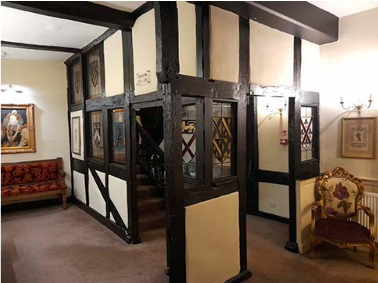
Figure 54: The box-framed stairwell at first-floor level. [Johanna Roethe © Historic England]
