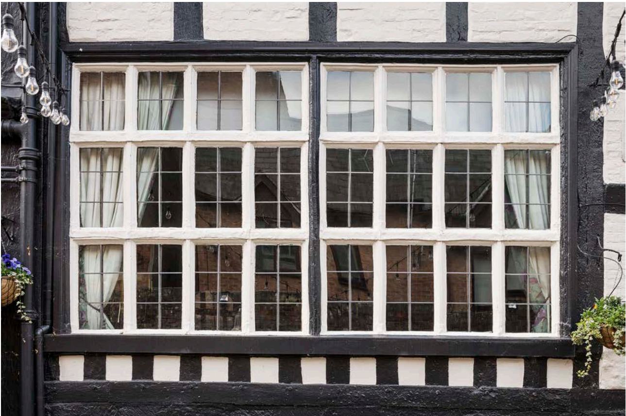
Figure 70: The large window in the north elevation of the north wing. [Steven Baker © Historic England Archive, DP325761]
