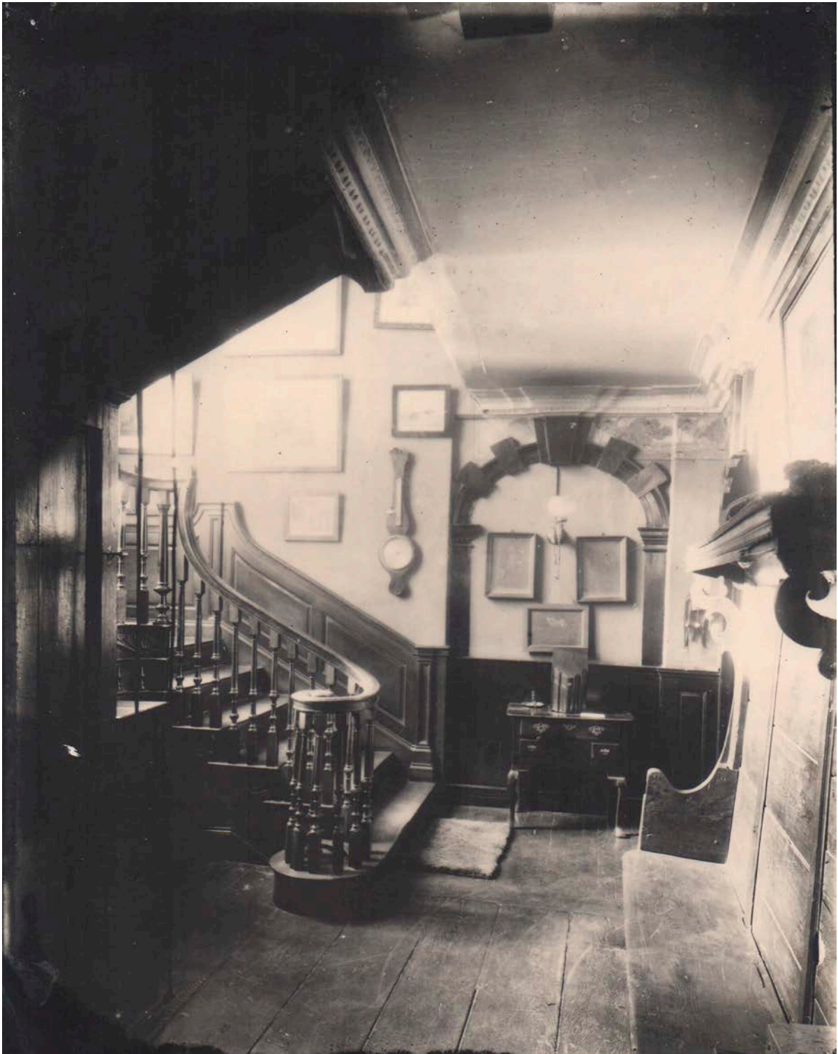
Figure 13: The stairwell in the front range, looking towards the blocked door into the hall in the north wing. The photograph was probably taken in around 1910, before the alterations for the Moore family. [The John Moore Society; reproduced with permission]
