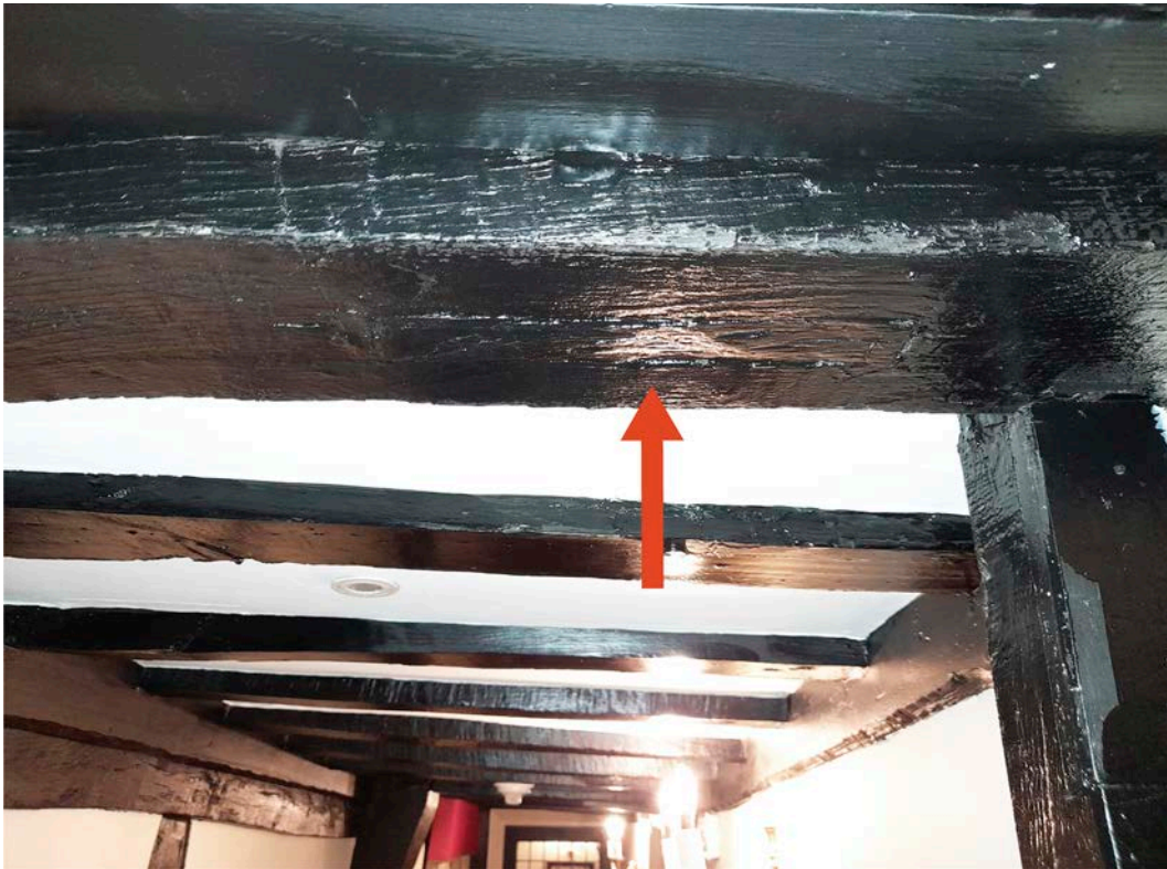
Figure 68: The mortice for an up-brace in the tiebeam at the east end of the north wing, with two off-centre peg holes above. [Johanna Roethe © Historic England]
