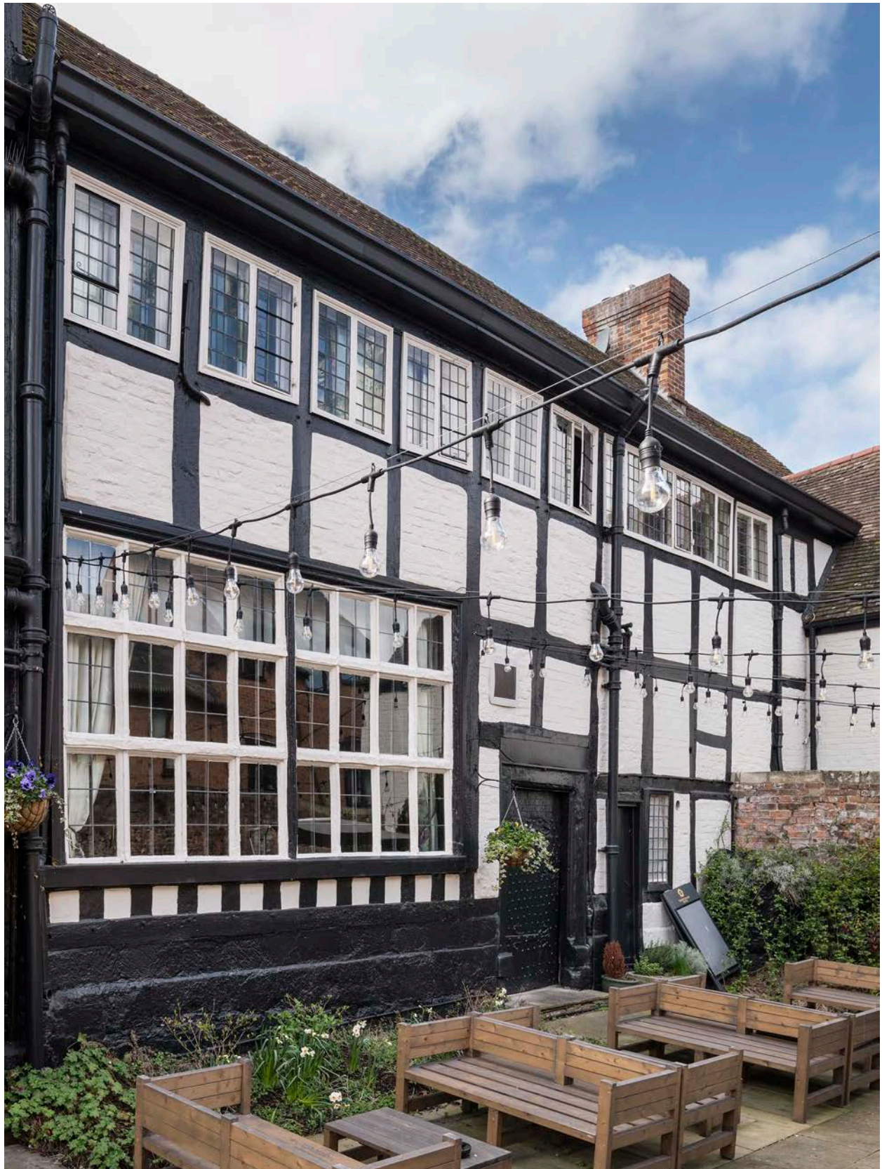
Figure 66: The north elevation of the north wing from the north-east. [Steven Baker © Historic England Archive, DP325760]
