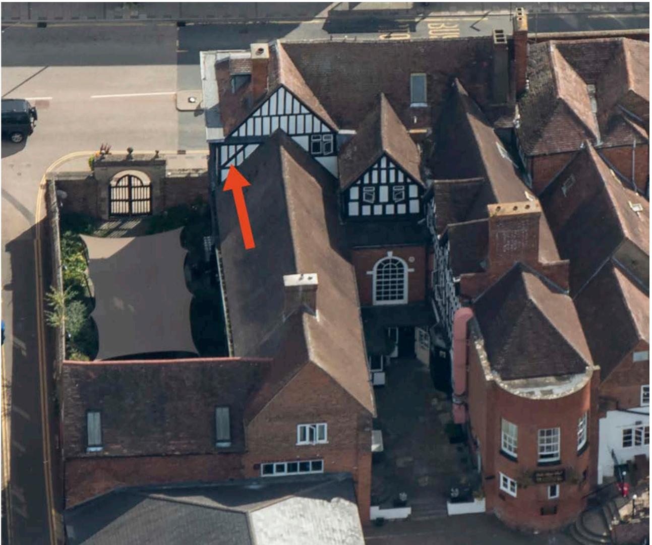
Figure 41: Aerial photograph of the Tudor House Hotel from the north-west. The red arrow indicates the remaining timber from the original, lower gable. [Damian Grady © Historic England Archive, 35124_023]
