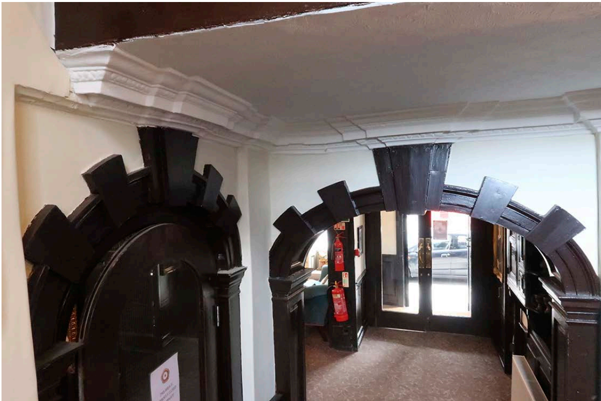
Figure 84: The timber arches on the ground floor, seen from the stair. [Johanna Roethe © Historic England]
