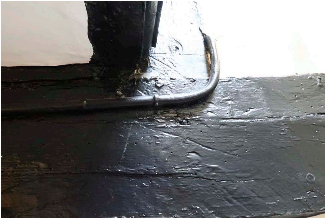
Figure 53: Carpenter's marks (possibly V for 5) on the south end of the south wing's easternmost truss, the fifth from the west. [Johanna Roethe © Historic England]
