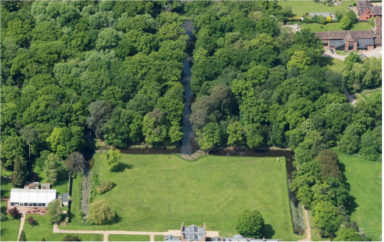
Figure 7: The ornamental canal looking west photographed in 2018. Traces of the St Andrew's crosses are also visible in the lawn. 33637_021 18-MAY-2018 © Historic England Archive.
