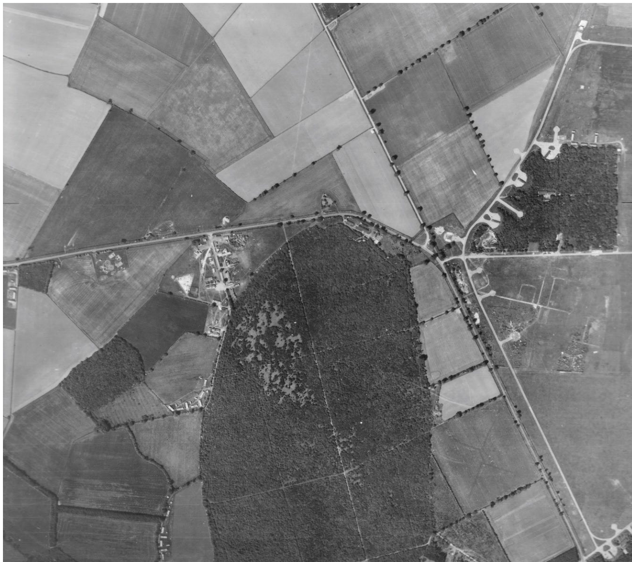
Figure 29: Extract of RAF aerial photographs showing the western perimeter road and hard-standings and dispersals of RAF Collyweston. To the west of Collyweston Great Wood is further dispersed accommodation huts and sewage works. Patchy tree growth within the wood is due to disturbance caused by historic quarrying. RAF/CPE/UK/2109 4026 28-MAY-1947 Source: Historic England Archive (RAF Photography).
