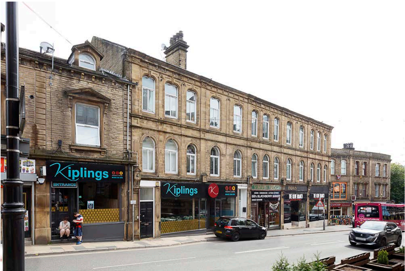
Figure 73: Row of shops at nos 20-28 Town Hall Street, viewed from the east. [Alun Bull, 2022 © Historic England, DP372542].
