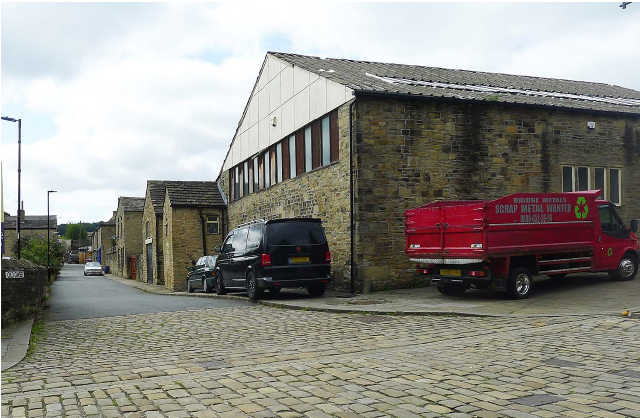
Figure 56: Wharf Garage at the corner of Old Cawsey, viewed from the east. [Lucy Jessop, 2021 © Historic England].
