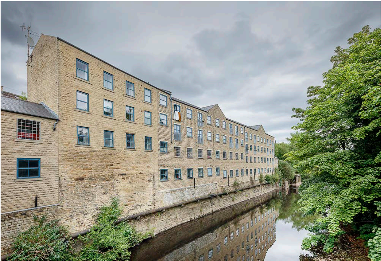
Figure 52: Kingfisher Chase, built in the 1990s following the demolition of Lock Hill Mills on the same site, viewed from the south-west. The lower courses of stonework and a portion of the left (west) taller section of the building appear to incorporate older reused stone. [Alun Bull, 2022 © Historic England, DP372750].
