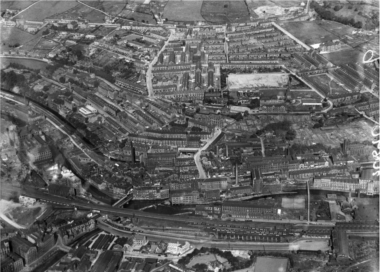
Figure 23: Aerial photograph of Sowerby Bridge from the south, taken in 1931 [© Historic England Archive (Aerofilms Collection), EPW036870].
