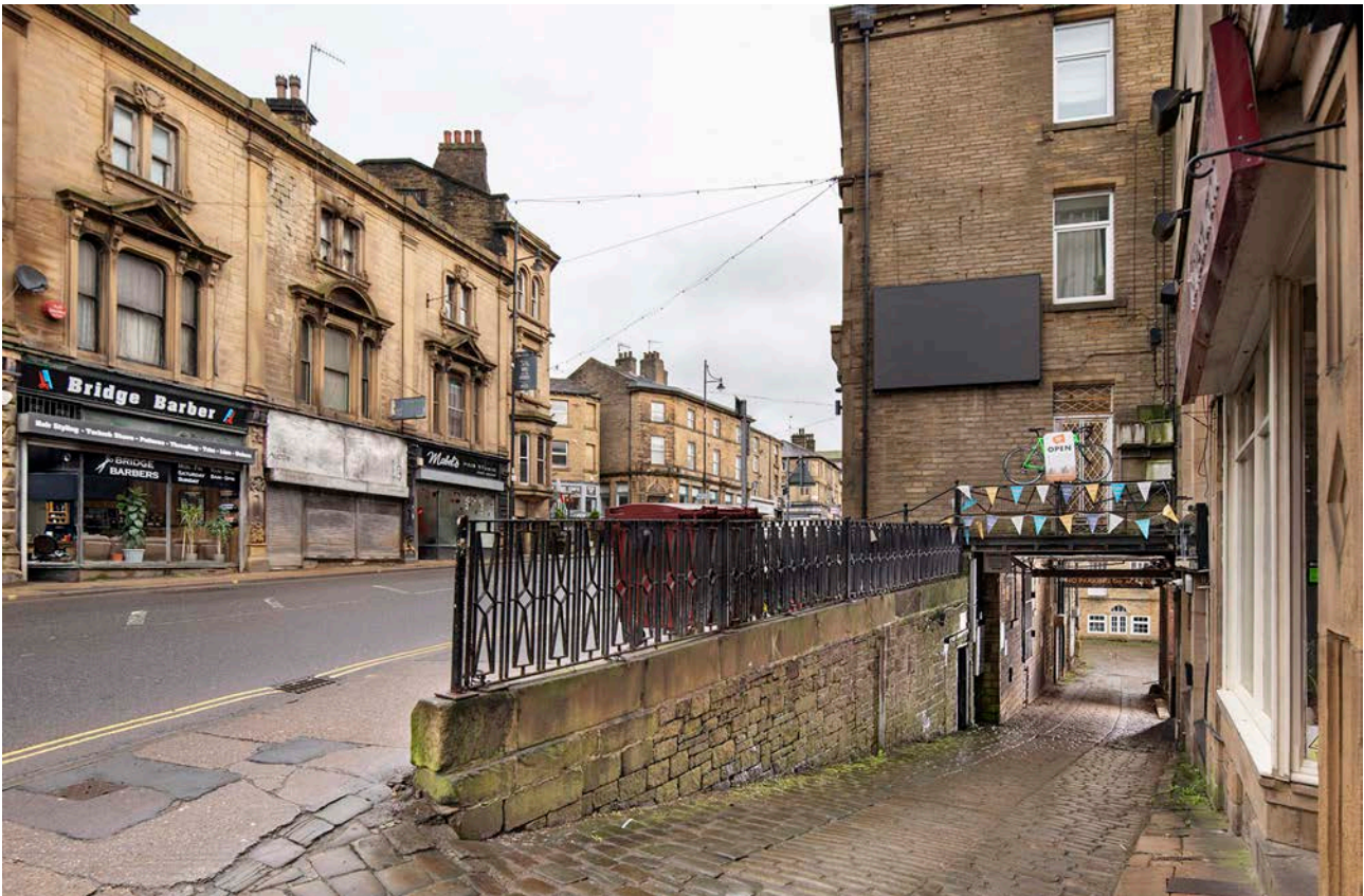
Figure 42: Passageway leading to the former mill yard of Sowerby Bridge Mills and demonstrating the way in which the topography has been used to the best advantage of construction. [James O. Davies, 2024 © Historic England, DP437018].
