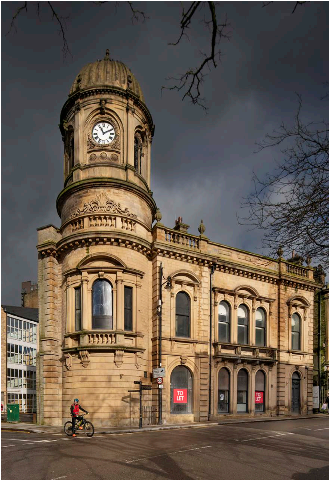
Figure 71: Former Sowerby Bridge Town Hall, opened in 1857, viewed from south-east. [James O. Davies, 2024 © Historic England, DP437048].
