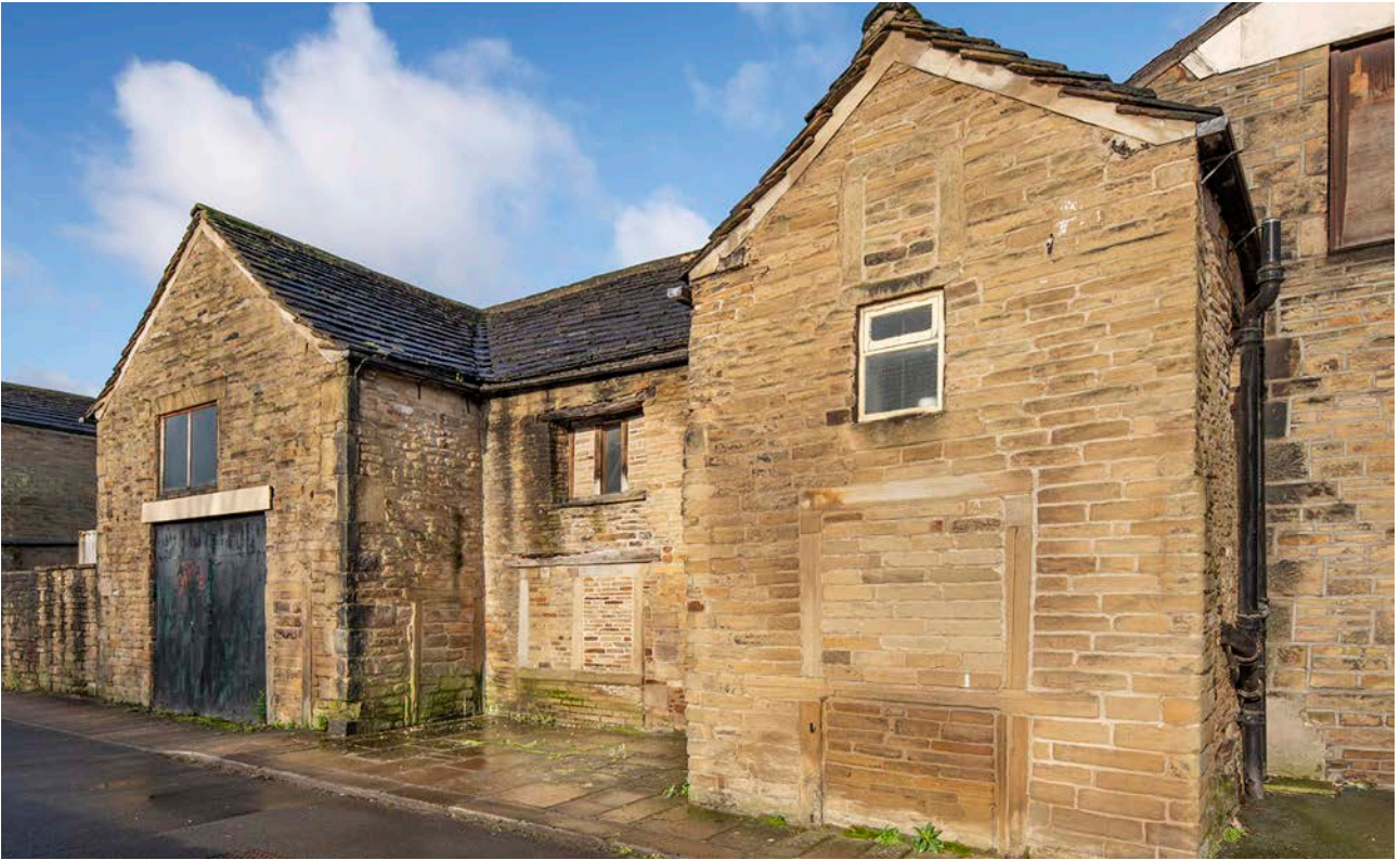
Figure 57: South elevation of older sections of Wharf Garage showing mullioned windows and stone quoins that may be indicative of a 16th-century date, viewed from the south. [James O. Davies, 2024 © Historic England, DP436990].
