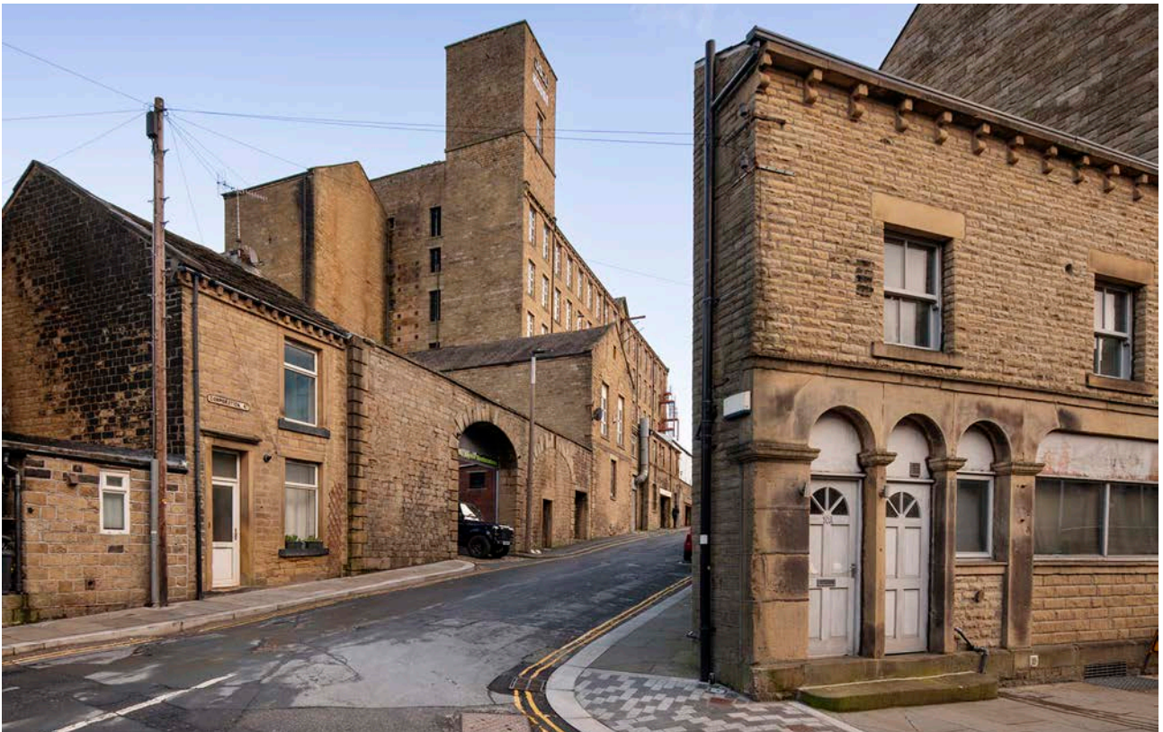
Figure 36: Corporation Mill, Corporation Street taken from south-west. [James O. Davies, 2024 © Historic England, DP436997].
