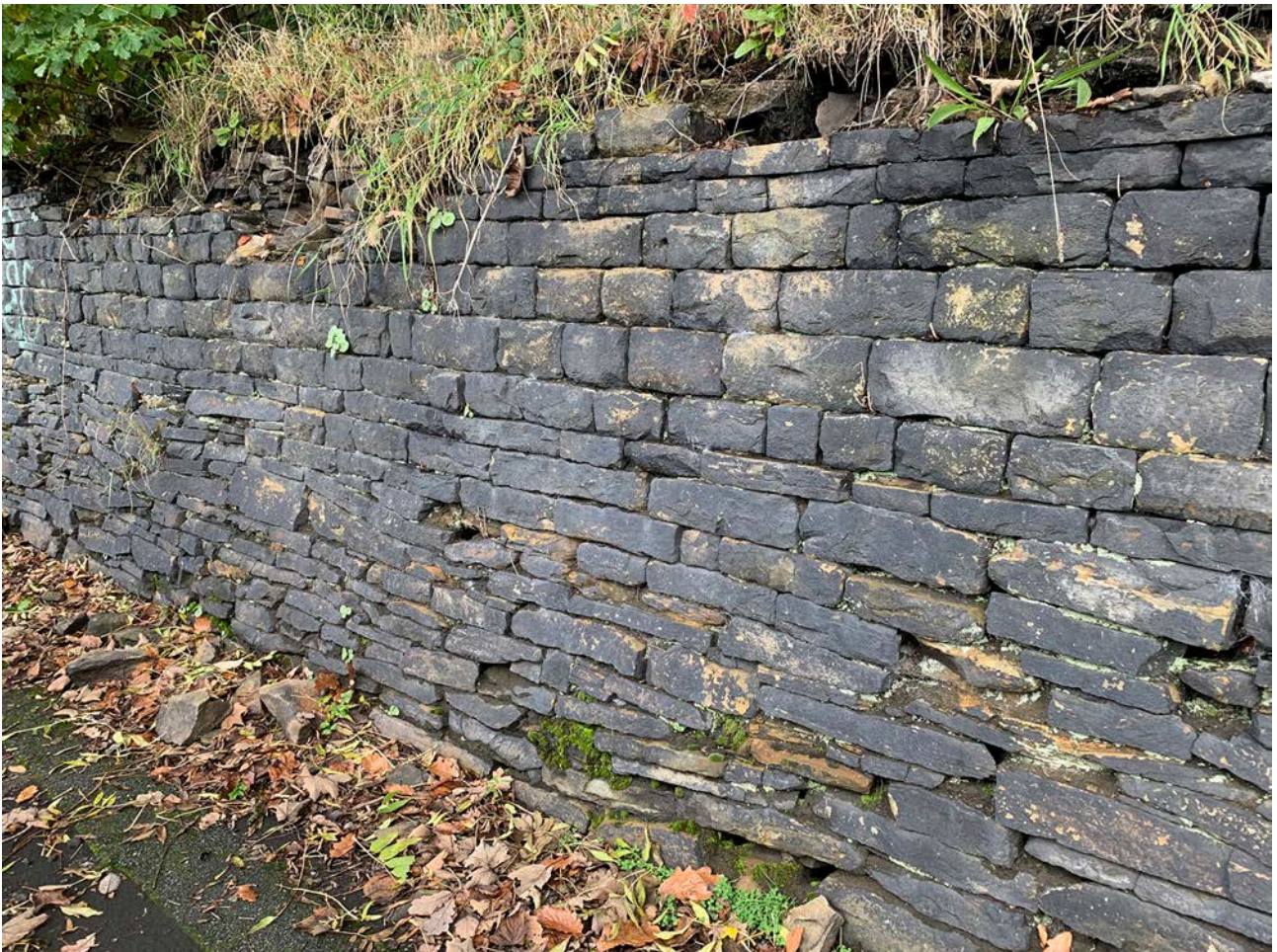
Figure 22: Blackened stonework of a drystone wall along Hollins Mill Lane. [Clare Howard, 2023 © Historic England].
