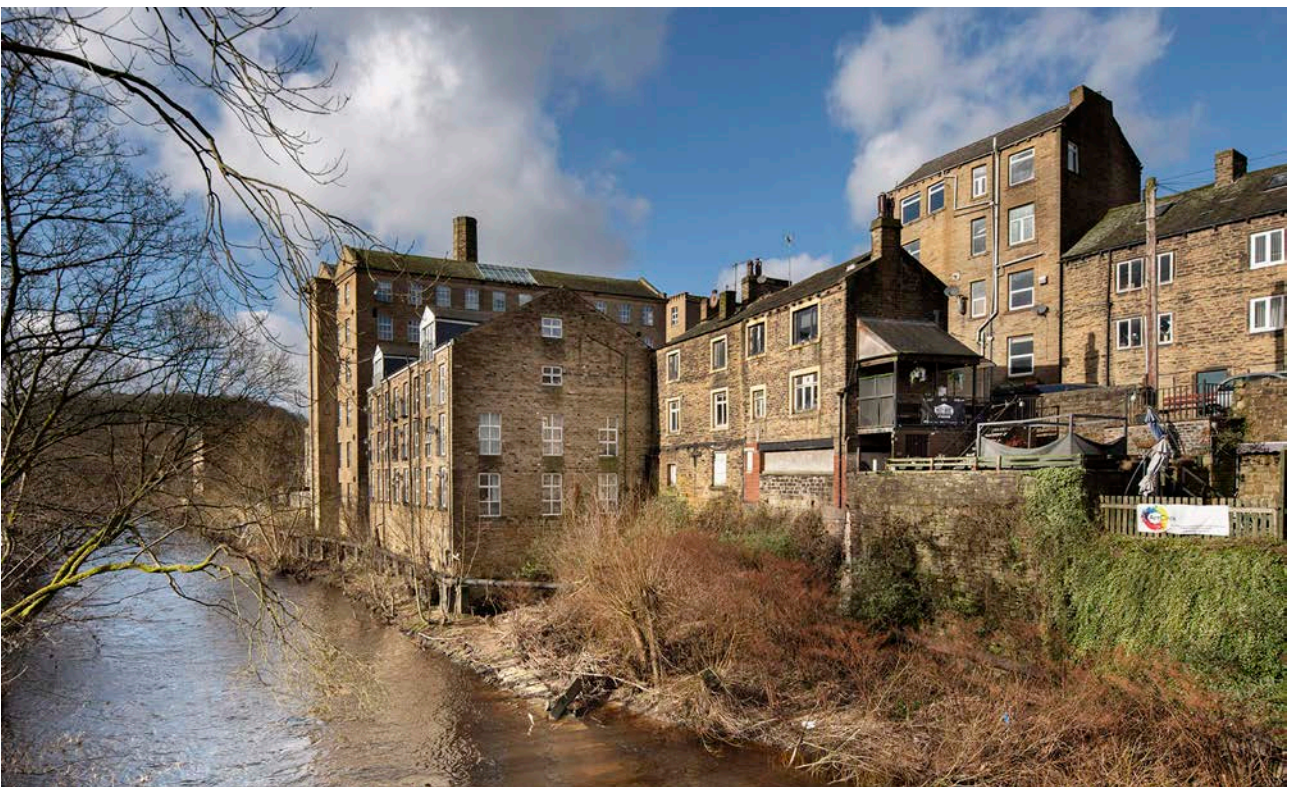
Figure 48: Carlton Mill and weaving shed following the Sowerby Bridge Riverside Development project. [James O. Davies, 2024 © Historic England, DP436993].
