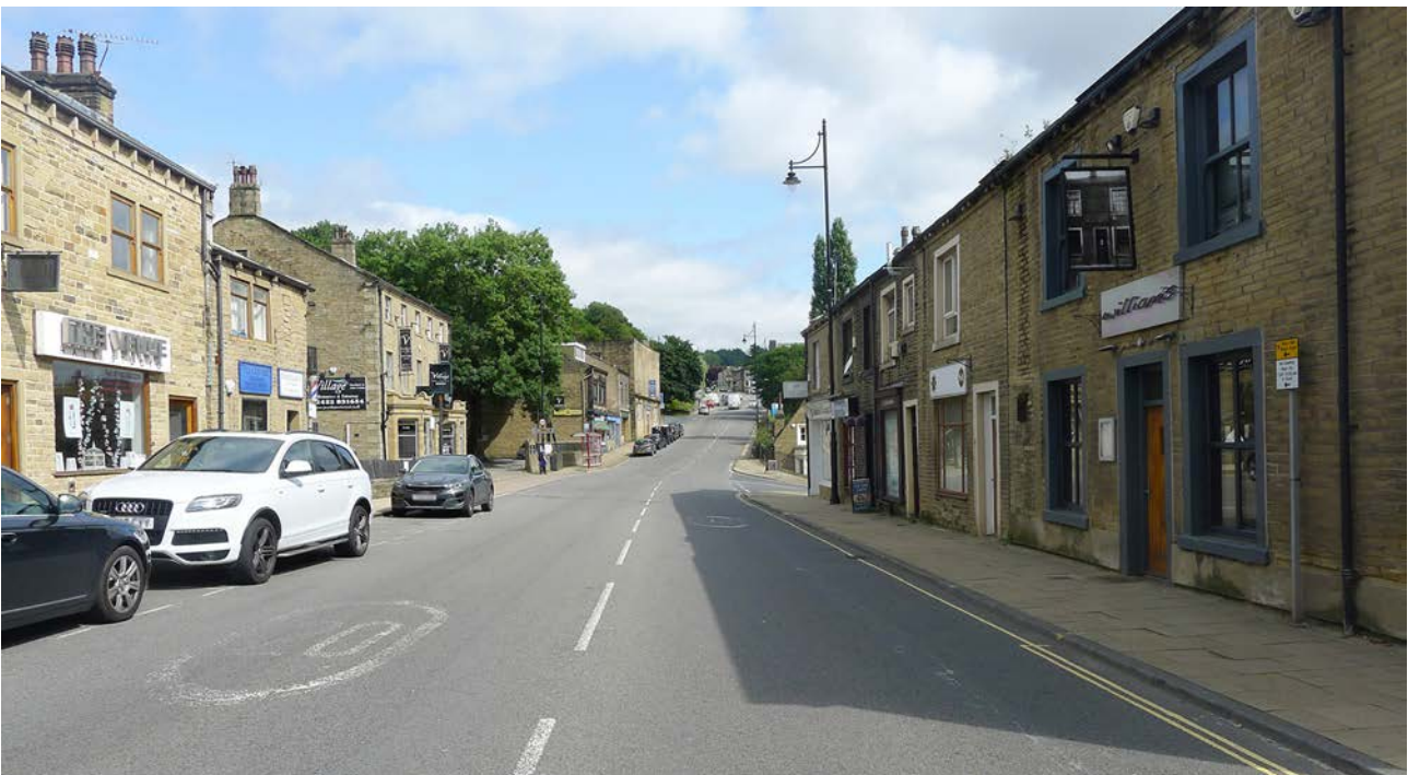
Figure 94: View of eastern part of Wharf Street showing lower buildings, a wider street and increased amount of space, viewed from west (Lucy Jessop, 2021 © Historic England).
