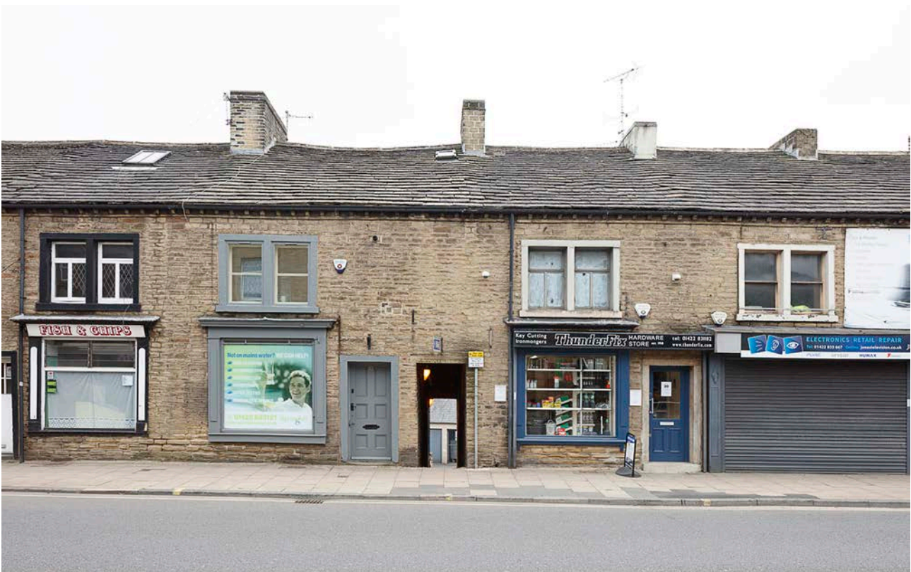
Figure 89: Late 18th-/early 19th-century back-to-back houses on the south side of Wharf Street, viewed from north. [Alun Bull, 2022 © Historic England, DP372559].
