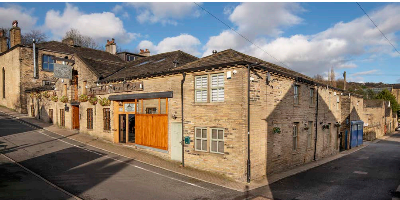
Figure 54: Former warehouse, now the Hog's Head Brew House, Stanley Street, viewed from the south. [James O. Davies, 2024 © Historic England, DP437012].
