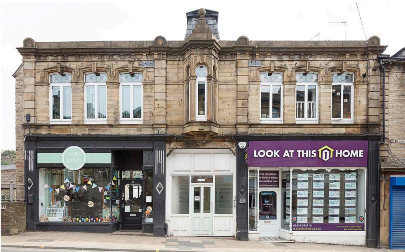
Figure 75: Nos 38 and 40 Town Hall Street, built as a pair of shop about 1906, viewed from north. [Alun Bull, 2022 © Historic England, DP372566].
