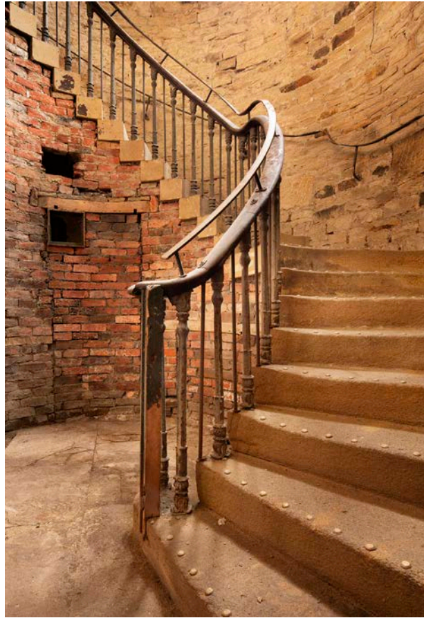
Figure 72: Staircase inside the tower of the former town hall. [James O. Davies, 2024 © Historic England, DP437042].
