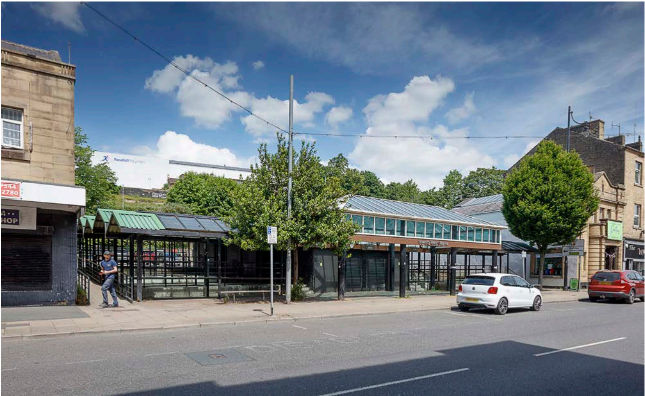
Figure 84: Former market (since demolished) on the site of the former Bank Foundry, viewed from north-west. [Alun Bull, 2022 © Historic England, DP372675].
