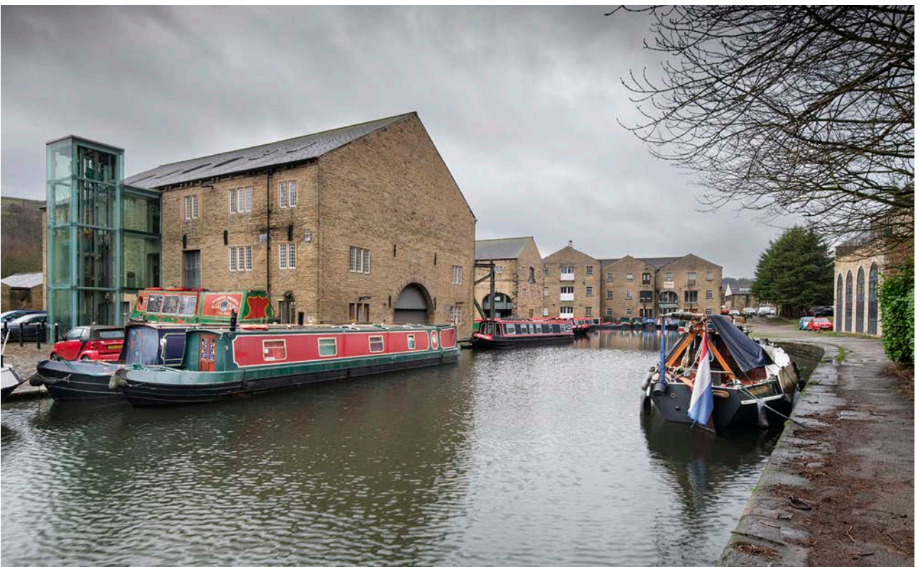
Figure 59: Sowerby Bridge Wharf showing large warehouses to the right and salt warehouse to the left, viewed from the north-east. [James O. Davies, 2024 © Historic England, DP436985].
