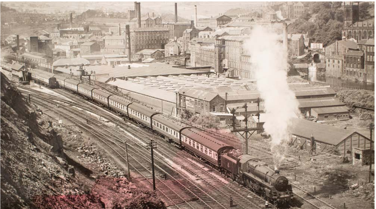
Figure 15: Undated photograph of Sowerby Bridge from the south-east showing the railway, Christ Church, and the mills and foundries on both sides of the Calder. [Calderdale Libraries, 32 923 512 and National Railway Museum].
