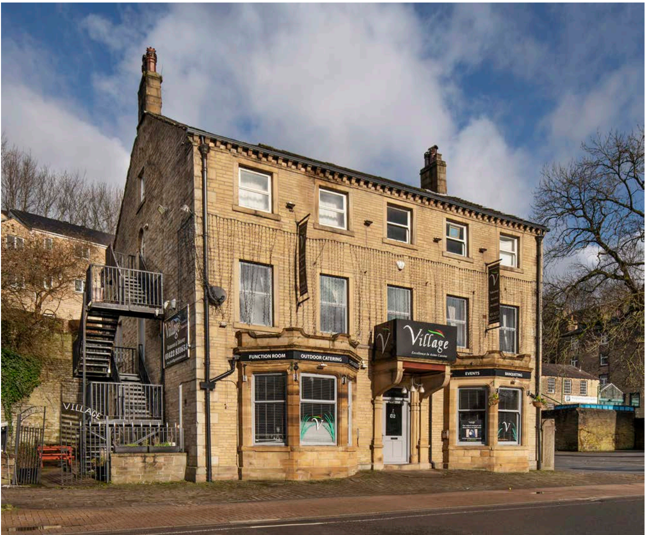
Figure 96: Former public house, perhaps originally a domestic house, now called Village, viewed from south. [James O. Davies, 2024 © Historic England, DP437013].
