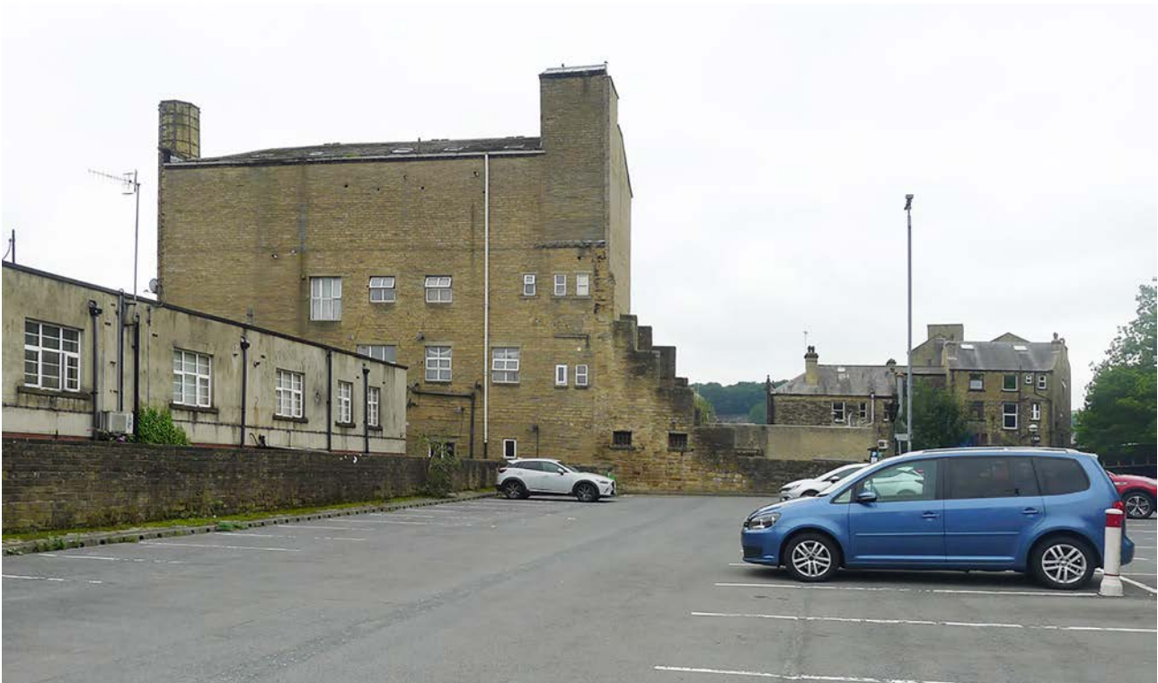
Figure 82: Site of Bank Foundry and the rear of former Centre Mills, viewed from the north east. [Lucy Jessop, 2021 © Historic England].
