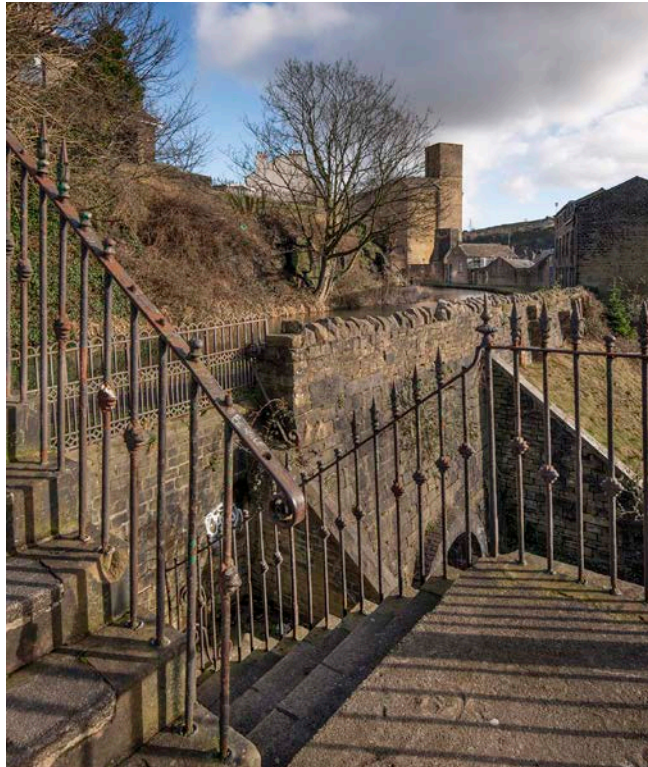
Figure 35: Revetment wall and stone stairwell leading to iron bridge over the Rochdale Canal, taken from south. [James O. Davies, 2024 © Historic England, DP437008].
