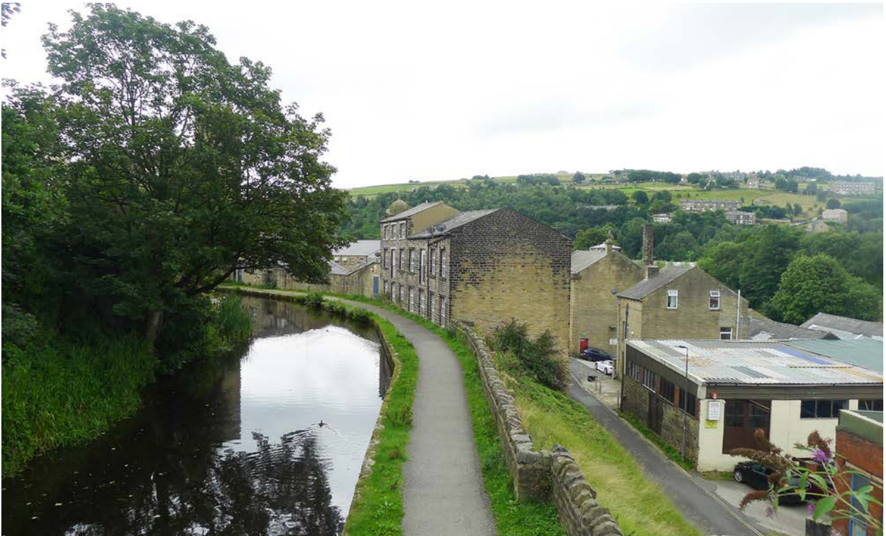
Figure 30: Rochdale Canal with Hollins Mill Lane set at a lower level to its right (south) [Lucy Jessop, 2021 © Historic England].
