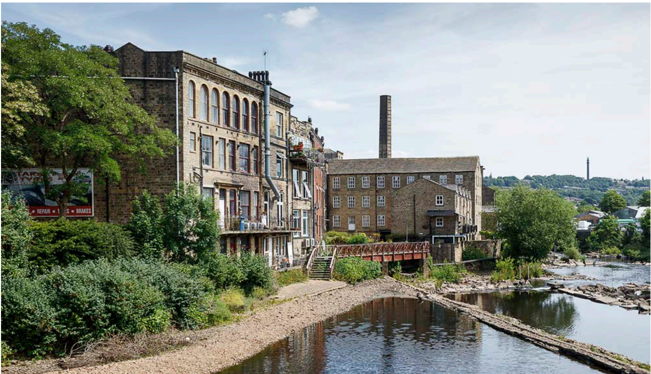
Figure 61: View of the River Calder with the rear of properties along Town Hall Street and Sowerby Bridge Mills on its north bank, viewed from County Bridge to the west. [Alun Bull, 2022 © Historic England, DP372574].
