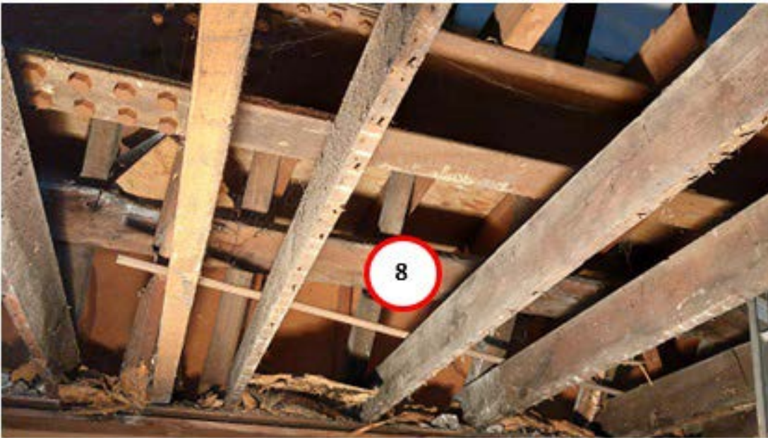
Figure 4 Annotated photograph of bay 2, viewed looking east (photograph Robert Howard)
