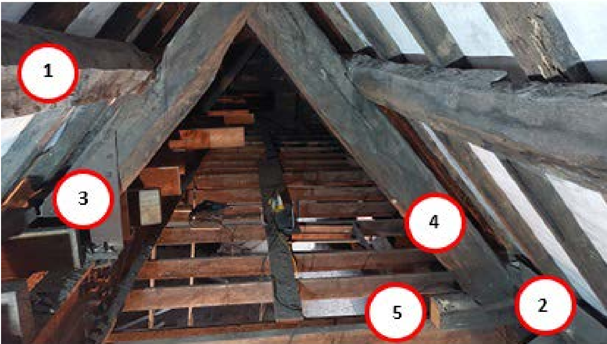
Figure 2 Annotated photograph of truss 1/bay 1, viewed looking south (photograph Robert Howard)
