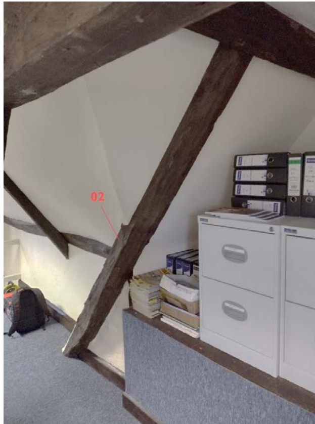
Figure 3: View of the turned principal rafter (towd02) looking south-east [photo Martin Bridge]
