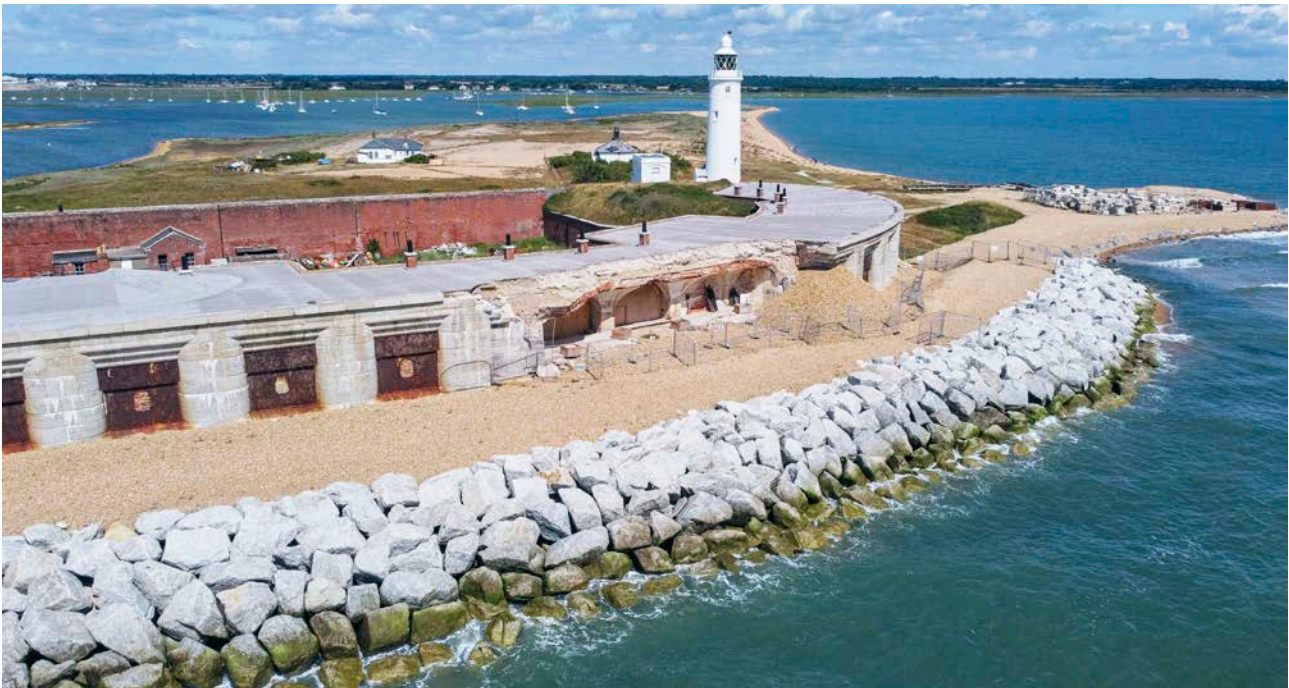
Figure 12: A rock armour revetment has been added to the East Wing of Hurst Castle following the collapse. © Historic England. English Heritage Trust
