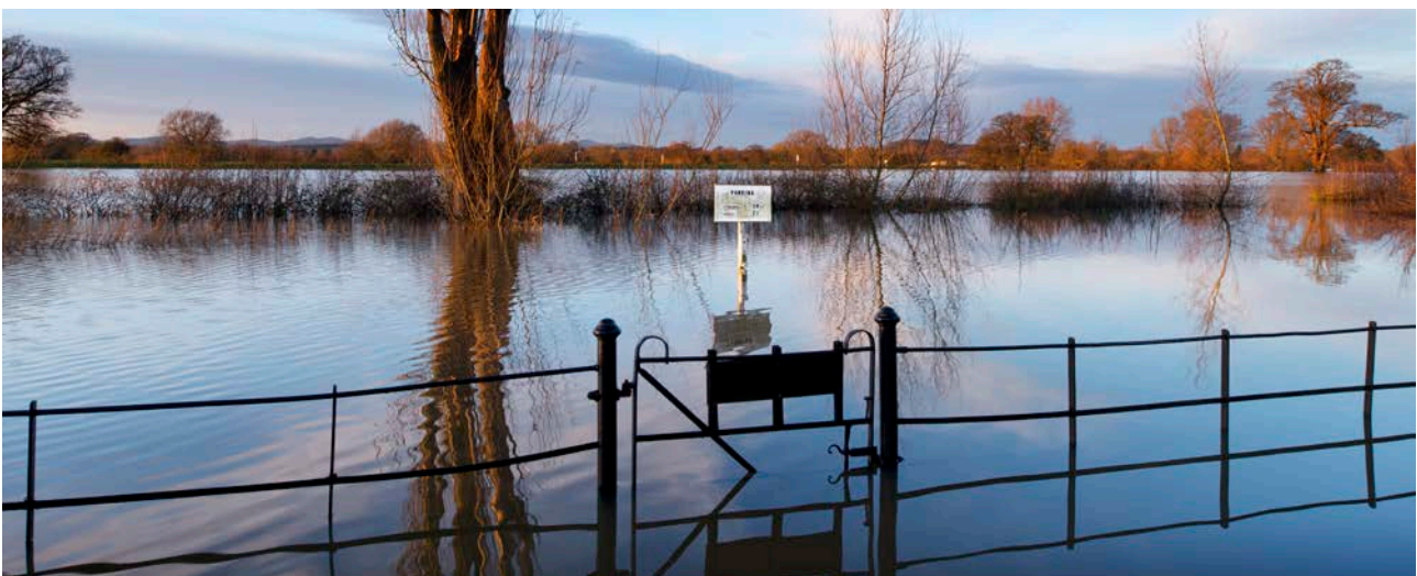
Figure 1: A flooded car park near Odda's Chapel, Tewkesbury, in 2016. Flooding can cause damage to historic buildings and landscapes, as well as access issues for visitors, staff and emergency responders. © Historic England
