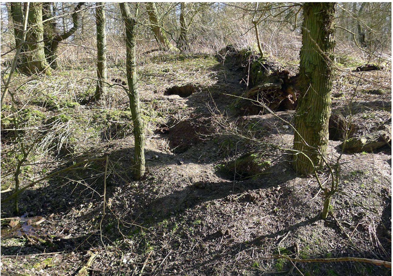
Figure 19 – Badger damage at the north-west corner of the moat island From the west (Sarah Newsome, February 2015, © Historic England)
