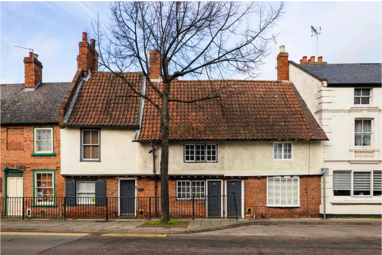
Figure 90: Nos 40-44 Castle Gate, which contains timbers dendrochronologically dated to 1330. [Stella Fitzgerald © HEA DP313605.]
