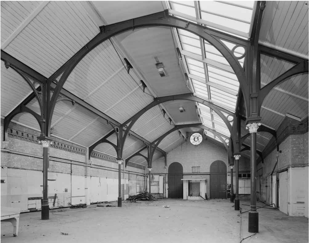
Figure 69: Market Hall in the late 20th century prior to redevelopment [© HEA BB93_29922.]
