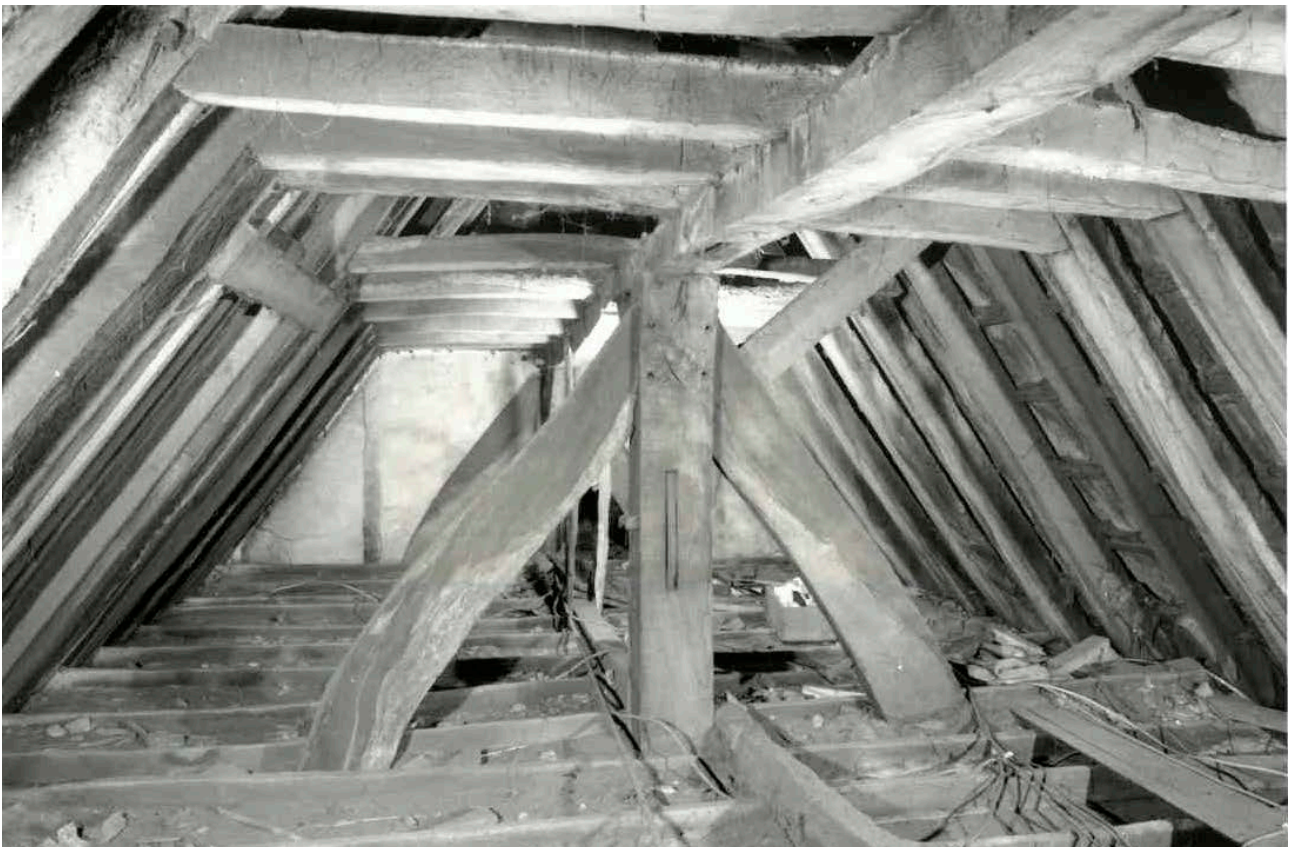
Figure 48: Roof structure over 22-24 Kirk Gate. [© HEA AA97_576.]
