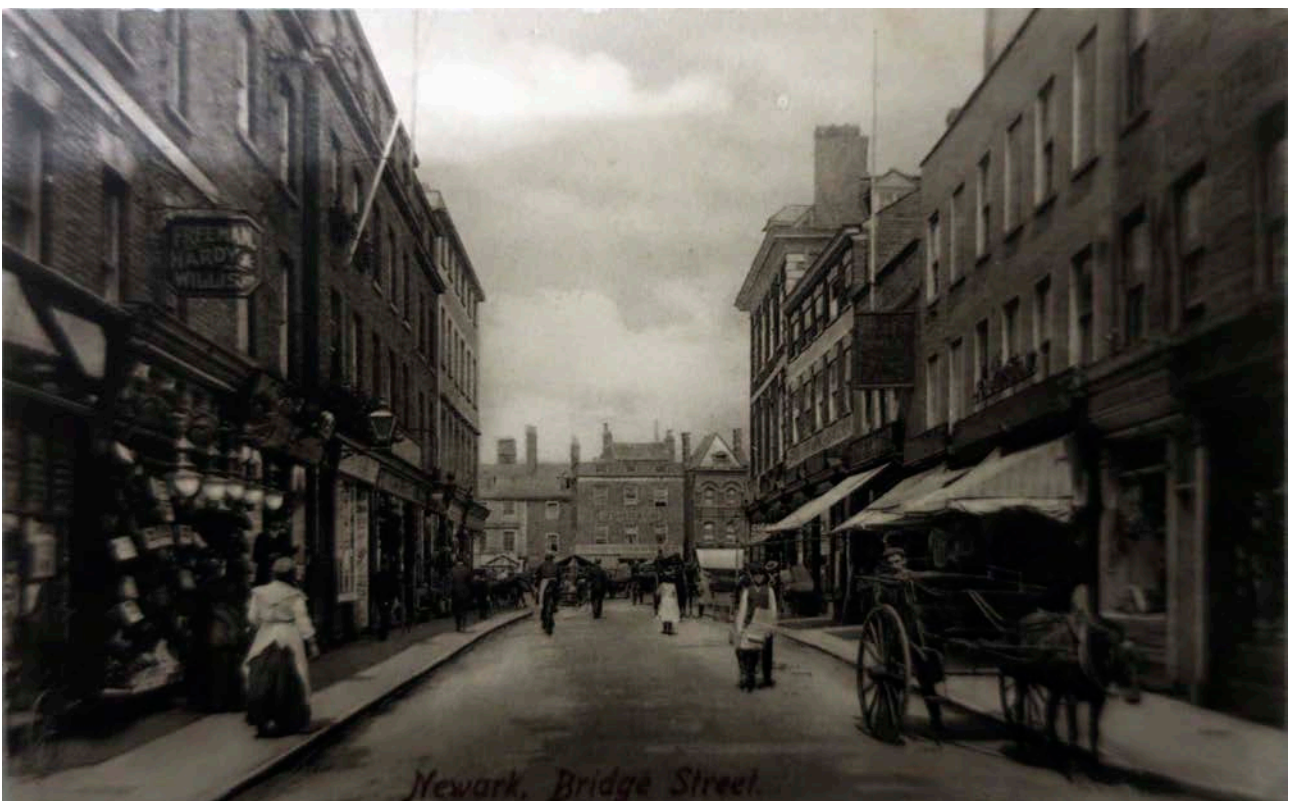
Figure 74: Bridge Street in around 1900 looking south towards the Market Place. [© Newark Resource Centre ref. 6080.]
