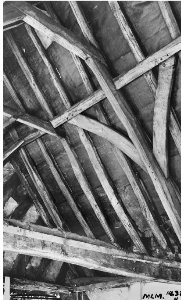
Figure 39: Queen's Head Hotel roof structure prior to restoration [© HEA OP36285.]
