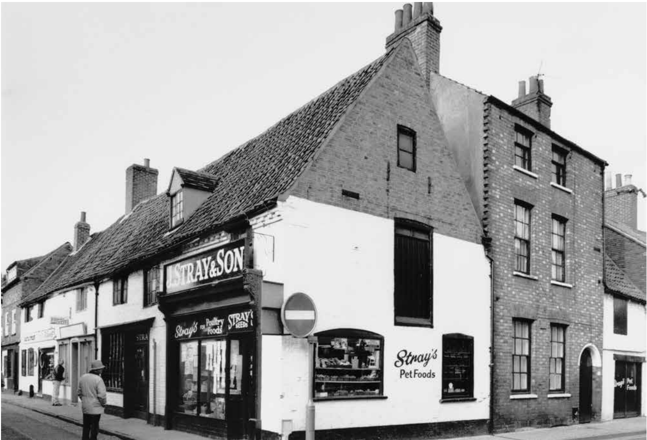
Figure 70: Nos 17-21 Boar Lane with 18 Middle Gate beyond [© HEA OP36288.]
