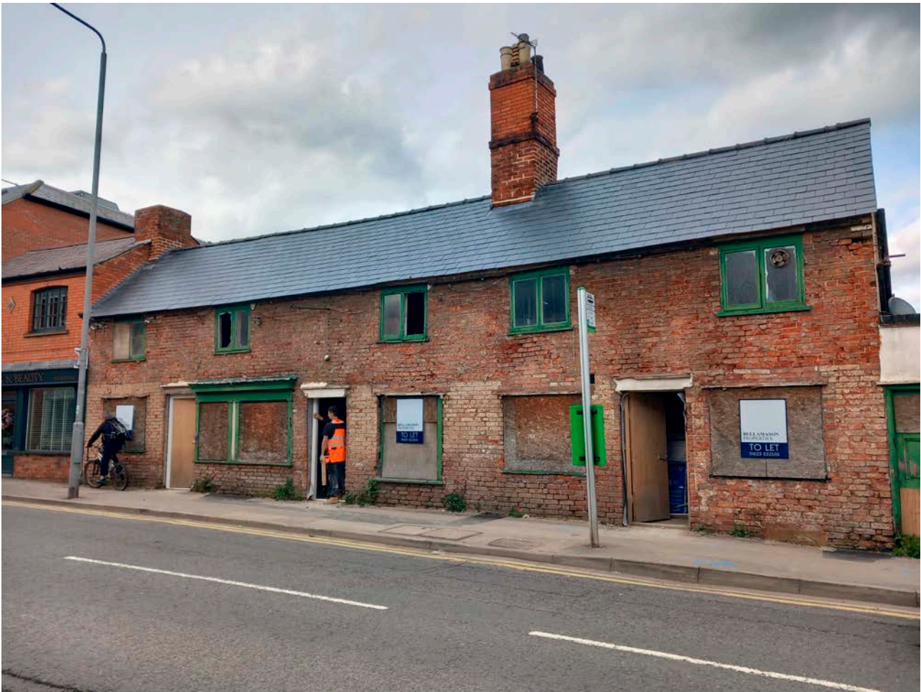
Figure 133: 4-6 Portland Street under renovation in April 2023. [Aimee Henderson © Historic England.]
