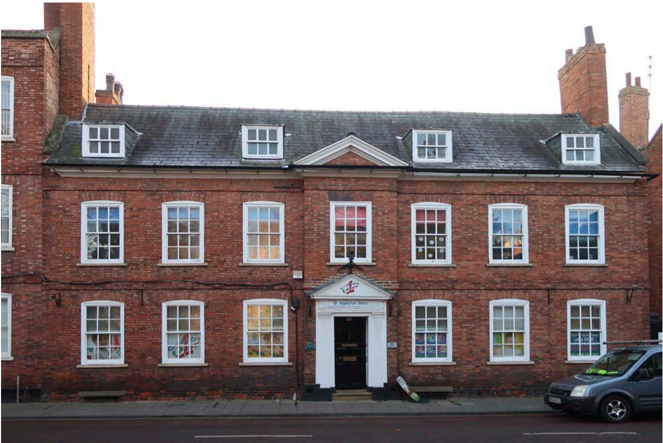
Figure 126: Martin Foster House, Appleton Gate. [Aimee Henderson © Historic England.]
