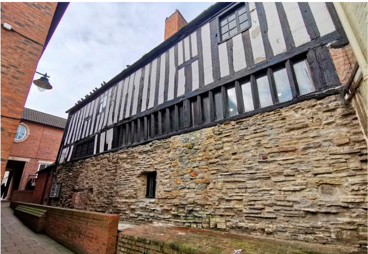
Figure 60: The Governor's House, rear range west elevation. [Aimee Henderson © Historic England.]
