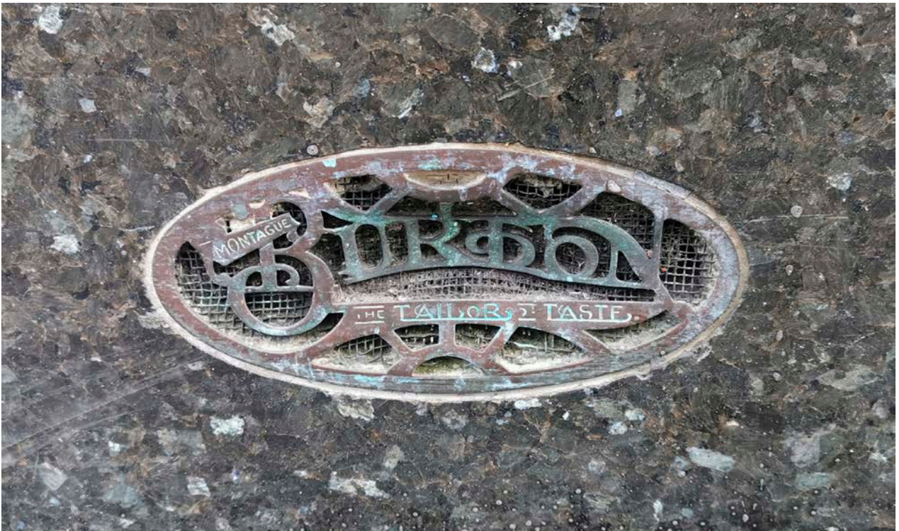
Figure 65: Bronze 'Burton' vent at 16-17 Stodman Street. [Aimee Henderson © Historic England.]
