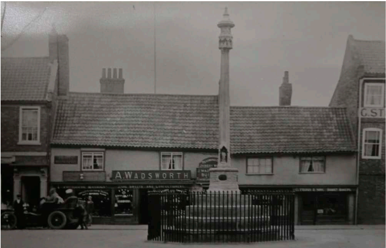
Figure 130: Undated early 20th century photograph of Beaumont Cross looking eastwards. [© Newark Resource Centre ref. 2362.]
