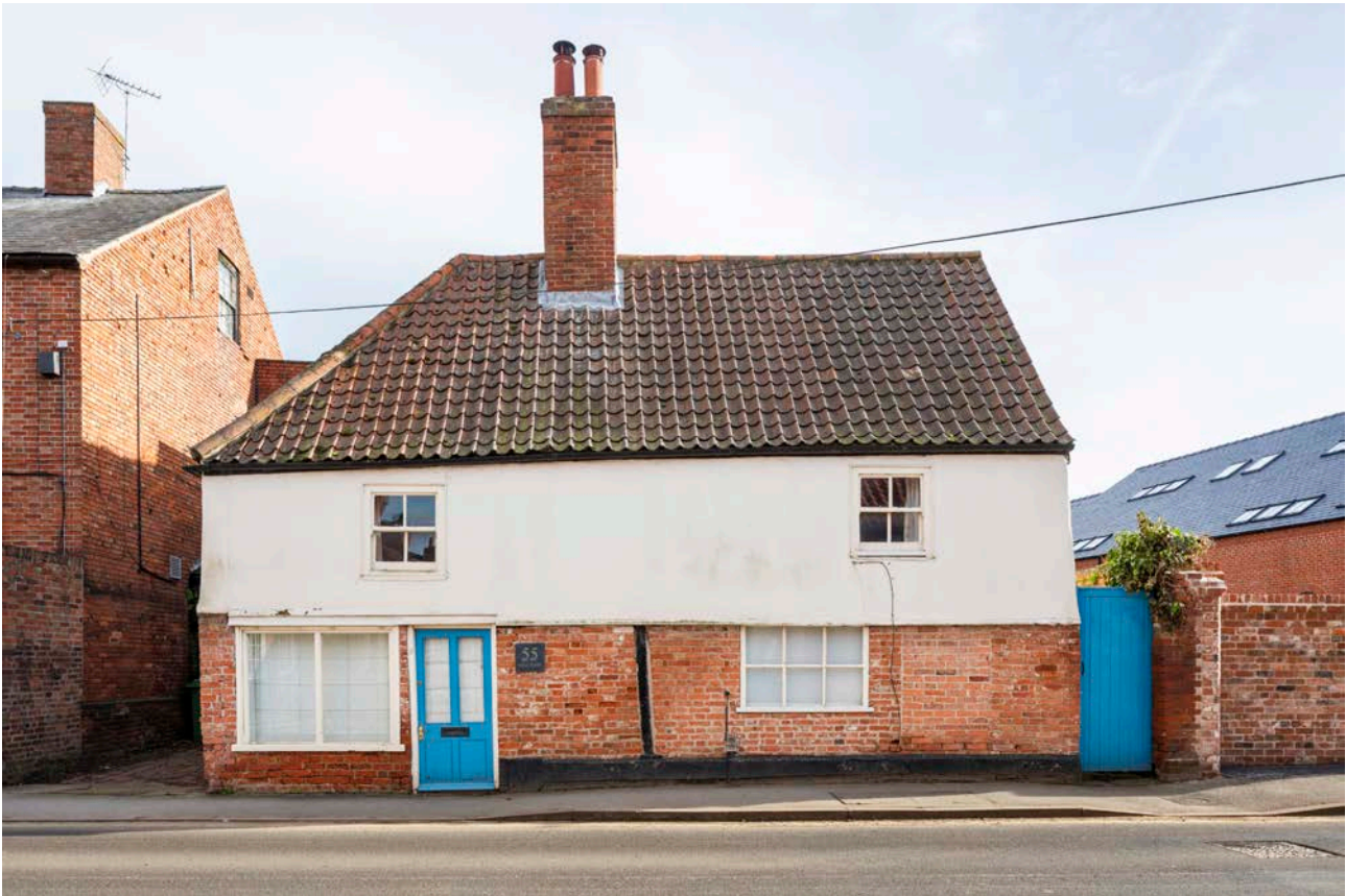
Figure 113: No. 55 Mill Gate, a 17th-century timber-framed building later adapted to form part of a maltings complex to the rear. [Stella Fitzgerald © HEA DP313604.]
