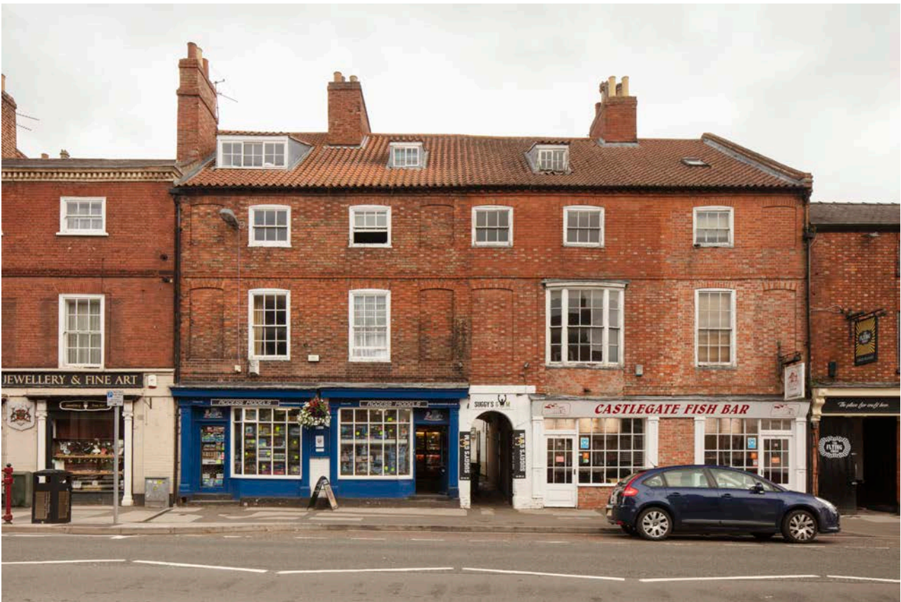
Figure 92: Nos 45-51 Castle Gate, Newark showing the use of buff-coloured header bricks to create a subtle chequer pattern. [Pat Payne © HEA DP393313.]
