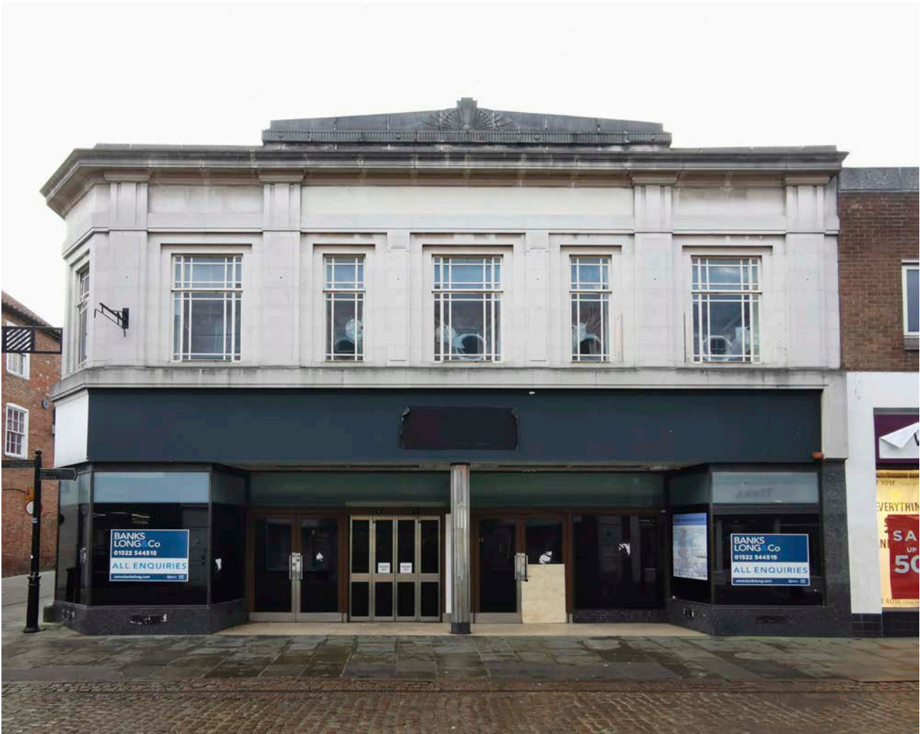
Figure 66: Former Marks and Spencers, 32 Stodman Street. [Aimee Henderson © Historic England.]
