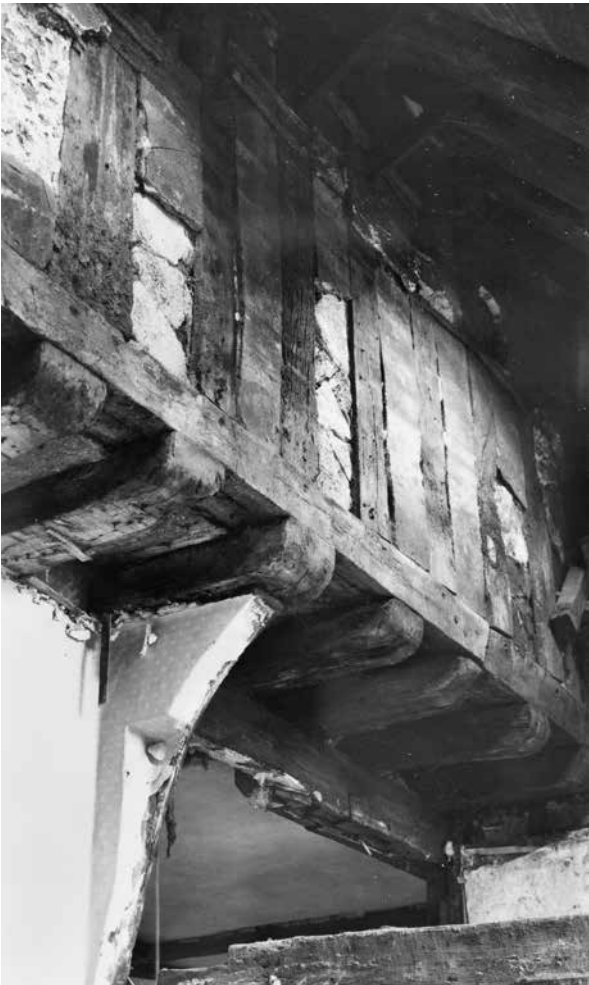
Figure 38: Queen's Head Hotel west elevation showing jetty prior to restoration [© HEA OP36286.]
