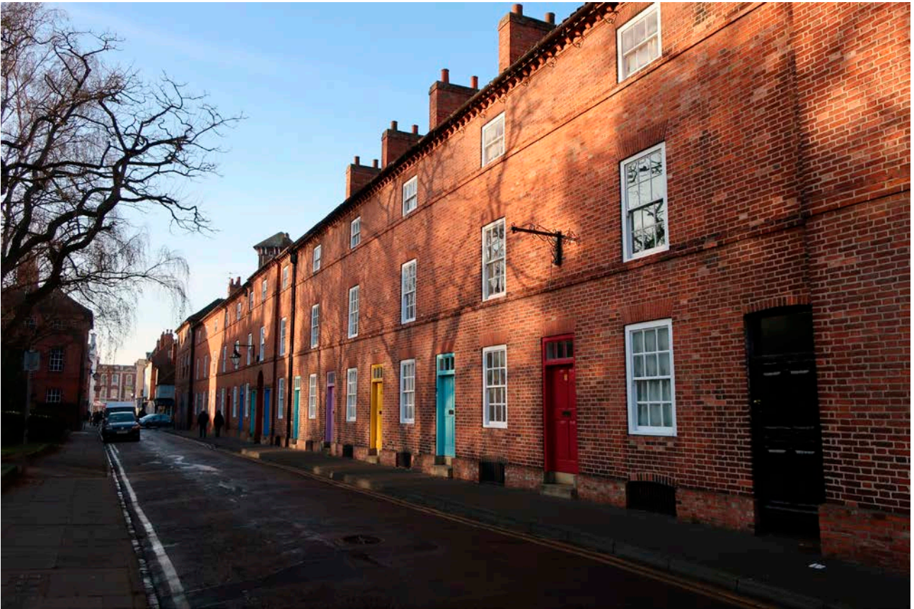
Figure 83: Wilson Street, west terrace in 2021. [Aimee Henderson © Historic England.]
