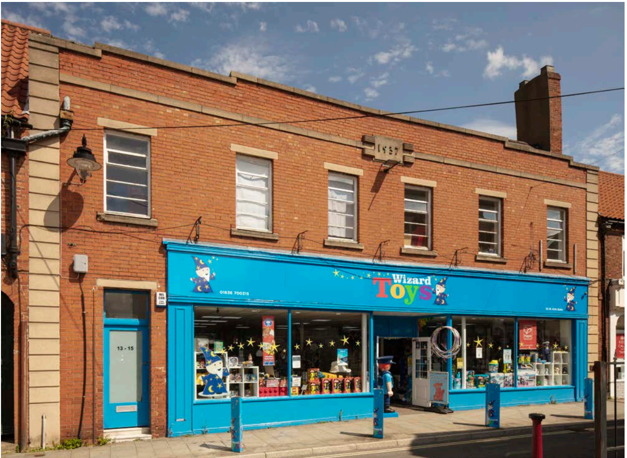
Figure 53: Former Co-operative Store and associated warehouse and hall, 13-17 Kirk Gate. [Pat Payne © HEA DP393308.]
