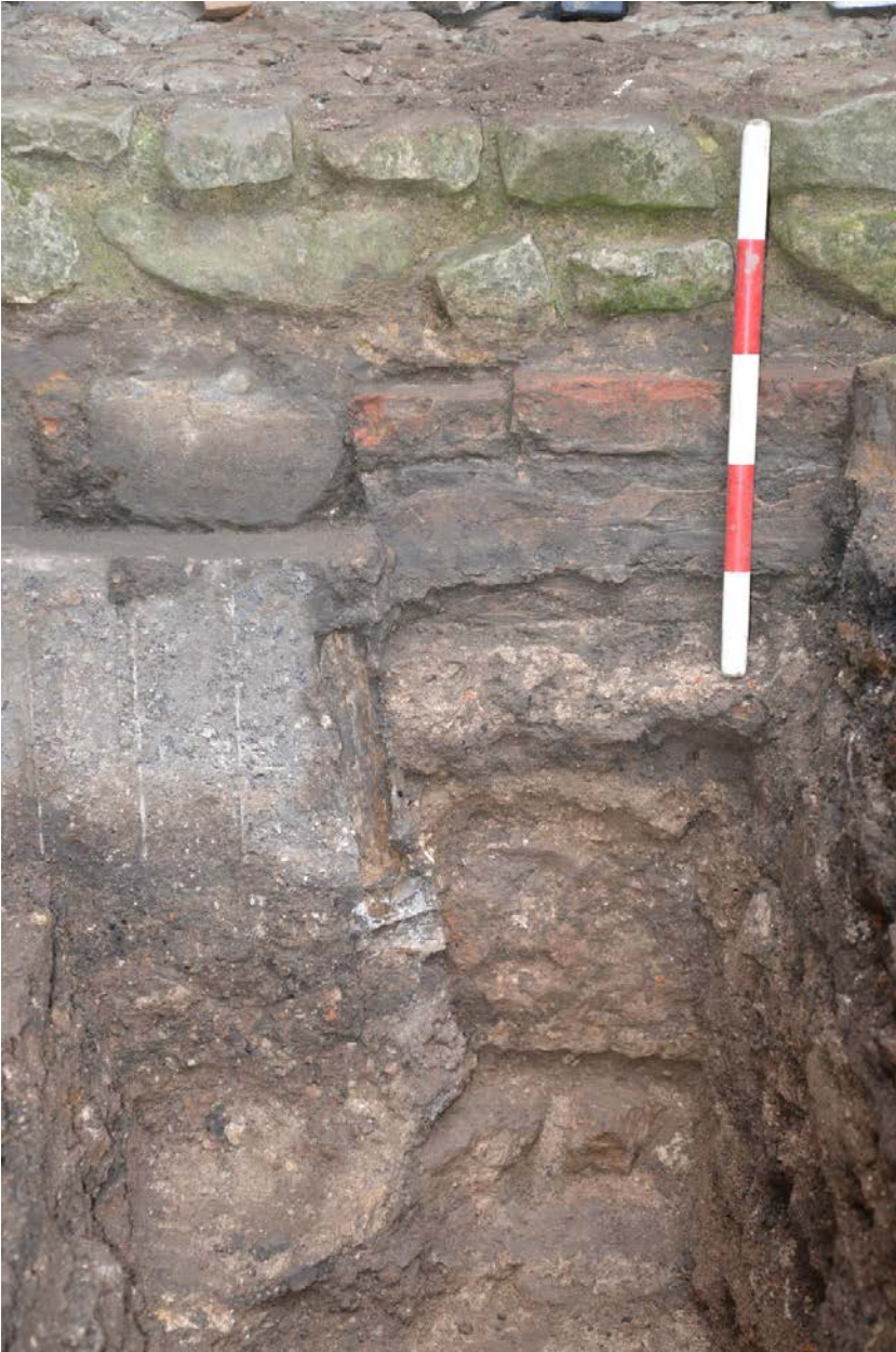
Figure 6 Mortar floor 90218 and wall footing 90219 cut by pit 90209. Source © Historic England, Pr7166-7162.
