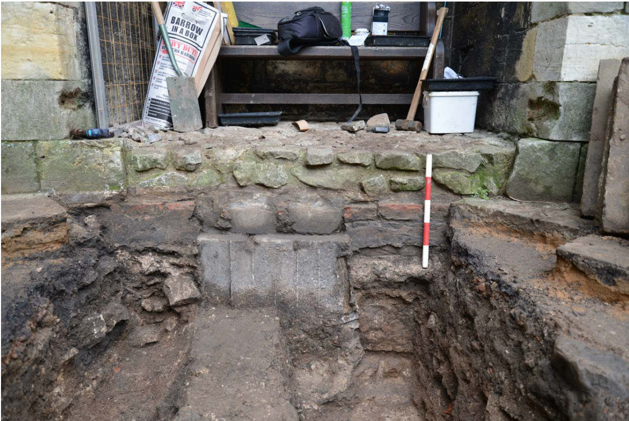
Figure 4 Brick floor 90214 and mortar base 90220. Source © Historic England, Pr7166-7159
