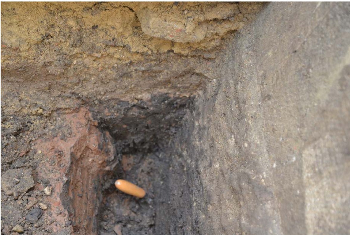
Figure 21 Wall foundation and pink clay subsoil. Source © Historic England Pr7166-7947.
