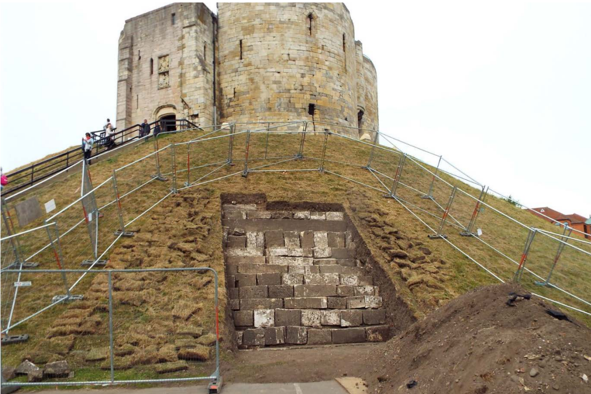
Figure 18 Stepped masonry blocks in Test Pit 9. Source © Historic England Pr7166-7926.
