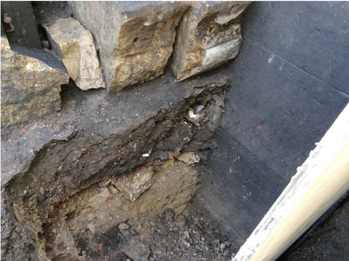
Figure 20 Section through modern backfill against wall. Source © Historic England Pr7166- 7932.
