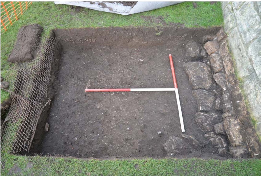
Figure 13 Wall foundations 90405 and sondage. Source © Historic England, Pr7166-7145.
