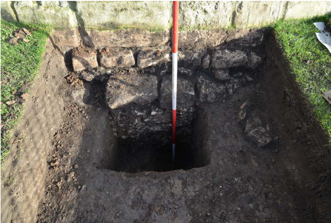
Figure 12 Tower wall foundations 90505 and pebble path 90502. Source © Historic England, Pr7166-7133.
