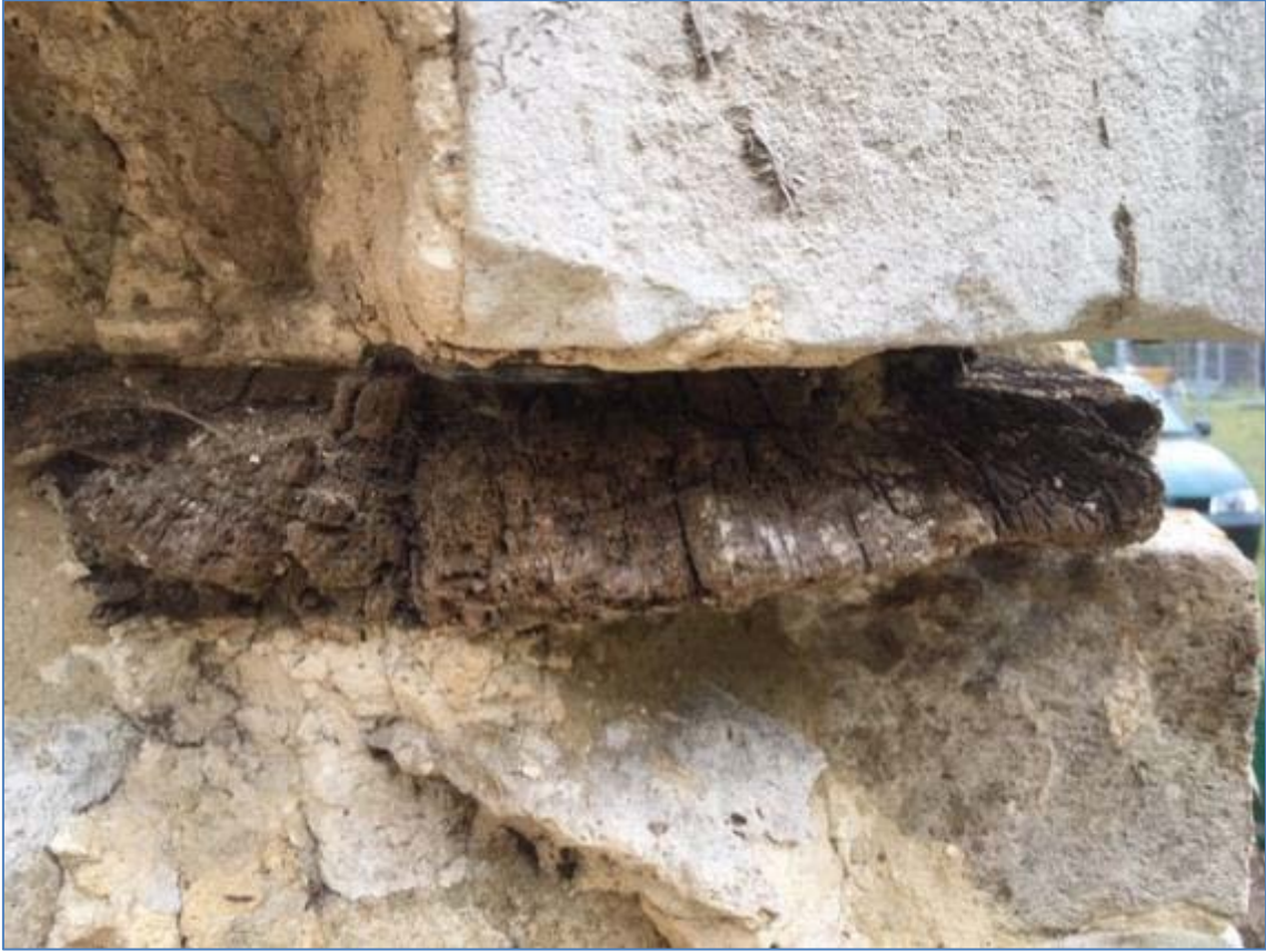
Figure 3: Thin sill timber adjacent to the door, photograph taken from the north (Alison Arnold)
