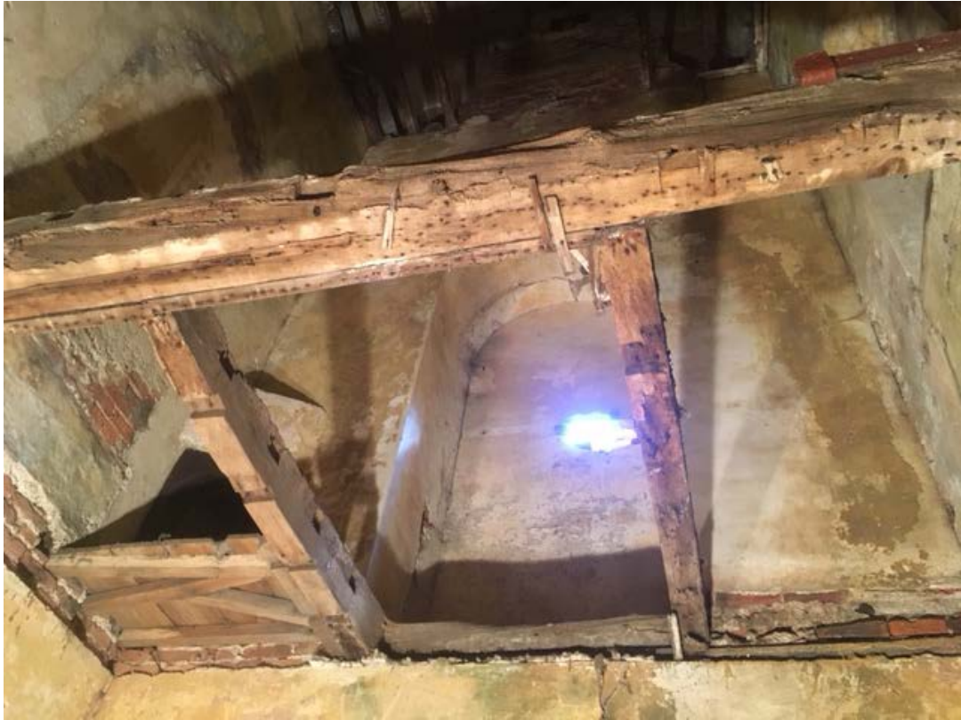
Figure 3: Tower range; surviving floor beams (photograph by Alison Arnold)
