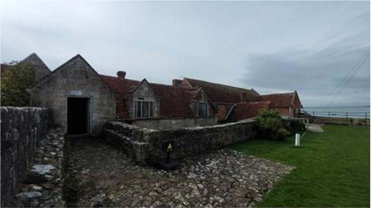
Figure 2: General exterior view of the gabled windows, taken from the gun platform looking south. [photograph Robert Howard]
