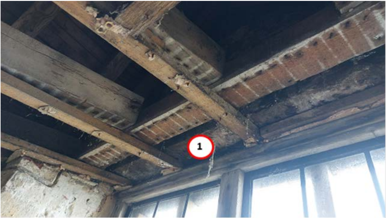
Figure 4: Sampled timber to the east gable window. [photograph Robert Howard]
