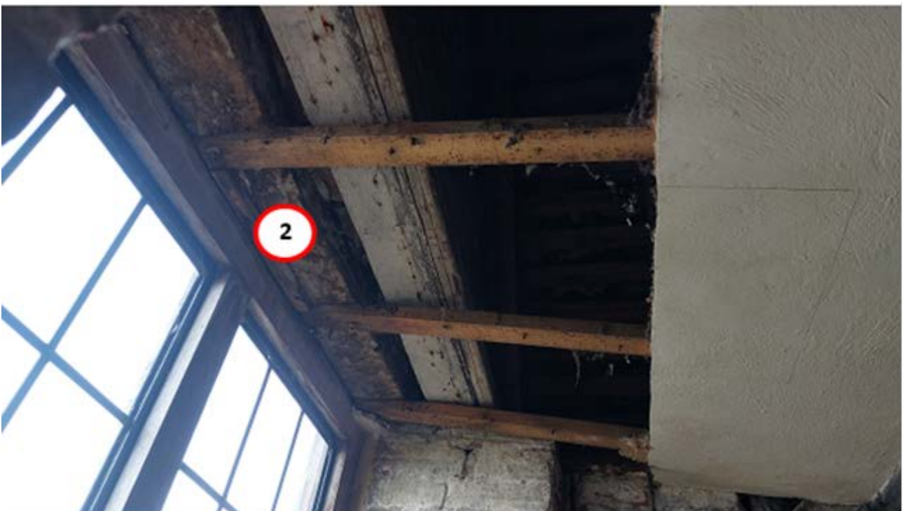
Figure 5: Sampled timber to the west gable window. [photograph Robert Howard]
