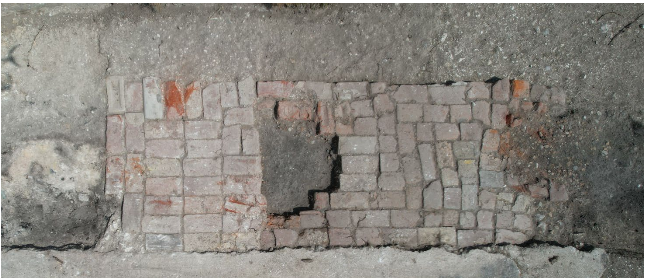
Figure 10: Drone image showing an area of brickwork excavated and cleaned up by the young people.
