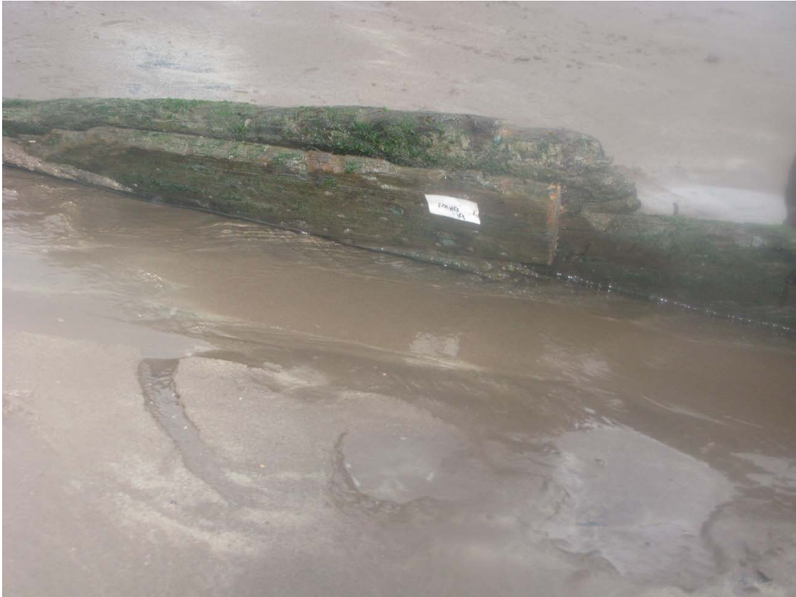
Figure 2: Sampled sheathing timber MBW14 from north-east (photograph by Rod Bale)
