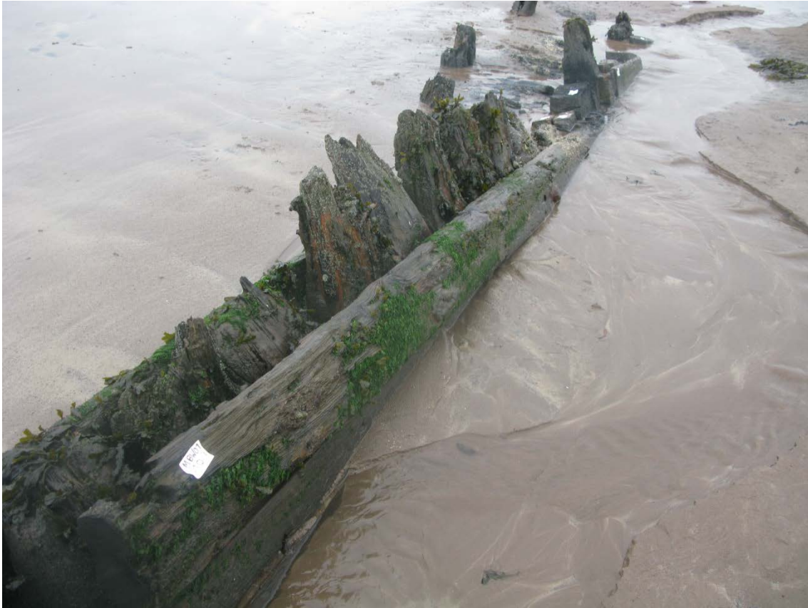
Figure 15: Photograph from south showing sampled stringer MBW10 (tagged timber in foreground), which was sampled at the foreground end. Timbers MBW06, MBW07, and MBW08 are visible at the point where the stringer enters the sand (photograph by Rod Bale)
