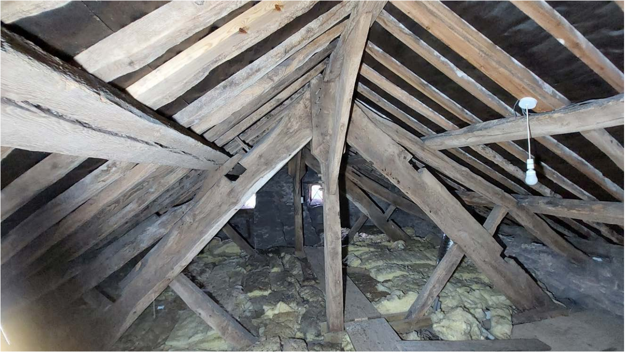
Figure 9: Roof, truss 2, photograph taken from the south. [Alison Arnold]
