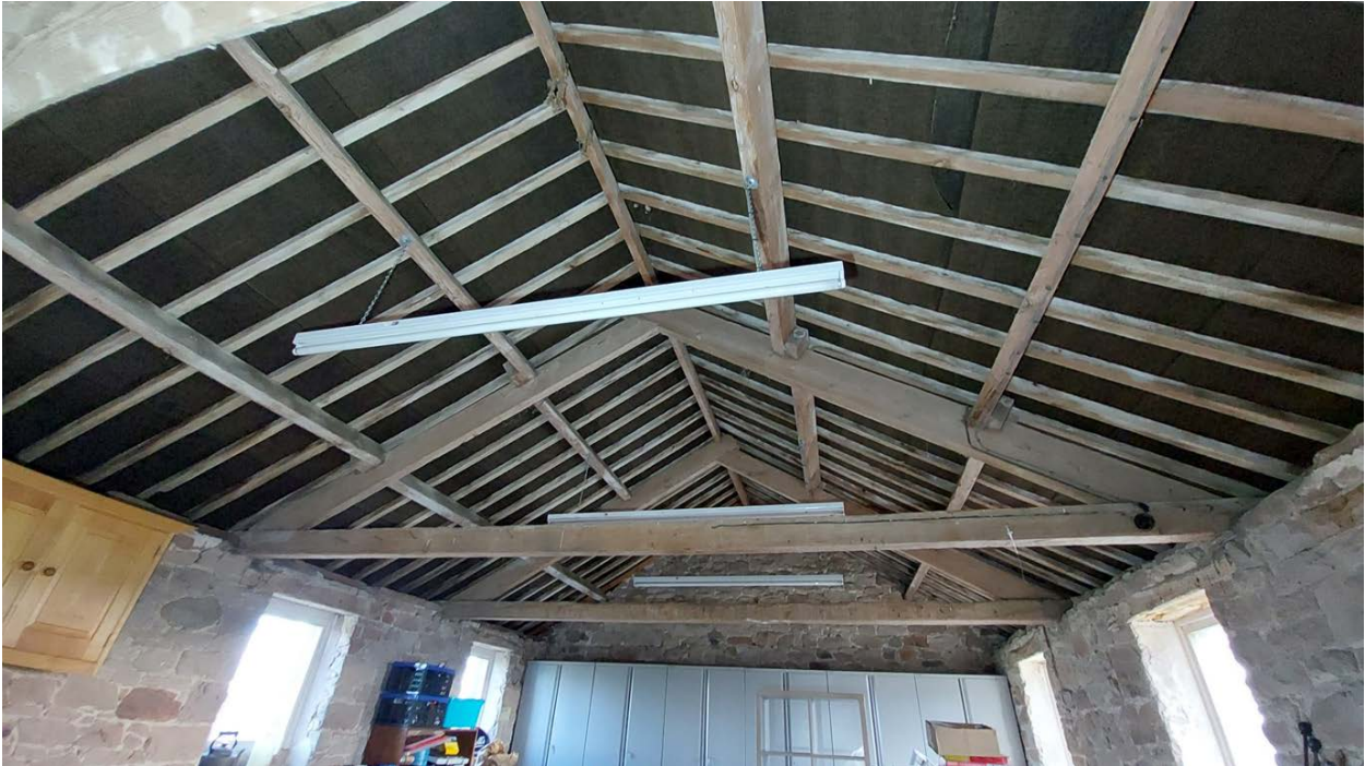
Figure 12: Granary roof, photograph taken from the west. [Alison Arnold]
