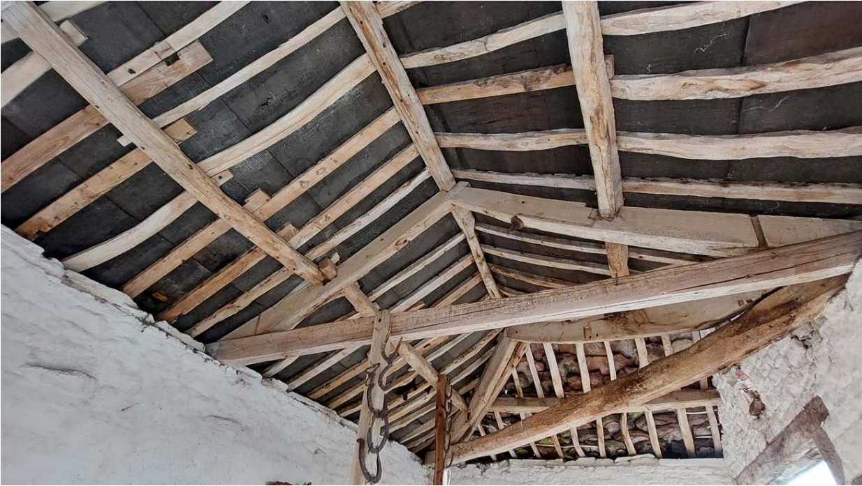
Figure 13: Bottom barn roof, photograph taken from the west. [Alison Arnold]
