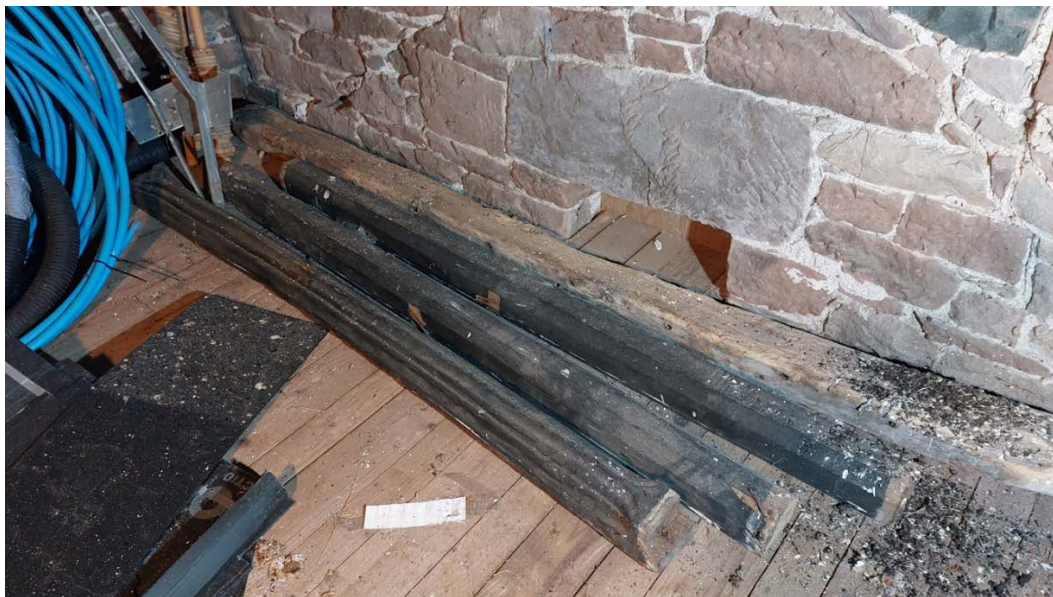
Figure 8: Ex situ joists stored in the granary. [Alison Arnold]
