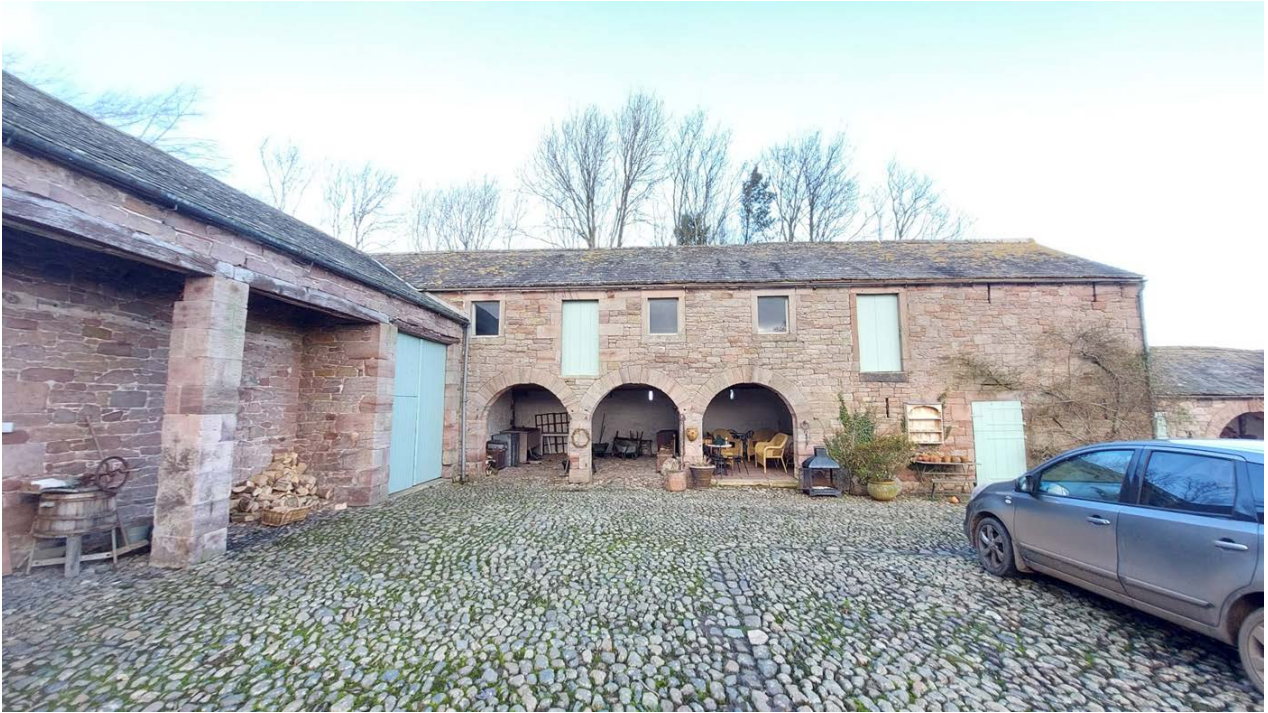
Figure 4: Main barn (left) and granary, photograph taken from the south. [Alison Arnold]
