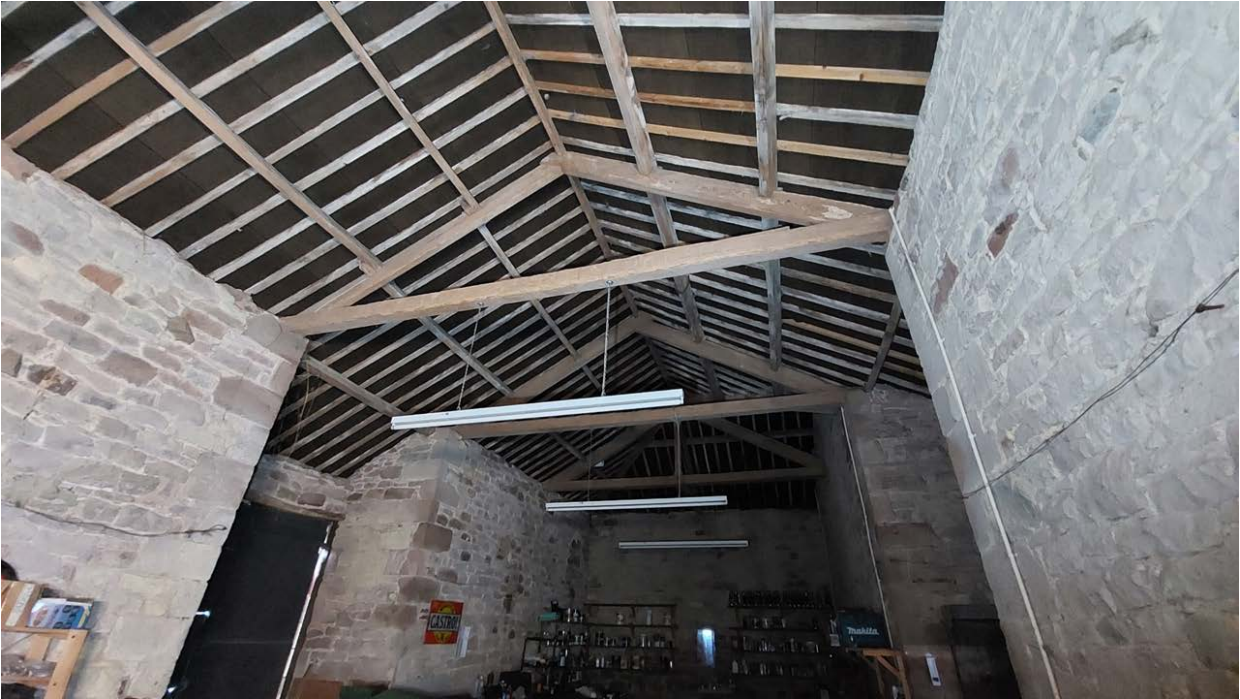
Figure 11: Main barn, roof, photograph taken from the south. [Alison Arnold]
